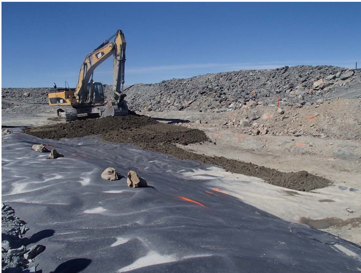
Photograph SD3-338: From Sta. 20+610/-43 m, looking NW. Placement of a first 0.5 m thick lift of compacted sieved till over the LLDPE geomembrane on the upstream toe liner tie-in with an excavator from Sta. 20+588 m to 20+599 m.
