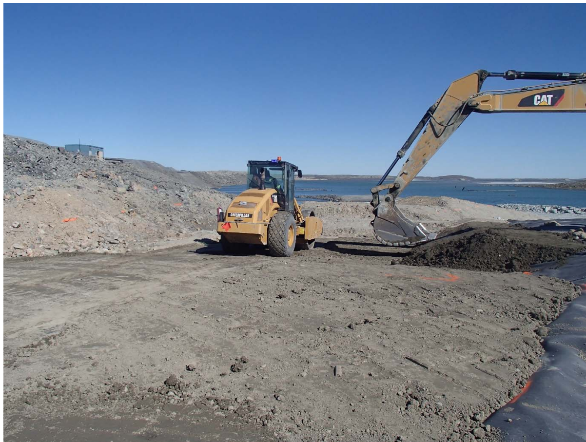
Photograph SD3-339: From Sta. 20+600/-29 m, looking E. Compaction of a first 0.5 m thick lift of compacted sieved till on the upstream toe liner tie-in with an excavator from Sta. 20+588 m to 20+599 m.
