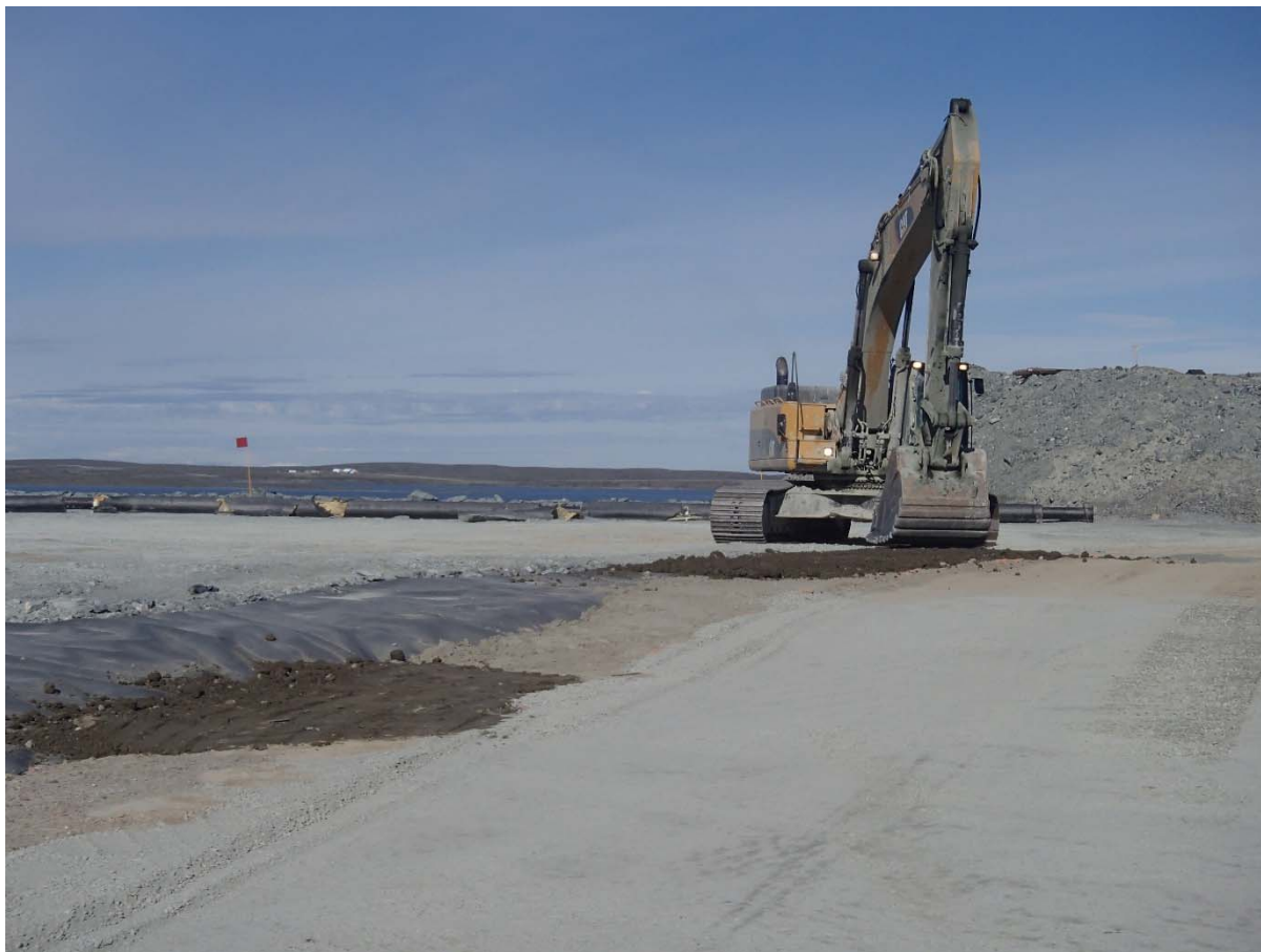
Photograph SD3-352: From Sta. 20+600/-59 m, looking SW. Corrections to the layer of compacted sieved till placed against the upstream slope from Sta. 20+599 m to 20+613 m.
