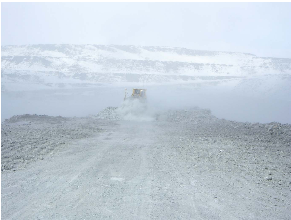
Photograph CD-1800: From Sta. 0+500/-14 m looking N. Placement a 2 m thick (approx.) lift of intermediate volcanic (IV) rockfill from El. 143 m to El. 145 m from 0+435 to 0+535m (o.s. -28 to -18 m).
