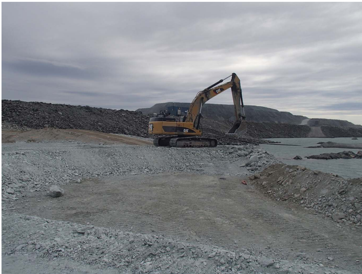
Photograph SD3-347: From Sta. 20+640/-41 m, looking W. Placement of a third 0.5 m thick lift of fine UM rockfill (0-500 mm) upstream of the low quality till (0-150mm) from El. 143 m to 143.5 m from Sta. 20+688 m to 20+619 m.
