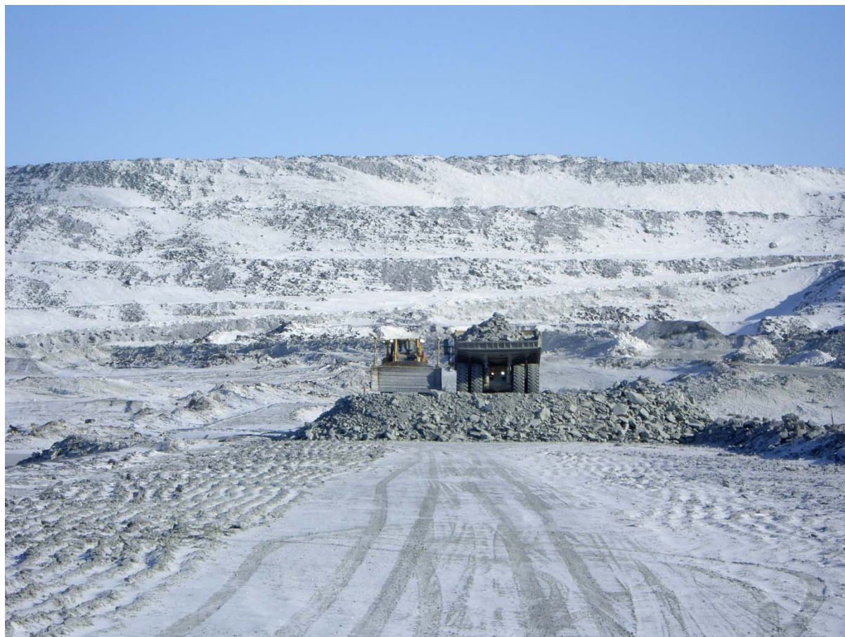
Photograph CD-1798: From Sta. 0+500/-15 m looking N. Placement a 2 m thick (approx.) lift of volcanic rockfill from El. 143 m to El. 145 m from 0+340 to 0+435 m (o.s. -28 to -18 m).
