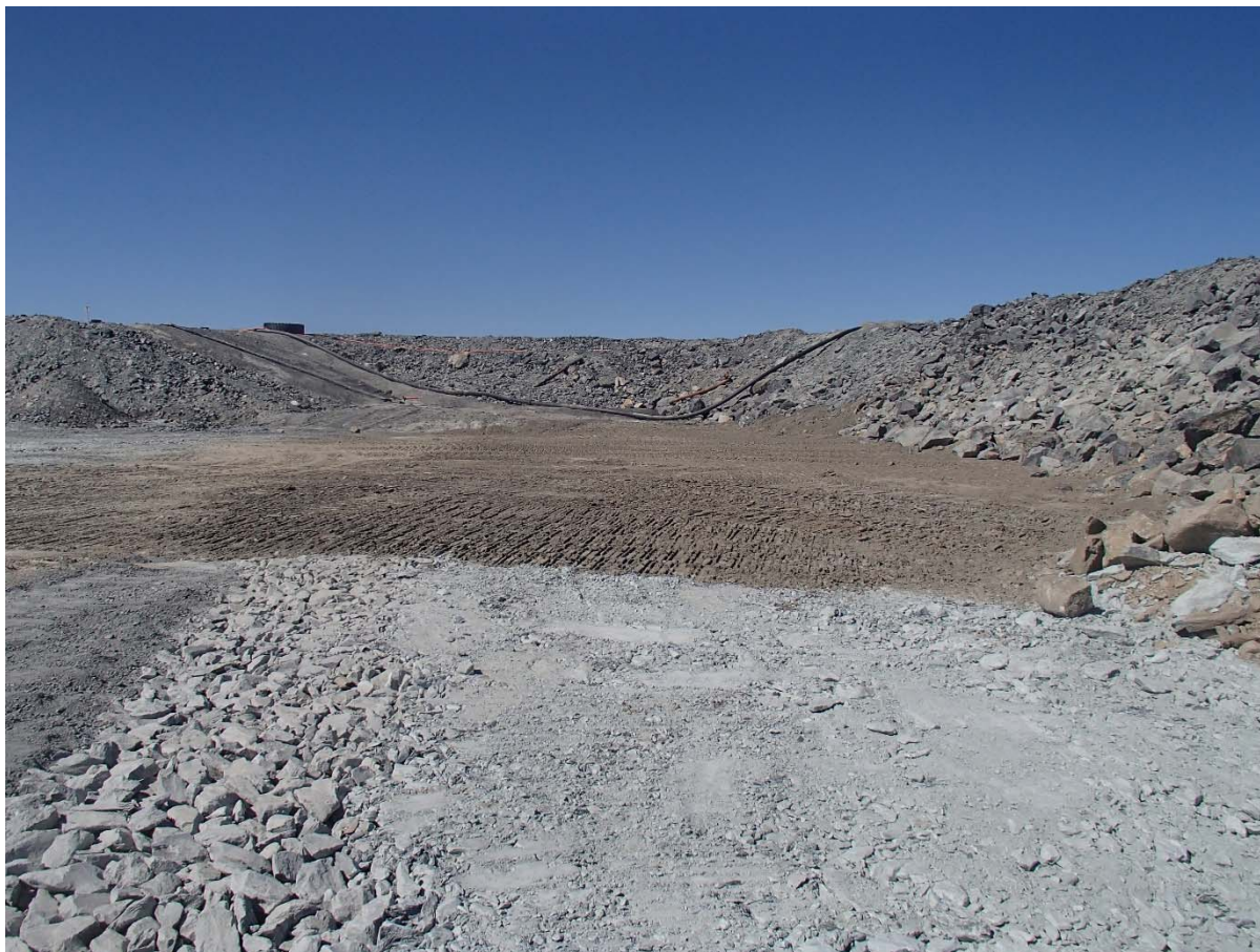
Photograph SD3-343: From Sta. 20+590/-40 m, looking NW. View of the depression between SD2 and SD3 backfilled with low quality till up to El. 145 m.
