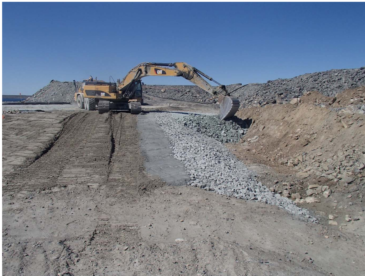
Photograph SD3-341: From Sta. 20+600/-58 m, looking W. Placement of a first 0.5 m thick lift of fine rockfill on the upstream slope of the upstream toe liner tie-in with an excavator from Sta. 20+588 m to 20+599 m.
