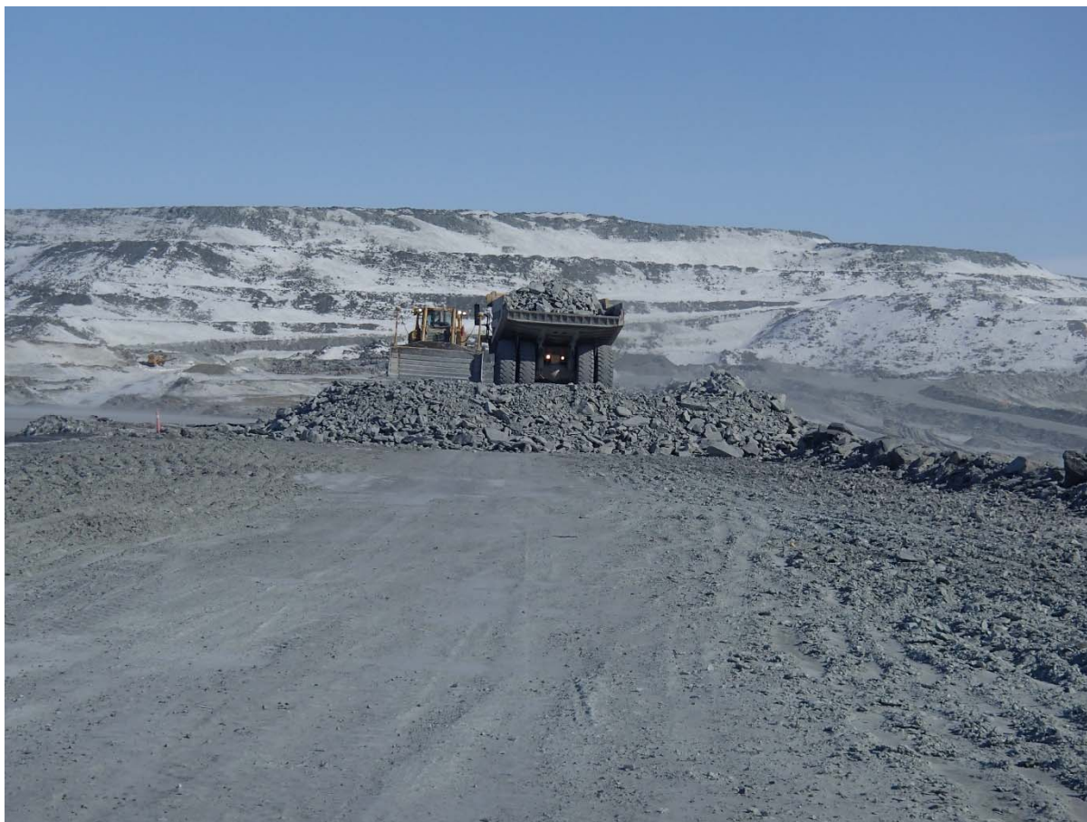
Photograph CD-1802: From Sta. 0+770/-16 m looking N. Placement a 2 m thick (approx.) lift of intermediate volcanic (IV) rockfill from El. 143 m to El. 145 m from approx. Sta. 0+525 to 0+710 m (o.s. -28 to -18 m).
