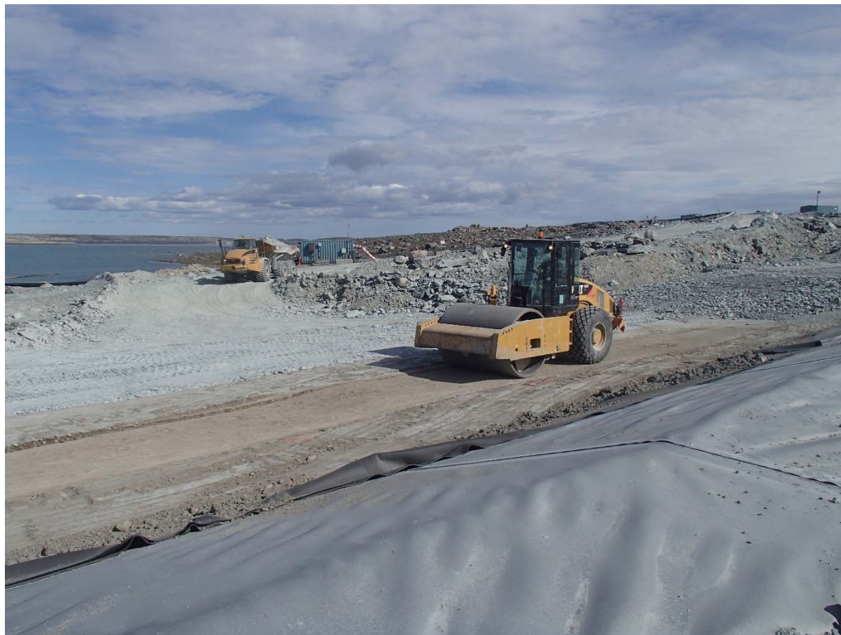
Photograph SD3-351: From Sta. 20+740/-24 m, looking SE. Compaction of the 0.5 m lift of low quality till (0-150 mm) at El. 143.5 m with a 10-tonne smooth-drum compactor with vibration (4 passes) from Sta. 20+619 m to 20+777 m.
