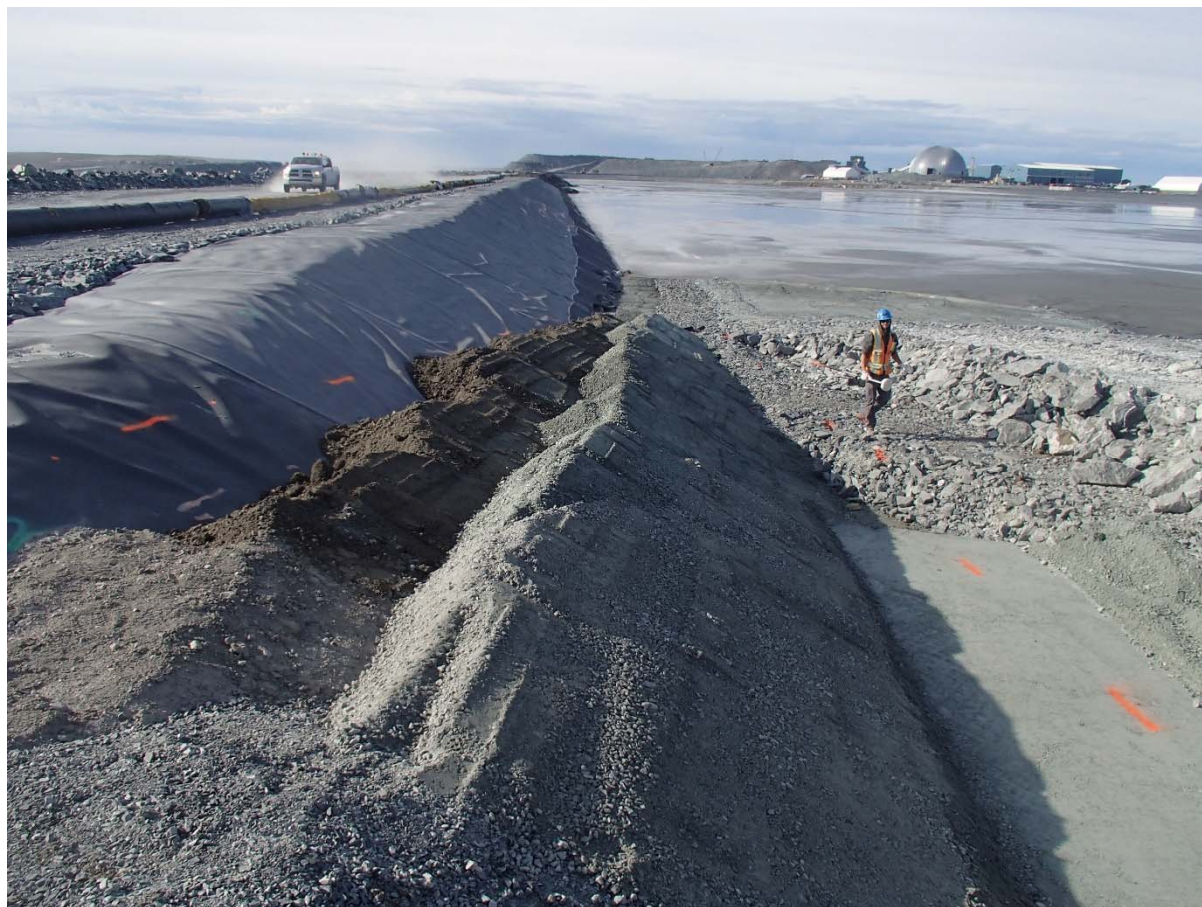
Photograph CD-1896: From Sta. 0+140/-30 m, looking S. Placement of 0.5 m thick layers of compacted sieved till and fine filter on the upstream slope of Central Dike with an excavator from Sta. 0+147 m to 0+177 m.
