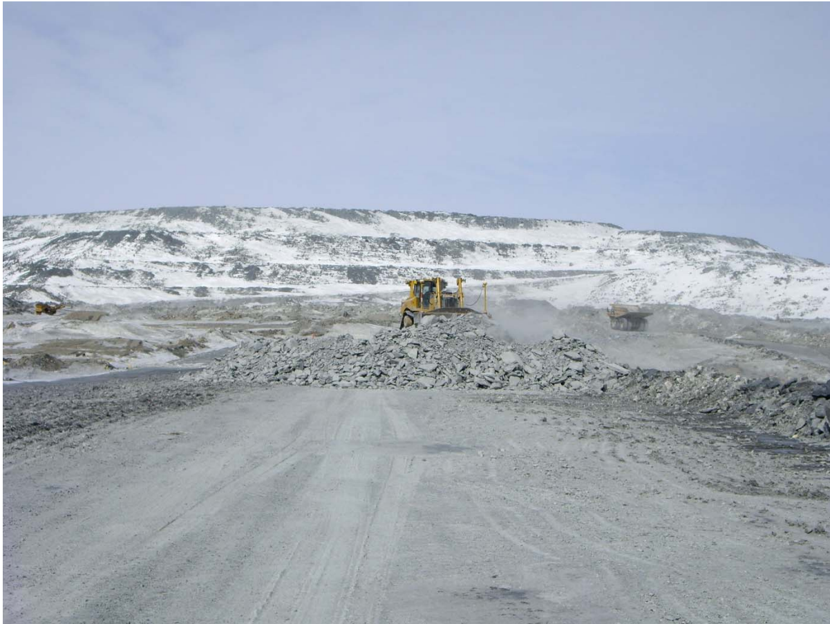
Photograph CD-1797: From Sta. 0+320/-20 m looking N. Placement a 2 m thick (approx.) lift of volcanic rockfill from El. 143 m to El. 145 m from 0+250 to 0+400 m (o.s. -28 to -18 m).
