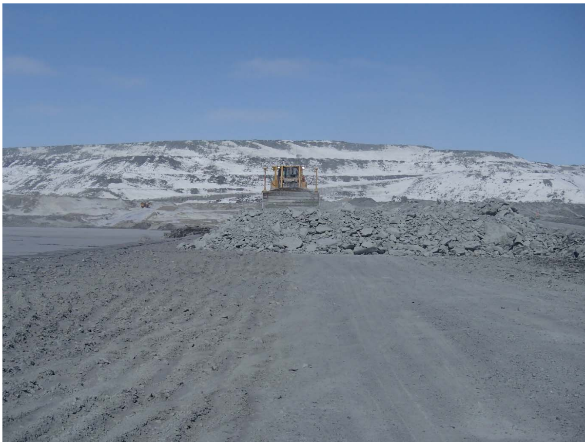
Photograph CD-1801: From Sta. 0+650/-10 m looking N. Placement a 2 m thick (approx.) lift of intermediate volcanic (IV) rockfill from El. 143 m to El. 145 m from 0+535 to 0+625m (o.s. -28 to -18 m).
