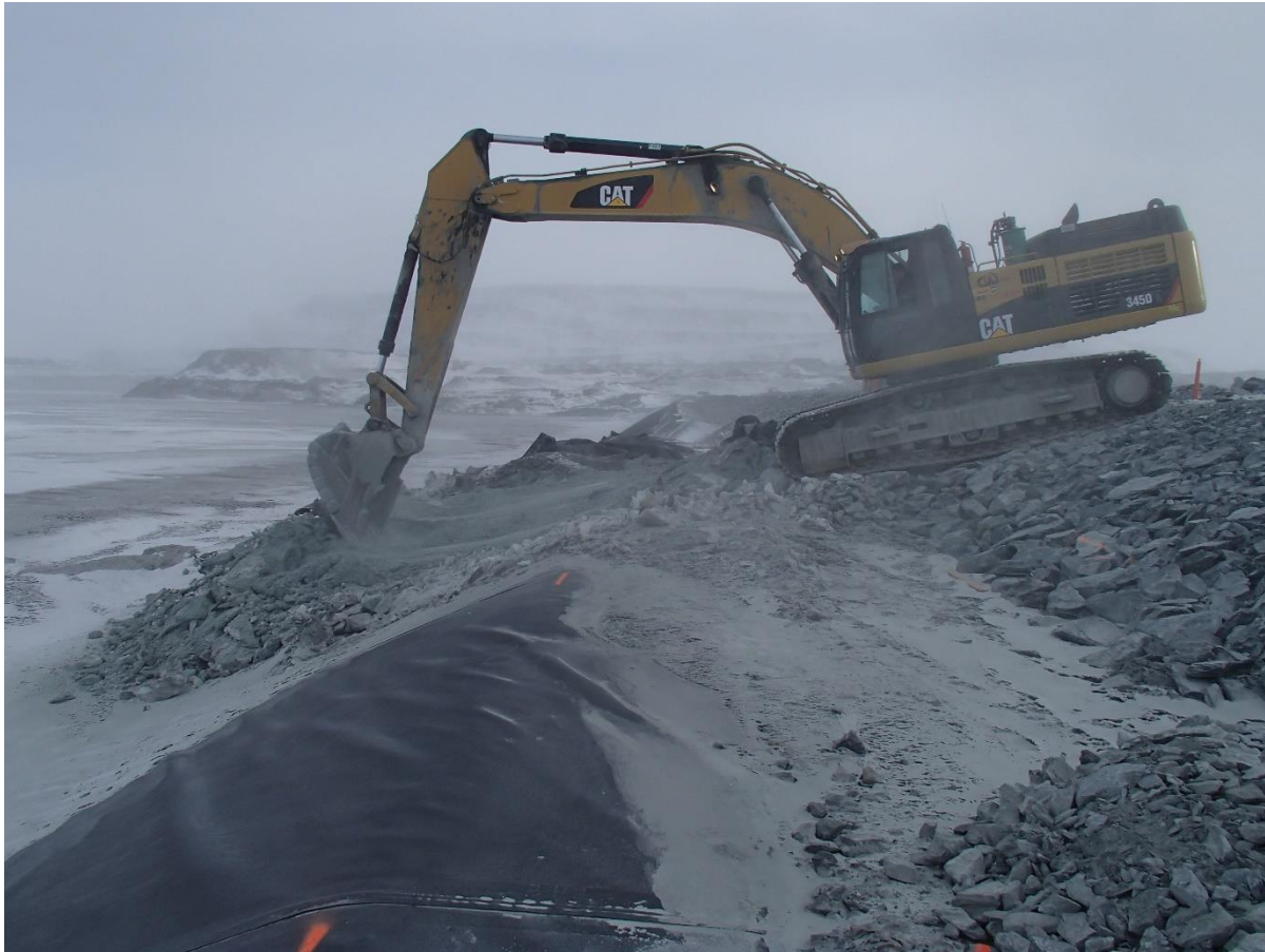
Photograph CD-1830: From Sta 0+420/-26 m, looking N. Removal of the deposition point finger materials with an excavator at Sta. 0+390 m.
