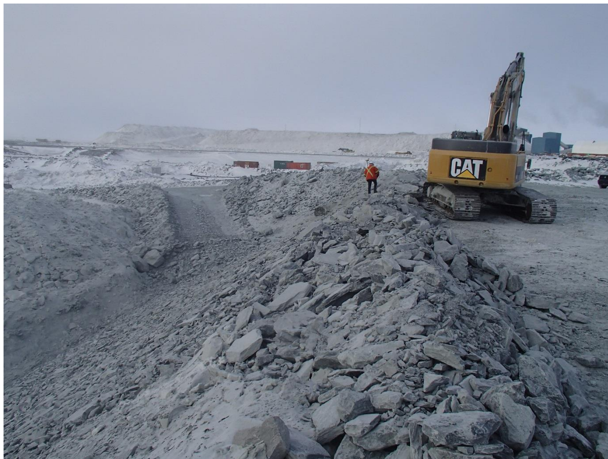
Photograph CD-1813: From Sta. 0+980/-2, looking S. Placement of intermediate volcanic (IV) rockfill on the existing downstream slope up to approx. El. 143 m, from approx. Sta. 0+980 to 40+780 m.
