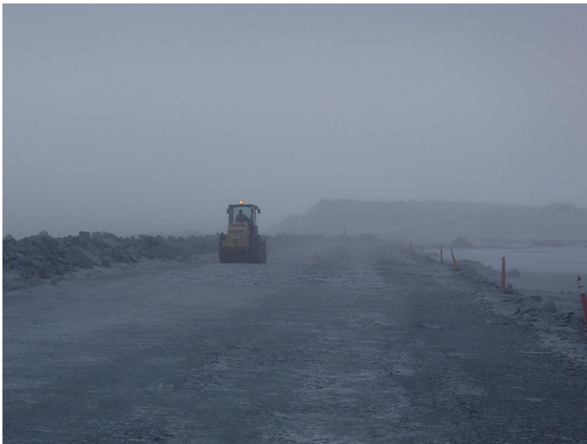
Photograph CD-1810: From Sta. 0+335/-15 m looking S. Compaction of the 2 m lift (approx.) of IV rockfill at El. 145 m with a 10-tonne smooth-drum compactor with vibration (6 passes) from Sta. 0+350 to 0+540 m (o.s. -19 to -7 m).
