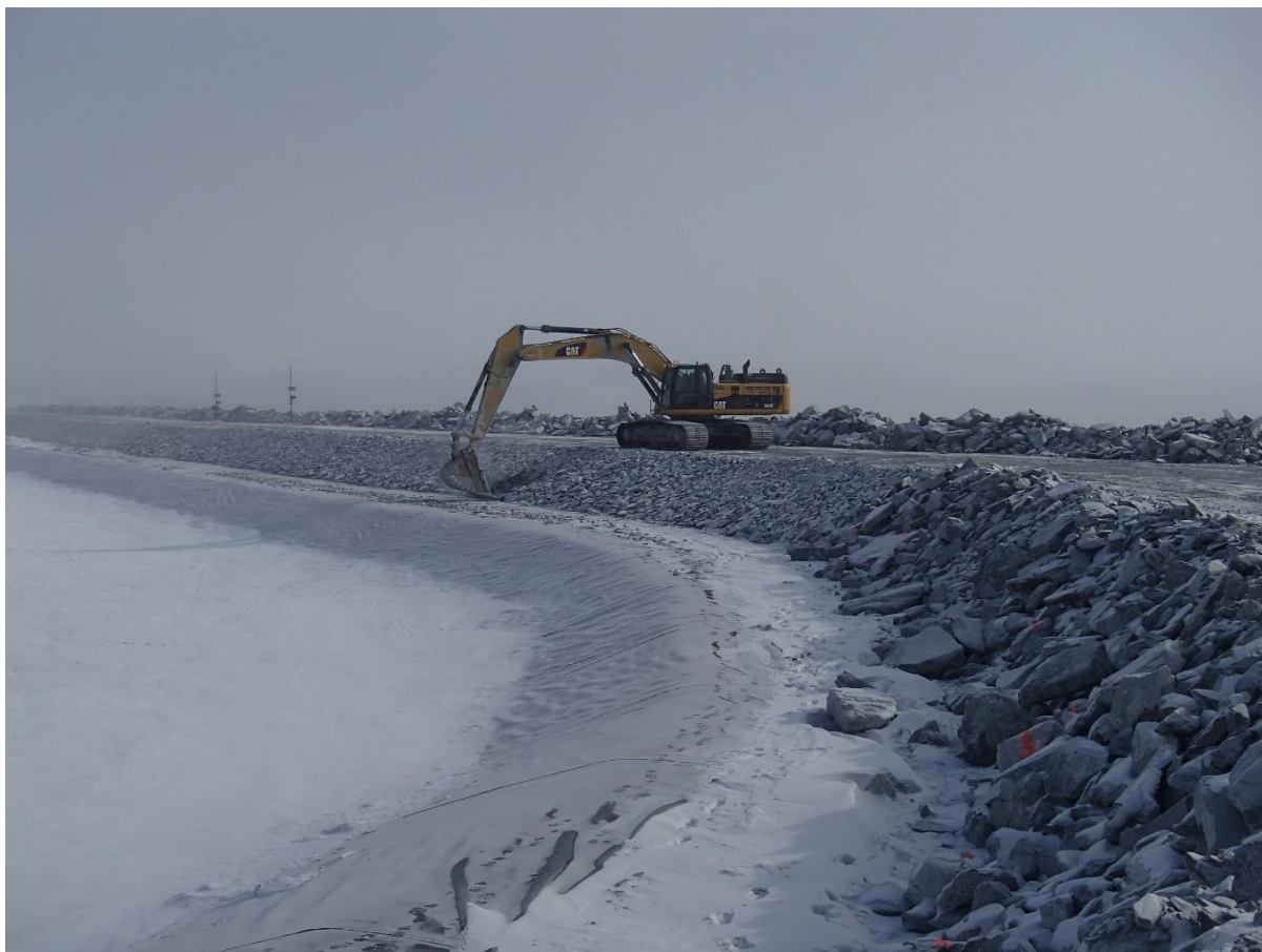
Photograph CD-1824: From Sta 40+760/-25 m, looking NE. Profiling of the upstream slope (2H:1V) from El. 143 to 145 m with an excavator between Sta. 0+830 m and 40+730 m.
