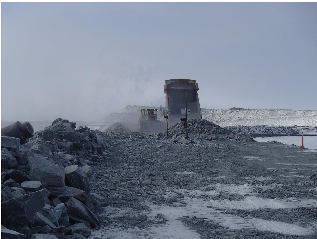
Photograph CD-1820: From Sta. 0+790/-7, looking S. Placement of a 2 m thick (approx.) lift of intermediate volcanic (IV) rockfill from El. 143 m to El. 145 m from approx. Sta. 0+880 m to 0+830 m (o.s. -28 to -11 m).
