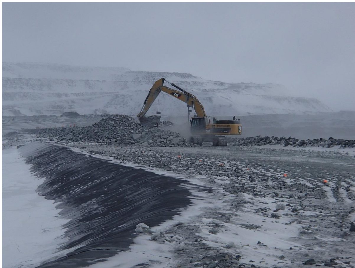
Photograph CD-1814: From Sta. 0+970/-10, looking NE. Placement of intermediate volcanic (IV) rockfill around the instruments at approx. Sta. 0+830 m with the excavator.
