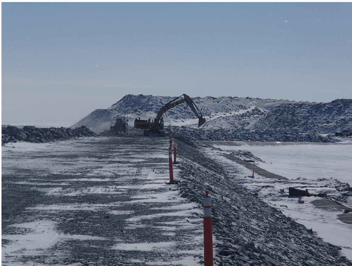
Photograph CD-1819: From Sta. 0+560/-21, looking S. Profiling of the upstream slope (2H:1V) from El. 143 to 145 m with an excavator between Sta. 0+560 m and 0+830 m.
