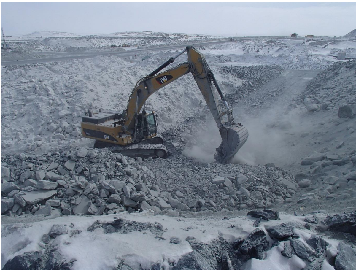
Photograph CD-1812: From Sta. 0+985/-11 m looking SE. Placement of intermediate volcanic (IV) rockfill on the existing downstream slope up to approx. El. 140 m, from approx. Sta. 0+985 to 40+780 m.
