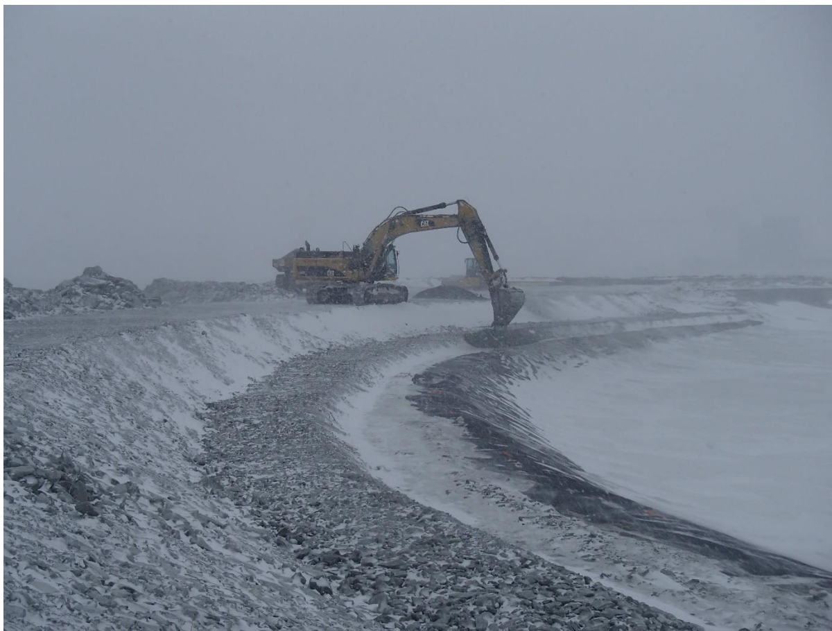
Photograph CD-1827: From Sta 0+940/-16 m, looking SW. Placement of a 0.5 m thick lift of fine filter from El. 143 m to 143.5 m with an excavator from Sta. 40+730 m to 0+ 835 m.
