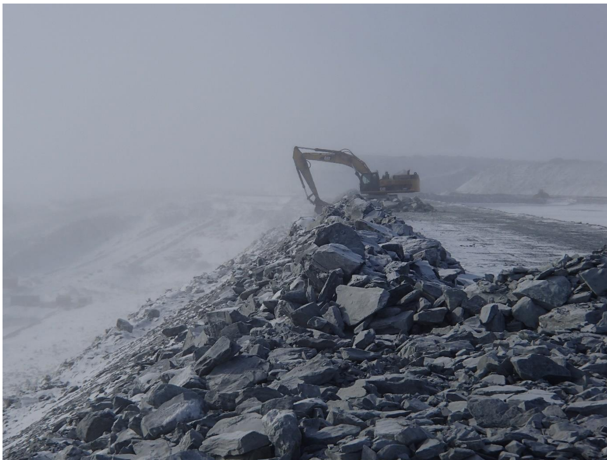
Photograph CD-1825: From Sta 0+430/+9 m, looking S. Profiling of the downstream slope (1.5H:1V) from El. 143 to 145 m with an excavator between Sta. 0+330 m and 0+440 m and between Sta. 0+530 m and 0+745 m.
