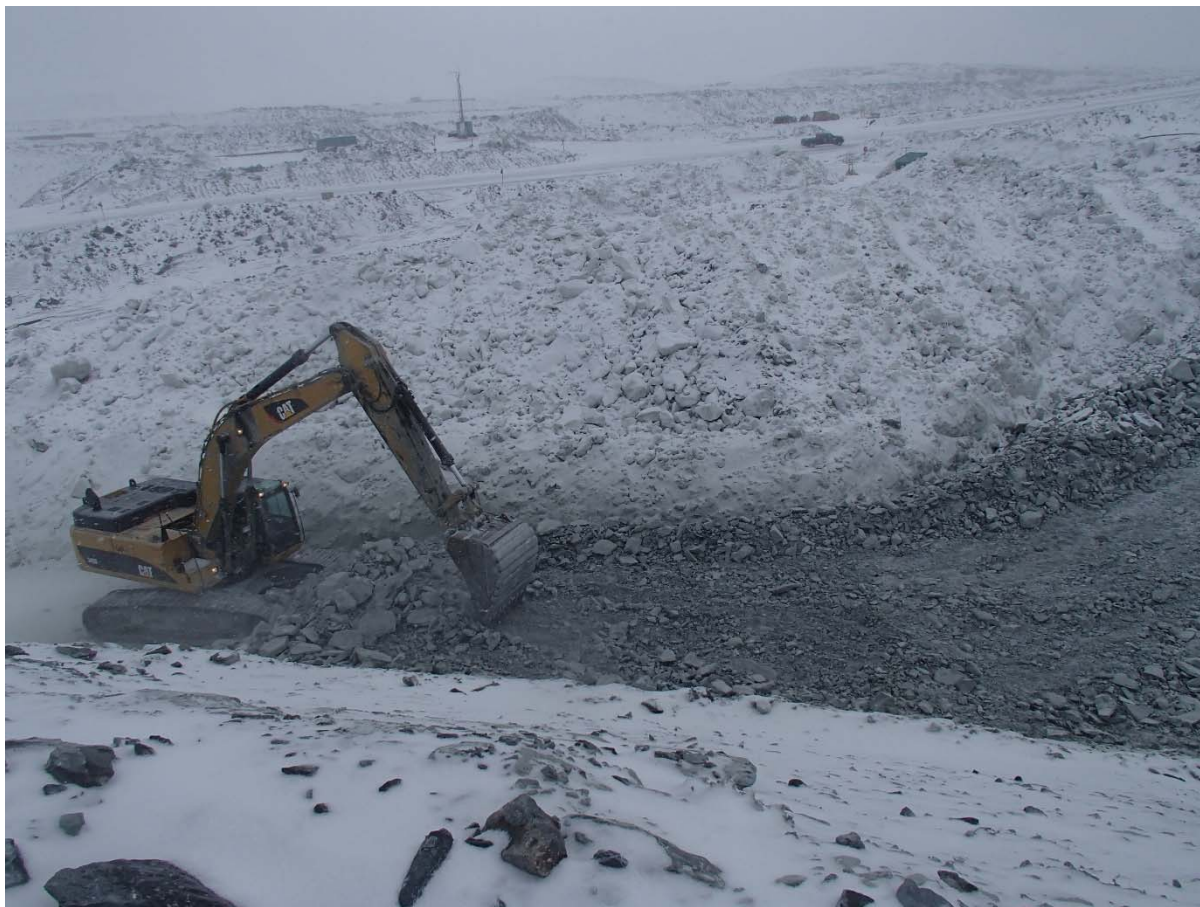
Photograph CD-1808: From Sta. 40+790/-14 m looking E. Placement a 1.5 m thick (approx.) lift of intermediate volcanic (IV) rockfill from approx. Sta. 40+780 to 40+805 m (o.s. -6 to 9 m).
