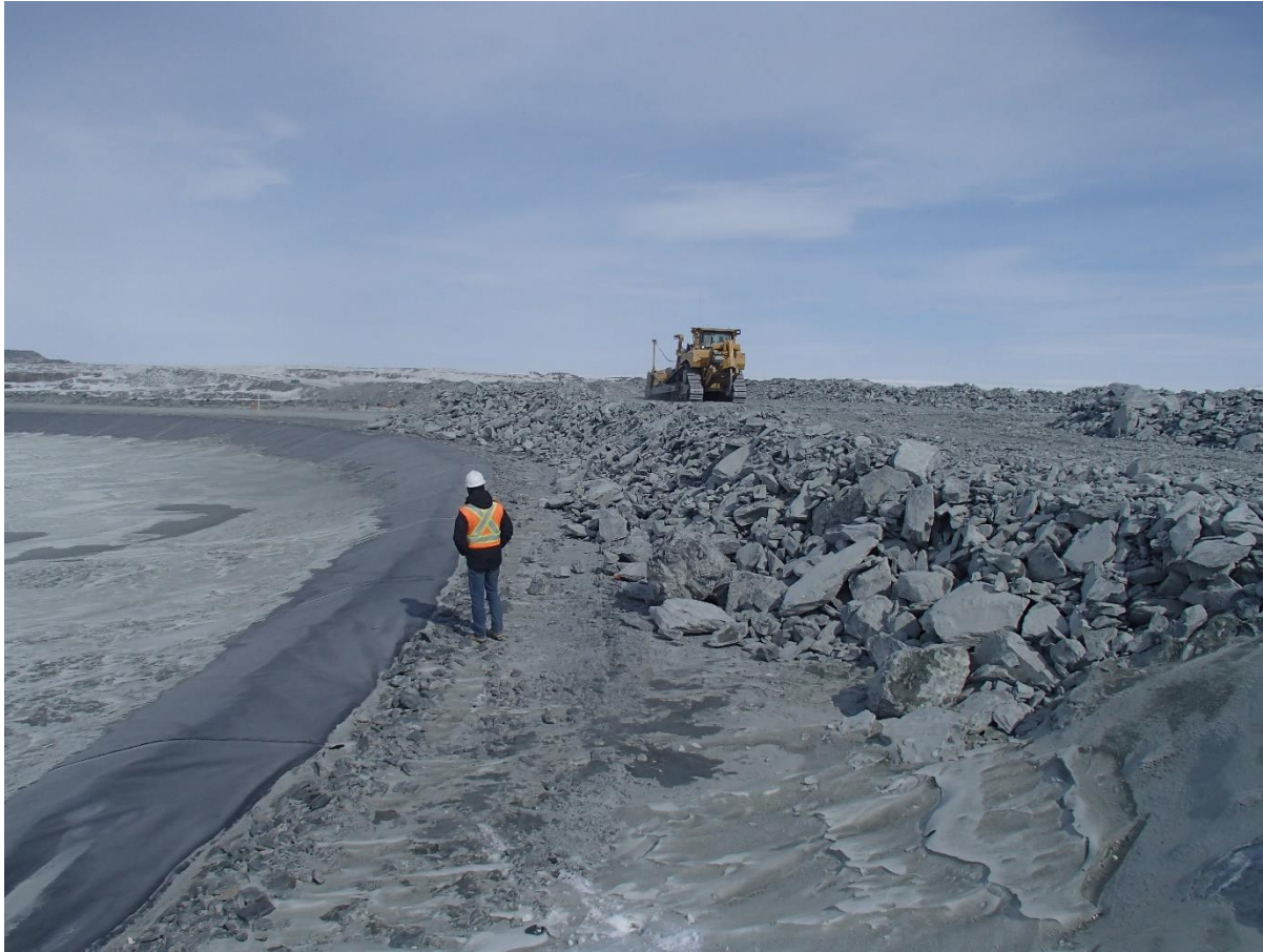
Photograph CD-1817: From Sta. 40+700/-10, looking NE. View of the rockfill lift thickness at the junction of Saddle Dam 5 and Central Dike, approx. 2.5 m thick.
