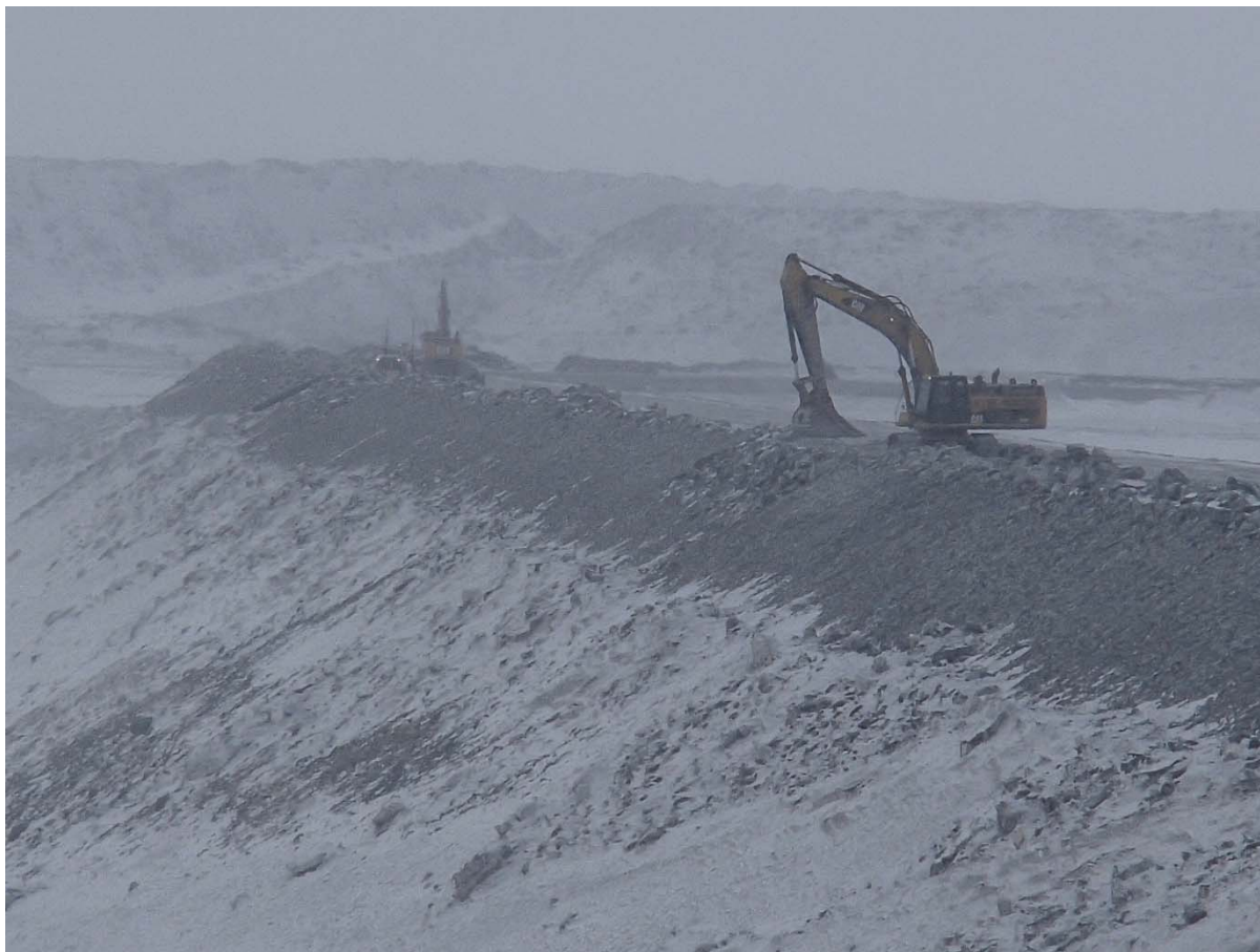
Photograph CD-1850: From Sta. 0+160/+20 m, looking SW. Profiling of the downstream slope (1.5H:1V) from El. 143 to 145 m with an excavator between Sta. 0+440 m and 0+530 m and between Sta. 0+745 m and 0+835 m.
