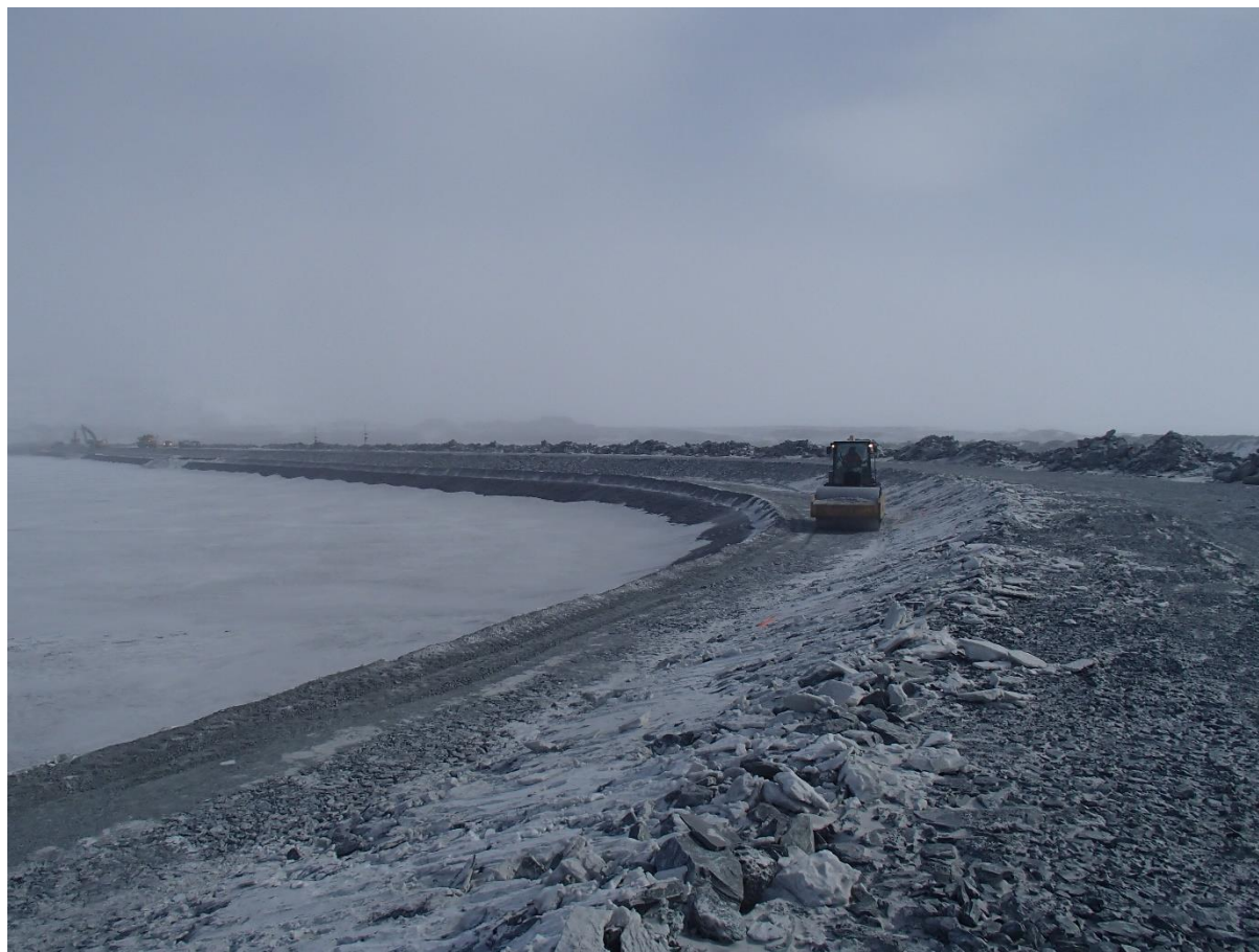
Photograph CD-1831: From Sta 40+730/-24 m, looking NE. Compaction of the first 0.5 m lift (approx.) of fine and coarse filters material at El. 143.5 m with a 10-tonne smooth-drum compactor with vibration (6 passes) from Sta. 40+730 m to 0+830 m and from Sta. 0+175 m to 0+490 m.
