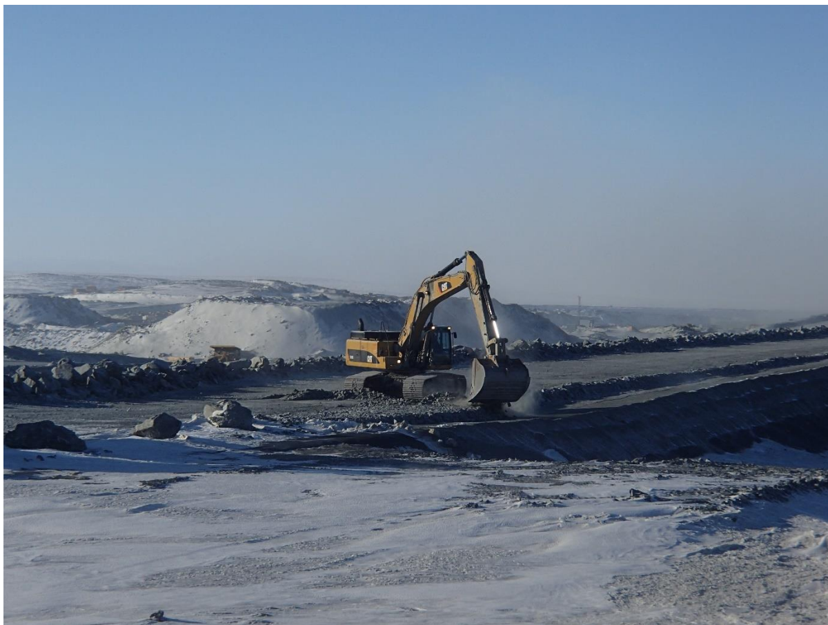
Photograph CD-1844: From Sta 0+080/-49 m, looking SW. Placement of a fourth 0.5 m thick lift of coarse filter from El. 144.5 m to 145 m with an excavator from Sta. 0+170 m to 40+730 m.
