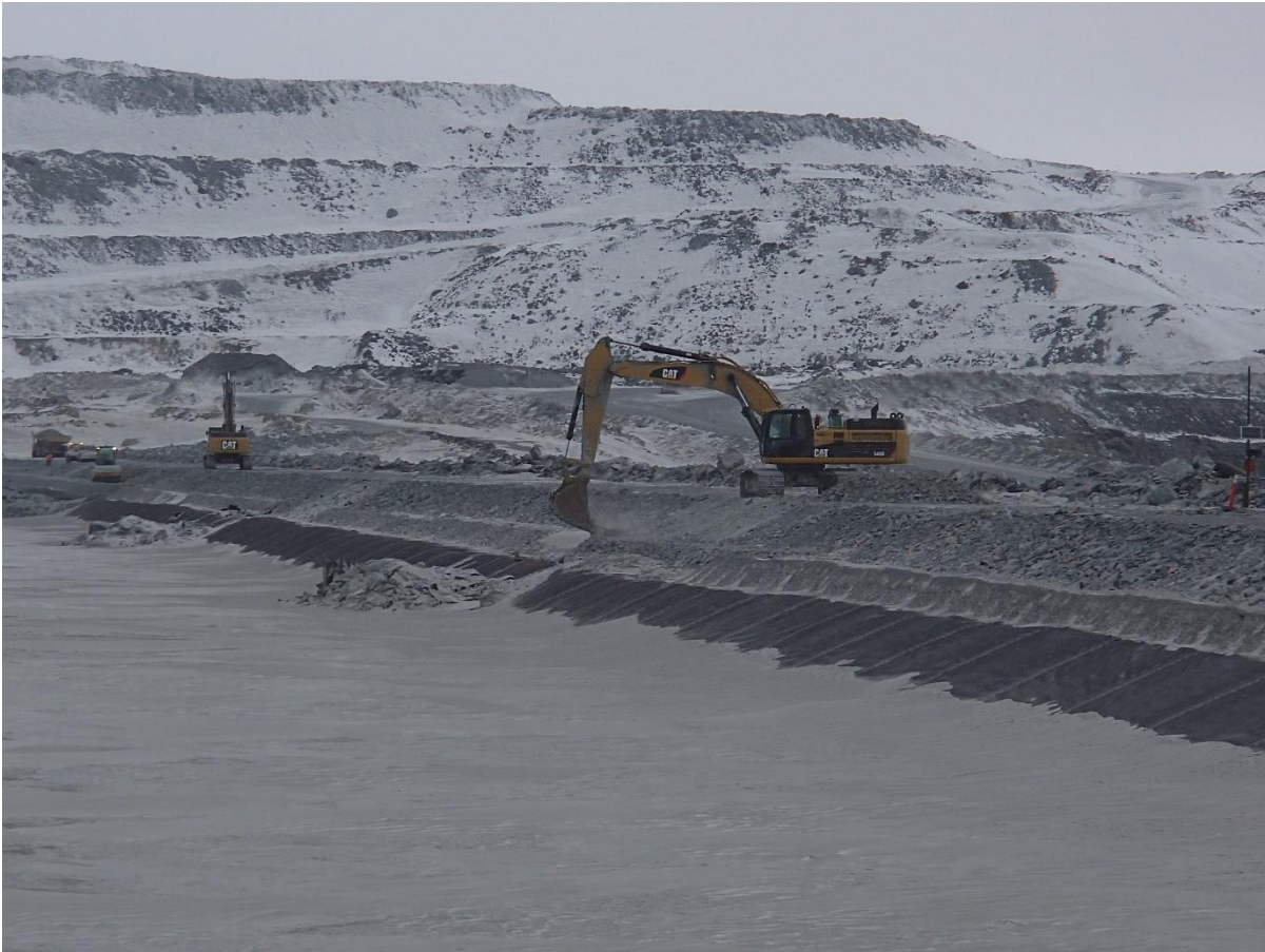
Photograph CD-1834: From Sta 40+760/-23 m, looking NE. Placement of a first 0.5 m thick lift of coarse filter from El. 143 m to 143.5 m on length of approx. 5 m with an excavator at the location of the deposition finger at Sta 0+520 m and 0+660 m.
