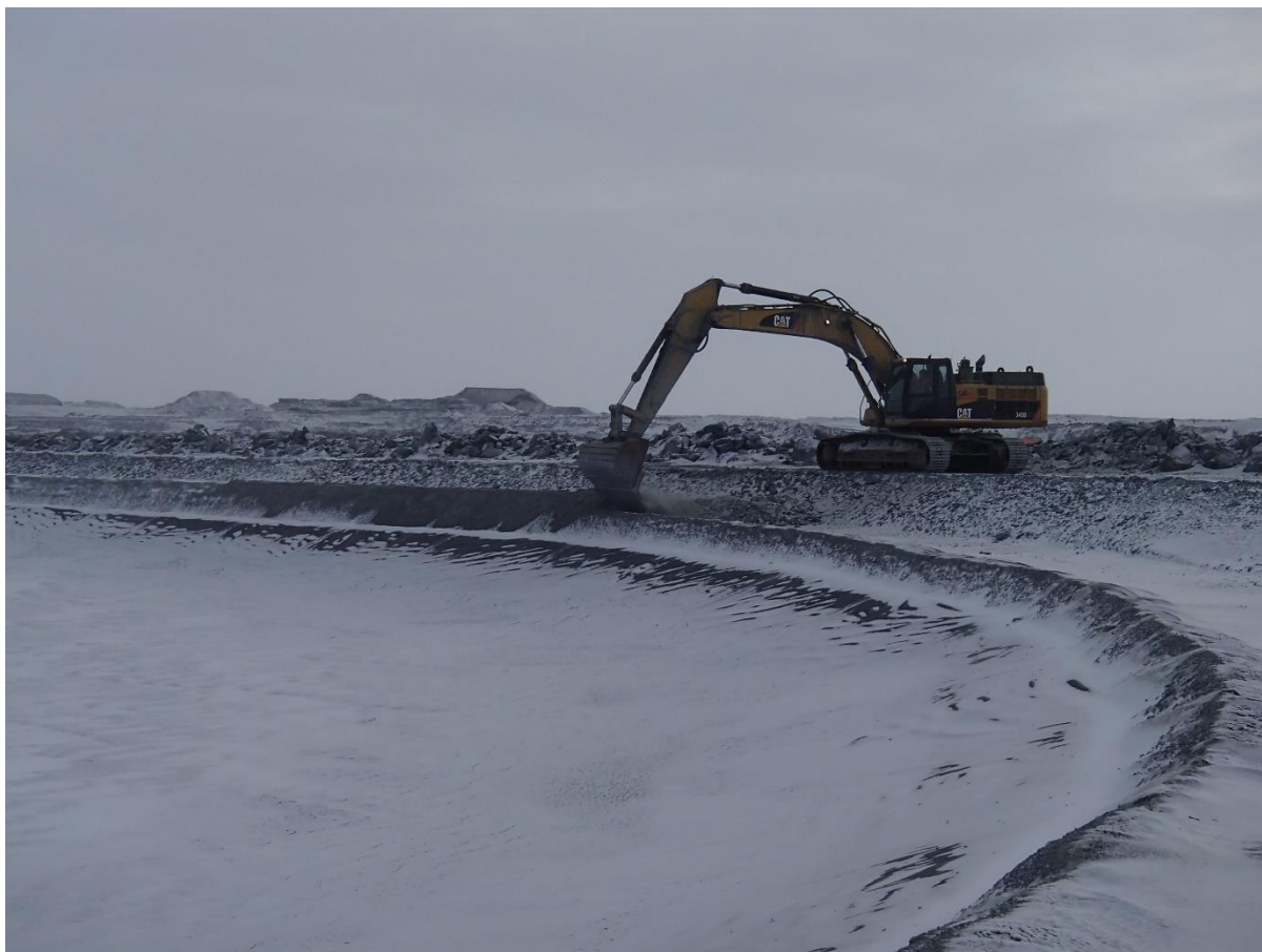
Photograph CD-1838: From Sta 40+750/-31 m, looking NE. Placement of a second 0.5 m thick lift of fine filter from El. 143.5 m to 144 m upstream of the coarse filter with an excavator from Sta. 0+500 m to 0+835 m and from 0+930 to 40+730 m.
