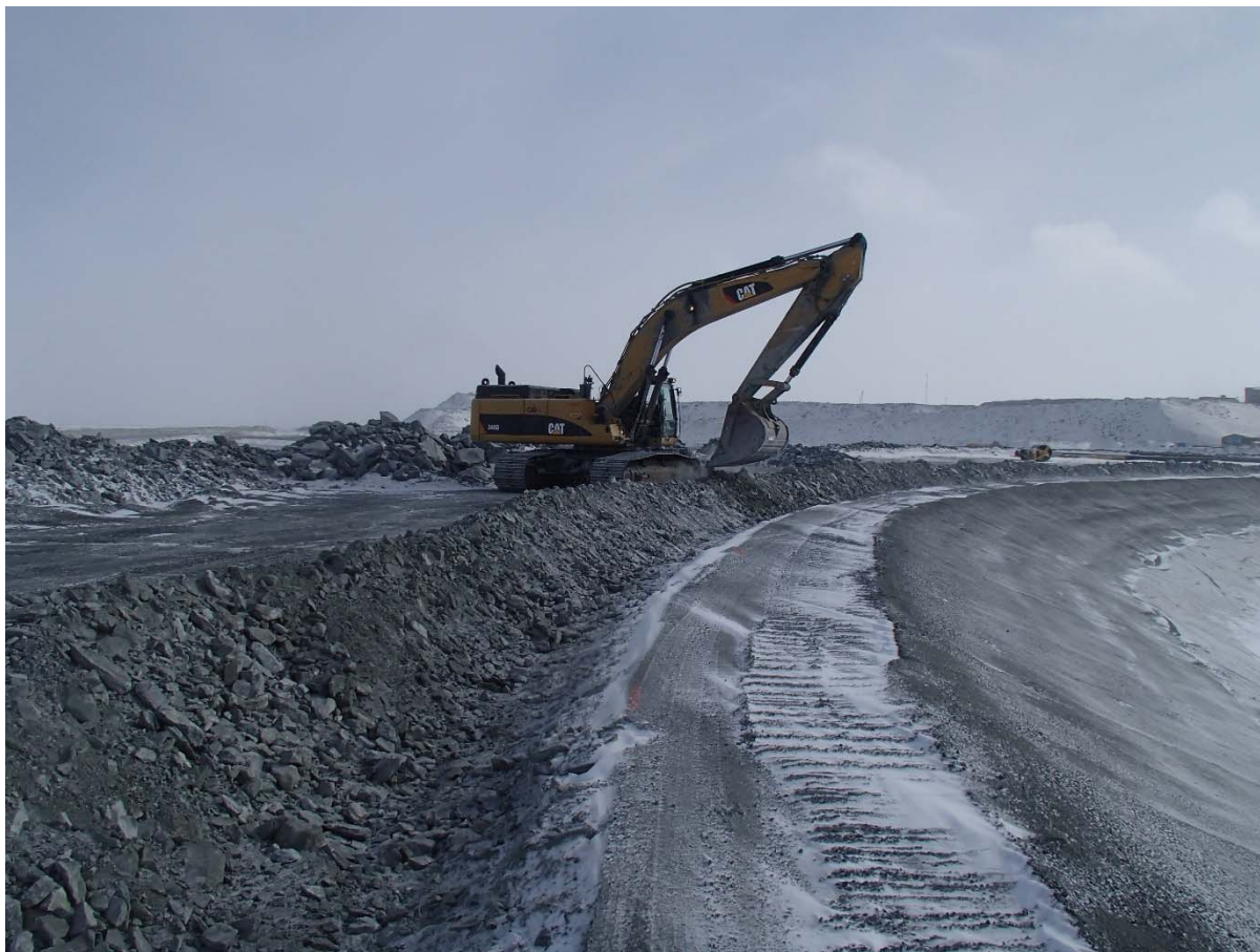
Photograph CD-1851: From Sta. 0+910/-18 m, looking S. Excavation of the LLDPE geomembrane crest anchoring trench from Sta. 40+730 m to 0+830 m.
