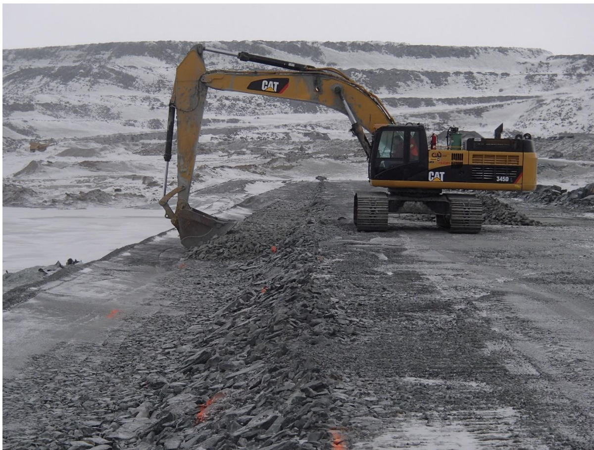
Photograph CD-1841: From Sta 0+475/-14 m, looking N. Placement of a third 0.5 m thick lift of coarse filter from El. 144 m to 144.5 m with an excavator from Sta. 0+335 m to 40+730 m.
