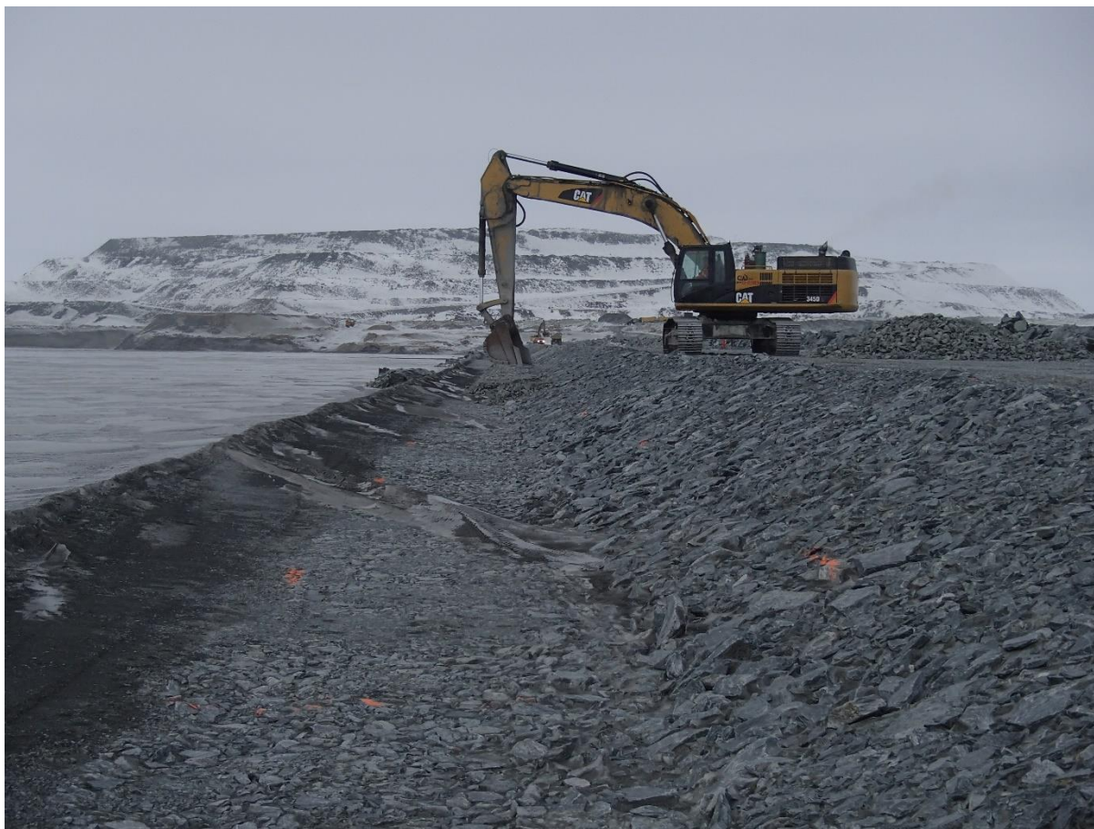
Photograph CD-1837: From Sta 0+940/-25m, looking N. Placement of a second 0.5 m thick lift of coarse filter from El. 143.5 m to 144 m with an excavator from Sta. 0+290 to 0+500 m and from Sta. 0+835 to 0+930 m.
