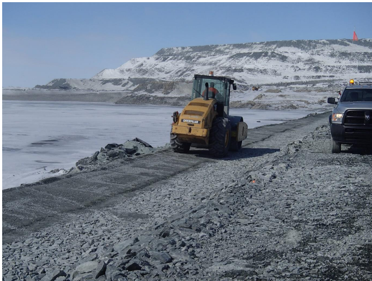
Photograph CD-1840: From Sta 0+575/-15 m, looking NW. Compaction of the second 0.5 m lift (approx.) of fine and coarse filters material at El. 144 m with a 10-tonne smooth-drum compactor with vibration (4 passes) from Sta 0+500 m to 40+730 m.
