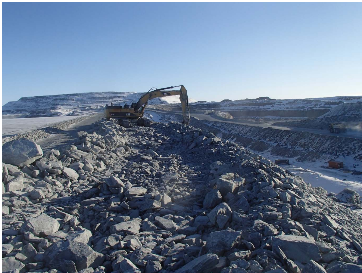
Photograph CD-1854: From Sta. 0+960/-13 m, looking N. Profiling of the downstream slope (1.5H:1V) from El. 143 to 145 m with an excavator between Sta. 0+940 m and 0+990 m.
