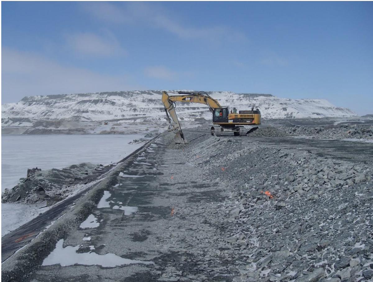
Photograph CD-1838: From Sta 0+835/-20 m, looking N. Placement of a second 0.5 m thick lift of coarse filter from El. 143.5 m to 144 m with an excavator from Sta. 0+500 m to 0+835 m and from 0+930 to 40+730 m.
