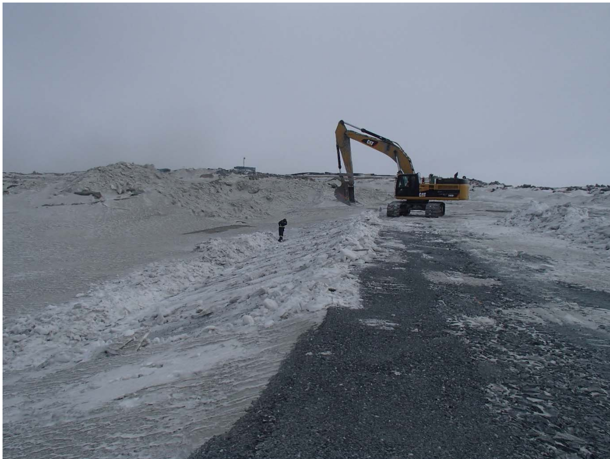
Photograph SD-297: From Sta. 20+730/-10 m, looking SE. Removal of snow on the upstream slope of SD3 with an excavator, from Sta. 20+640 to 20+760 m.
