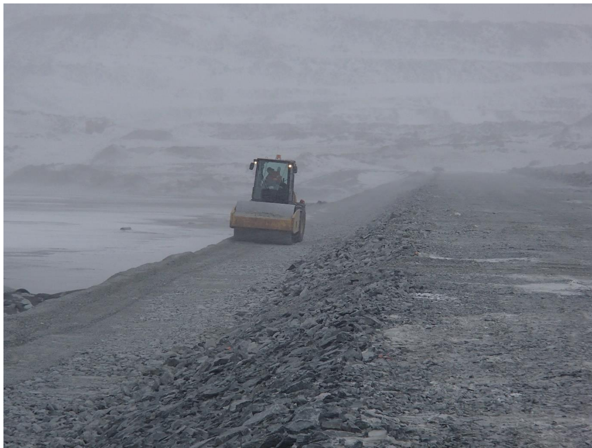
Photograph CD-1835: From Sta 0+830/-20m, looking N. Compaction of the first 0.5 m lift (approx.) of fine and coarse filters material at El. 143.5 m with a 10-tonne smooth-drum compactor with vibration (6 passes) from Sta 0+490 to 0+835 m.
