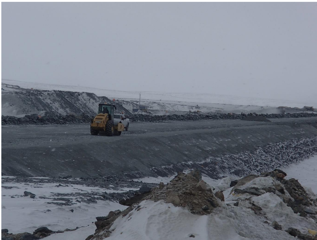
Photograph CD-1847: From Sta 0+085/-48 m, looking SE. Compaction of the fourth 0.5 m lift (approx.) of fine and coarse filters material at El. 145 m with a 10-tonne smooth-drum compactor with vibration (4 passes) from Sta 0+170 m to 0+930 m.
