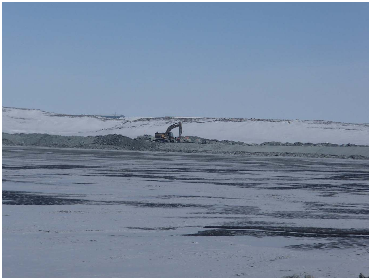
Photograph NCIS-018: From Sta. 2+310 m (approx.), looking NW. Profiling of the upstream slope (3H:1V) from El. 150 to 152 m with an excavator from Sta. 1+989 m to 1+860 m.
