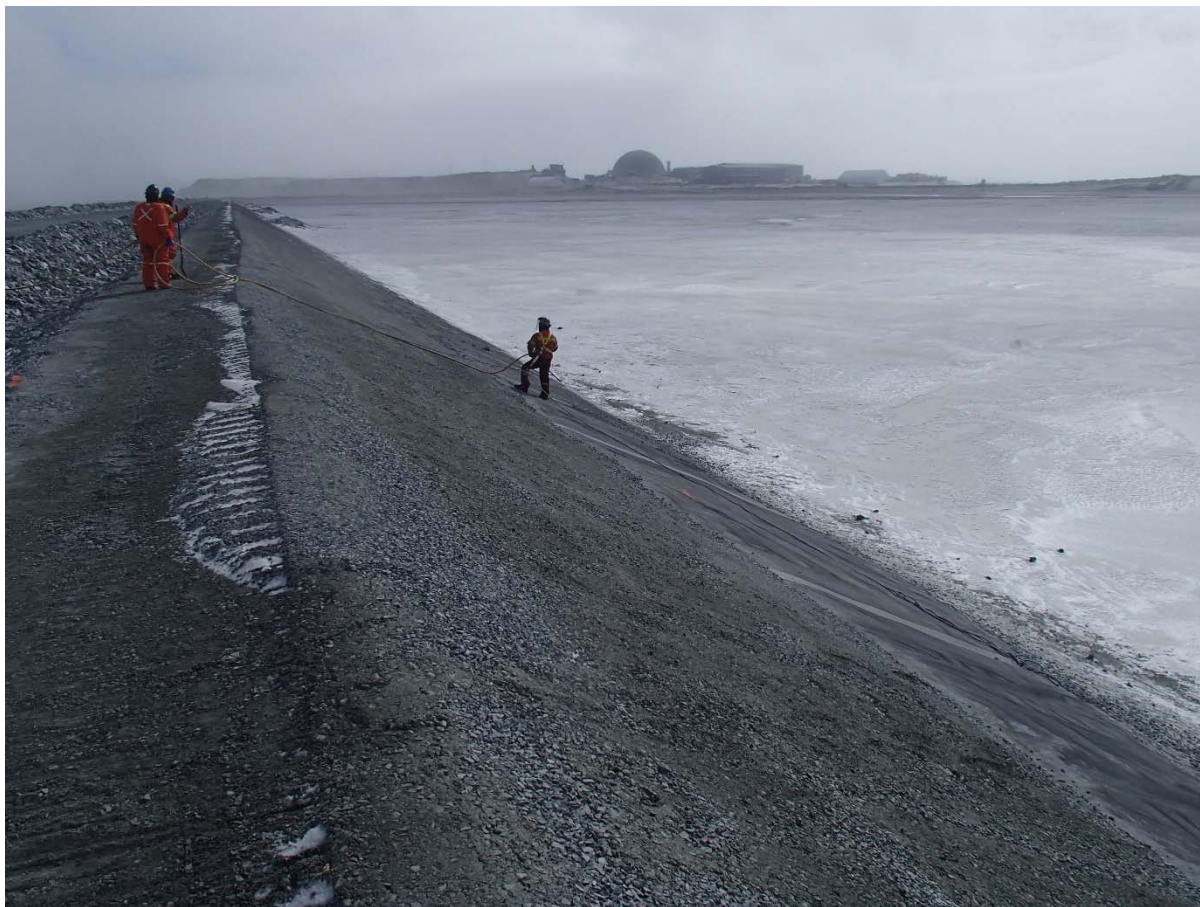
Photograph CD-1855: From Sta. 0+230/-22 m, looking S. Clean-up of the existing LLDPE with pressurized air stream in preparation for liner installation between Sta. 0+170 m and 40+780 m
