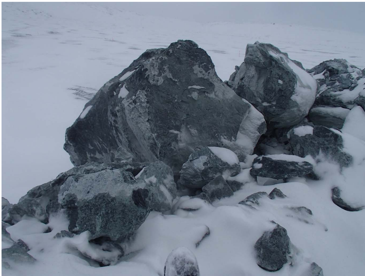
Photograph NCIS-006: View of oversize boulders on the UM rockfill lift at El. 152 m.
