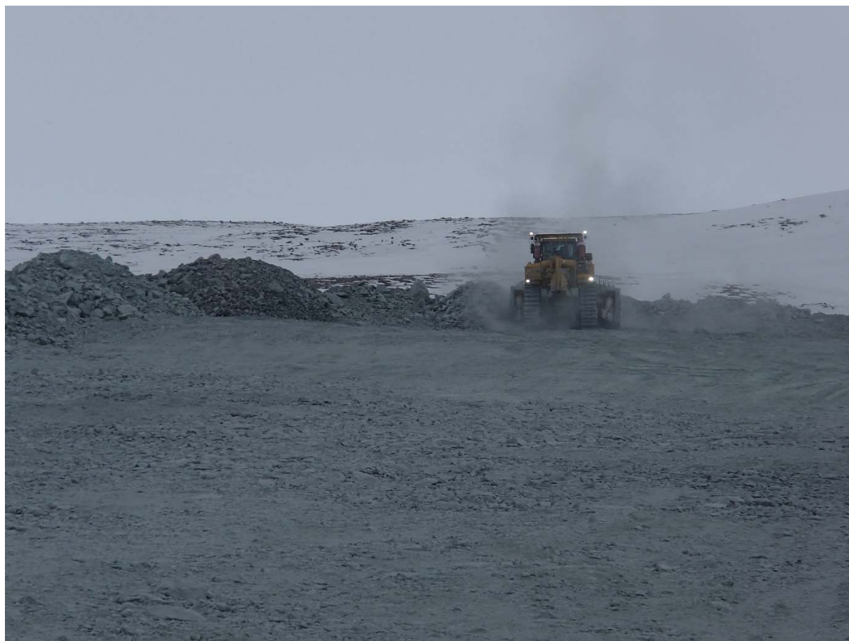
Photograph NCIS-011: From Sta. 2+000 m (approx.), looking SW. Placement a 2 m thick (approx.) lift of UM rockfill from El. 150 m to El. 152 m (approx.) with a dozer from Sta. 1+880 m to 1+767 m (o.s. unavailable).
