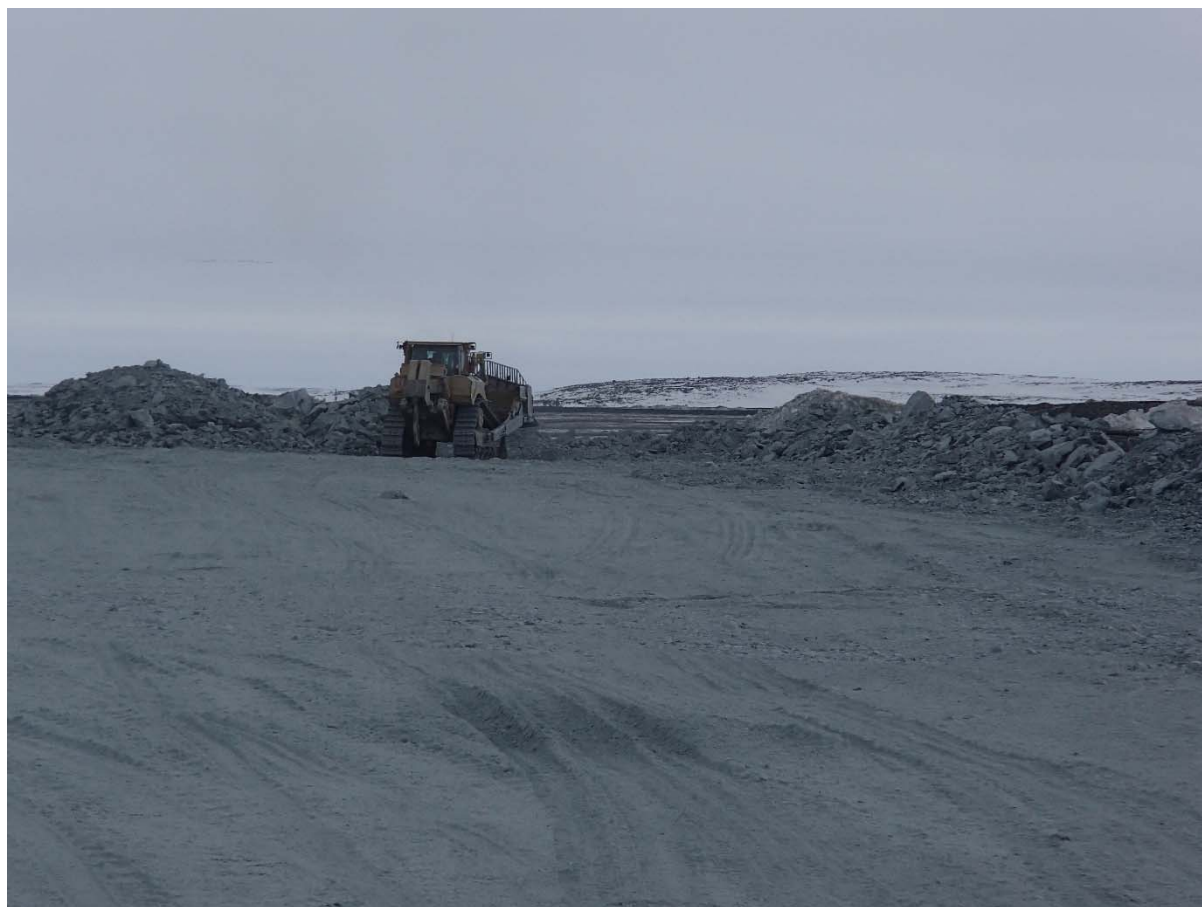
Photograph NCIS-021: From Sta. 1+550 m (approx.), looking S. Placement a 2 m thick (approx.) lift of UM rockfill from El. 150 m to El. 152 m (approx.) with a dozer from Sta. 1+535 m to 1+500 m (o.s. unavailable).
