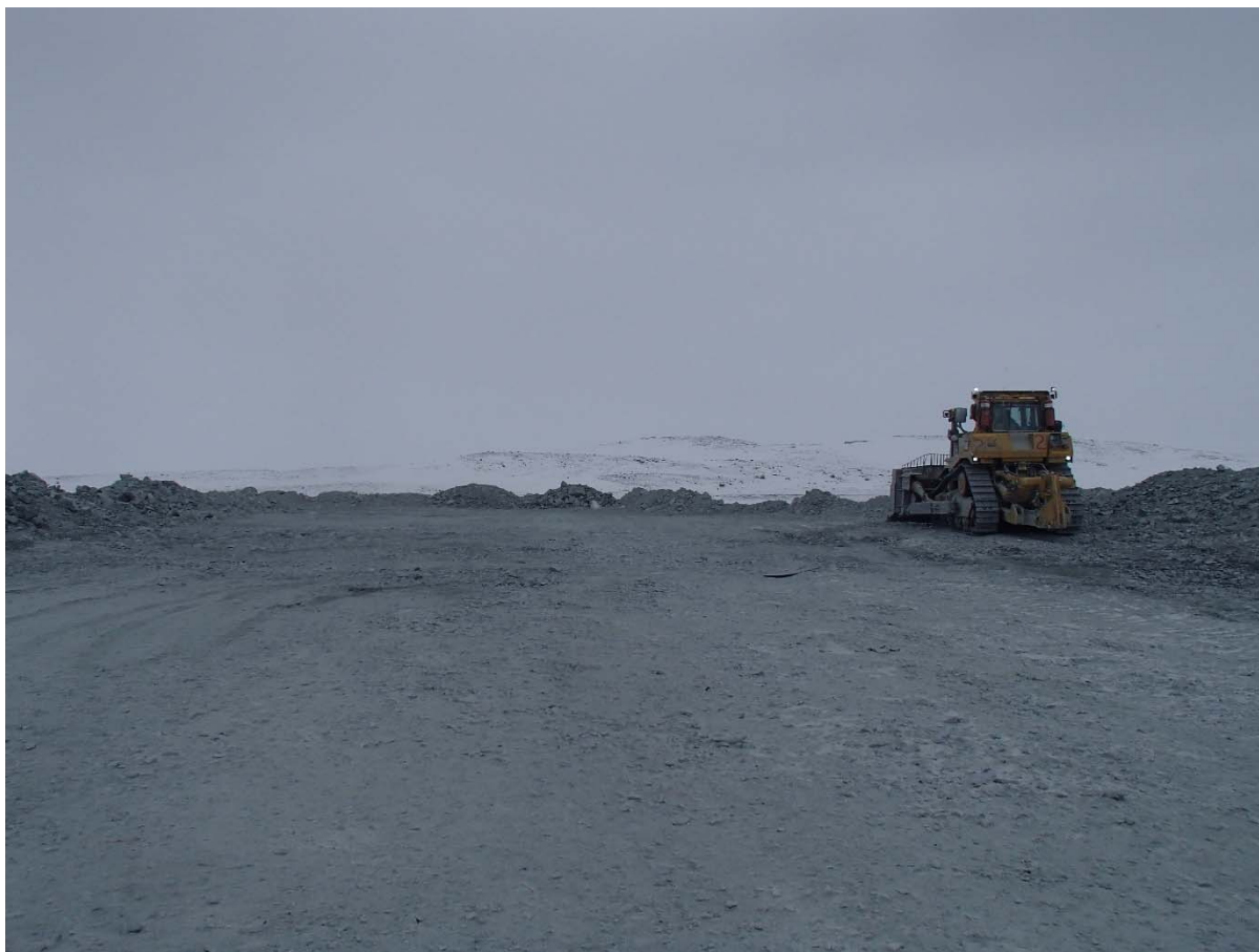
Photograph NCIS-009: Placement a 2 m thick (approx.) lift of UM rockfill from El. 150 m to El. 152 m (approx.) with a dozer from Sta. 1+880 m to 1+825 m (o.s. unavailable).
