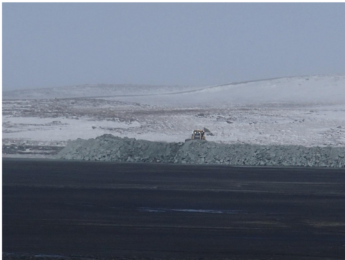
Photograph NCIS-023: From Sta. 2+570 m (approx.), looking W. Placement of a 2 m thick (approx.) lift of UM rockfill from El. 150 m to El. 152 m (approx.) with a dozer from Sta. 1+500 m to 1+450 m (o.s. unavailable). The material is of good quality and is well graded.
