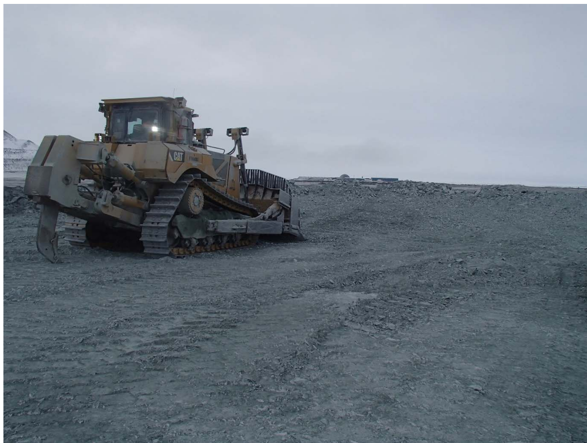
Photograph NCIS-020: From Sta. 1+570 m (approx.), looking S. Placement a 2 m thick (approx.) lift of UM rockfill from El. 150 m to El. 152 m (approx.) with a dozer from Sta. 1+564 m to 1+535 m (o.s. unavailable).
