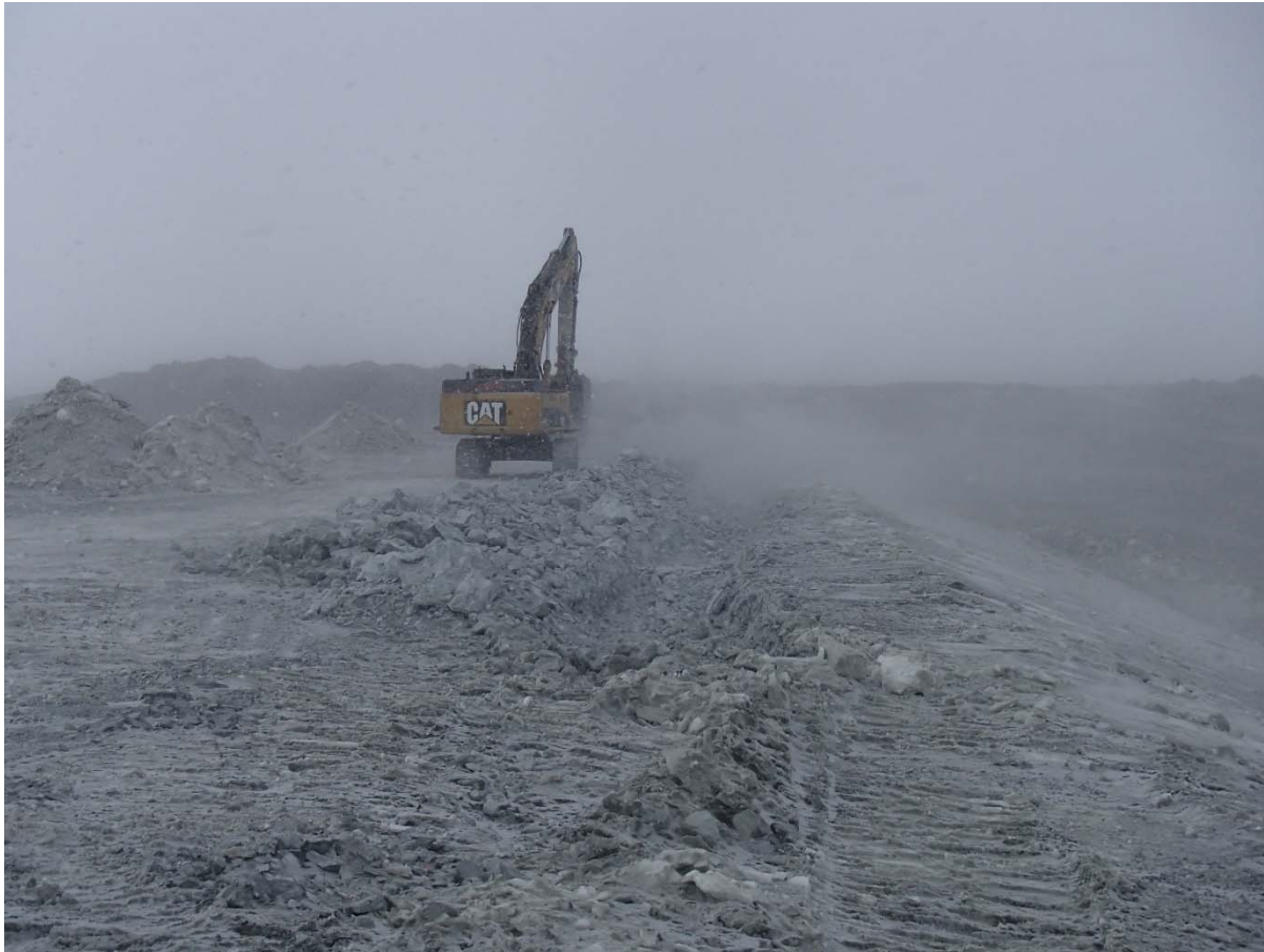
Photograph SD3-300: From Sta. 20+790/-33 m, looking NW. Excavation of the LLDPE geomembrane crest anchoring trench with an excavator from Sta. 20+675 m to 20+780 m.
