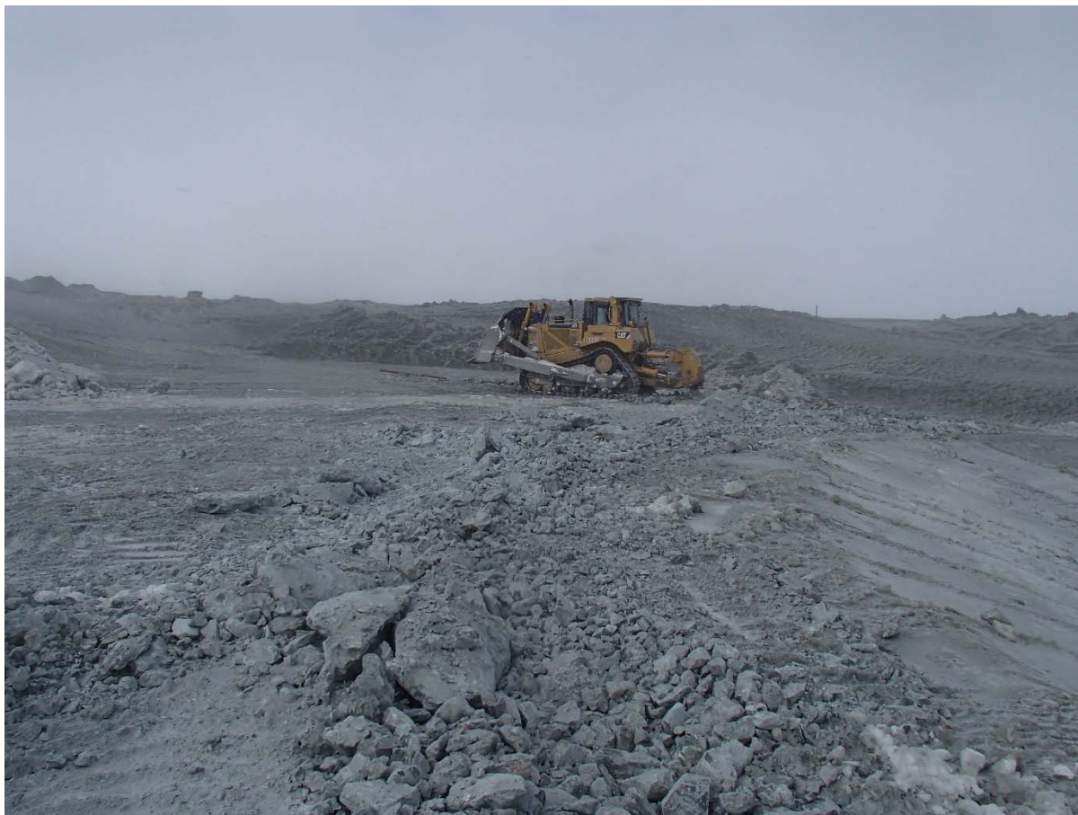
Photograph SD3-299: From Sta. 20+620/-26 m, looking NW. Scarification of the frozen ultramafic volcanic (UM) rockfill on the crest with a dozer for the anchoring trench excavation between Sta. 20+605 m and 20+780 m.
