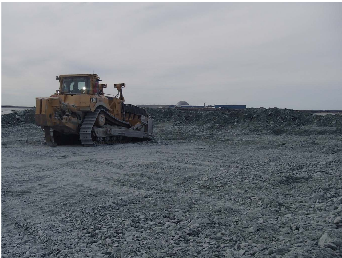
Photograph NCIS-041: From Sta. 1+220/-7 m (approx.), looking S. Placement of a 1.5 to 2 m thick (approx.) lift of UM rockfill from El. 148 m to El. 150 m (approx.) with a dozer from Sta. 1+197 m to 1+150 m (-7 m to -41 m).
