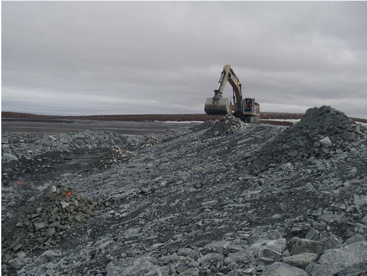
Photograph NCIS-047: From Sta. 2+580/-35 m (approx.), looking N. Placement of a 0.5 m thick lift of coarse filter in the upstream slope from El. 150 m to 152 m with an excavator from Sta. 2+560 m to 2+640 m.
