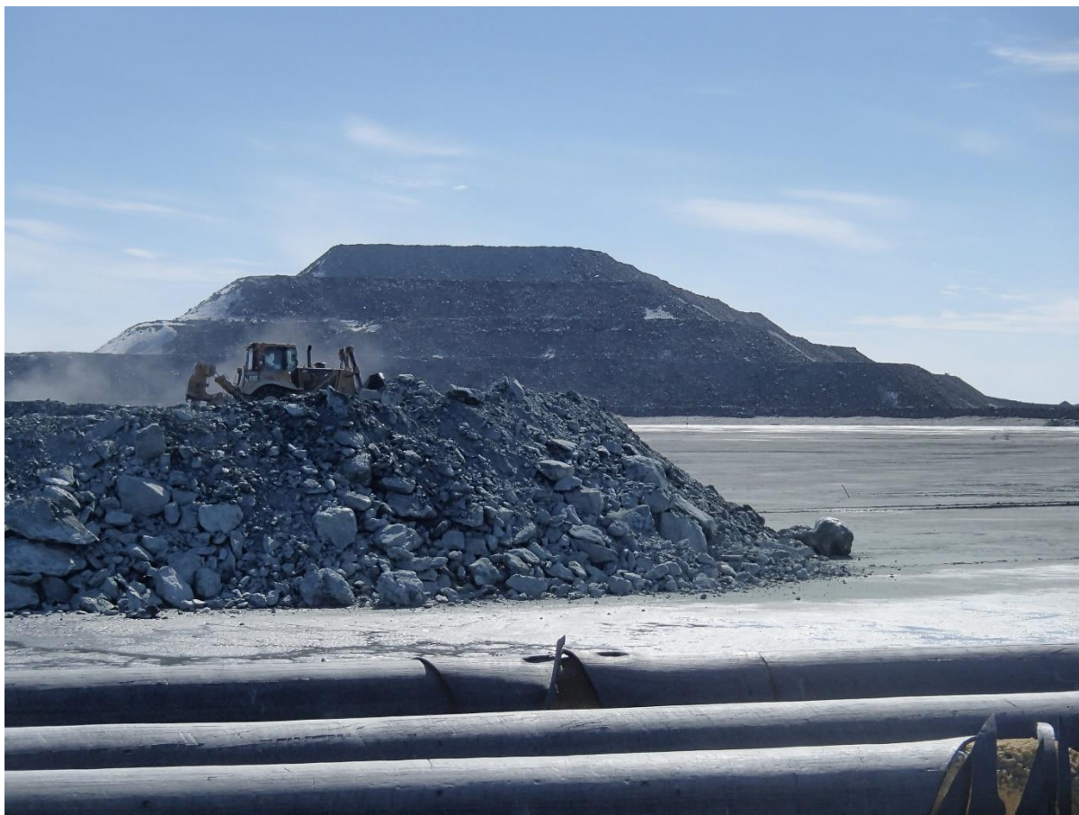
Photograph NCIS-027: From Sta. 1+360/+67 m, looking S. Placement of a 2 m thick (approx.) lift of UM rockfill from El. 150 m to El. 152 m (approx.) with a dozer from Sta. 1+365 m to 1+360 m (o.s. +9 m to -28 m).
