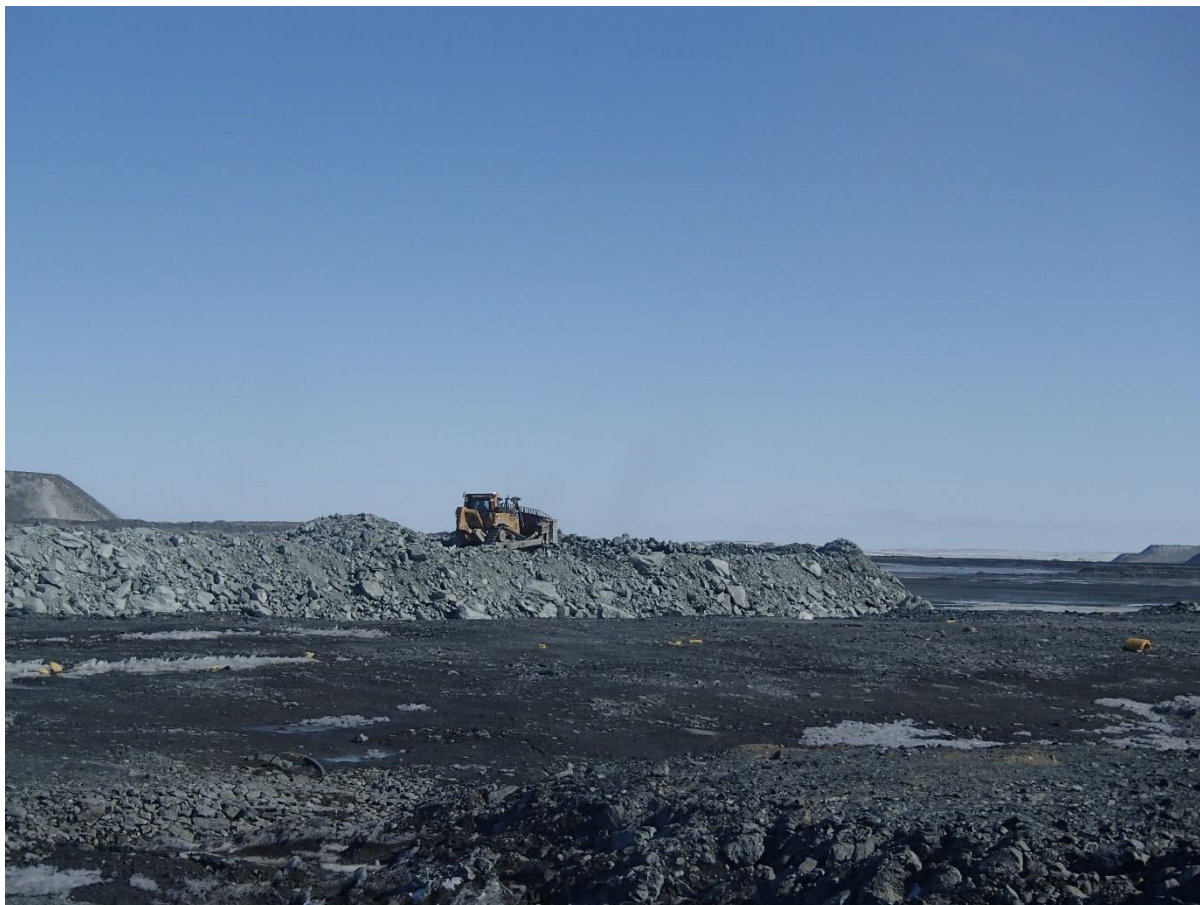
Photograph NCIS-025: From Sta. 1+475 m (approx.), looking SE. Placement of a 2 m thick (approx.) lift of UM rockfill from El. 150 m to El. 152 m (approx.) with a dozer from Sta. 1+450 m to 1+390 m (o.s. unavailable). The material is of good quality and is well graded.
