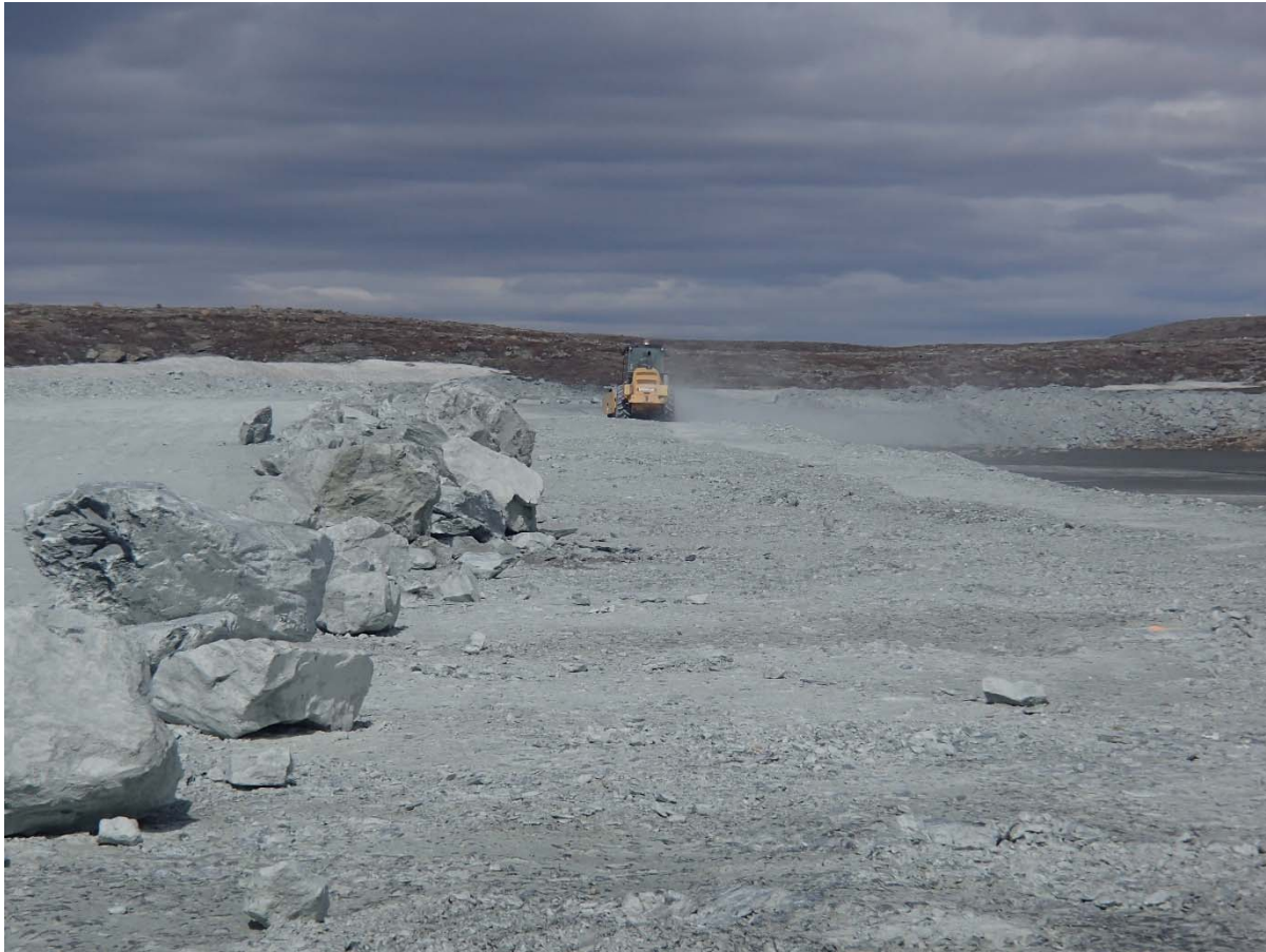
Photograph NCIS-032: From Sta. 1+400/-24 m (approx.), looking N. Compaction of the 2 m lift (approx.) of ultramafic (UM) rockfill at El. 152 m with a 10-tonne smooth-drum compactor with vibration (6 passes) between the haul truck traffic lane and the upstream slope from Sta. 1+660 to 1+380 m (o.s. -45 to -24 m).
