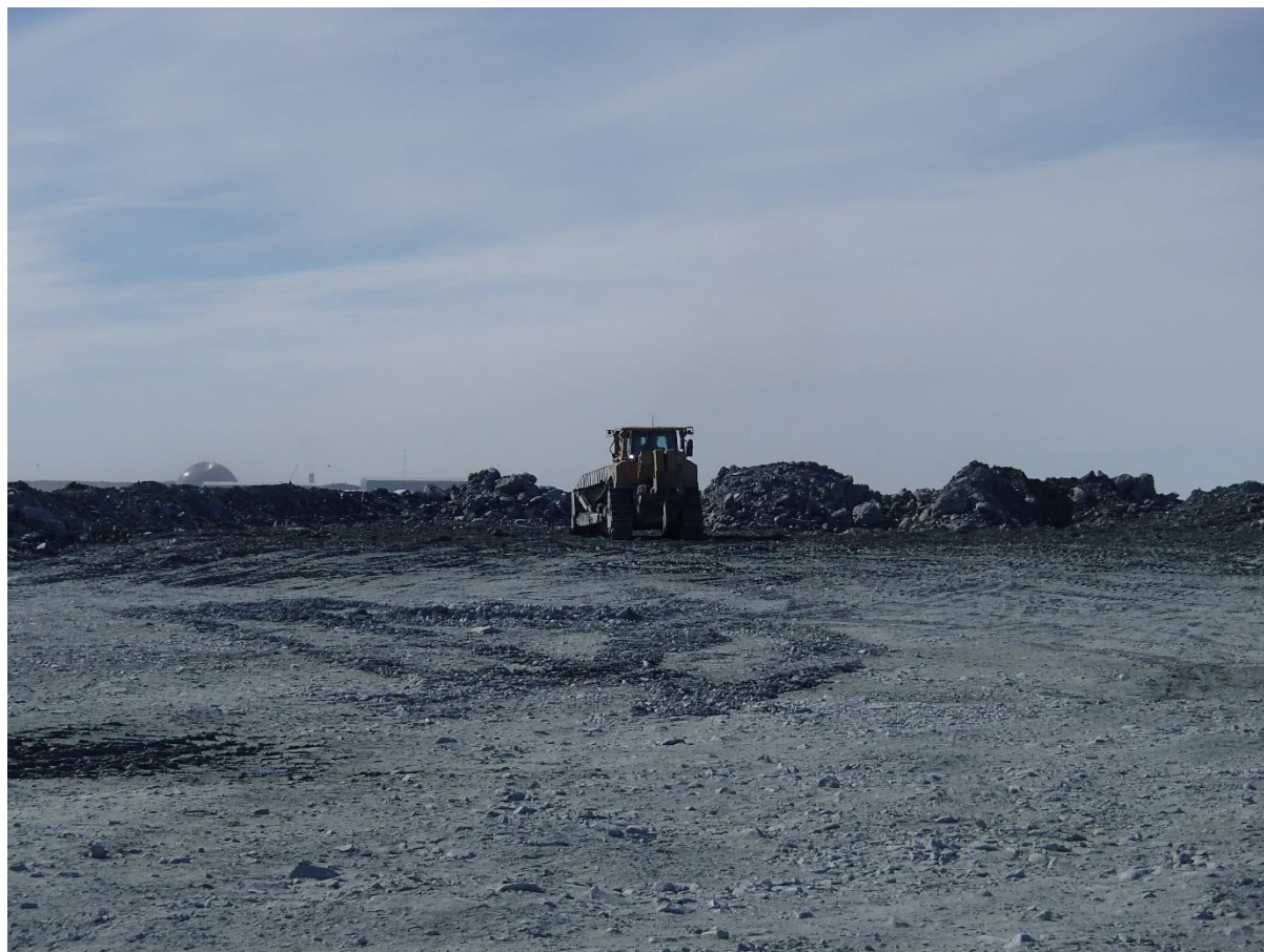
Photograph NCIS-026: From Sta. 1+440/+2 m, looking S. Placement of a 2 m thick (approx.) lift of UM rockfill from El. 150 m to El. 152 m (approx.) with a dozer from Sta. 1+390 m to 1+365 m (o.s. +10 m to -29 m).
