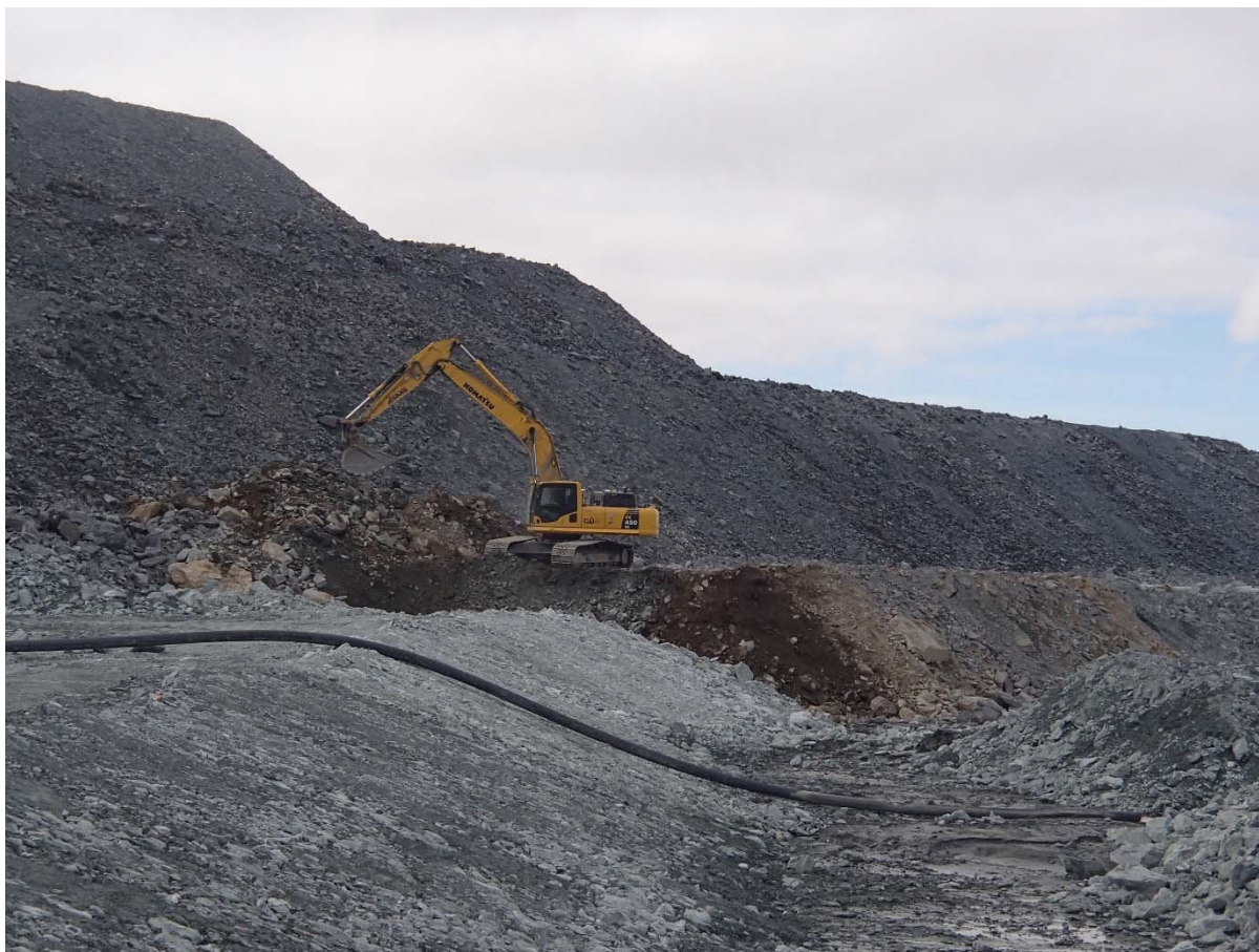
Photograph NCIS-046: From Sta. 2+680/-18 m (approx.), looking SE. Removal of till material mixed with the UM rockfill of the capping (about 1 to 2 m thick along the slope) with an excavator from Sta. 2+760 m to 2+850 m (o.s. -35 to -17 m).
