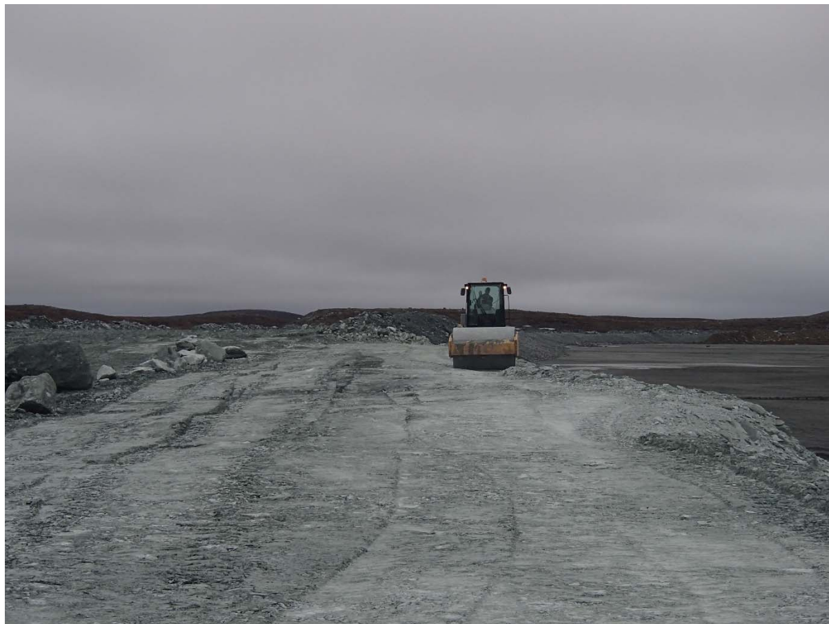
Photograph NCIS-043: From Sta. 1+250/-38 m (approx.), looking N. Compaction of the 1.5 to 2 m lift (approx.) of ultramafic (UM) rockfill at El. 150 m with a 10-tonne smooth-drum compactor with vibration (6 passes) between the haul truck traffic lane and the upstream slope from Sta. 1+330 to 1+200 m (o.s. -53 to -24 m).
