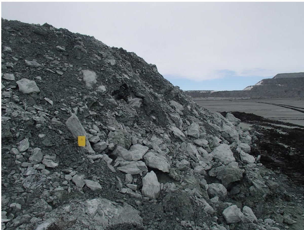
Photograph NCIS-028: From Sta. 1+340/+3 m, looking E. View of the UM rockfill lift approximately 3.2 m thick.
