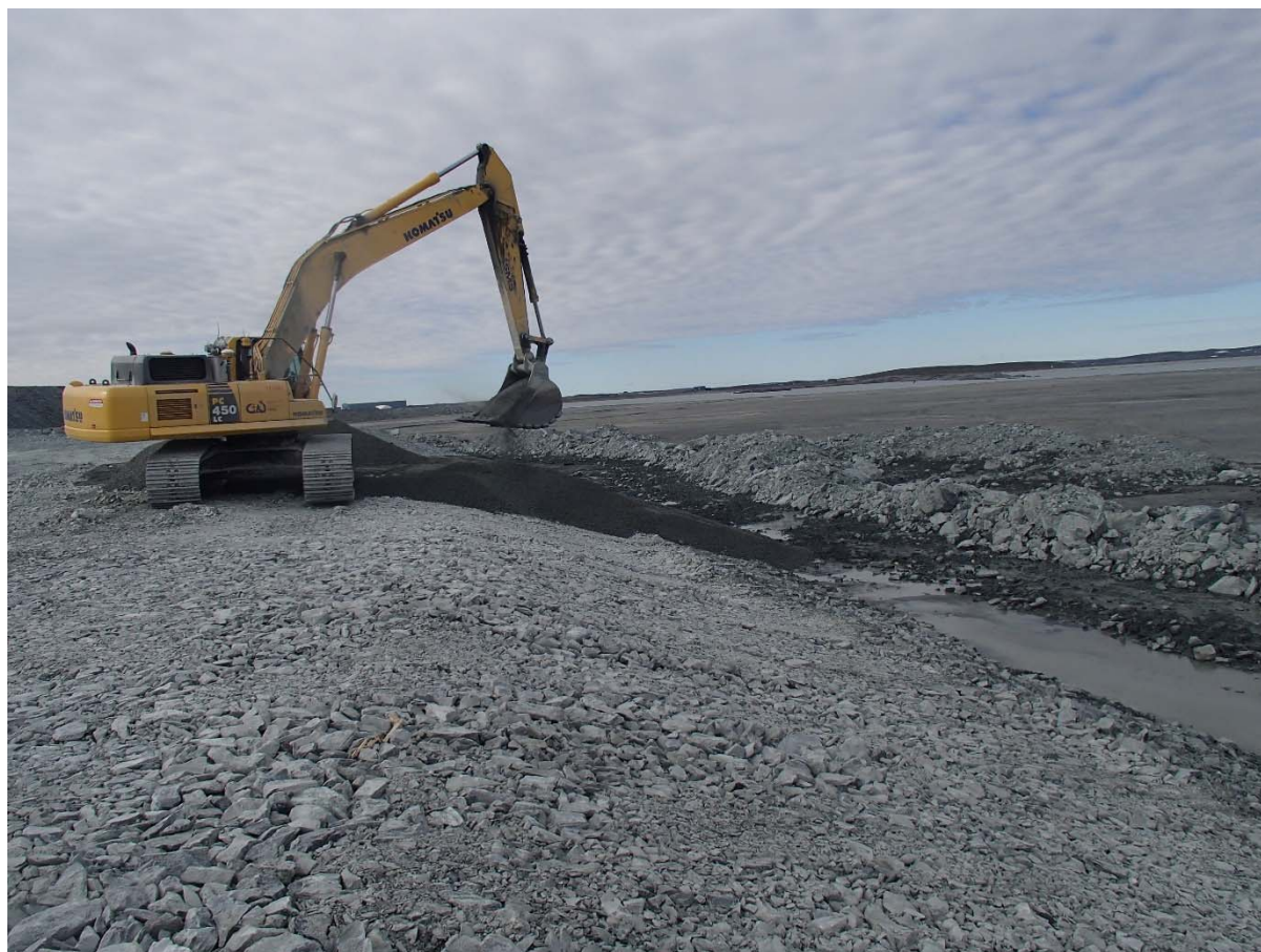
Photograph NCIS-036: From Sta. 1+900/-21 m (approx.), looking SE. Placement of a 0.5 m thick lift of fine filter over the coarse filter in the upstream slope from El. 150 m to 152 m with an excavator from Sta. 2+542 m to 2+475 m.
