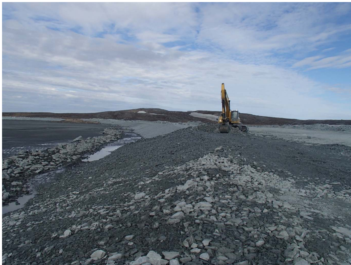
Photograph NCIS-030: From Sta. 2+140/-29 m (approx.), looking W. Placement of a 0.5 m thick lift of coarse filter in the upstream slope from El. 150 m to 152 m with an excavator from Sta. 2+105 m to 1+930 m. Notice the presence of water ponding at the bottom of the slope.
