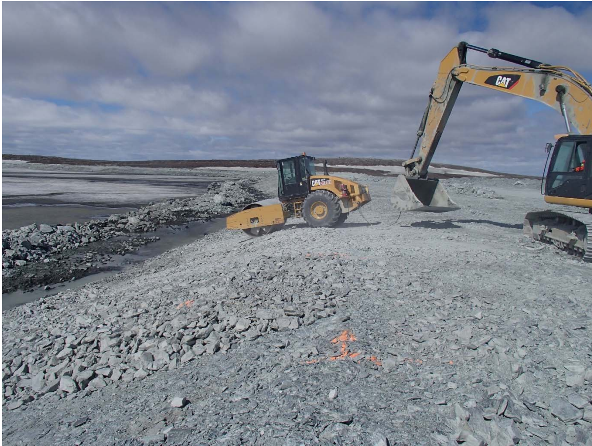
Photograph NCIS-035: From Sta. 2+550/-25 m (approx.), looking N. Compaction of the 0.5 m lift (approx.) of coarse filter between El. 150 and 152 m with a 10-tonne smooth-drum compactor (4 passes) in the upstream slope from Sta. 2+524 m to 2+450 m.
