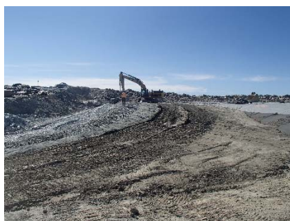
SD3-336 (2018-07-14), looking S from Sta. 20+755/-48 m. Placement of a fourth 0.5 m thick lift of fine filter, coarse filter and fine rockfill on the upstream slope of the upstream toe liner tie-in with an excavator from Sta. 20+770 to 20+800 m.
