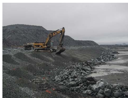
NCIS-042 (2018-06-25), looking SE from Sta. 2+210/-27 m. Placement of a 0.5 m thick lift of fine filter over the coarse filter in the upstream slope from El. 150 m to 152 m with an excavator from Sta. 2+305 m to 2+040 m.
