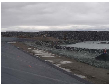
SD3-319 (2018-07-08), looking NE from Sta. 20+740/-31 m. Placement of IV rockfill in the water up to El. 142m with an excavator from Sta. 20+730 m to 20+610 m, at the bottom of the upstream slope of SD3 to widen the rockfill layer and allow access to the erosion protection.
