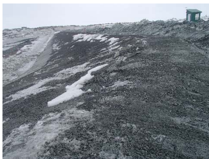
SD3-304 (2018-05-21), looking SE from Sta. 20+620/-36 m. Smoothing of the surface of the fine filter with an excavator on top of the upstream slope from Sta. 20+600 m to 20+780 m.
