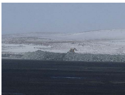
NCIS-023 (2018-05-31), looking W from Sta. 2+570 m. Placement of a 2 m thick (approx.) lift of UM rockfill from El. 150 m to El. 152 m (approx.) with a dozer from Sta. 1+500 m to 1+450 m (o.s. unavailable). The material is of good quality and is well graded.
