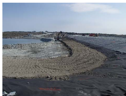
SD3-323 (2018-07-09), looking S from Sta. 20+610/-43 m. Placement of the first 0.5 m thick lift of low quality till (0-150 mm) from El. 142 m to 142.5 m from Sta. 20+610 m to 20+715 m.
