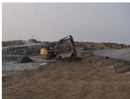
SD3-324 (2018-07-10), looking S from Sta. 20+680/-39 m. Placement of a 0.5 m thick lift of low quality till (0-150 mm) from El. 142 m to 142.5 m from Sta. 20+715 m to 20+760 m.
