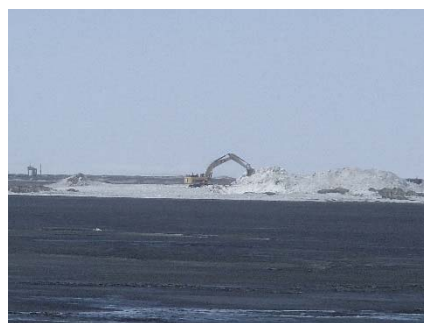
NCIS-024 (2018-05-31), looking SW from Sta. 2+570 m. Removal of the snow bank in the footprint with an excavator from Sta. 1+160 m to 1+120 m (approx.).
