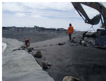
SD3-308 (2018-06-06), looking SW from Sta. 20+620/-48 m. Installation of the geotextile on the upstream slope 3H:1V between El. 143 m and 145 m from Sta. 20+620 m to 20+630 m.
