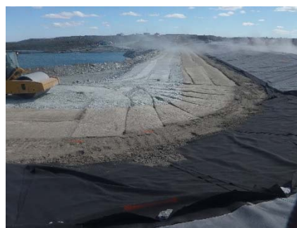
SD3-331 (2018-07-12), looking S from Sta. 20+610/-43 m. Compaction of the 0.5 m lift of low quality till (0-150 mm) at El. 143 m with a 10-tonne smooth-drum compactor with vibration (4 passes) from Sta. 20+610 m to 20+760 m.
