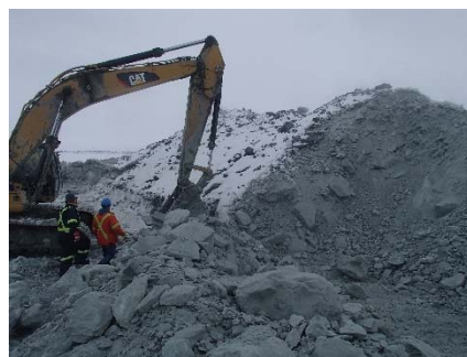
NCIS-003 (2018-05-19). Excavation of the snow-rich upstream toe material on an average width of 2 to 3 m with an excavator.
