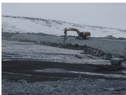
NCIS-017 (2018-05-24), looking SW from Sta. 2+290 m. Profiling of the upstream slope (3H:1V) from El. 150 to 152 m with an excavator from Sta. 2+138 m to 1+989 m.
