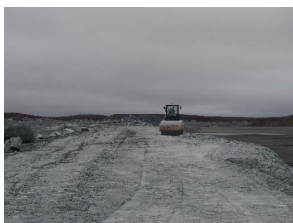
NCIS-043 (2018-06-25), looking N from Sta. 1+250/-38 m. Compaction of the 1.5 to 2 m lift (approx.) of ultramafic (UM) rockfill at El. 150 m with a 10-tonne smooth-drum compactor with vibration (6 passes) between the haul truck traffic lane and the upstream slope from Sta. 1+330 to 1+200 m (o.s. -53 to -24 m).
