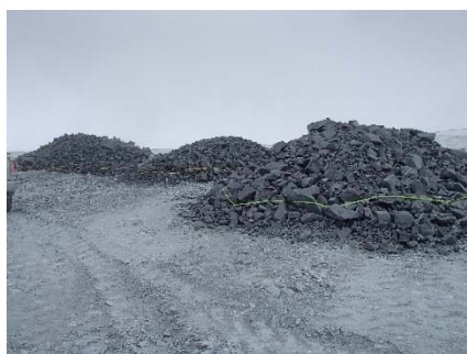
NCIS-016 (2018-05-23), looking SE from Sta. 1+750 m. View of the Iron Formation rockfill (PAG material) piles on the North Cell Internal Structure.
