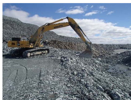
NCIS-045 (2018-06-25), looking S from Sta. 2+760/-40 m. Profiling of the upstream slope (3H:1V) from El. 150 to 152 m with an excavator from Sta. 2+715 m to 2+825 m.
