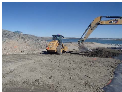
SD3-339 (2018-07-15), looking E from Sta. 20+600/-29 m. Compaction of a first 0.5 m thick lift of compacted sieved till on the upstream toe liner tie-in with an excavator from Sta. 20+588 m to 20+599 m.
