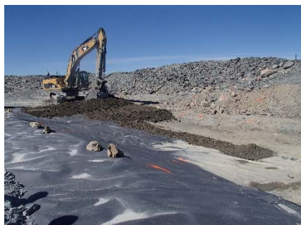
SD3-338 (2018-07-14), looking NW from Sta. 20+610/-43 m. Placement of a first 0.5 m thick lift of compacted sieved till over the LLDPE geomembrane on the upstream toe liner tie-in with an excavator from Sta. 20+588 m to 20+599 m.
