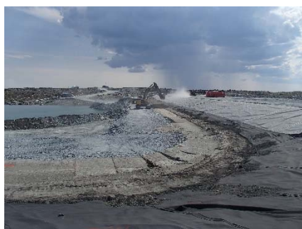
SD3-329 (2018-07-11), looking N from Sta. 20+820/-34 m. Placement of a 0.5 m thick lift of low quality till (0-150 mm) from El. 142.5 m to 143 m from Sta. 20+610 m to 20+760 m.
