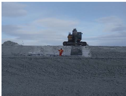
SD3-298 (2018-05-16), looking S from Sta. 20+680/-88 m. Removal of snow on the upstream slope of SD3 above El. 142 m, from Sta. 20+620 m to 20+780 m.
