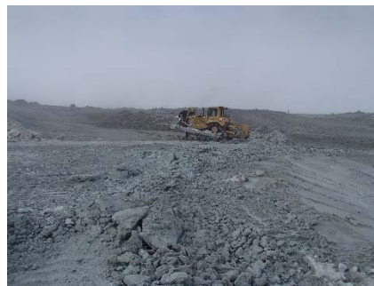
SD3-299 (2018-05-16), looking NW from Sta. 20+620/-26 m. Scarification of the frozen ultramafic volcanic (UM) rockfill on the crest with a dozer for the anchoring trench excavation between Sta. 20+605 m and 20+780 m.
