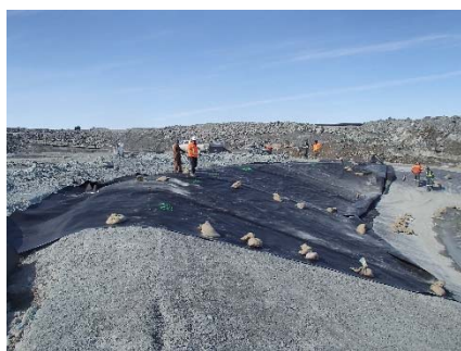
SD3-309 (2018-06-06), looking N from Sta. 20+640/-26 m. Installation of the LLDPE liner on the upstream slope 3H:1V between El. 143 m and 145 m from Sta. 20+620 m to 20+630 m (panel numbers 934 to 939).
