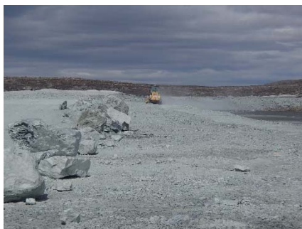
NCIS-032 (2018-06-20), looking N from Sta. 1+400/-24 m. Compaction of the 2 m lift (approx.) of ultramafic (UM) rockfill at El. 152 m with a 10-tonne smooth-drum compactor with vibration (6 passes) between the haul truck traffic lane and the upstream slope from Sta. 1+660 to 1+380 m (o.s. -45 to -24 m).
