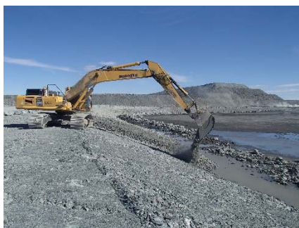
NCIS-029 (2018-06-19), looking SE from Sta. 2+120/-27 m. Placement of a 0.5 m thick lift of coarse filter in the upstream slope from El. 150 m to 152 m with an excavator from Sta. 2+280 m to 2+105 m.
