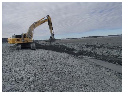
NCIS-036 (2018-06-22), looking SE from Sta. 1+900/-21 m. Placement of a 0.5 m thick lift of fine filter over the coarse filter in the upstream slope from El. 150 m to 152 m with an excavator from Sta. 2+542 m to 2+475 m.
