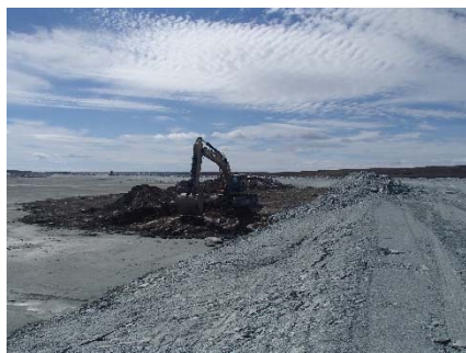
NCIS-031 (2018-06-20), looking SW from Sta. 1+880/-21 m. Final clean-up of the dike footprint with an excavator to reach a good quality bedrock from Sta. 1+800 to 1+850 m (o.s. -42 to -33 m).
