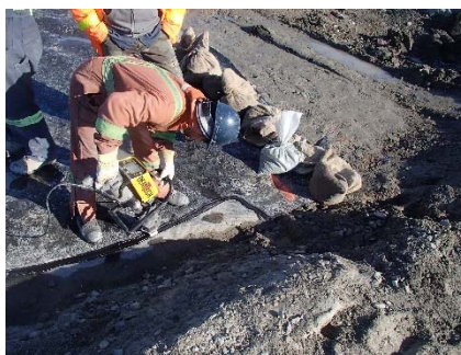
SD3-316 (2018-06-09), looking NW from Sta. 20+610/-45 m. Repairs on the extrusion fillet seam between LLDPE panel 965 and the existing LLDPE panel at Sta. 20+600 m (approx.).
