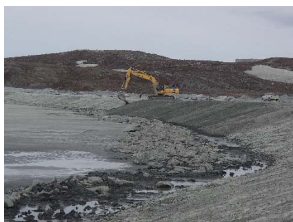
NCIS-040 (2018-06-24), looking W from Sta. 2+185/-25 m. Placement of a 0.5 m thick lift of fine filter over the coarse filter in the upstream slope from El. 150 m to 152 m with an excavator from Sta. 2+305 m to 2+460 m and from Sta. 1+980 m to 1+835 m.
