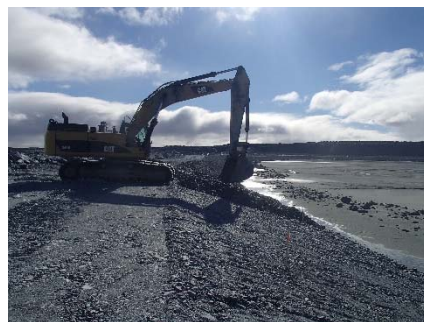
NCIS-033 (2018-06-21), looking E from Sta. 1+900/-21 m. Placement of a 0.5 m thick lift of coarse filter in the upstream slope from El. 150 m to 152 m with an excavator from Sta. 1+930 m to 1+715 m.
