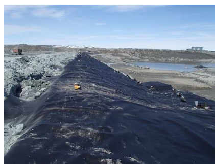
SD3-311 (2018-06-07), looking N from Sta. 20+810/-26 m. Installation of the LLDPE liner on the upstream slope 3H:1V between El. 143 m and 145 m from Sta. 20+630 m to 20+800 m (panel numbers 939 to 964).
