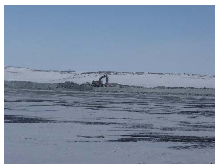
NCIS-018 (2018-05-25), looking NW from Sta. 2+310 m. Profiling of the upstream slope (3H:1V) from El. 150 to 152 m with an excavator from Sta. 1+989 m to 1+860 m.
