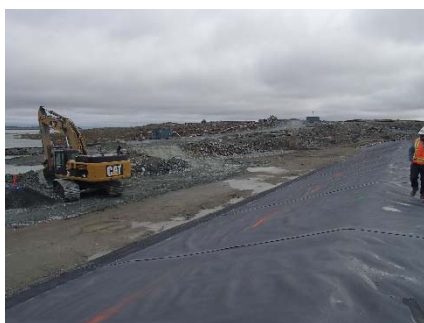
SD3-318 (2018-07-07), looking SE from Sta. 20+710/-24 m. Placement of IV rockfill in the water up to El. 142m with an excavator from Sta. 20+785 m to 20+730 m, at the bottom of the upstream slope of SD3 to widen the rockfill layer and allow access to the erosion protection.
