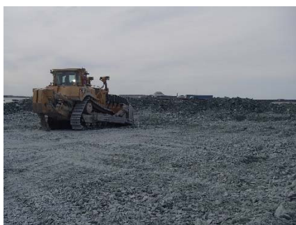
NCIS-041 (2018-06-24), looking S from Sta. 1+220/-7 m. Placement of a 1.5 to 2 m thick (approx.) lift of UM rockfill from El. 148 m to El. 150 m (approx.) with a dozer from Sta. 1+197 m to 1+150 m (-7 m to -41 m).
