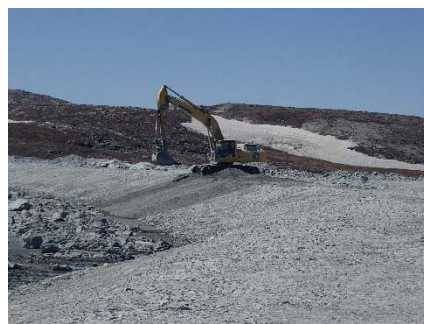
NCIS-039 (2018-06-23), looking W from Sta. 2+200/-24 m. Placement of a 0.5 m thick lift of fine filter over the coarse filter in the upstream slope from El. 150 m to 152 m with an excavator from Sta. 2+460 m to 2+475 m and from Sta. 2+065 m to 1+980 m.
