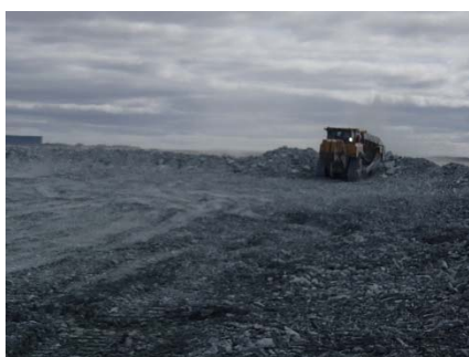
NCIS-044 (2018-06-25), looking S from Sta. 1+200/-19 m. Placement of a 1.5 to 2 m thick (approx.) lift of UM rockfill from El. 148 m to El. 150 m (approx.) with a dozer from Sta. 1+150 m to 1+120 m (-92 m to +10 m). The material is of good quality and is well graded.
