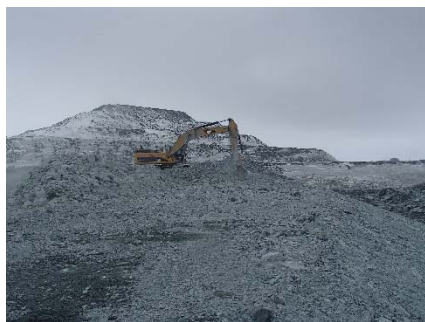
NCIS-013 (2018-05-22), looking NE from Sta. 2+600 m. Correction of the crest elevation with an excavator to achieve a closer elevation to 152 m around Sta. 2+650 m.
