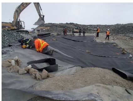
SD3-315 (2018-06-08), looking W from Sta. 20+615/-46 m. Installation of the geotextile on the upstream slope 3H:1V between El. 143 m and 145 m from Sta. 20+593 m to 20+610 m and installation of the LLDPE liner on the upstream slope 3H:1V between El. 143 m and 145 m from Sta. 20+593 m to 20+610 m (panel numbers 965 to 967).
