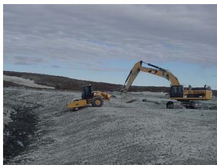
NCIS-037 (2018-06-22), looking NW from Sta. 1+550/-25 m. Compaction of the 0.5 m lift (approx.) of coarse filter between El. 150 and 152 m with a 10-tonne smooth-drum compactor (4 passes) in the upstream slope from Sta. 2+450 to 1+805 m.
