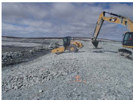
NCIS-035 (2018-06-21), looking N from Sta. 2+550/-25 m. Compaction of the 0.5 m lift (approx.) of coarse filter between El. 150 and 152 m with a 10-tonne smooth-drum compactor (4 passes) in the upstream slope from Sta. 2+524 m to 2+450 m.
