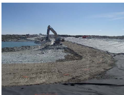
SD3-330 (2018-07-12), looking S from Sta. 20+610/-43 m. Placement of a second 0.5 m thick lift of fine rockfill (0-500 mm) upstream of the low quality till (0-150mm) from El. 142.5 m to 143 m from Sta. 20+610 m to 20+760 m.
