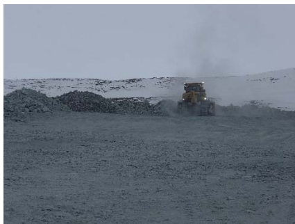
NCIS-011 (2018-05-22), looking SW from Sta. 2+000 m. Placement a 2 m thick (approx.) lift of UM rockfill from El. 150 m to El. 152 m (approx.) with a dozer from Sta. 1+880 m to 1+767 m (o.s. unavailable).
