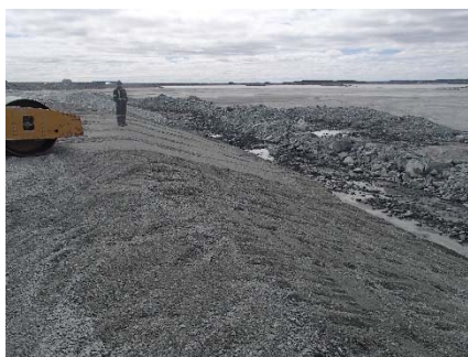
NCIS-038 (2018-06-22), looking SE from Sta. 2+510/-28 m. Compaction of the 0.5 m lift (approx.) of fine filter between El. 150 and 152 m with a 10-tonne smooth-drum compactor (4 passes) in the upstream slope from Sta. 2+542 m to 2+475 m.
