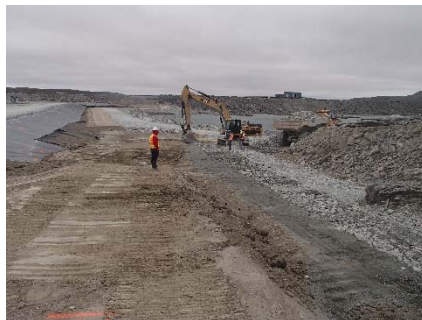
SD3-333 (2018-07-13), looking N from Sta. 20+817/-29 m. Placement of a second 0.5 m thick lift of fine rockfill on the upstream slope of the upstream toe liner tie-in with an excavator from Sta. 20+775 m to 20+800 m.
