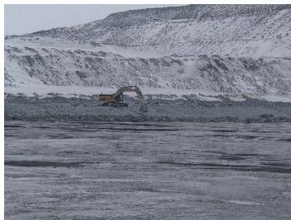
NCIS-010 (2018-05-21). Profiling of the upstream slope (3H:1V) from El. 150 to 152 m with an excavator from Sta. 2+777 m to 2+400 m.
