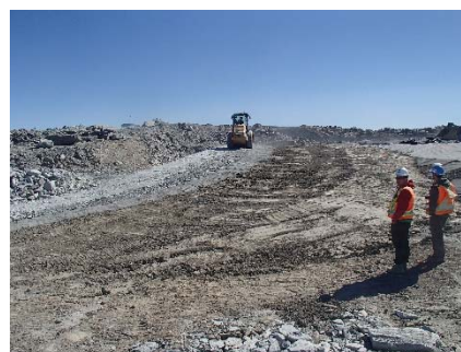
SD3-337 (2018-07-14), looking S from Sta. 20+760/-37 m. Compaction of the fourth 0.5 m thick lifts of fine filter, coarse filter and fine rockfill on the upstream slope of the upstream toe liner tie-in with a 10 tonne smooth-drum compactor with vibrations (4 passes) from Sta. 20+770 to 20+800 m.
