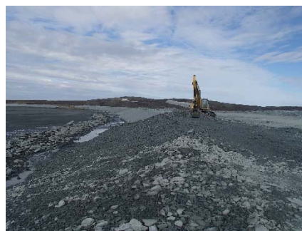
NCIS-030 (2018-06-20), looking W from Sta. 2+140/-29 m. Placement of a 0.5 m thick lift of coarse filter in the upstream slope from El. 150 m to 152 m with an excavator from Sta. 2+105 m to 1+930 m. Notice the presence of water ponding at the bottom of the slope.
