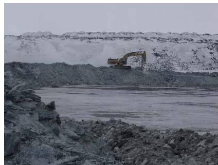
NCIS-012 (2018-05-22), looking NW from Sta. 2+000 m. Profiling of the upstream slope (3H:1V) from El. 150 to 152 m with an excavator from Sta. 2+325 m to 2+275 m (approx.).
