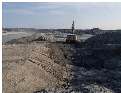
SD3-326 (2018-07-11), looking N from Sta. 20+820/-34 m. Placement of the 0.5 m thick lift of low class till, fine filter, coarse filter and fine rockfill on the upstream slope of the upstream toe liner tie-in with an excavator from Sta. 20+780 to 20+810 m.
