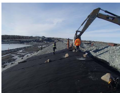
SD3-310 (2018-06-07), looking S from Sta. 20+635/-24 m. Installation of the geotextile on the upstream slope 3H:1V between El. 143 m and 145 m from Sta. 20+630 m to 20+800 m.
