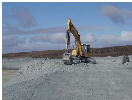
NCIS-034 (2018-06-21), looking W from Sta. 1+900/-21 m. Profiling of the upstream slope (3H:1V) from El. 150 to 152 m with an excavator from Sta. 1+860 m to 1+750 m.
