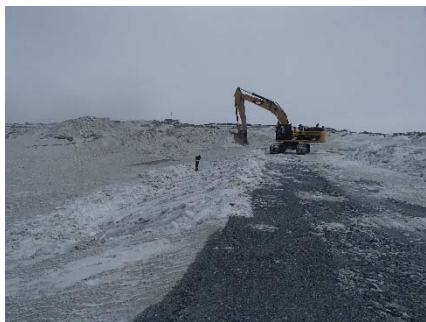
SD3-297 (2018-05-14), looking SE from Sta. 20+730/-10 m. Removal of snow on the upstream slope of SD3 with an excavator, from Sta. 20+640 to 20+760 m.
