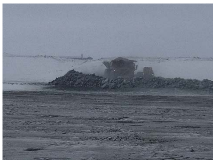
NCIS-008 (2018-05-20). Placement a 2 m thick (approx.) lift of UM rockfill from El. 150 m to El. 152 m (approx.) with a dozer. The material is of good quality and is well graded.
