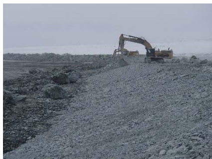
NCIS-007 (2018-05-20). Profiling of the upstream slope (3H:1V) from El. 150 to 152 m with an excavator.
