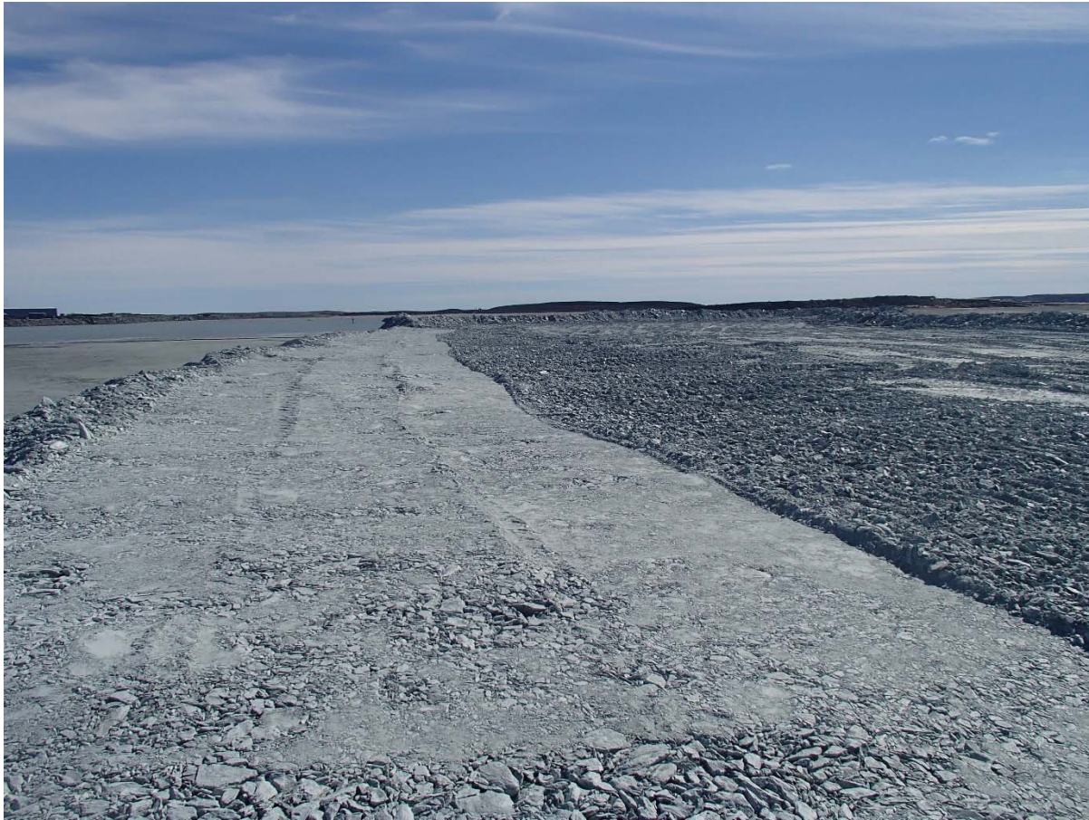
Photograph NCIS-050: From Sta. 1+230/-55 m (approx.), looking S. Compaction of the 1.5 to 2 m lift (approx.) of ultramafic (UM) rockfill at El. 150 m with a 10-tonne smooth-drum compactor with vibration (6 passes) between the haul truck traffic lane and the upstream slope from Sta. 1+220 to 1+130 m (o.s. -91 to -44 m).
