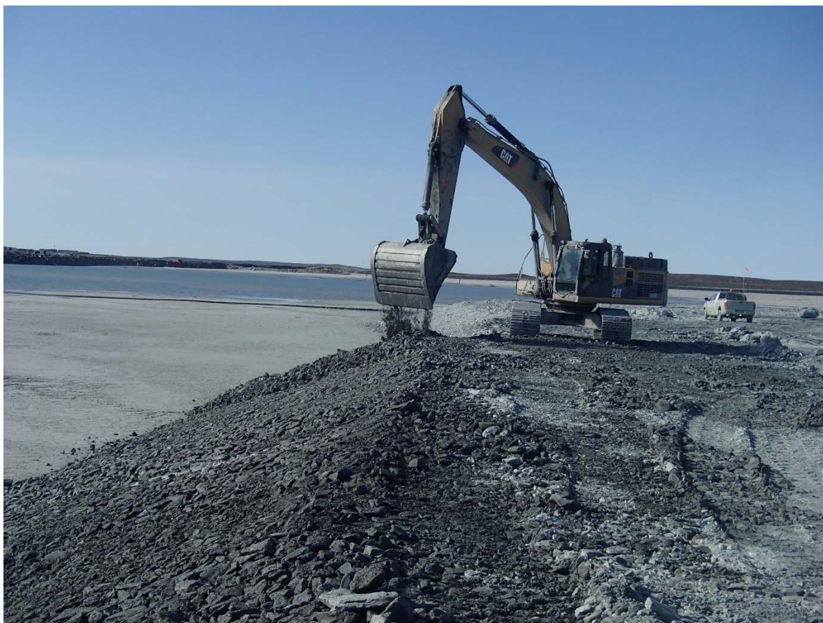
Photograph NCIS-063: From Sta. 1+200/-65 m (approx.), looking SW. Placement of a 0.5 m thick lift of coarse filter in the upstream slope from El. 148 m to 150 m with an excavator from Sta. 1+270 m to 1+100 m.
