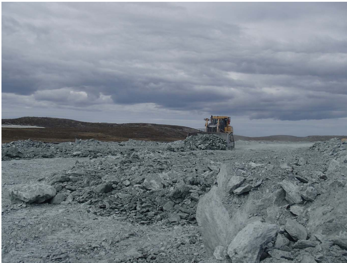
Photograph NCIS-069: From Sta. 1+180/-56 m (approx.), looking NW. Placement of a 2 m thick (approx.) lift of UM rockfill from El. 150 m to El. 152 m (approx.) with a dozer from Sta. 1+235 m to 1+160 m (-60 m to -44 m). The material is of good quality and is well graded.
