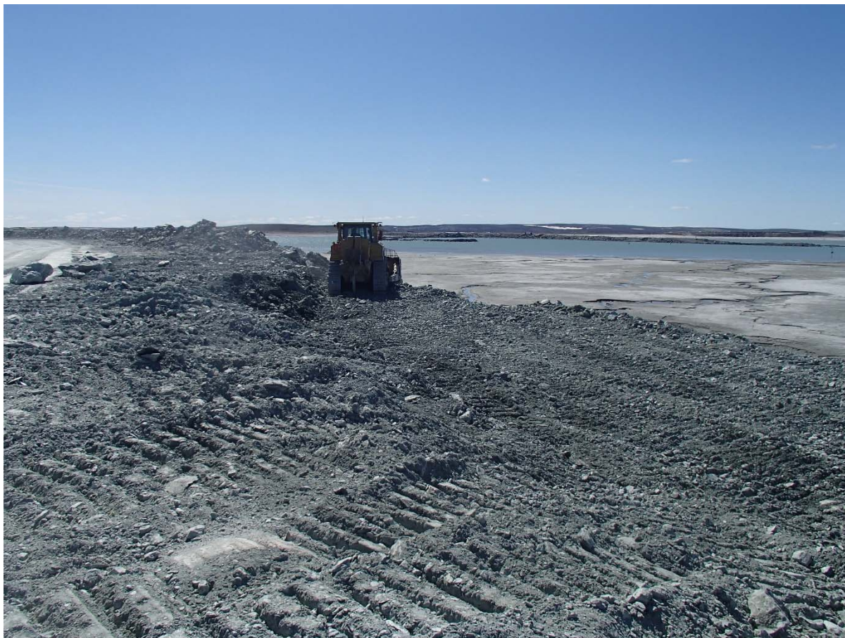
Photograph NCIS-057: From Sta. 3+010/-15 m (approx.), looking SW. Removing of UM rockfill material from the capping with a dozer to level the surface to El. 152 m from Sta. 2+980 m to 3+050 m (o.s. -30 to -20 m).
