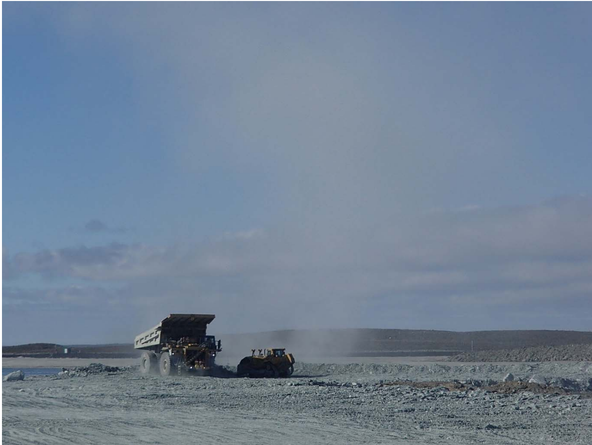
Photograph NCIS-059: From Sta. 1+330/-34 m (approx.), looking S. Placement of a 1.5 to 2 m thick (approx.) lift of UM rockfill from El. 148 m to El. 150 m (approx.) with a dozer from Sta. 1+120 m to 1+100 m (-96 m to -60 m). The material is of good quality and is well graded.
