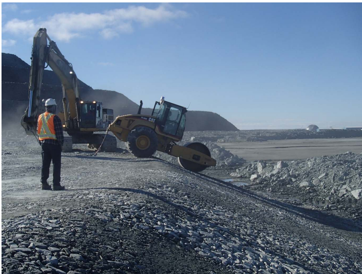
Photograph NCIS-054: From Sta. 2+580/-31 m (approx.), looking SE. Compaction of the 0.5 m lift (approx.) of coarse filter between El. 150 and 152 m with a 10-tonne smooth-drum compactor with vibration (4 passes) in the upstream slope from Sta. 2+560 m to 2+815 m.
