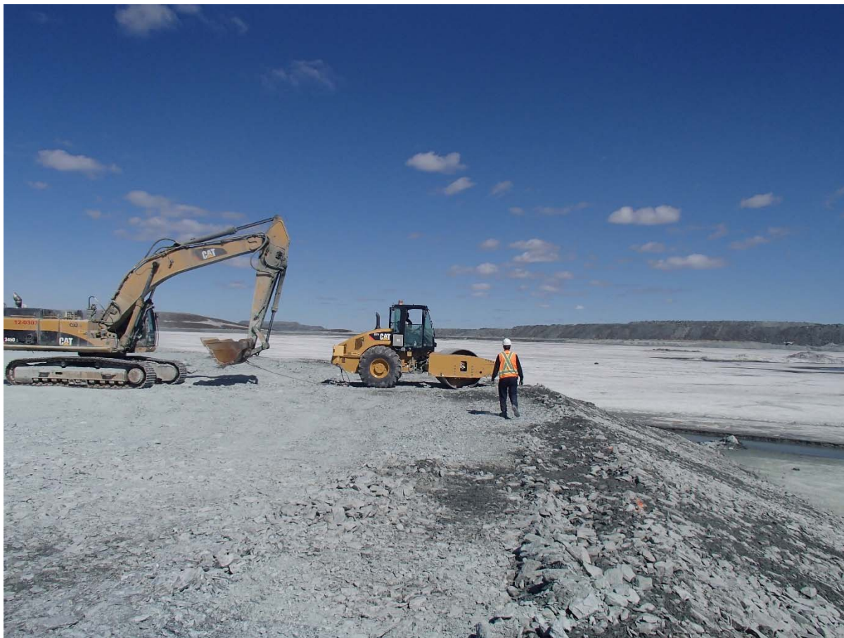
Photograph NCIS-065: From Sta. 1+140/-96 m (approx.), looking NE. Compaction of the 0.5 m lift of coarse filter between El. 148 and 150 m with a 10-tonne smooth-drum compactor with vibration (4 passes) in the upstream slope from Sta. 1+270 m to 1+100 m.
