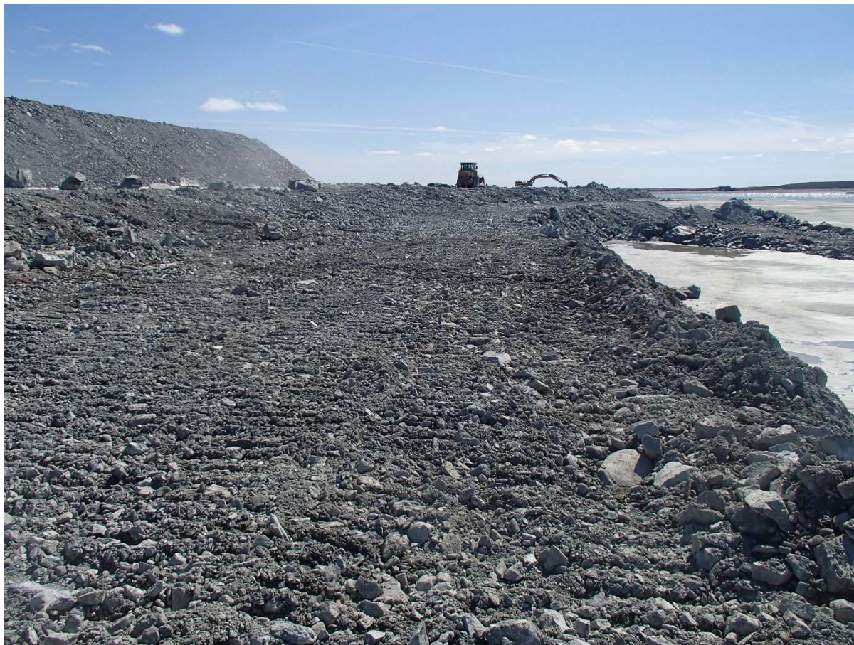
Photograph NCIS-053: From Sta. 2+840/-37 m (approx.), looking S. Removing of UM rockfill material from the capping with a dozer to level the surface to El. 152 m from Sta. 2+850 m to 2+980 m (o.s. -38 to -24 m).
