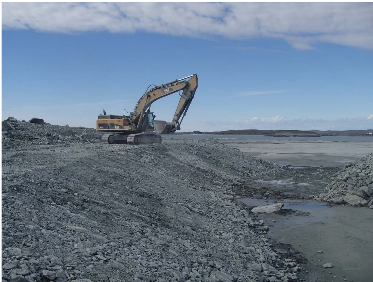
Photograph NCIS-067: From Sta. 2+880/-26 m (approx.), looking SW. Profiling of the upstream slope (3H:1V) from El. 150 to 152 m with an excavator from Sta. 2+860 m to 2+975 m.
