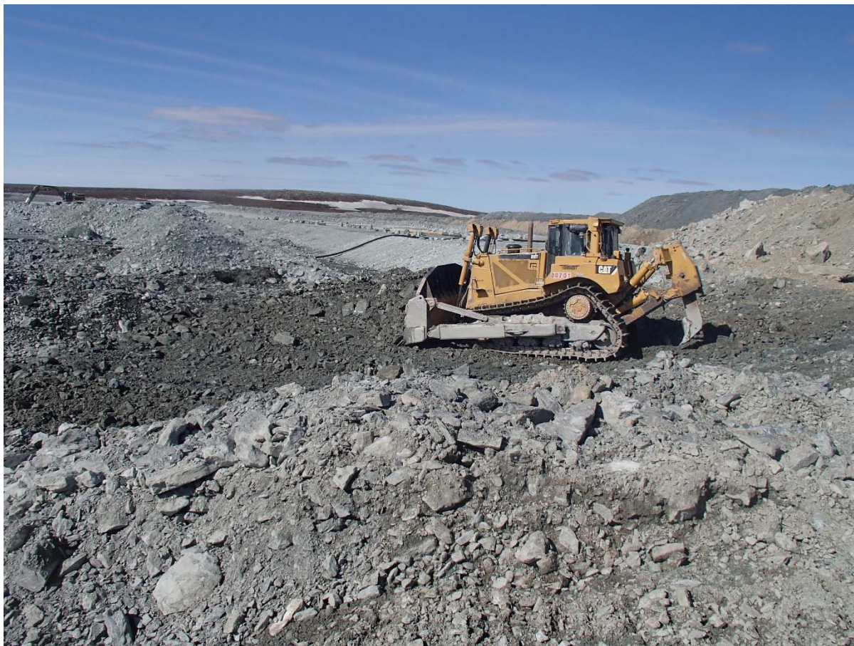
Photograph NCIS-049: From Sta. 2+870/-28 m (approx.), looking N. Removing of UM rockfill material from the capping with a dozer to level the surface to El. 150 m from Sta. 2+760 m to 2+850 m (o.s. -29 to -17 m).
