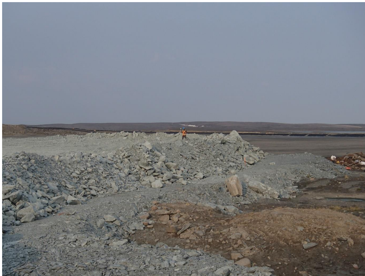
Photograph NCIS-085: From Sta 1+150/-67m (approx.), looking SW. Placement of a 2 m thick (approx.) lift of UM rockfill from El. 150 m to El. 152 m (approx.) with a dozer from Sta. 1+130 m to 1+100 m (-55 m to -78 m).
