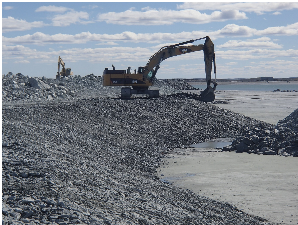
Photograph NCIS-075: From Sta. 2+860/-36 m (approx.), looking S. Placement of a 0.5 m thick lift of coarse filter in the upstream slope from El. 150 m to 152 m with an excavator from Sta. 2+815 m to 2+980 m.
