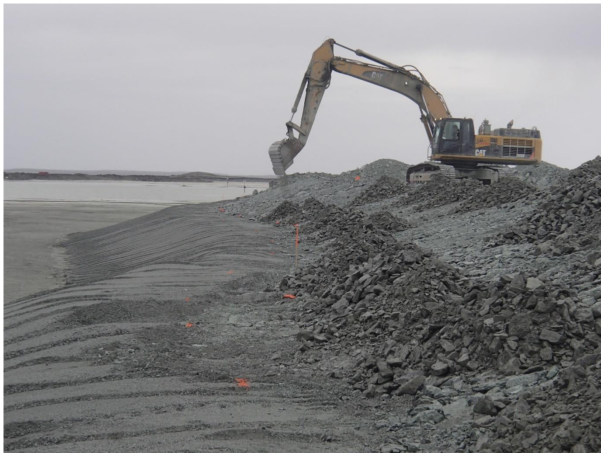
Photograph NCIS-079: From Sta. 1+280/-39 m (approx.), looking SW. Placement of a 0.5 m thick lift of coarse filter in the upstream slope from El. 150 m to 152 m with an excavator from Sta. 1+300 m to 1+200 m.
