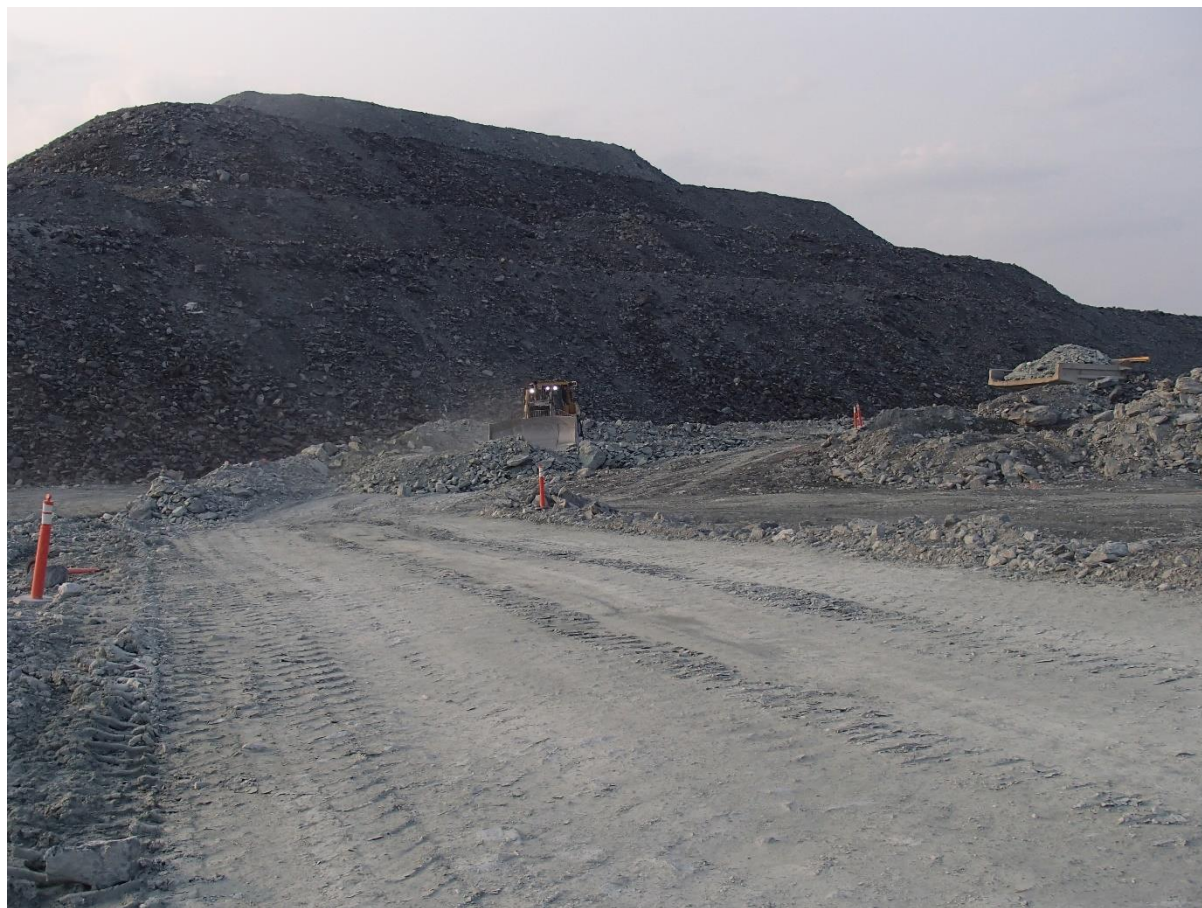
Photograph NCIS-086: From Sta 2+750/+14 m (approx.), looking E. Placement of a 2 m thick (approx.) lift of UM rockfill from El. 152 m to El. 154 m (approx.) with a dozer from Sta. 2+780 m to 2+760 m (-60 m to -44 m).
