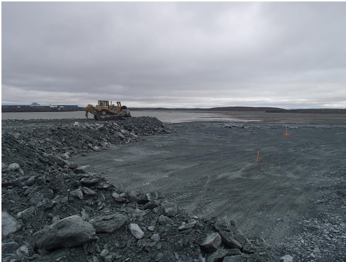
Photograph NCIS-082: From Sta 1+140/-52 m (approx.), looking SW. Placement of a 2 m thick (approx.) lift of IV rockfill from El. 150 m to El. 152 m (approx.) with a dozer from Sta. 1+160 m to 1+170 m (-64 m to -111 m). The material is of good quality and is well graded.
