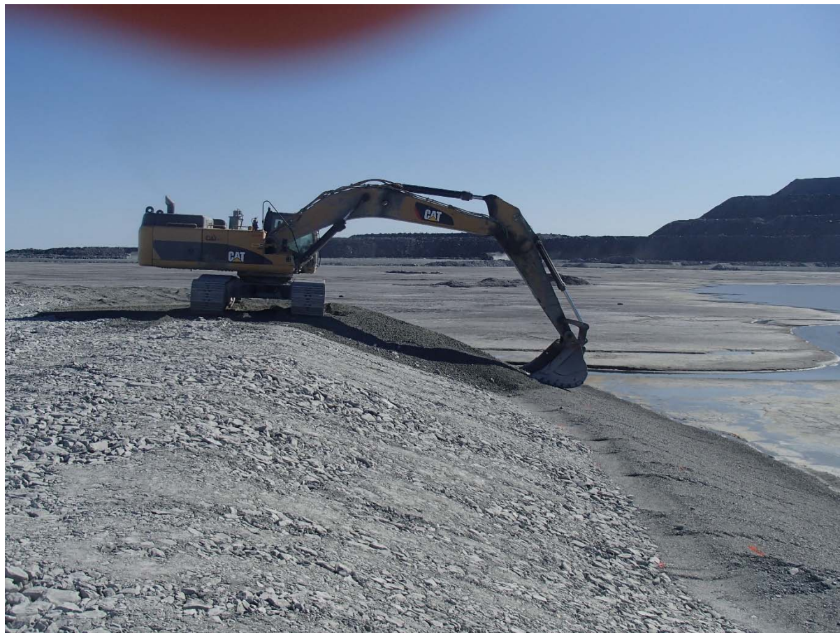
Photograph NCIS-101: From Sta. 1+120/-89 m (approx.), looking N. Placement of a 0.5 m thick lift of fine filter in the upstream slope from El. 150 m to 152 m with an excavator from Sta. 1+113 m to 1+205 m.
