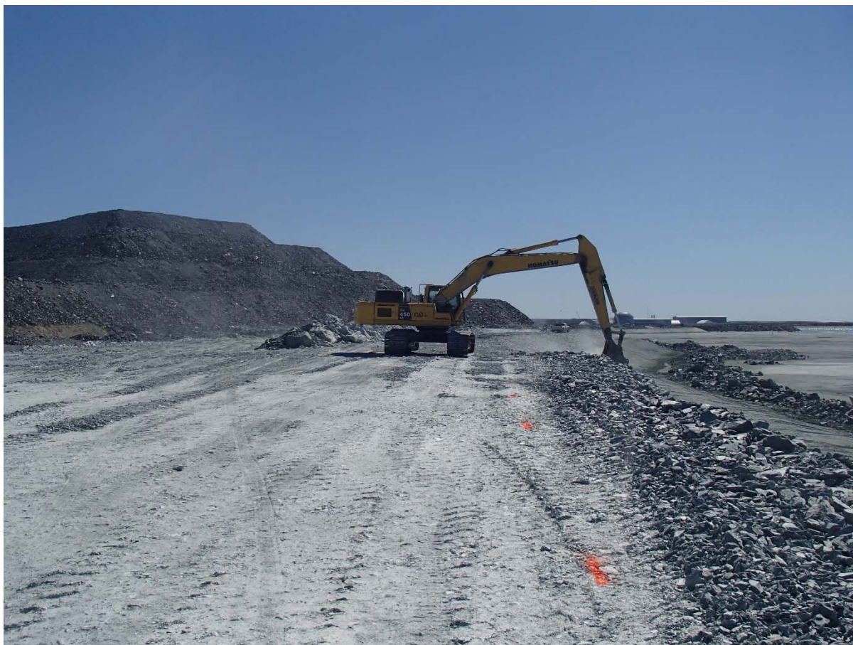
Photograph NCIS-095: From Sta 2+375/-18 m (approx.), looking S. Profiling of the upstream slope (3H:1V) from El. 152 to 154 m with an excavator from Sta. 2+545 m to 2+410 m.
