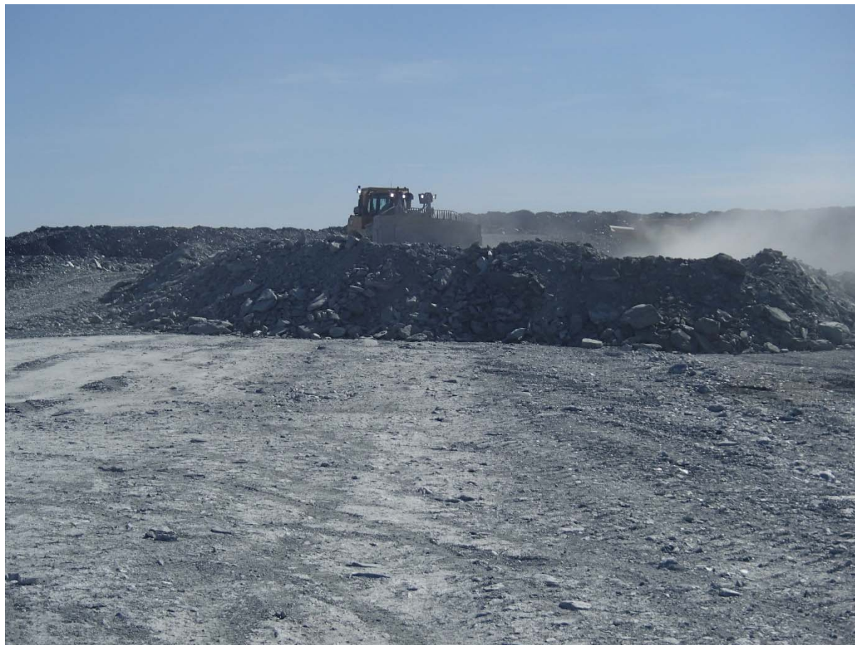
Photograph NCIS-098: From Sta. 2+040/-9 m (approx.), looking E. Placement of a 2 m thick (approx.) lift of UM rockfill from El. 152 m to El. 154 m (approx.) with a dozer from Sta. 2+103 m to 1+984 m (+7 m to -22 m). The material is of good quality and is well graded.
