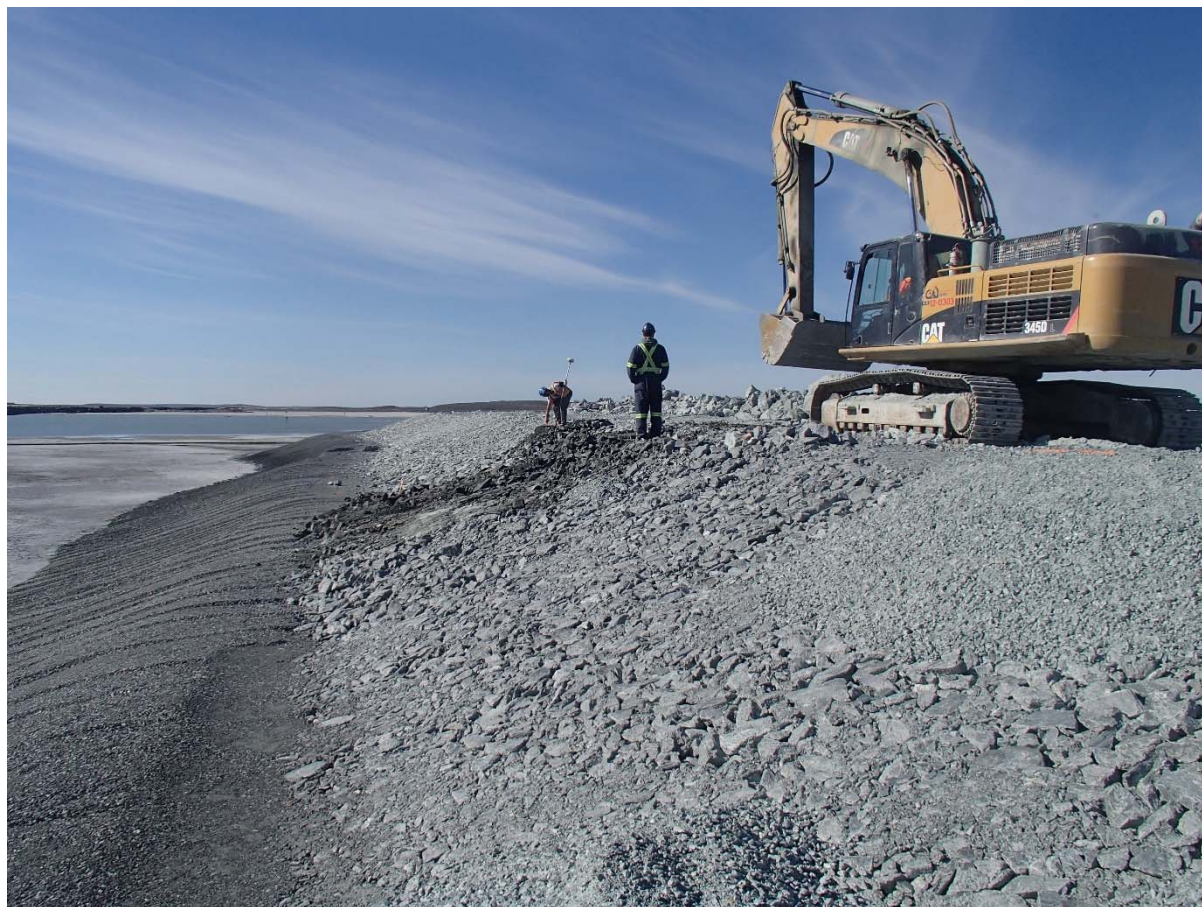
Photograph NCIS-097: From Sta. 1+180/-75 m (approx.), looking SW. Placement of a 0.5 m thick lift of coarse filter in the upstream slope from El. 150 m to 152 m with an excavator from Sta. 1+200 m to 1+113 m.
