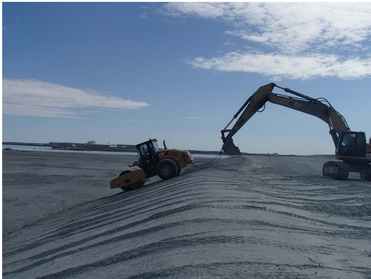
Photograph NCIS-107: From Sta. 1+380/-38 m (approx.), looking S. Compaction of the 0.5 m lift (approx.) of fine filter between El. 150 m and 152 m with a 10-tonne smooth-drum compactor with vibration (4 passes) in the upstream slope from Sta. 1+251 m to 1+660 m.
