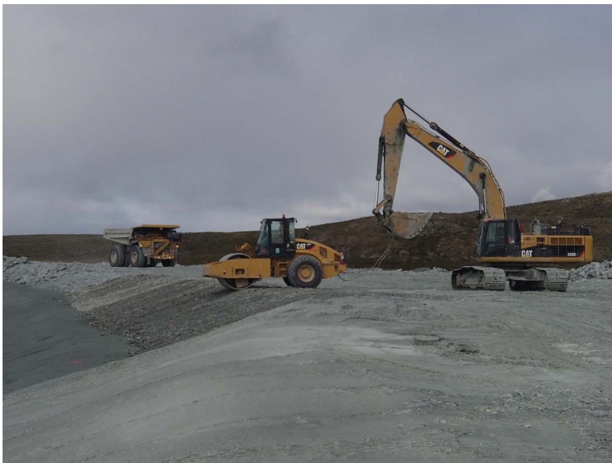
Photograph NCIS-131: From Sta. 1+940/-20 m (approx.), looking W. Compaction of the 0.5 m lift (approx.) of coarse filter between El. 152 m and 154 m with a 10-tonne smooth-drum compactor with vibration (4 passes) in the upstream slope from Sta. 1+890 m to 1+826 m.
