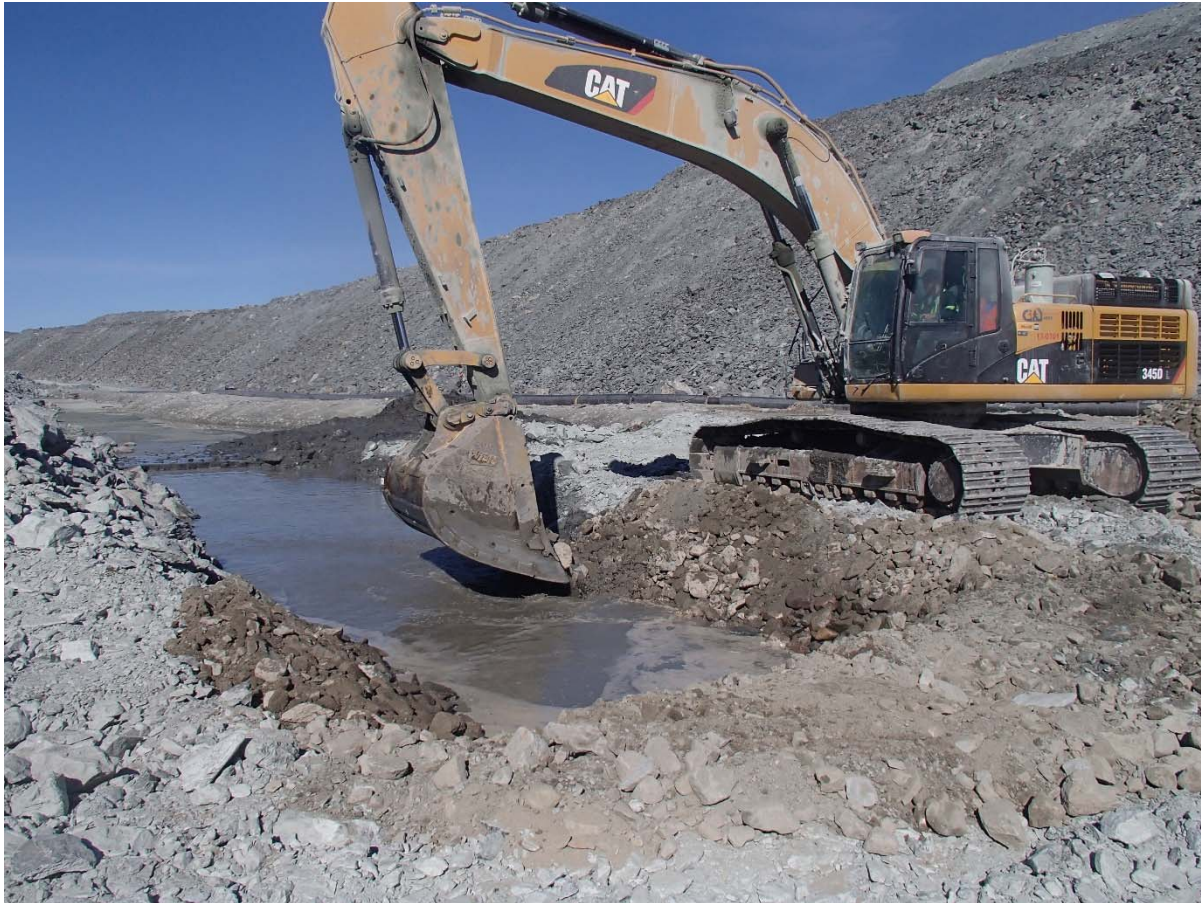
Photograph NCIS-121: From Sta.3+050/+26 m (approx.), looking NE. Placement of a 0.3 m thick (approx.) layer of till sieving reject material on the bottom and on the slopes of the sump.
