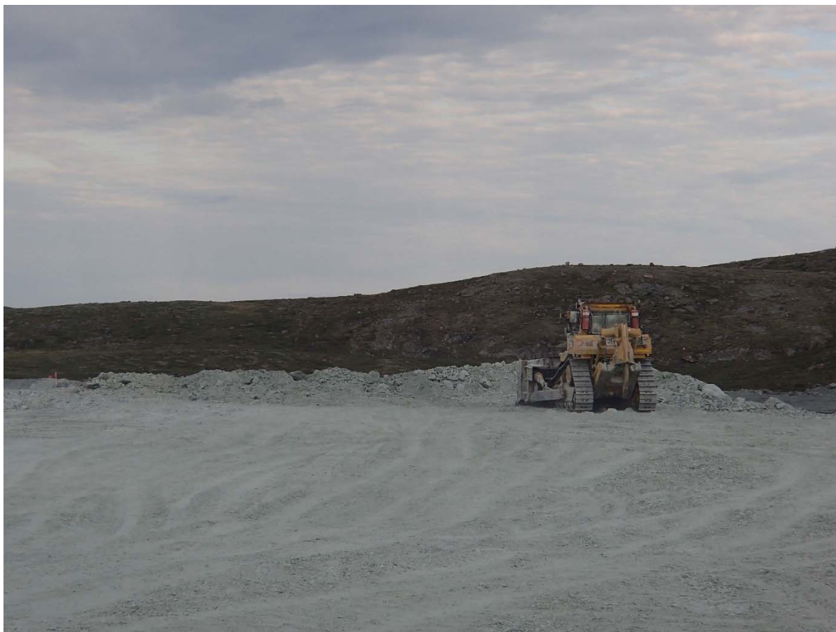
Photograph NCIS-122: From Sta. 1+960/-6 m (approx.), looking W. Placement of a 2 m thick (approx.) lift of UM rockfill from El. 152 m to El. 154 m (approx.) with a dozer from Sta. 1+830 m to 1+860 m (+8 m to -23 m).
