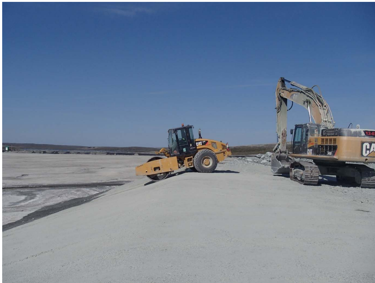
Photograph NCIS-126: From Sta. 1+140/-98 m (approx.), looking W. Compaction of the 0.5 m lift (approx.) of fine filter between El. 150 m and 152 m with a 10-tonne smooth-drum compactor with vibration (4 passes) in the upstream slope from Sta. 1+240 m to 1+100 m.
