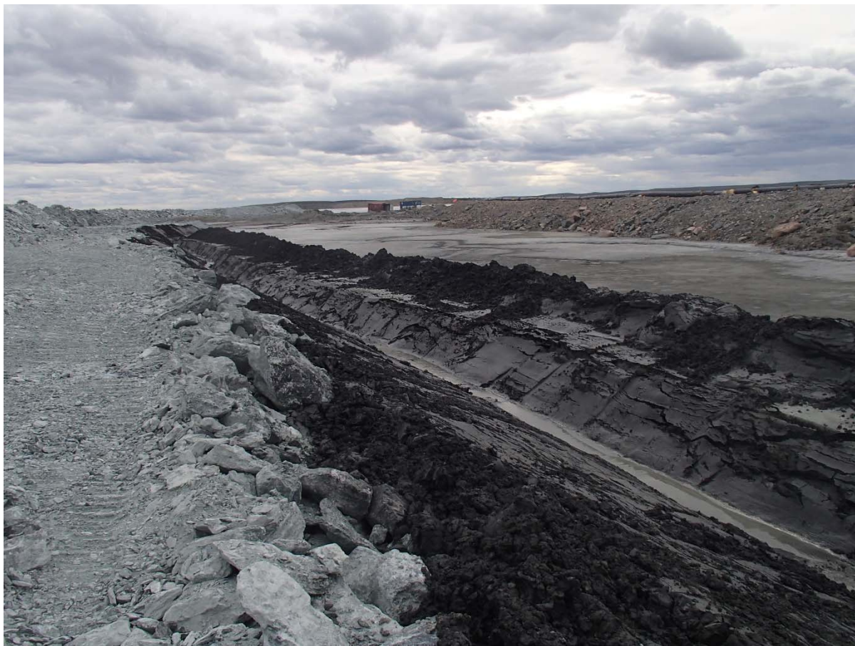
Photograph NCIS-137: From Sta. 1+380/+14 m (approx.), looking SW. Excavation of a 0.8 m (approx.) deep, 1 m wide shallow ditch in the tailings with an excavator from Sta. 1+300 m to 1+200 m.
