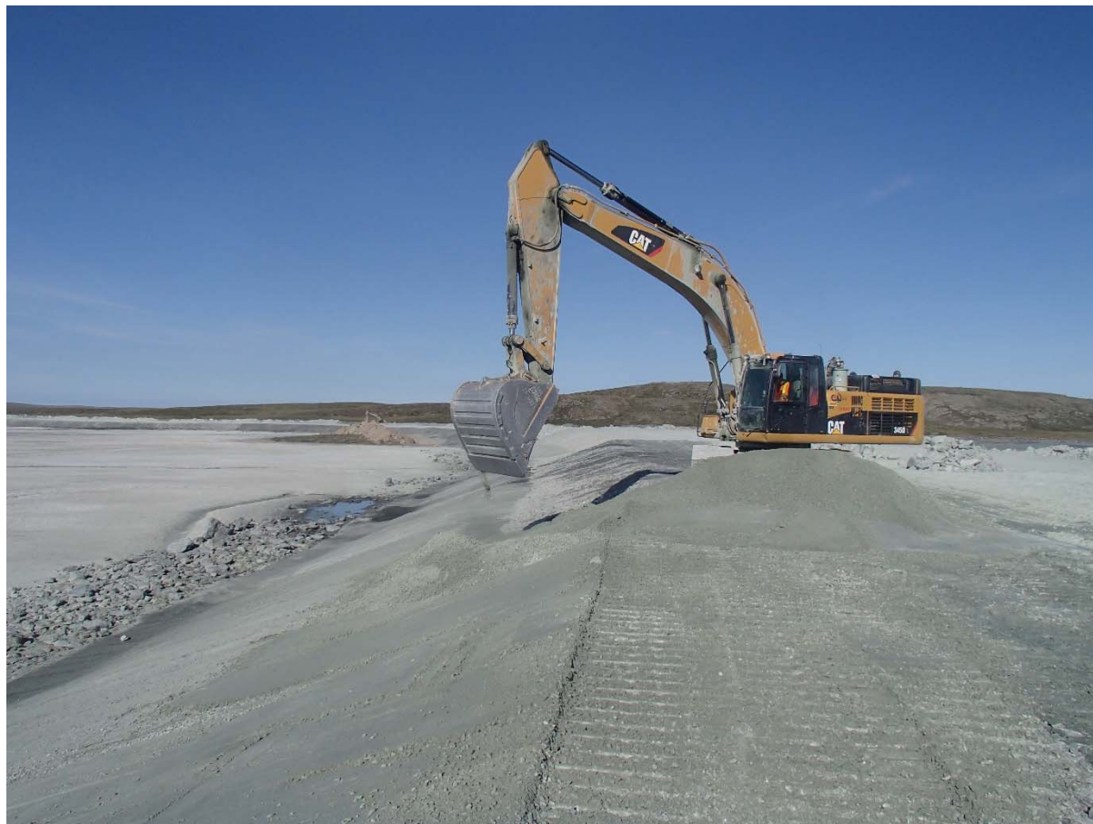
Photograph NCIS-117: From Sta. 2+050/-25 m (approx.), looking SW. Placement of a 0.5 m thick lift of fine filter in the upstream slope from El. 152 m to 154 m with an excavator from Sta. 2+090 m to 1+890 m.
