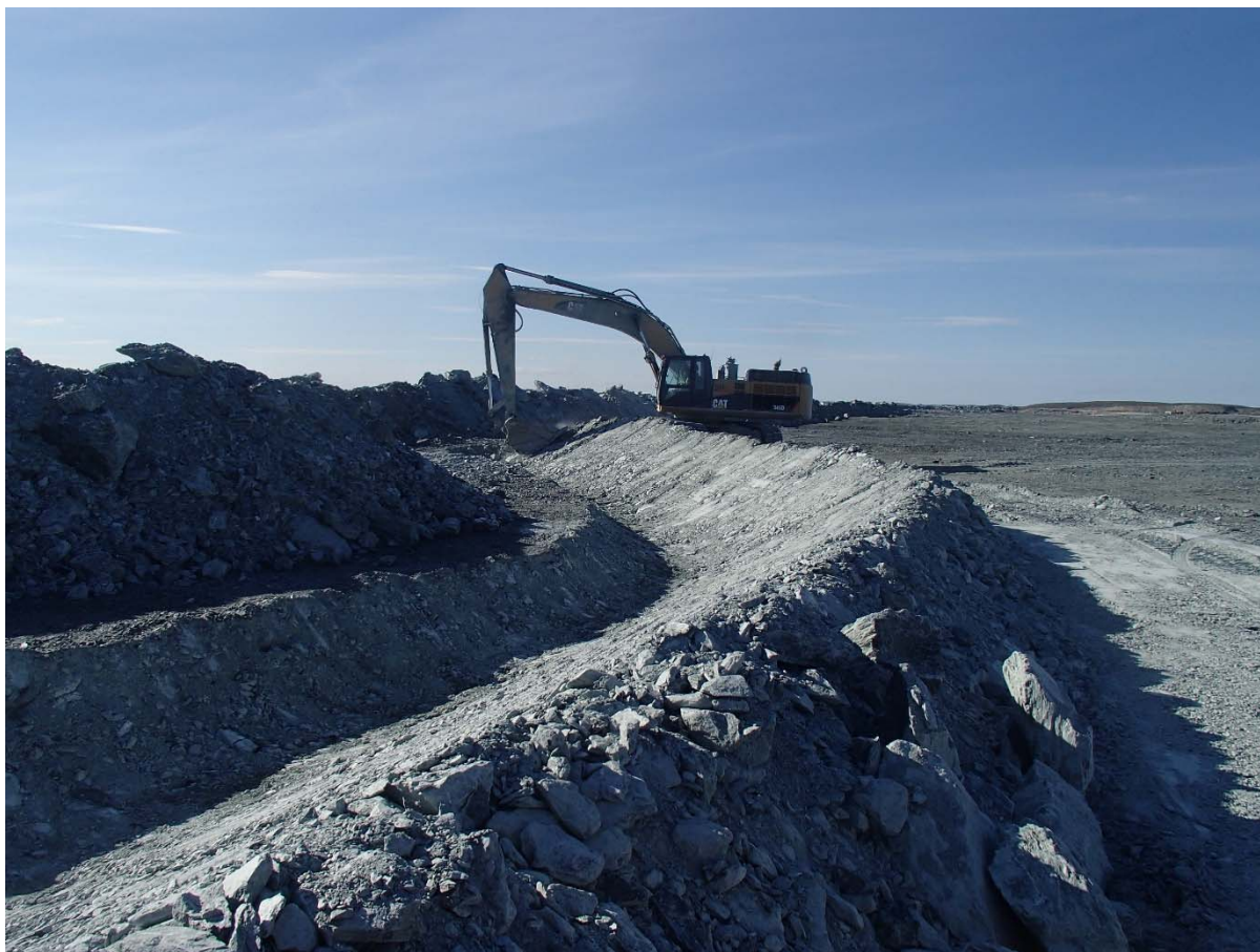
Photograph NCIS-116: From Sta. 1+700/+37 m (approx.), looking SE. Excavation of a 0.8 m (approx.) deep, 1 m wide shallow ditch in the rockfill capping with an excavator from Sta. 1+500 m to 1+455 m.
