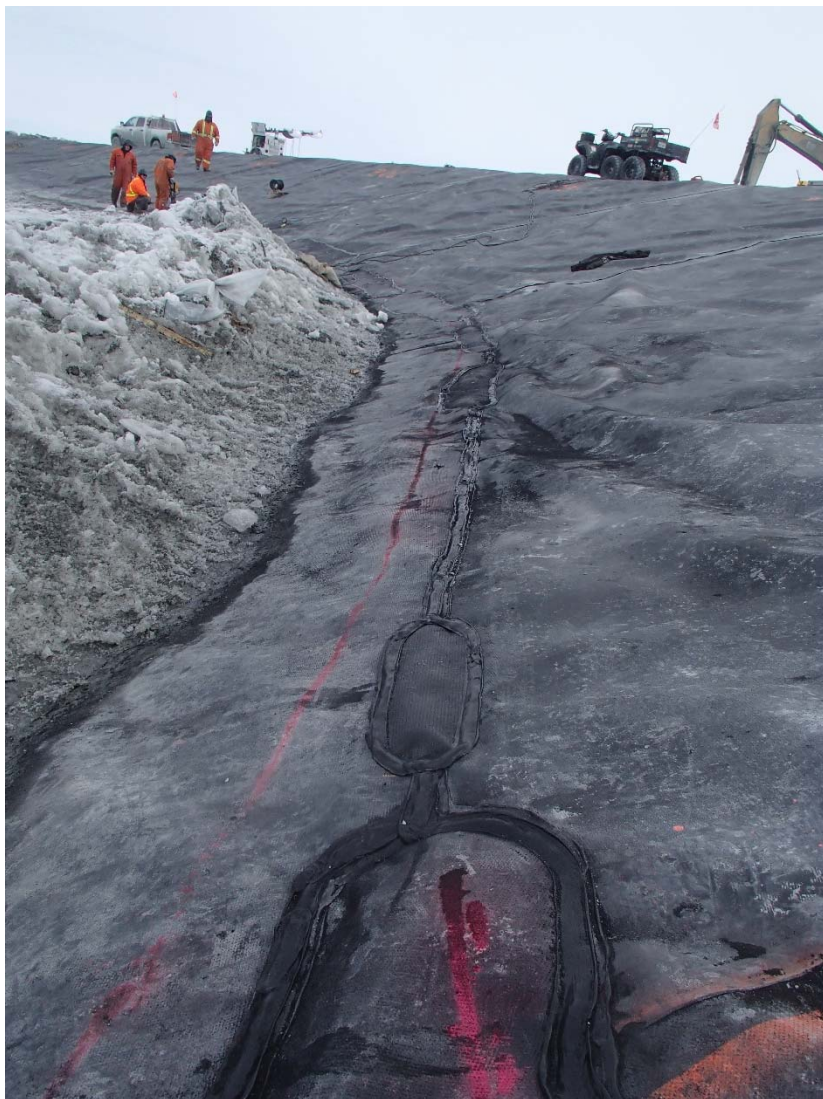
Photograph CD-1867: From Sta. 40+680/-37 m, looking E. View of repair patches on the extrusion weld at the bottom of the panels.
