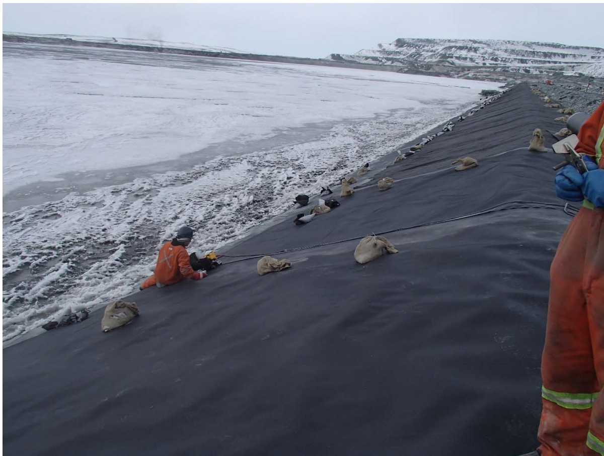
Photograph CD-1866: From Sta. 0+940/-25 m, looking NW. Installation of the LLDPE liner on the upstream slope 2H:1V between El. 143 m and 145 m from Sta. 0+950 m to 0+935 m (panel numbers 818 and 819).
