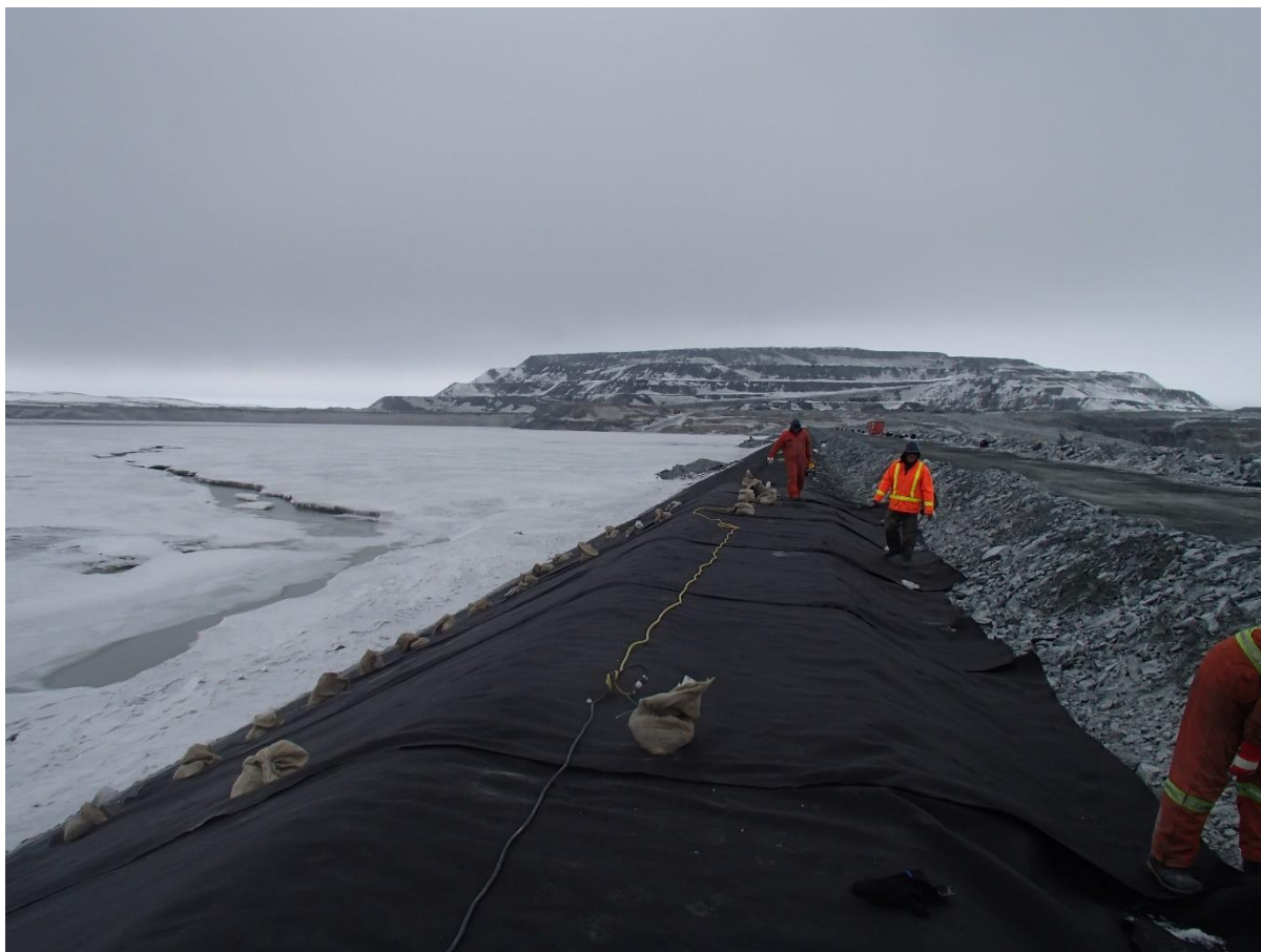
Photograph CD-1873: From Sta. 0+760/-26 m, looking N. Installation of the geotextile on the upstream slope 2H:1V between El. 143 m and 145 m from Sta. 0+760 m to 0+740 m.
