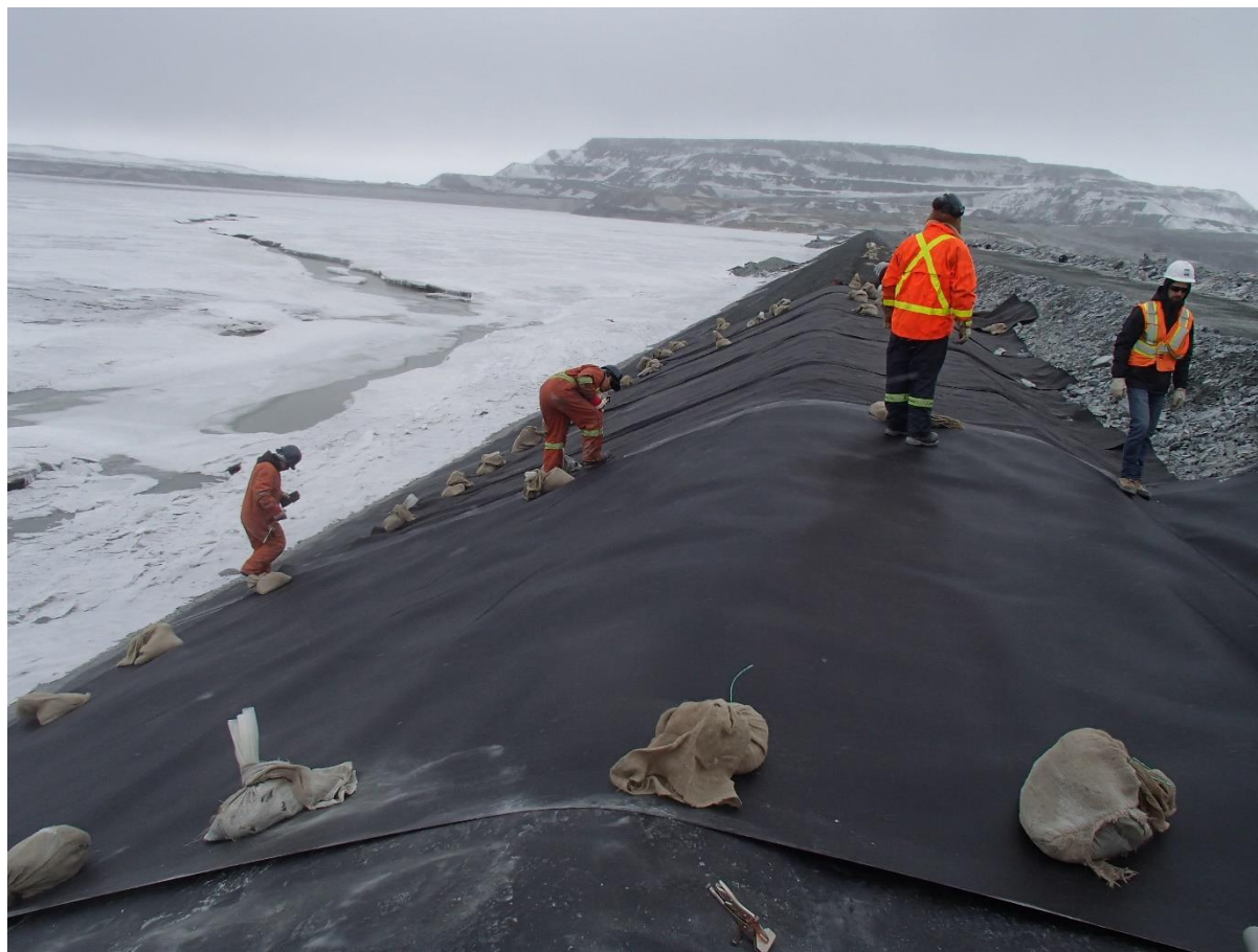
Photograph CD-1874: From Sta. 0+760/-26 m, looking N. Installation of the geotextile on the upstream slope 2H:1V between El. 143 m and 145 m from Sta. 0+760 m to 0+740 m.
