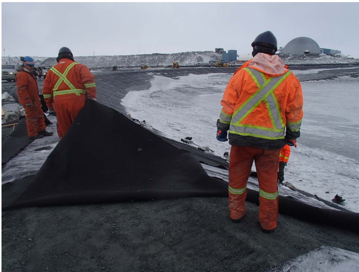
Photograph CD-1868: From Sta. 0+915/-24 m, looking S. Removal of the wet geotextile in place from Sta. 0+935 m to 0+900 m.
