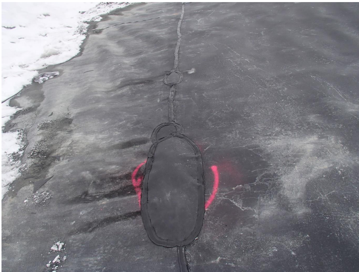
Photograph CD-1876: From Sta. 0+820/-26 m, looking N. View of repair patches on the extrusion weld at the bottom of panel 838.
