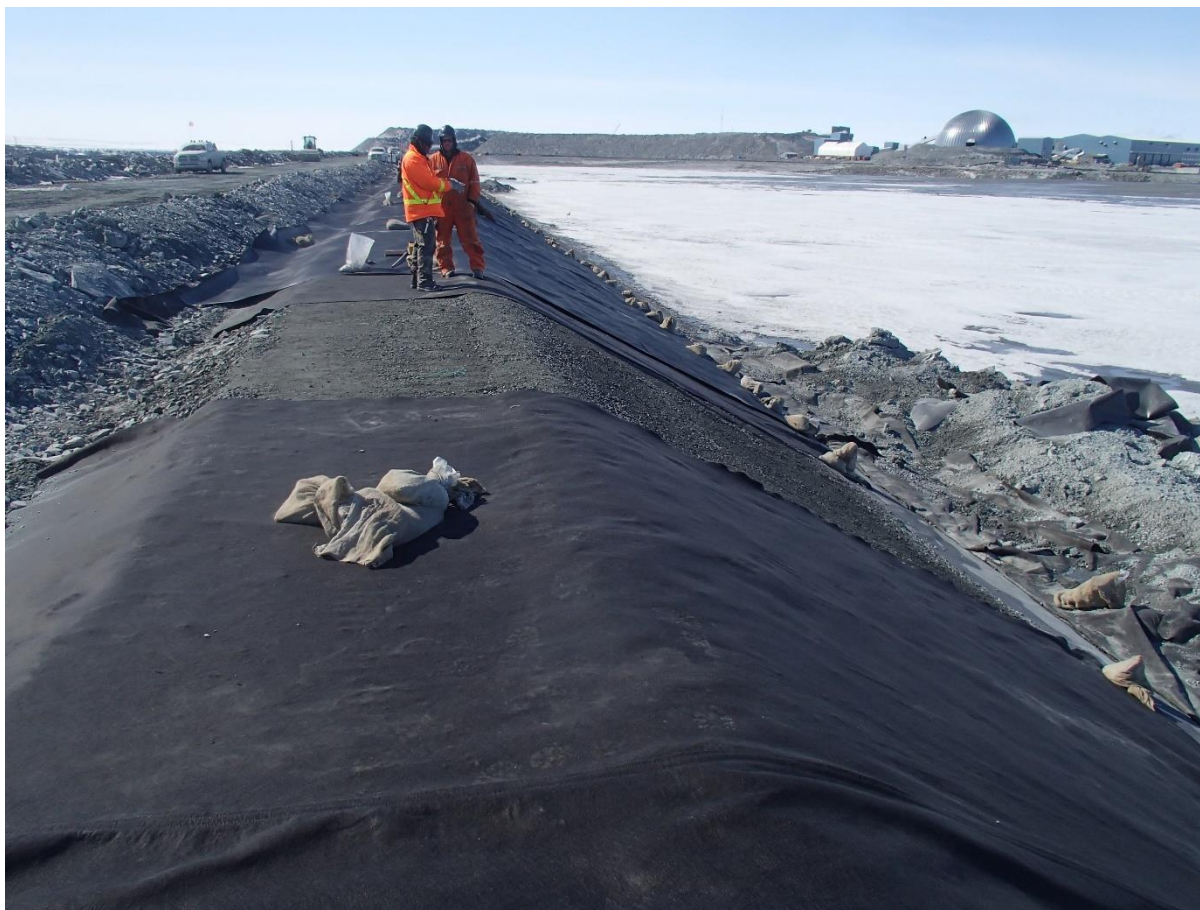
Photograph CD-1882: From Sta. 0+510/-25 m, looking S. View of the emplacement of the geotextile panel with a horizontal weld in the slope at Sta. 0+520 following its removal.
