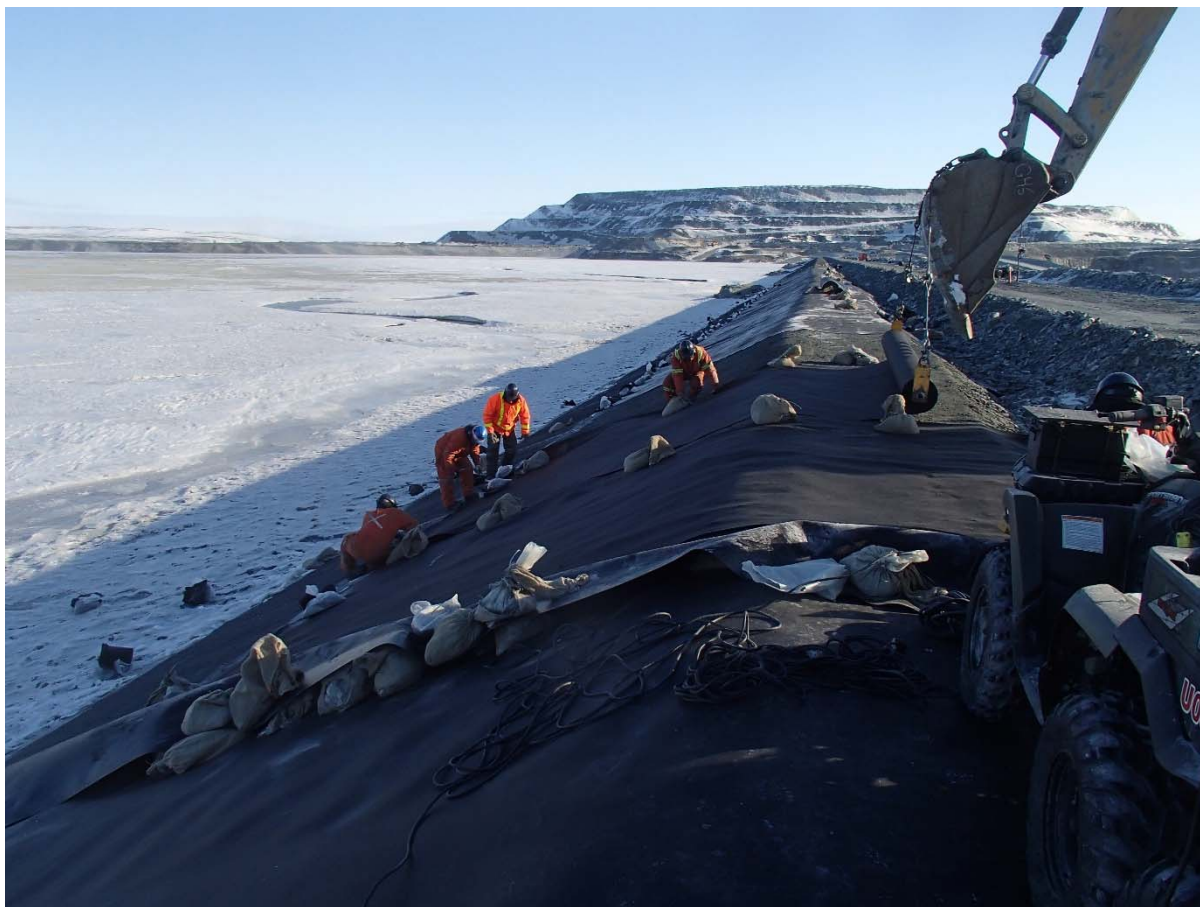
Photograph CD-1871: From Sta. 0+910/-25 m, looking N. Installation of the geotextile on the upstream slope 2H:1V between El. 143 m and 145 m from Sta. 0+900 m to 0+870 m.
