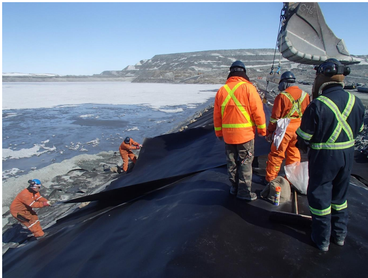
Photograph CD-1883: From Sta. 0+525/-26 m, looking N. Installation of the LLDPE liner on the upstream slope 2H:1V between El. 143 m and 145 m from Sta. 0+610 m to 0+480 m (panel numbers 868 to 886).
