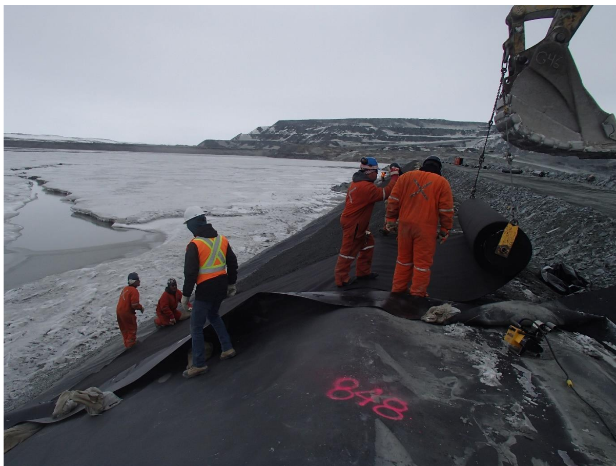
Photograph CD-1877: From Sta. 0+745/-26 m, looking N. Installation of the geotextile on the upstream slope 2H:1V between El. 143 m and 145 m from Sta. 0+740 m to 0+610 m.
