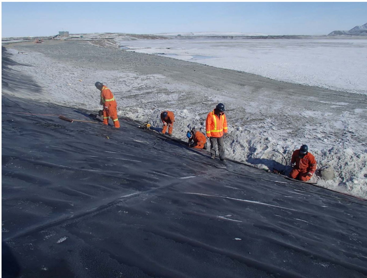
Photograph CD-1865: From Sta. 40+740/-35 m, looking NW. Repairs on the extrusion fillet seam at the bottom of the LLDPE liner panels between Sta. 40+680 m and 0+950 m, on panels 802 to 807, and 811 to 813.
