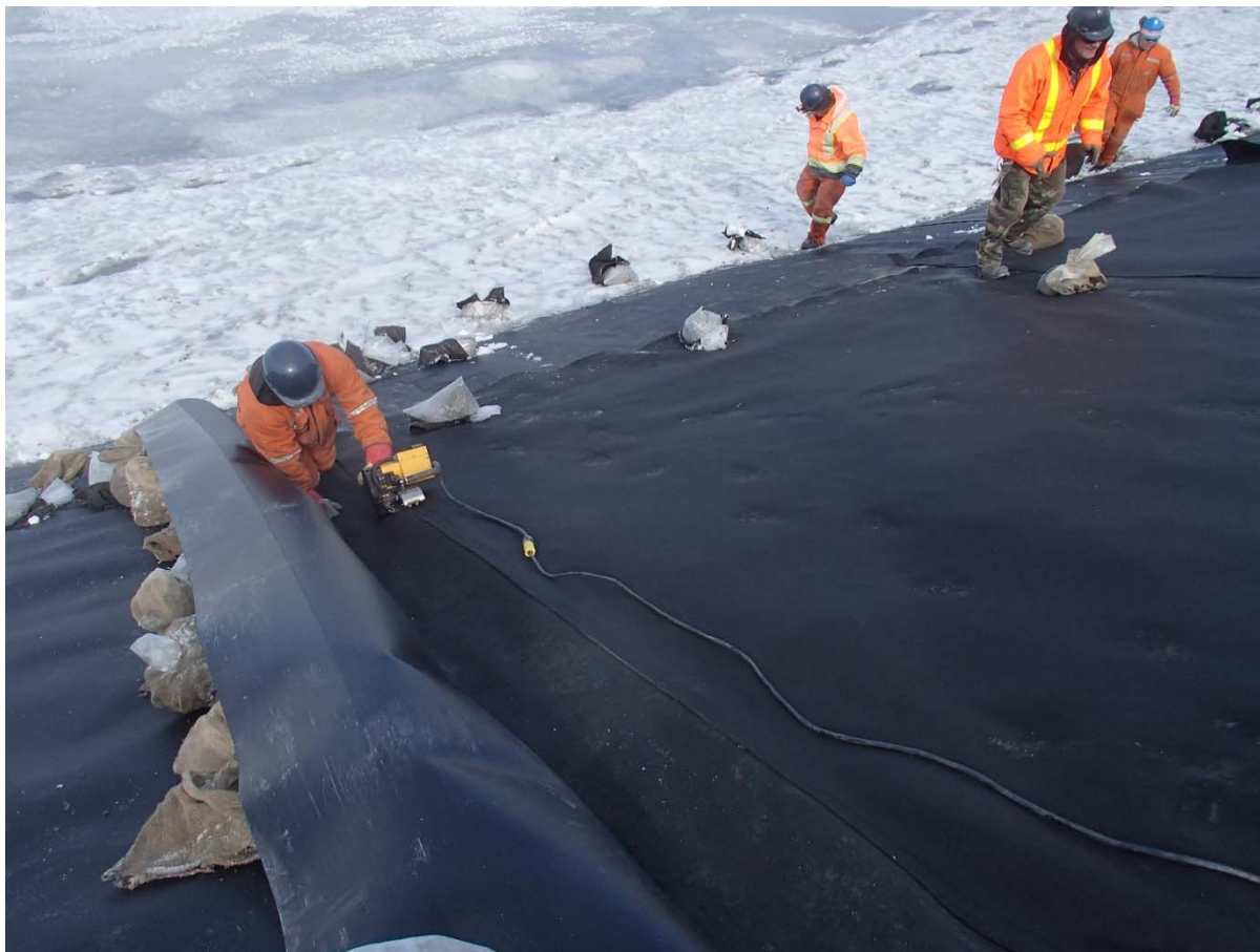
Photograph CD-1869: From Sta. 0+915/-30 m, looking W. Installation of the geotextile on the upstream slope 2H:1V between El. 143 m and 145 m from Sta. 0+935 m to 0+900 m.
