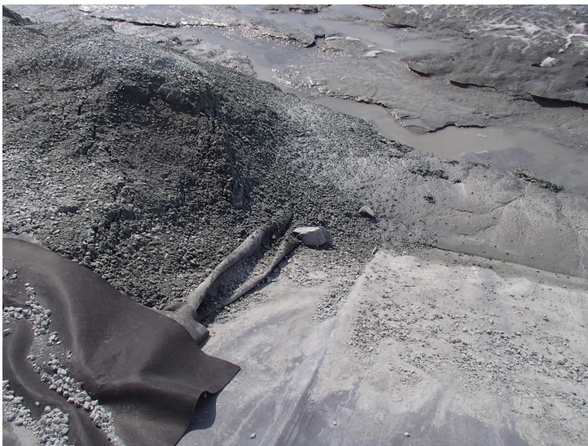
Photograph CD-1894: From Sta. 0+800/-28 m, looking E. View of a bloc in direct contact with the LLDPE liner following the construction of the deposition fingers on Central Dike.
