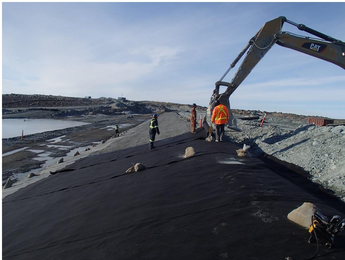
Photograph SD-310: From Sta. 20+635/-24 m, looking S. Installation of the geotextile on the upstream slope 2H:1V between El. 143 m and 145 m from Sta. 20+630 m to 20+800 m.
