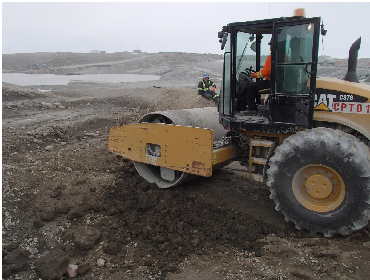
Photograph SD3-313: From Sta. 20+600/-52 m, looking S. Compaction of the 0.15 m-thick lift of compacted sieved till with a 10-tonne smooth-drum compactor without vibration from Sta. 20+596 m to 20+601 m.
