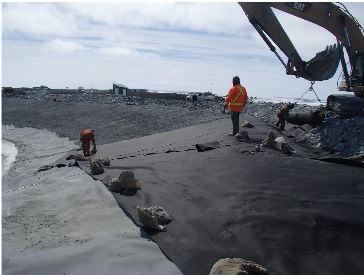
Photograph SD-308: From Sta. 20+620/-48 m, looking SW. Installation of the geotextile on the upstream slope 2H:1V between El. 143 m and 145 m from Sta. 20+620 m to 20+630 m.
