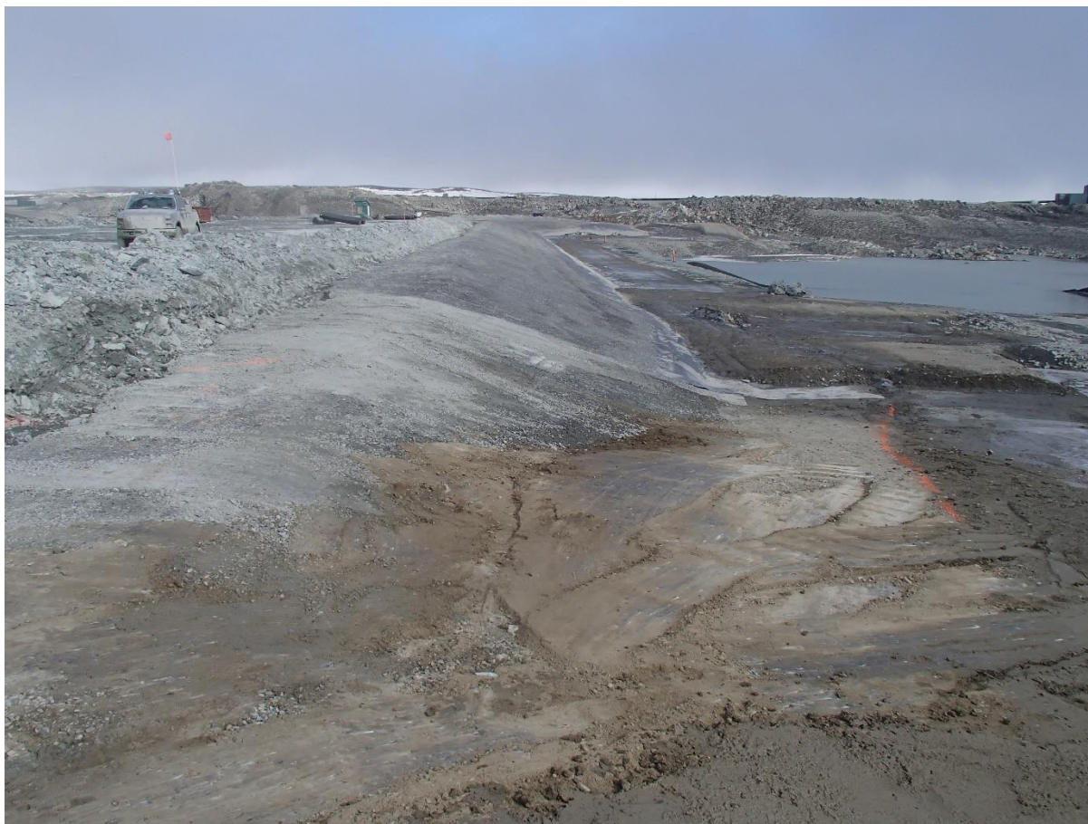
Photograph SD3-307: From Sta. 20+800/-25 m, looking N. View of the liner bedding ready for geosynthetics installation.
