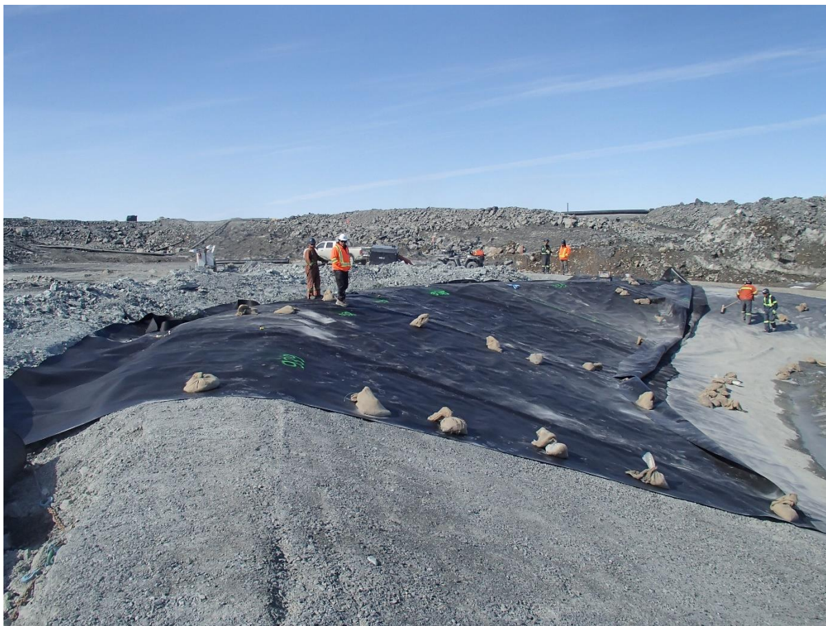
Photograph SD-309: From Sta. 20+640/-26 m, looking N. Installation of the LLDPE liner on the upstream slope 2H:1V between El. 143 m and 145 m from Sta. 20+620 m to 20+630 m (panel numbers 934 to 939).
