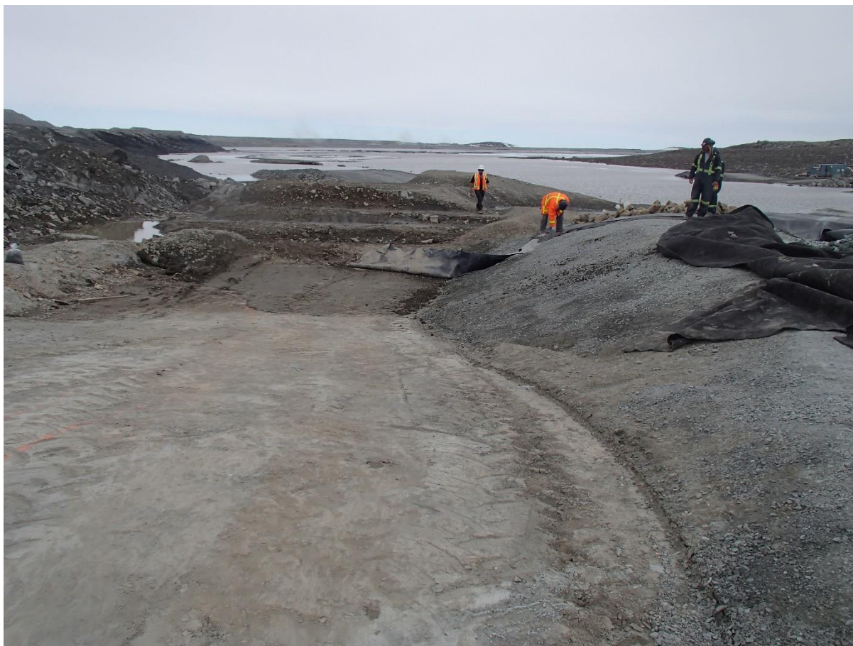
Photograph SD3-314: From Sta. 20+590/-32 m, looking E. View of the liner bedding ready for geosynthetics installation.
