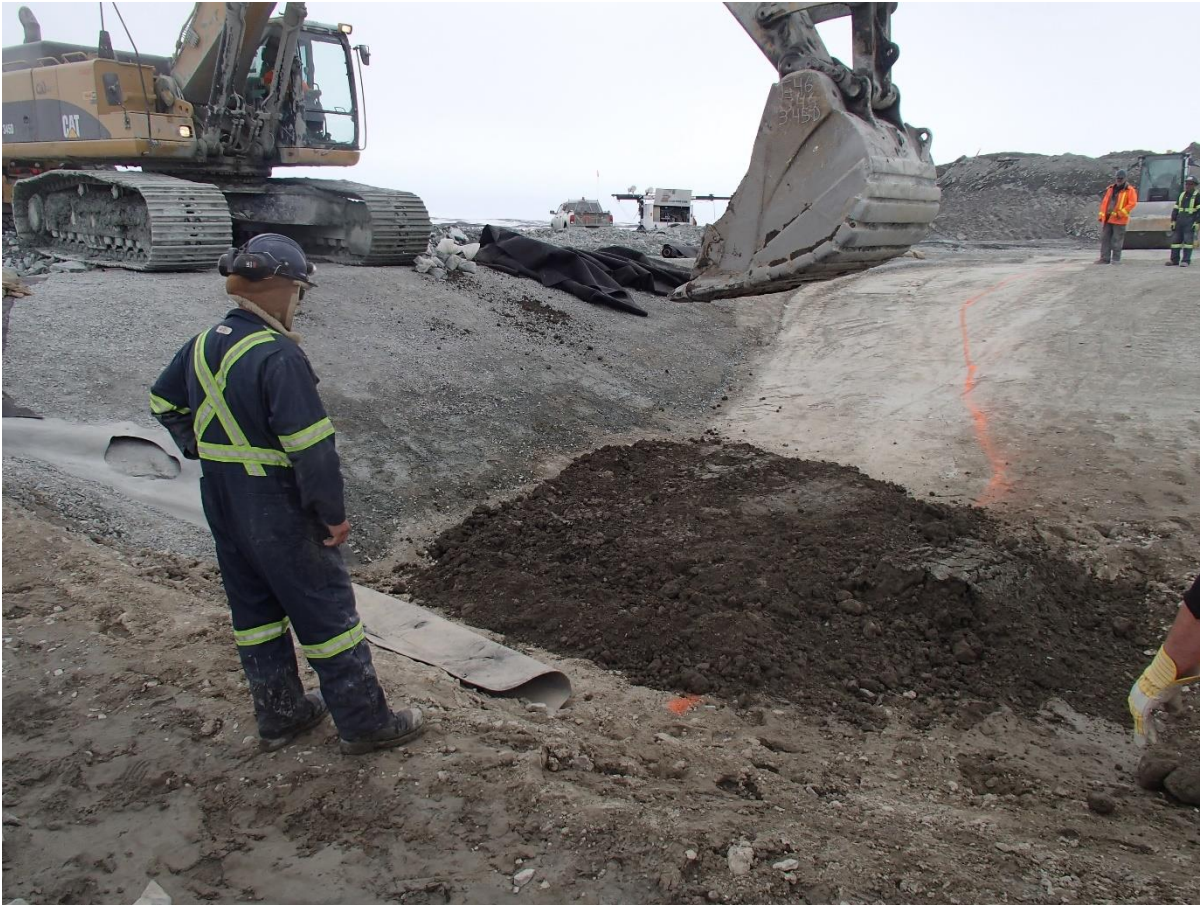
Photograph SD3-312: From Sta. 20+610/-48 m, looking W. Placement of a 0.15 m thick lift of compacted sieved till from Sta. 20+596.4 m to 20+601.6 m (o.s. -42.6 to -46.3 m) to fill the depression in the compacted sieved till layer.
