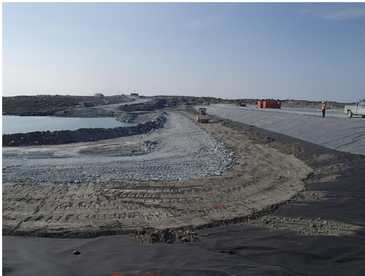
Photograph SD3-327: From Sta. 20+610/-43 m, looking S. Compaction of the 0.5 m lift of low quality till (0-150 mm) at El. 142.5 m with a 10-tonne smooth-drum compactor with vibration (4 passes) from Sta. 20+610 m to 20+615 m and from Sta. 20+635 m to 20+760 m.
