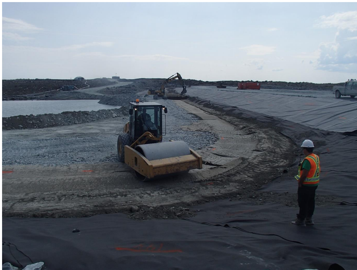
Photograph SD3-328: From Sta. 20+610/-43 m, looking S. Compaction perpendicularly to the longitudinal axis of Saddle Dam 3 of the 0.5 m lift of low quality till (0-150 mm) at El. 142.5 m with a 10-tonne smooth-drum compactor without vibration (4 passes) from Sta. 20+615m to 20+635 m.
