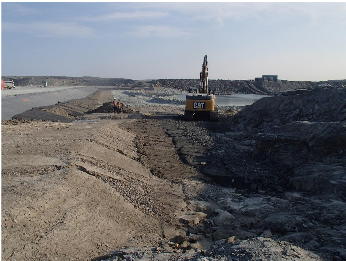
Photograph SD3-326: From Sta. 20+820/-34 m, looking N. Placement of the 0.5 m thick lift of low class till, fine filter, coarse filter and fine rockfill on the upstream slope of the upstream toe liner tie-in with an excavator from Sta. 20+780 to 20+810 m.
