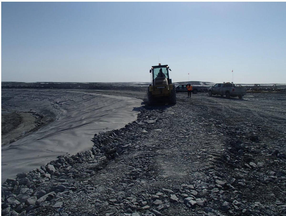
Photograph CD-1895: From Sta. 40+670/-15 m, looking E. Compaction of the geosynthetics tie-in material at El. 145 m with a 10-tonne smooth-drum compactor with vibration (4 passes) from Sta. 40+670 m to 0+950 m (approx.).
