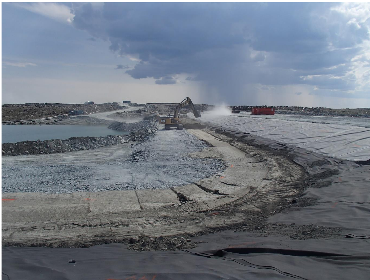
Photograph SD3-329: From Sta. 20+610/-43 m, looking S. Placement of a 0.5 m thick lift of low quality till (0-150 mm) from El. 142.5 m to 143 m from Sta. 20+610 m to 20+760 m.
