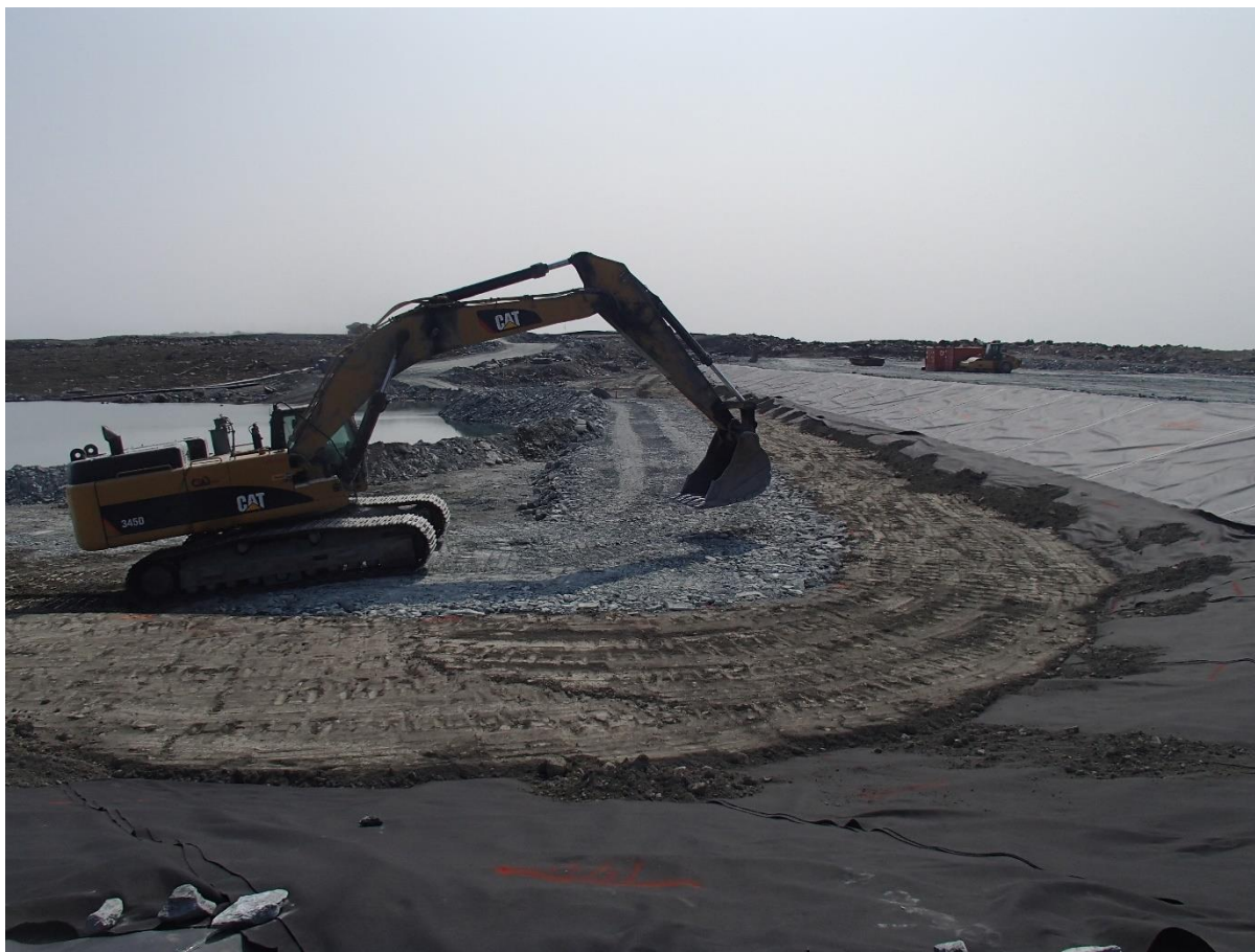
Photograph SD3-325: From Sta. 20+610/-43 m, looking S. Placement of a first 0.5 m thick lift of fine rockfill (0-500 mm) upstream of the low quality till from El. 142 m to 142.5 m from Sta. 20+610 m to 20+760 m.
