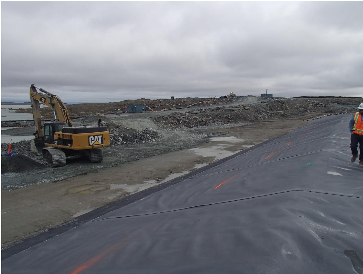
Photograph SD3-318: From Sta. 20+710/-24 m, looking SE. Placement of IV rockfill in the water up to El. 142m with an excavator from Sta. 20+785 m to 20+730 m, at the bottom of the upstream slope of SD3 to widen the rockfill layer and allow access to the erosion protection.
