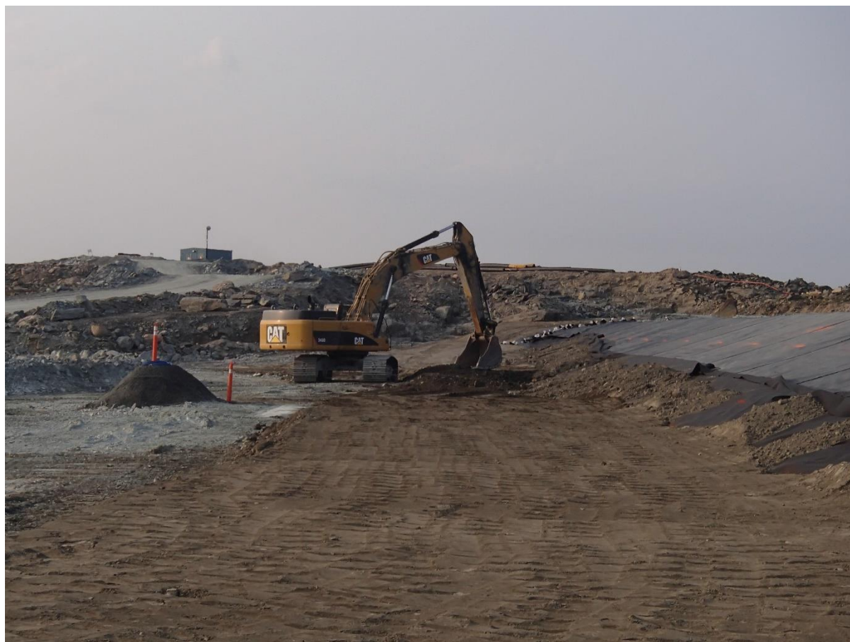
Photograph SD3-324: From Sta. 20+680/-39m, looking S. Placement of a 0.5 m thick lift of low quality till (0-150 mm) from El. 142 m to 142.5 m from Sta. 20+715 m to 20+760 m.
