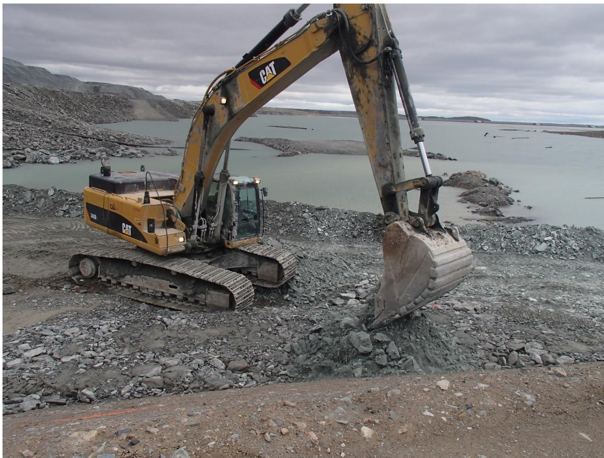
Photograph SD3-320: From Sta. 20+620/-67 m, looking E. Placement of a 1 m thick (approx.) lift of fine IV rockfill over the compacted till in the upstream slope from El. 142 m to 144 m with an excavator from Sta. 20+600 m to 20+610 m.
