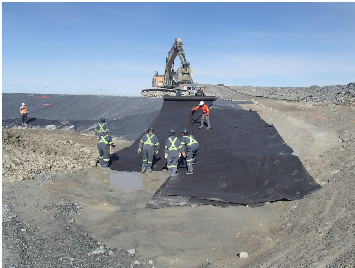
Photograph SD3-322: From Sta. 20+625/-63 m, looking W. Installation of two layers of geotextile on the upstream slope 3H:1V between El. 142 m and 143 m (approx.) from Sta. 20+610 m to 20+800 m.
