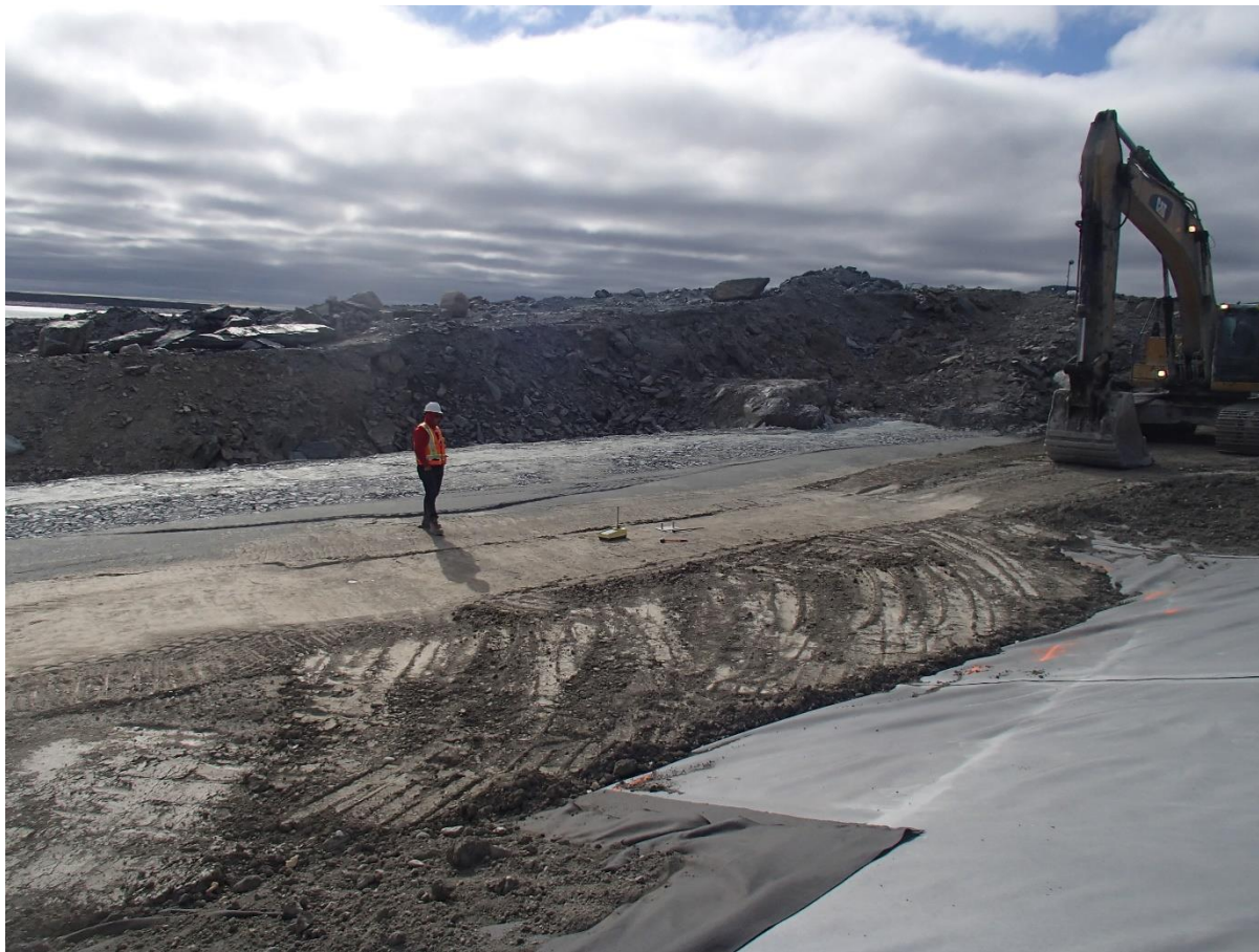
Photograph SD3-334: From Sta. 20+780/-26 m, looking SE. Compaction of the second 0.5 m thick lift of compacted sieved till and third lift of fine filter, coarse filter and fine rockfill of the upstream toe liner tie-in with a 10 tonne smooth-drum compactor with vibrations from Sta. 20+770 m to 20+800 m.
