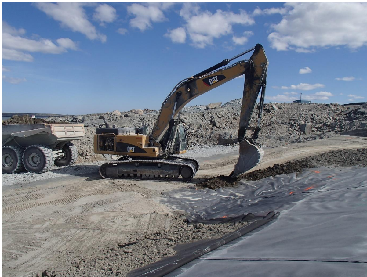
Photograph SD3-332: From Sta. 20+775/-23 m, looking SE. Placement of a first 0.5 m thick lift of compacted sieved till over the LLDPE geomembrane on the upstream toe liner tie-in with an excavator from Sta. 20+775 m to 20+800 m.
