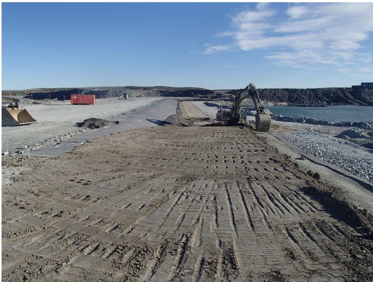
Photograph SD3-335: From Sta. 20+815/-27 m, looking N. Placement of a third 0.5 m thick lift of compacted sieved till on the upstream toe liner tie-in with an excavator from Sta. 20+760 m to 20+810 m.
