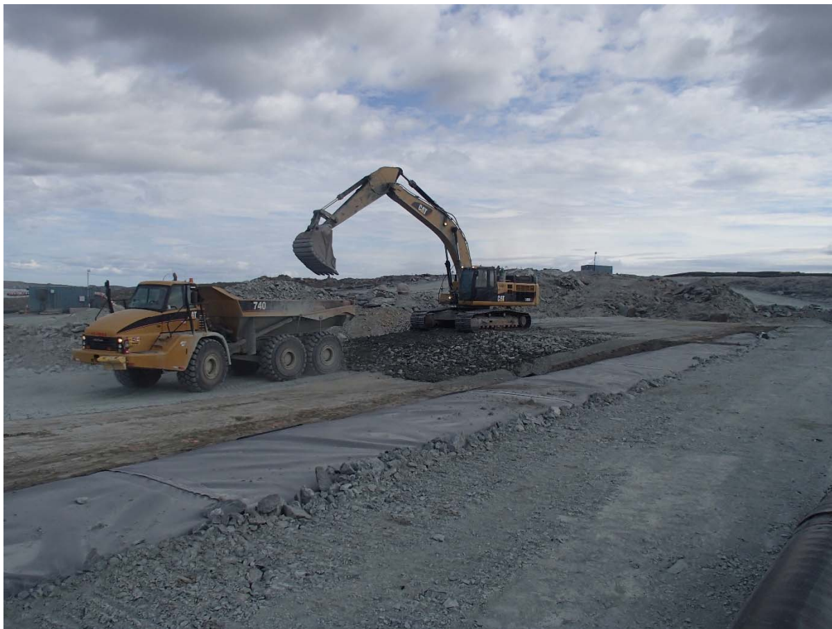
Photograph SD3-350: From Sta. 20+740/-24 m, looking SE. Placement of a 0.5 m thick lift of coarse filter on the top of the fine filter on the upstream toe liner tie-in with an excavator from Sta. 20+777 m to 20+807 m.
