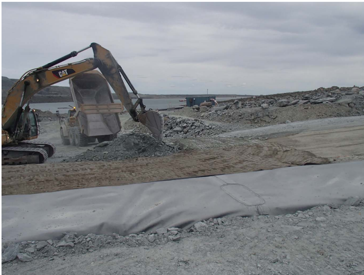
Photograph SD3-346: From Sta. 20+760/-21 m, looking E. Placement of a third 0.5 m thick lift of fine UM rockfill (0-500 mm) upstream of the low quality till (0-150mm) from El. 143 m to 143.5 m from Sta. 20+668 m to 20+777 m.
