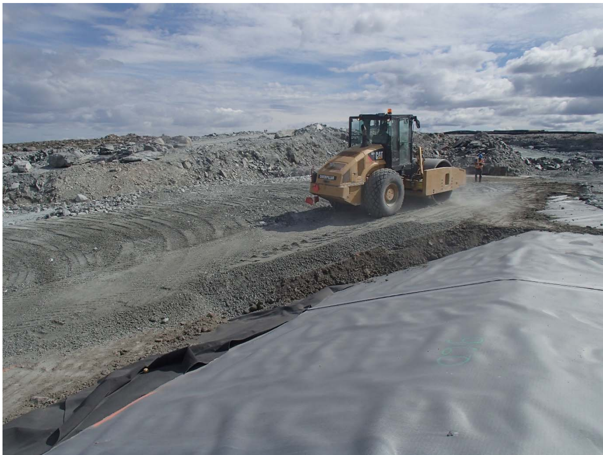
Photograph SD3-349: From Sta. 20+765/-29 m, looking SE. Compaction of the 0.5 m thick lift of fine filter on the top of the upstream toe liner tie-in with a 10 tonne smooth-drum compactor with vibration (4 passes) from Sta. 20+777 m to 20+807 m.
