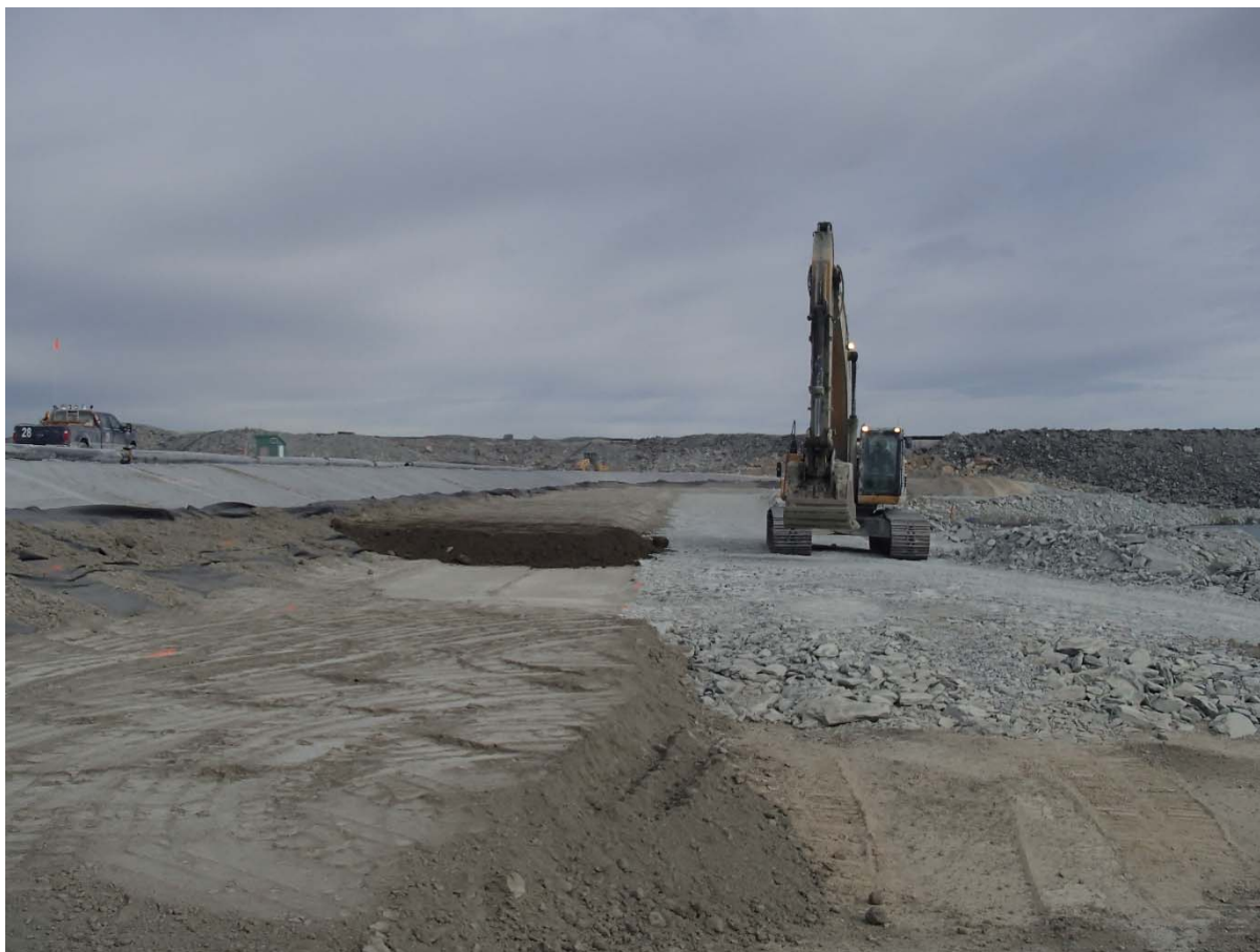
Photograph SD3-345: From Sta. 20+760/-42 m, looking NW. Placement of a fourth 0.5 m thick lift of low quality till (0-150 mm) from El. 143 m to 143.5 m from Sta. 20+619 m to 20+777 m.
