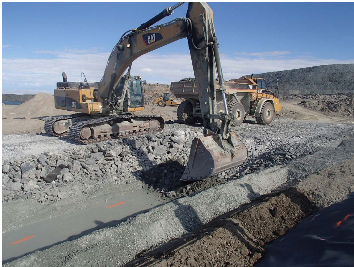
Photograph CD-1897: From Sta. 0+145/-30 m, looking NW. Placement of a 0.5 m thick lift of coarse filter on the top of the fine filter on the top of the upstream toe liner tie-in and on the upstream slope with an excavator from Sta. 0+147 m to 0+177 m.
