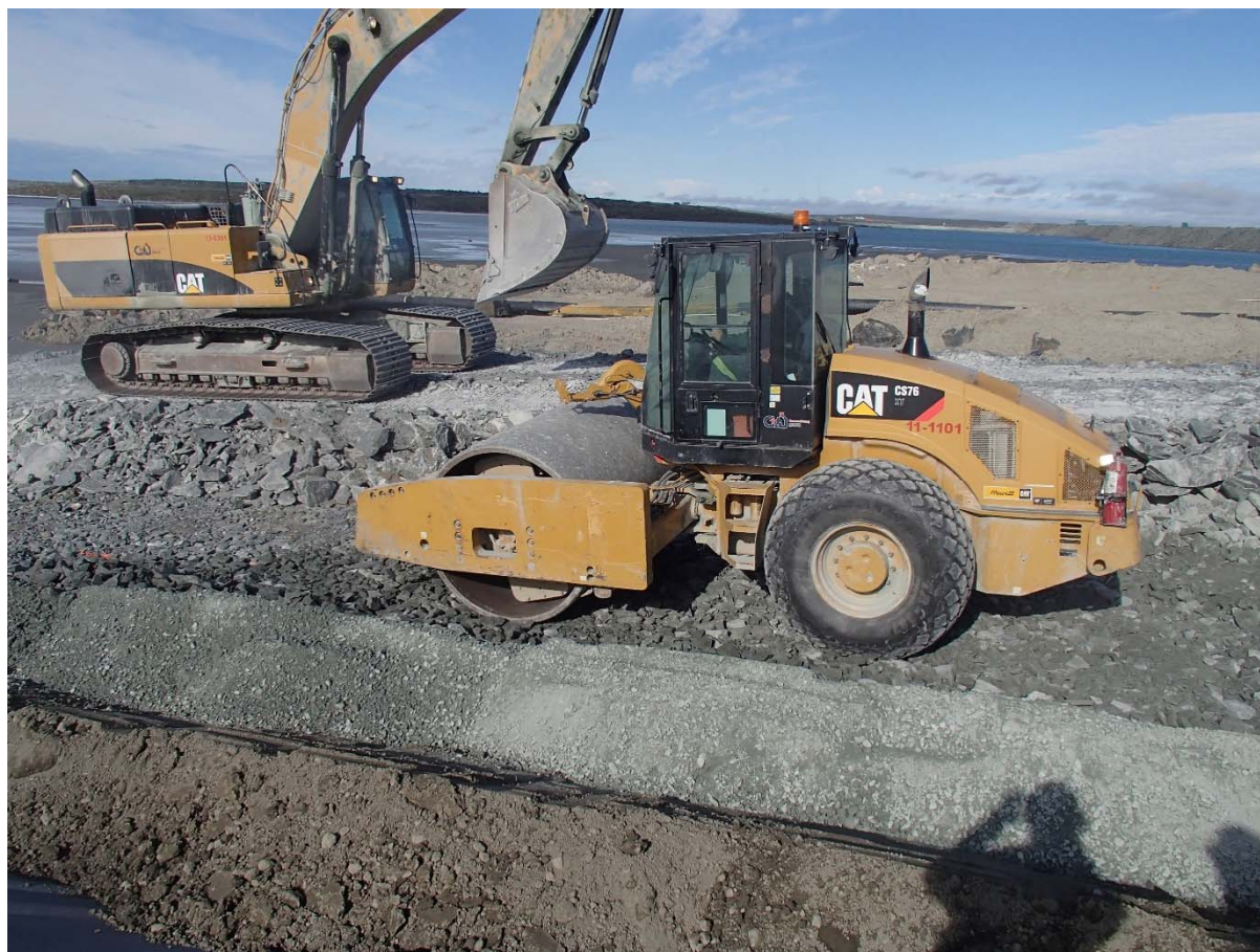
Photograph CD-1898: From Sta. 0+145/-30 m, looking W. Compaction of the 0.5 m thick lift of coarse filter on the top of the fine filter on the top of the upstream toe liner tie-in and on the upstream slope with a 10 tonne smooth-drum compactor with vibration (4 passes) from Sta. 0+147 m to 0+177 m.
