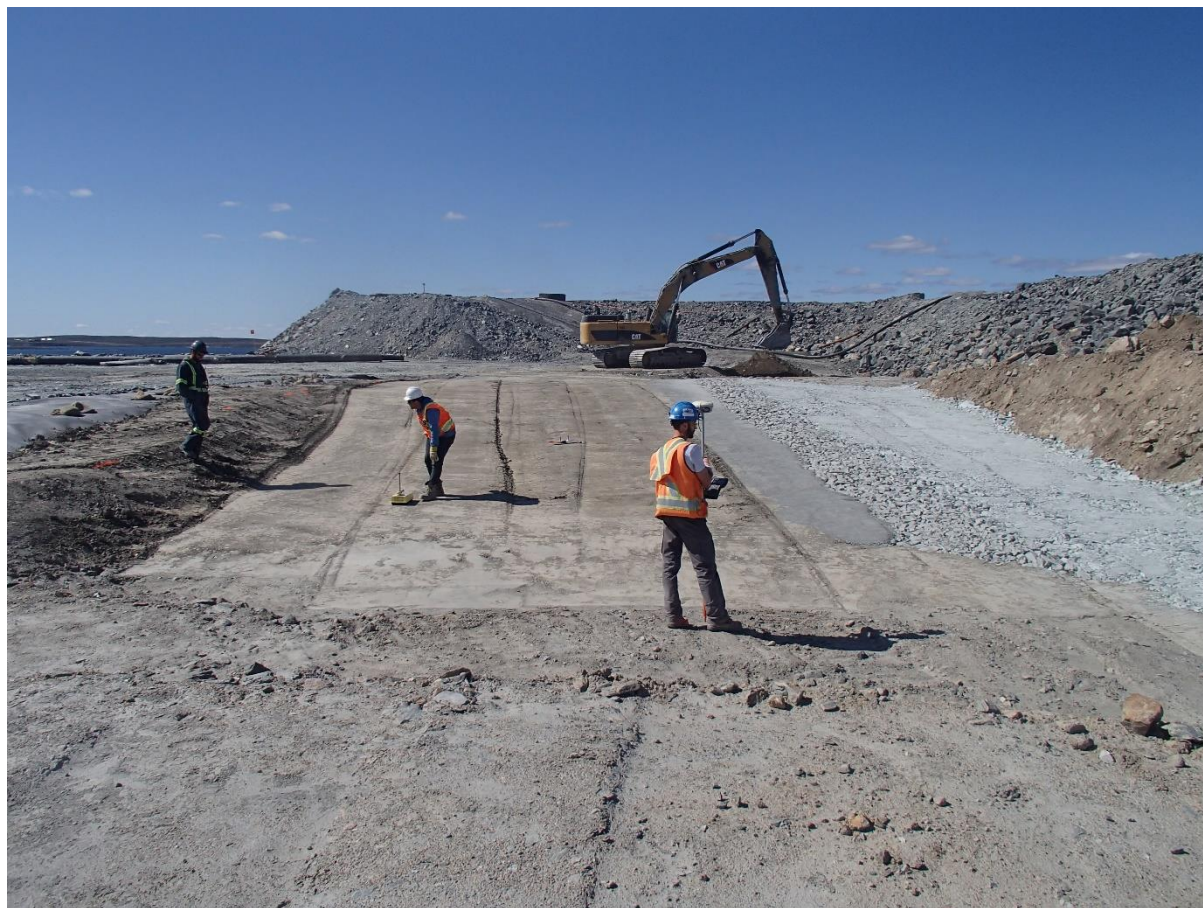
Photograph SD3-342: From Sta. 20+600/-57 m, looking W. View of the compaction test and view of the filling of the depression between SD2 and SD3 with low quality till up to El. 145 m.
