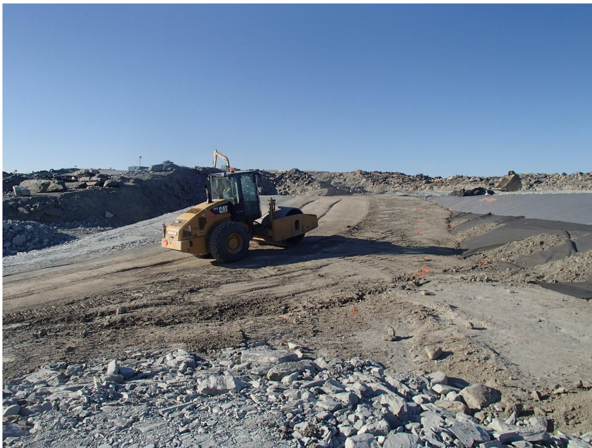
Photograph SD3-340: From Sta. 20+750/-40 m, looking S. Compaction of the third 0.5 m thick lift of compacted sieved till on the upstream toe liner tie-in with an excavator from Sta. 20+760 m to 20+820 m.
