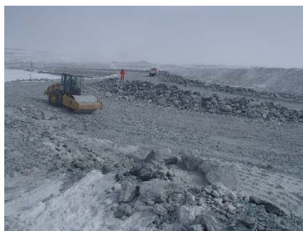
CD-1823 (2018-05-04), looking NE from Sta. 40+725/+8 m. Compaction of the two 2 m lifts (approx.) of intermediate volcanic (IV) rockfill at El. 143 and at El. 145 m with a 10-tonne smooth-drum compactor with vibration (6 passes) from Sta. 40+720 m to 40+750 m (o.s. -10 to +10 m).
