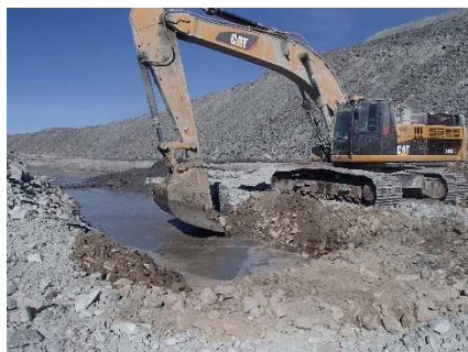
NCIS-121 (2018-07-26), looking NE from Sta. 3+050/+26 m (approx.). Placement of a 0.3 m thick (approx.) layer of till sieving reject material on the bottom and on the slopes of the sump.
