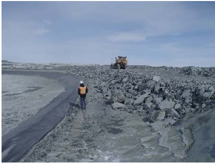
CD-1817 (2018-05-02), looking NE from Sta. 40+700/-10 m. View of the rockfill lift thickness at the junction of Saddle Dam 5 and Central Dike, approx. 2.5 m thick..
