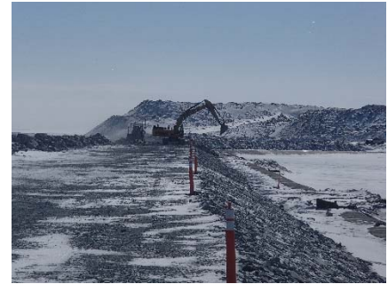
CD-1819 (2018-05-03), looking S from Sta. 0+560/-21 m. Profiling of the upstream slope (2H:1V) from El. 143 to 145 m with an excavator between Sta. 0+560 m and 0+830 m.
