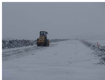
CD-1807 (2018-04-28), looking S from Sta. 0+200/-15 m. Compaction of the 2 m lift (approx.) of IV rockfill with a 10-tonne smooth-drum compactor with vibration (6 passes) from Sta. 0+150 to 0+280 m (o.s. -21 to 11 m).
