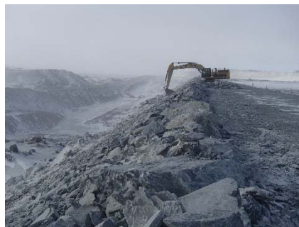
CD-1821 (2018-05-04), looking S from Sta. 0+175/+3 m. Profiling of the downstream slope (1.5H:1V) from El. 143 to 145 m with an excavator between Sta. 0+250 m and 0+330 m.
