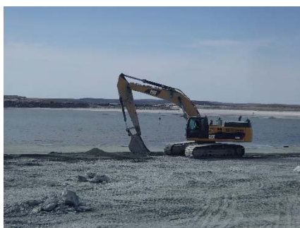
NCIS-068 (2018-07-01), looking S from Sta. 1+150/-62 m. Placement of a 0.5 m thick lift of fine filter over the coarse filter in the upstream slope from El. 148 m to 150 m with an excavator from Sta. 1+180 m to 1+100 m.
