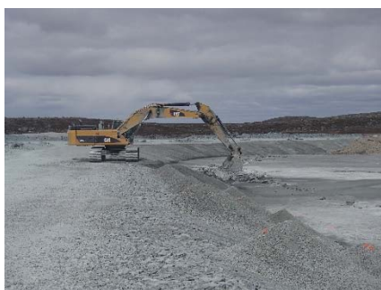
NCIS-062 (2018-06-29), looking N from Sta. 1+525/-33 m. Placement of a 0.5 m thick lift of fine filter over the coarse filter in the upstream slope from El. 150 m to 152 m with an excavator from Sta. 1+330 m to 1+260 m and from Sta. 1+595 m to 1+550 m.
