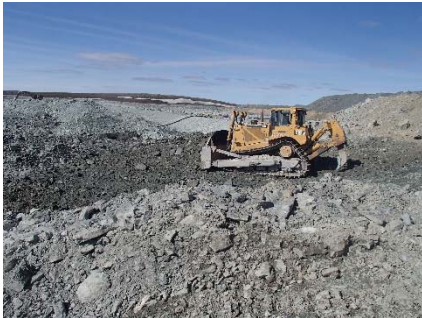
NCIS-049 (2018-06-26), looking N from Sta. 2+870/-28 m. Removing of UM rockfill material from the capping with a dozer to level the surface to El. 150 m from Sta. 2+760 m to 2+850 m (o.s. -29 to -17 m).
