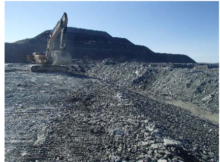
NCIS-051 (2018-06-27), looking SE from Sta. 2+630/-34 m. Placement of a 0.5 m thick lift of coarse filter in the upstream slope from El. 150 m to 152 m with an excavator from Sta. 2+640 m to 2+815 m.
