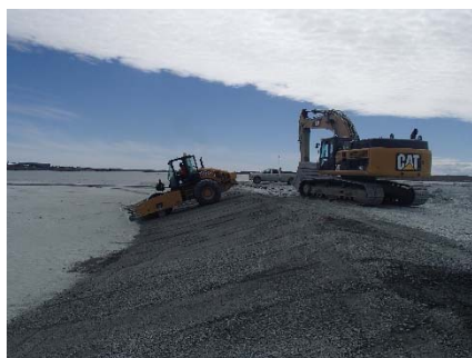
NCIS-070 (2018-07-01), looking S from Sta. 1+160/-89 m. Compaction of the 0.5 m lift of fine filter between El. 150 and 152 m with a 10-tonne smooth-drum compactor with vibration (4 passes) in the upstream slope from Sta. 1+335 m to 1+100 m.
