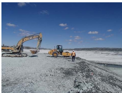
NCIS-065 (2018-06-30), looking NE from Sta. 1+140/-96 m. Compaction of the 0.5 m lift of coarse filter between El. 148 and 150 m with a 10-tonne smooth-drum compactor with vibration (4 passes) in the upstream slope from Sta. 1+270 m to 1+100 m.
