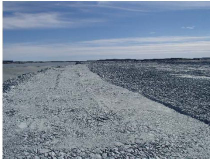
NCIS-050 (2018-06-26), looking S from Sta. 1+230/-55 m. Compaction of the 1.5 to 2 m lift (approx.) of ultramafic (UM) rockfill at El. 150 m with a 10-tonne smooth-drum compactor with vibration (6 passes) between the haul truck traffic lane and the upstream slope from Sta. 1+220 to 1+130 m (o.s. -91 to -44 m).
