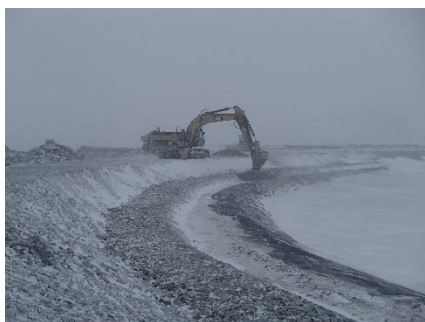
CD-1827 (2018-05-06), looking SW from Sta. 0+940/-16 m. Placement of a 0.5 m thick lift of fine filter from El. 143 m to 143.5 m with an excavator from Sta. 40+730 m to 0+835 m.
