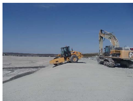
NCIS-126 (2018-07-27), looking W from Sta. 1+140/-98 m (approx.). Compaction of the 0.5 m lift (approx.) of fine filter between El. 150 m and 152 m with a 10-tonne smooth-drum compactor with vibration (4 passes) in the upstream slope from Sta. 1+240 m to 1+100 m.
