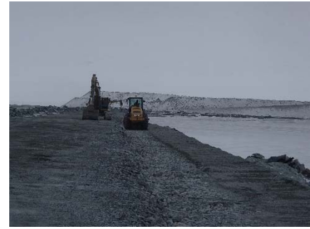
CD-1843 (2018-05-10), looking S from Sta. 0+460/-23 m. Compaction of the third 0.5 m lift (approx.) of fine and coarse filters material at El. 144.5 m with a 10-tonne smooth-drum compactor with vibration (4 passes) from Sta 0+335m to 0+900 m.
