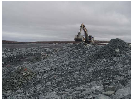
NCIS-047 (2018-06-26), looking N from Sta. 2+580/-35 m. Placement of a 0.5 m thick lift of coarse filter in the upstream slope from El. 150 m to 152 m with an excavator from Sta. 2+560 m to 2+640 m.
