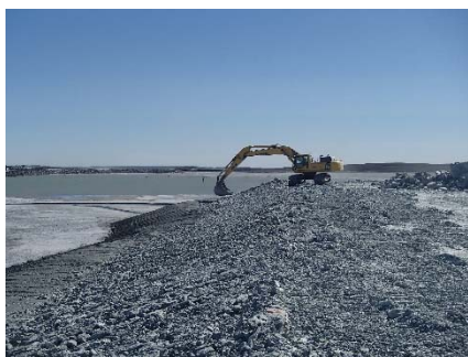
NCIS-092 (2018-07-14), looking S from Sta. 1+160/-77 m (approx.). Profiling of the upstream slope (3H:1V) from El. 150 to 152 m with an excavator from Sta. 1+185 m to 1+135 m.
