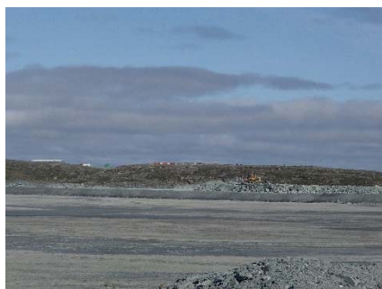
NCIS-106 (2018-07-21), looking NW from Sta. 2+620/-35 m (approx.). Placement of a 2 m thick (approx.) lift of UM rockfill from El. 152 m to El. 154 m (approx.) with a dozer from Sta. 1+947 m to 1+863 m (+14 m to -26 m).
