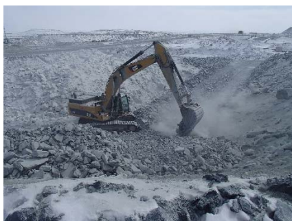
CD-1812 (2018-04-30), looking SE from Sta. 0+985/-11 m. Placement of intermediate volcanic (IV) rockfill on the existing downstream slope up to approx. El. 140 m, from approx. Sta. 0+985 to 40+780 m.
