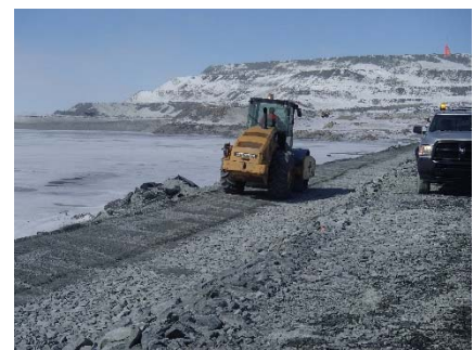
CD-1840 (2018-05-09), looking NW from Sta. 0+575/-15 m. Compaction of the second 0.5 m lift (approx.) of fine and coarse filters material at El. 144 m with a 10-tonne smooth-drum compactor with vibration (4 passes) from Sta 0+500 m to 40+730 m.
