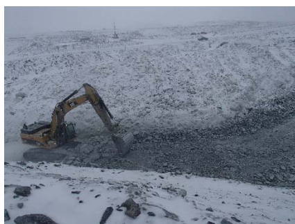
CD-1808 (2018-04-28), looking E from Sta. 40+790/-14 m. Placement a 2 m thick (approx.) lift of intermediate volcanic (IV) rockfill from approx. Sta. 40+780 to 40+805 m (o.s. -6 to 9 m).
