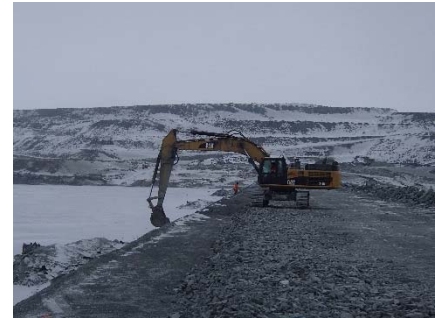
CD-1846 (2018-05-12), looking N from Sta. 0+835/-25 m. Profiling of the upstream slope (2H:1V) from El. 143 to 145 m with an excavator between Sta. 0+330 and 0+600 m and between Sta. 0+715 m and 40+730 m.
