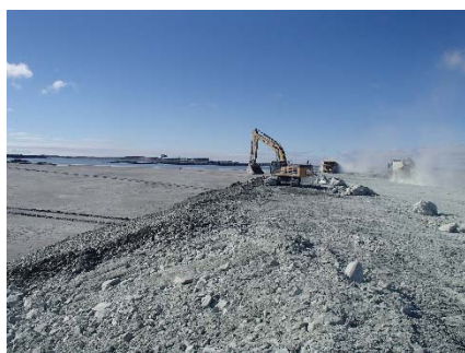
NCIS-058 (2018-06-29), looking S from Sta. 1+340/-34 m. Placement of a 0.5 m thick lift of coarse filter in the upstream slope from El. 148 m to 152 m with an excavator from Sta. 1+340 m to 1+270 m.
