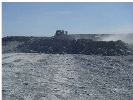
NCIS-098 (2018-07-19), looking E from Sta. 2+040/-9 m (approx.). Placement of a 2 m thick (approx.) lift of UM rockfill from El. 152 m to El. 154 m (approx.) with a dozer from Sta. 2+103 m to 1+984 m (+7 m to -22 m). The material is of good quality and is well graded.
