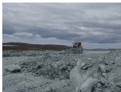
NCIS-069 (2018-07-01), looking NW from Sta. 1+180/-56 m. Placement of a 2 m thick (approx.) lift of UM rockfill from El. 150 m to El. 152 m (approx.) with a dozer from Sta. 1+235 m to 1+160 m (-60 m to -44 m). The material is of good quality and is well graded.
