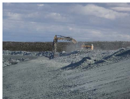
NCIS-108 (2018-07-22), looking N from Sta. 2+490/-32 m (approx.). Profiling of the upstream slope (3H:1V) from El. 152 to 154 m with an excavator from Sta. 2+159 m to 2+409 m.
