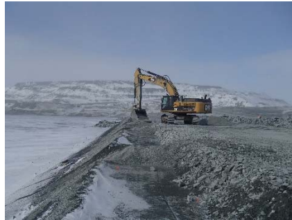
CD-1845 (2018-05-11), looking N from Sta. 0+660/-20 m. Profiling of the upstream slope (2H:1V) from El. 143 to 145 m with an excavator between Sta. 0+175 and 0+330 m and between Sta. 0+600 m and 0+715 m.
