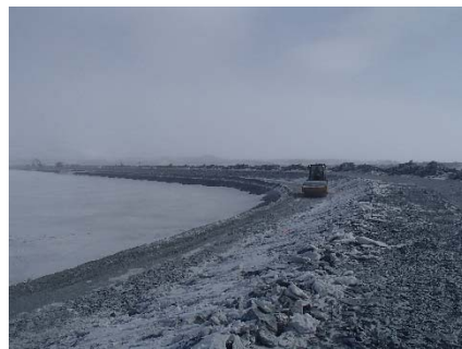
CD-1831 (2018-05-07), looking NE from Sta. 40+730/-24 m. Compaction of the 0.5 m lift (approx.) of fine and coarse filters material at El. 143.5 m with a 10-tonne smooth-drum compactor with vibration (6 passes) from Sta. 40+730 to 0+830 m.
