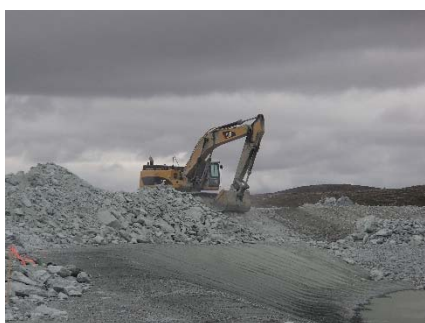
NCIS-134 (2018-07-30), looking NE from Sta. 1+630/-32 m (approx.). Completion of the profiling of the upstream slope (3H:1V) from El. 152 to 154 m with an excavator from Sta. 1+700 m to 1+660 m.
