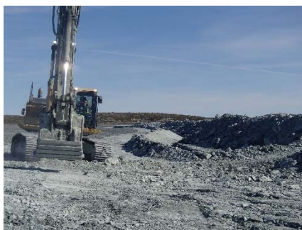
NCIS-119 (2018-07-26), looking N from Sta. 1+430/-22 m (approx.). Excavation of a 0.8 m (approx.) deep, 1 m wide shallow ditch in the rockfill capping with an excavator from Sta. 1+455 m to 1+400 m.
