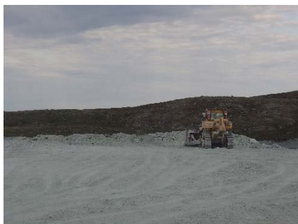
NCIS-122 (2018-07-27), looking W from Sta. 1+960/-6 m (approx.). Placement of a 2 m thick (approx.) lift of UM rockfill from El. 152 m to El. 154 m (approx.) with a dozer from Sta. 1+830 m to 1+860 m (+8 m to -23 m).
