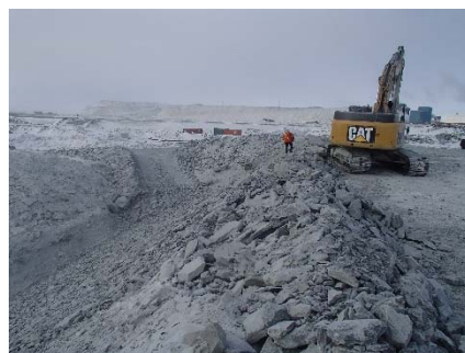
CD-1813 (2018-05-01), looking S from Sta. 0+980/-2 m. Placement of intermediate volcanic (IV) rockfill on the existing downstream slope up to approx. El. 143 m, from approx. Sta. 0+980 to 40+780 m.
