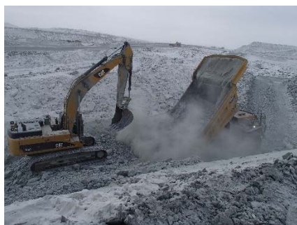
CD-1811 (2018-04-30), looking SE from Sta. 0+985/-11 m. Placement the second, third, fourth and fifth 1 m thick (approx.) lifts of intermediate volcanic (IV) rockfill from approx. Sta. 0+985 to 40+780 m (o.s. -8 to 8 m) with the excavator.
