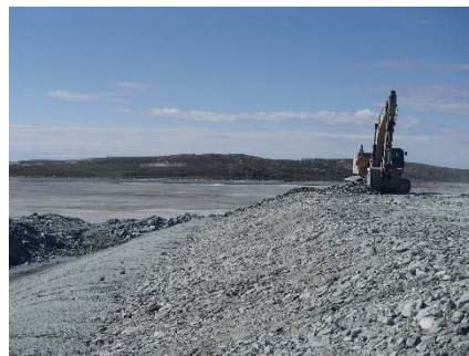
NCIS-102 (2018-07-20), looking W from Sta. 2+680/-21 m (approx.). Placement of a 0.5 m thick lift of coarse filter in the upstream slope from El. 152 m to 154 m with an excavator from Sta. 2+575 m to 2+710 m and from Sta. 2+411 m to 2+460 m.
