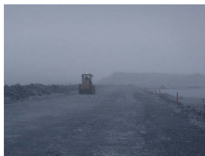
CD-1810 (2018-04-30), looking S from Sta. 0+335/-15 m. Compaction of the 2 m lift (approx.) of IV rockfill at El. 145 m with a 10-tonne smooth-drum compactor with vibration (6 passes) from Sta. 0+350 to 0+540 m (o.s. -19 to -7 m).
