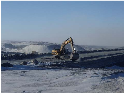
CD-1844 (2018-05-11), looking SE from Sta. 0+080/-49 m. Placement of a fourth 0.5 m thick lift of coarse filter from El. 144.5 m to 145 m with an excavator from Sta. 0+170 m to 40+730 m.
