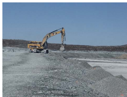
NCIS-066 (2018-06-30), looking N from Sta. 1+400/-34 m. Placement of a 0.5 m thick lift of fine filter over the coarse filter in the upstream slope from El. 150 m to 152 m with an excavator from Sta. 1+595 m to 1+550 m.
