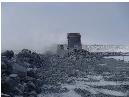
CD-1820 (2018-05-04), looking S from Sta. 0+790/-7 m. Placement of a 2 m thick (approx.) lift of intermediate volcanic (IV) rockfill from El. 143 m to El. 145 m from approx. Sta. 0+880 m to 0+830 m (o.s. -28 to -11 m).
