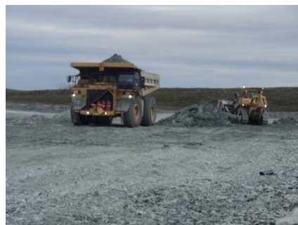
NCIS-096 (2018-07-18), looking N from Sta. 2+355/+9 m (approx.). Placement of a 2 m thick (approx.) lift of UM rockfill from El. 152 m to El. 154 m (approx.) with a dozer from Sta. 2+190 m to 2+103 m (+7 m to -22 m).
