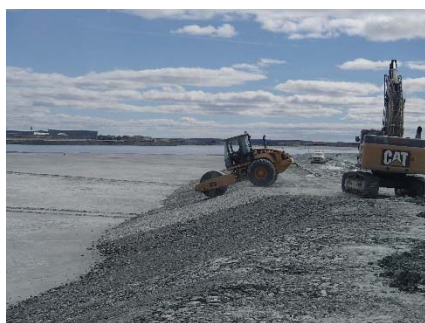
NCIS-061 (2018-06-29), looking S from Sta. 1+365/-35 m. Compaction of the 0.5 m lift of coarse filter between El. 148 and 152 m with a 10-tonne smooth-drum compactor with vibration (4 passes) in the upstream slope from Sta. 1+340 m to 1+270 m.
