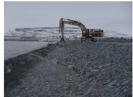
CD-1837 (2018-05-08), looking N from Sta. 0+940/-25 m. Placement of a second 0.5 m thick lift of coarse filter from El. 143.5 m to 144 m with an excavator from Sta. 0+290 m to 0+500 and from Sta. 0+835 m to 0+930 m.
