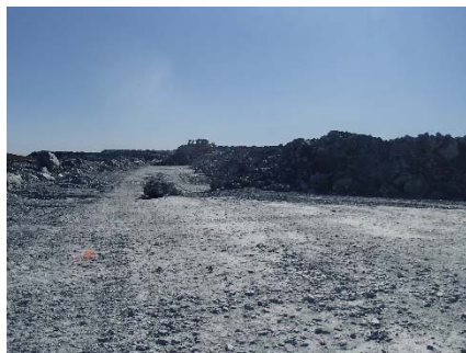
NCIS-100 (2018-07-20), looking E from Sta. 1+960/+10 m (approx.). Placement of a 2 m thick (approx.) lift of UM rockfill from El. 152 m to El. 154 m (approx.) with a dozer from Sta. 1+984 m to 1+947 m (+14 m to -26 m). The material is of good quality and is well graded.
