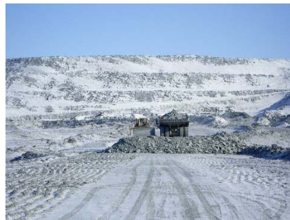
CD-1798 (2018-04-24), looking N from Sta. 0+500/-15 m. Placement a 2 m thick (approx.) lift of intermediate volcanic rockfill from El. 143 m to El. 145 m from 0+340 to 0+435 m (o.s. -28 to -18 m).
