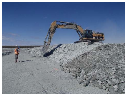
NCIS-103 (2018-07-20), looking NE from Sta. 2+420/-27 m (approx.). Profiling of the upstream slope (3H:1V) from El. 152 to 154 m with an excavator from Sta. 2+400 m to 2+410 m. Oversize boulders were removed.
