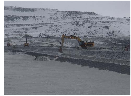
CD-1834 (2018-05-08), looking NE from Sta. 40+760/-23 m. Placement of a first 0.5 m thick lift of coarse filter from El. 143 m to 143.5 m on length of approx. 5 m with an excavator at the location of the deposition finger at Sta 0+520 m and 0+660 m.
