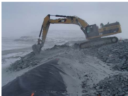
CD-1830 (2018-05-07), looking N from Sta. 0+420/-26 m. Removal of the deposition finger materials with an excavator at Sta. 0+390 m.
