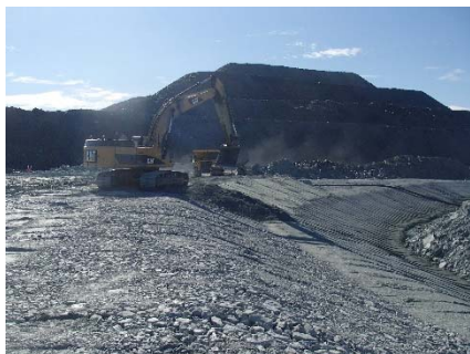
NCIS-104 (2018-07-21), looking SE from Sta. 2+650/-23 m (approx.). Placement of a 0.5 m thick lift of fine filter in the upstream slope from El. 152 m to 154 m with an excavator from Sta. 2+710 m to 2+445 m.
