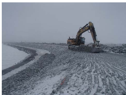
CD-1826 (2018-05-06), looking NE from Sta. 40+770/-27 m. Placement of a 0.5 m thick lift of coarse filter from El. 143 m to 143.5 m with an excavator from Sta. 40+730 m to 0+775 m.
