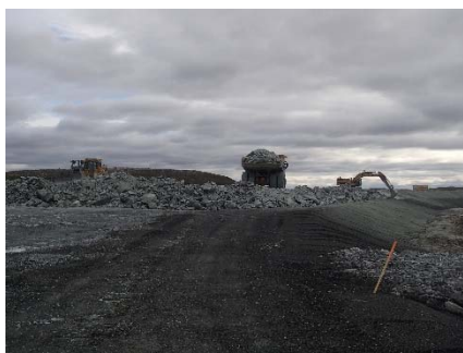
NCIS-128 (2018-07-28), looking NE from Sta. 1+680/-42 m (approx.). Placement of a 2 m thick (approx.) lift of UM rockfill from El. 152 m to El. 154 m (approx.) with a dozer from Sta. 1+830 m to 1+660 m (+8 m to -31 m) and profiling of the upstream slope (3H:1V) from El. 152 to 154 m with an excavator from Sta. 1+880 m to 1+780 m.
