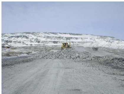
CD-1797 (2018-04-23), looking N from Sta. 0+380/-20 m. Placement a 2 m thick (approx.) lift of intermediate volcanic rockfill from El. 143 m to El. 145 m from 0+250 to 0+400 m (o.s. -28 to -18 m).
