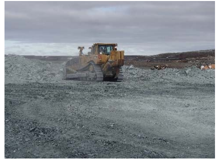
NCIS-048 (2018-06-26), looking SW from Sta. 1+120/-92 m. Placement of a 1.5 to 2 m thick (approx.) lift of UM rockfill from El. 148 m to El. 150 m (approx.) with a dozer from Sta. 1+125 m to 1+115 m (-92 m to -47 m).
