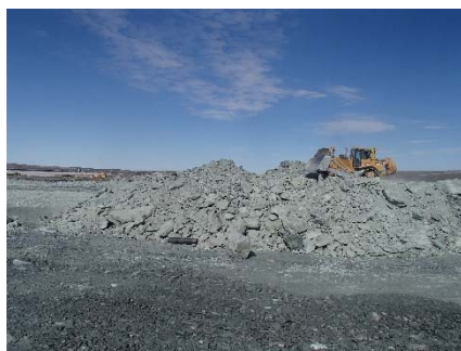
NCIS-064 (2018-06-30), looking W from Sta. 1+200/-65 m. Placement of a 2 m thick (approx.) lift of UM rockfill from El. 150 m to El. 152 m (approx.) with a dozer from Sta. 1+320 m to 1+235 m (-65 m to -45 m). The material is of good quality and is well graded.
