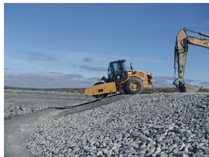
NCIS-105 (2018-07-21), looking NW from Sta. 2+630/-34 m (approx.). Compaction of the 0.5 m lift (approx.) of coarse filter between El. 152 m and 154 m with a 10-tonne smooth-drum compactor with vibration (4 passes) in the upstream slope from Sta. 2+710 m to 2+411 m.
