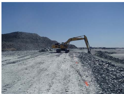
NCIS-095 (2018-07-16), looking S from Sta. 2+375/-18 m (approx.). Profiling of the upstream slope (3H:1V) from El. 152 to 154 m with an excavator from Sta. 2+545 m to 2+410 m.
