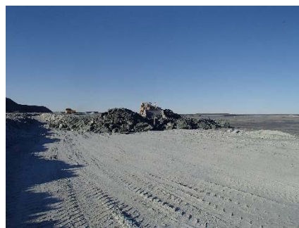
NCIS-093 (2018-07-15), looking S from Sta. 2+260/+12 m (approx.). Placement of a 2 m thick (approx.) lift of UM rockfill from El. 152 m to El. 154 m (approx.) with a dozer from Sta. 2+290 m to 2+280 m (+9 m to -22 m).
