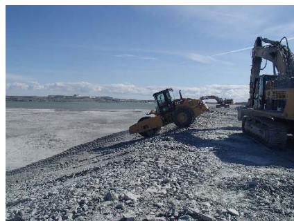
NCIS-099 (2018-07-19), looking SE from Sta. 1+180/-76 m (approx.). Compaction of the 0.5 m lift (approx.) of coarse filter between El. 150 m and 152 m with a 10-tonne smooth-drum compactor with vibration (4 passes) in the upstream slope from Sta. 1+200 m to 1+170 m.
