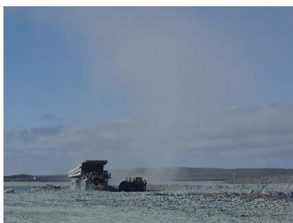
NCIS-059 (2018-06-29), looking S from Sta. 1+330/-34 m. Placement of a 1.5 to 2 m thick (approx.) lift of UM rockfill from El. 148 m to El. 150 m (approx.) with a dozer from Sta. 1+120 m to 1+100 m (-96 m to -60 m). The material is of good quality and is well graded.
