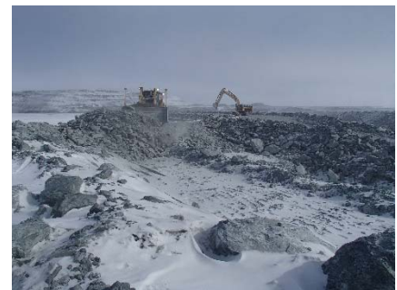
CD-1822 (2018-05-04), looking N from Sta. 40+725/+7 m. Placement of two 2 m thick lifts of IV rockfill from El. 141 m to El. 145 m from approx. Sta. 40+720 m to 40+750 m (o.s. -10 to +10 m) and profiling of the upstream slope (2H:1V) from El. 143 to 145 m with an excavator between Sta. 0+830 m and 0+980 m.
