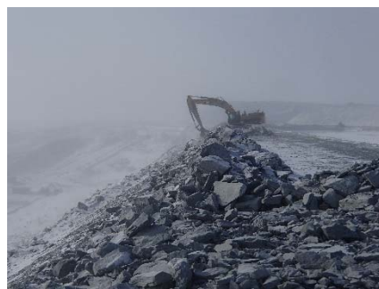
CD-1825 (2018-05-05), looking S from Sta. 0+430/+9 m. Profiling of the downstream slope (1.5H:1V) from El. 143 to 145 m with an excavator between Sta. 0+330 m and 0+440 m and between Sta. 0+530 m and 0+745 m.
