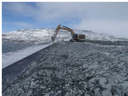
CD-1829 (2018-05-06), looking N from Sta. 0+340/-24 m. Placement of a 0.5 m thick lift of coarse filter from El. 143 m to 143.5 m with an excavator from Sta. 0+170 m to 0+460 m and placement of a 0.5 m thick lift of fine filter from Sta. 0+170 m to 0+380 m.
