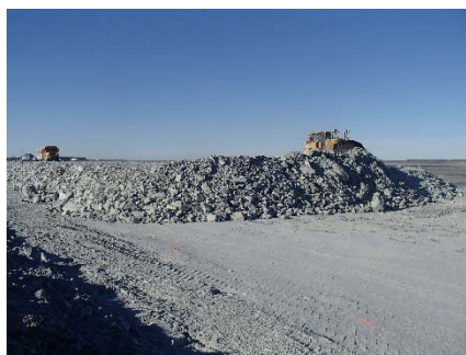
NCIS-091 (2018-07-14), looking S from Sta. 2+330/+13 m (approx.). Placement of a 2 m thick (approx.) lift of UM rockfill from El. 152 m to El. 154 m (approx.) with a dozer from Sta. 2+370 m to 2+290 m (+9 m to -22 m).
