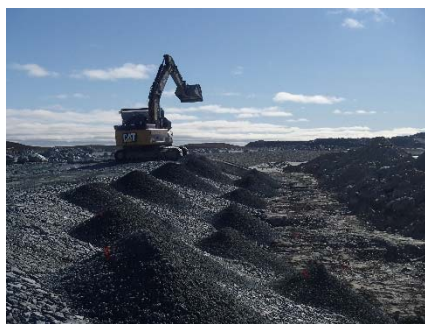
NCIS-055 (2018-06-28), looking NE from Sta. 1+730/-42 m. Placement of a 0.5 m thick lift of fine filter over the coarse filter in the upstream slope from El. 150 m to 152 m with an excavator from Sta. 1+820 m to 1+595 m.
