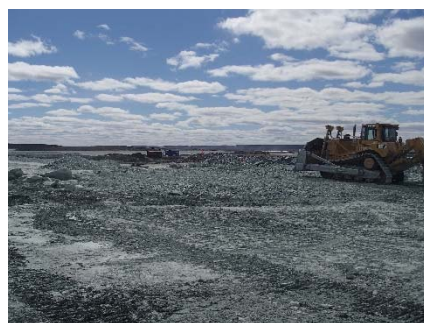
NCIS-060 (2018-06-29), looking SW from Sta. 1+365/-35 m. Placement of a 2 m thick (approx.) lift of UM rockfill from El. 150 m to El. 152 m (approx.) with a dozer from Sta. 1+340 m to 1+320 m (-19 m to +16 m). The material is of good quality and is well graded.
