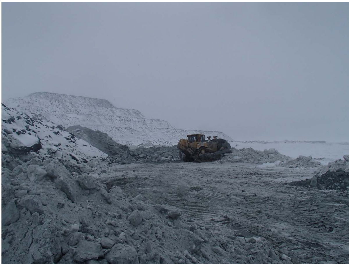
Photograph NCIS-005: Removal of the excavated material, pushed with a dozer towards the center of the North Cell to clear the upstream toe.
