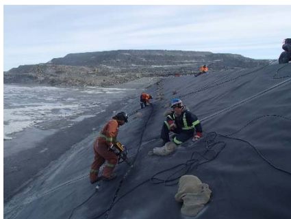
CD-1890 (2018-06-05), looking N from Sta. 0+310/-26 m. View of the extrusion welding.
