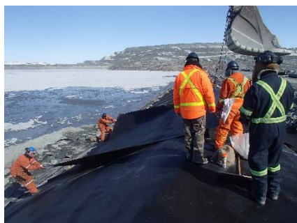
CD-1883 (2018-06-02), looking N from Sta. 0+525/-26 m. Installation of the LLDPE liner on the upstream slope 2H:1V between El. 143 m and 145 m from Sta. 0+610 m to 0+480 m (panel numbers 868 to 886).
