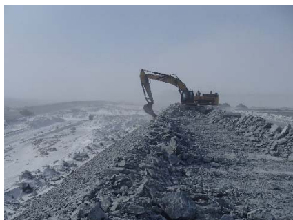
CD-1853 (2018-05-14), looking S from Sta. 0+850/+3 m. Profiling of the downstream slope (1.5H:1V) from El. 143 to 145 m with an excavator between Sta. 0+835 m and 0+940.
