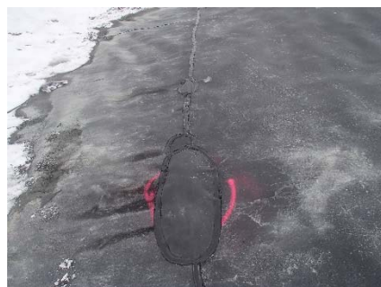
CD-1876 (2018-05-30), looking N from Sta. 0+820/-26 m. View of repair patches on the extrusion weld at the bottom of the panel 838.
