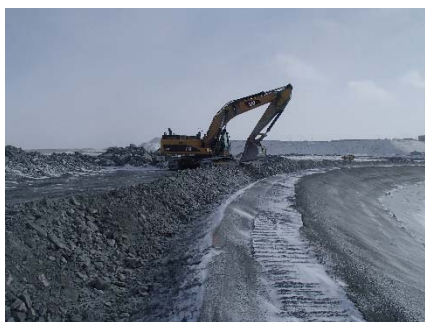
CD-1851 (2018-05-13), looking S from Sta. 0+910/-18 m. Excavation of the LLDPE geomembrane crest anchoring trench from Sta. 40+730 m to 0+830 m.
