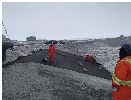
CD-1859 (2018-05-22), looking SW from Sta. 40+780/-38 m. Installation of the geotextile on the upstream slope 3H:1V (SD5 side) to 2H:1V (Central Dike side) between El. 143 m and 145 m from Sta. 40+640 m to 0+830 m.
