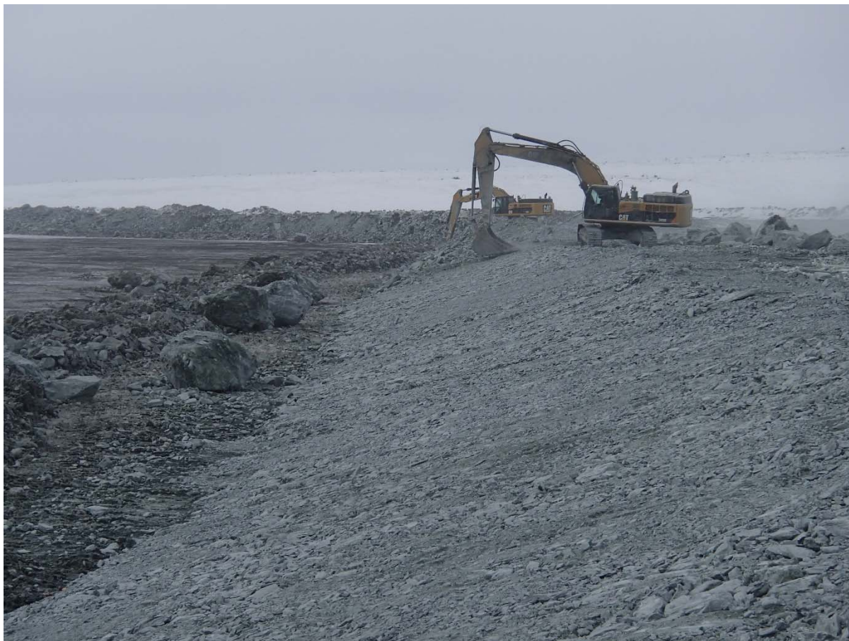
Photograph NCIS-007: Profiling of the upstream slope (3H:1V) from El. 150 to 152 m with an excavator.
