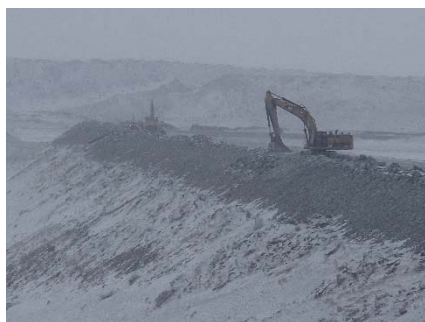
CD-1850 (2018-05-13), looking SW from Sta. 0+160/+20 m. Profiling of the downstream slope (1.5H:1V) from El. 143 to 145 m with an excavator between Sta. 0+440 m and 0+530 m and between Sta. 0+745 m and 0+835 m.
