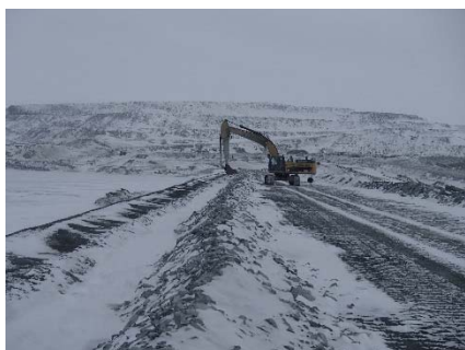
CD-1857 (2018-05-21), looking N from Sta. 0+700/-20 m. Snow removal in the anchoring trench with an excavator between Sta. 0+170 m and 40+780 m.
