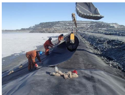
CD-1886 (2018-06-03), looking N from Sta. 0+485/-26 m. Installation of the LLDPE liner on the upstream slope 2H:1V between El. 143 m and 145 m from Sta. 0+480 m to 0+320 m (panel numbers 887 to 910).
