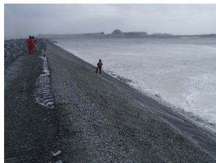
CD-1855 (2018-05-16), looking S from Sta. 0+230/-22 m. Clean-up of the existing LLDPE with pressurized air stream in preparation for liner installation between Sta. 0+170 m and 40+780 m3.
