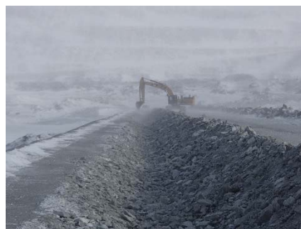
CD-1852 (2018-05-14), looking N from Sta. 0+500/-25 m. Excavation of the LLDPE geomembrane crest anchoring trench from Sta. 0+830 m to 0+170 m.
