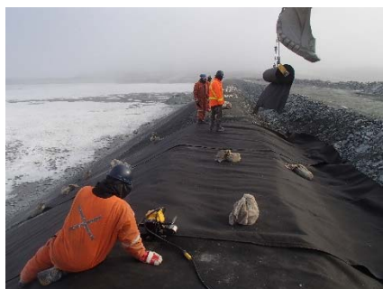
CD-1880 (2018-06-02), looking N from Sta. 0+600/-25 m. Installation of the geotextile on the upstream slope 2H:1V between El. 143 m and 145 m from Sta. 0+610 m to 0+480 m.
