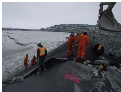
CD-1877 (2018-06-01), looking N from Sta. 0+745/-22 m. Installation of the geotextile on the upstream slope 2H:1V between El. 143 m and 145 m from Sta. 0+740 m to 0+610 m.
