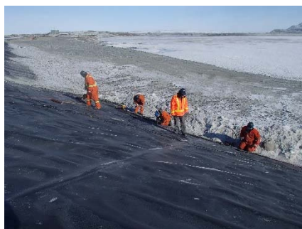
CD-1865 (2018-05-25), looking NW from Sta. 40+740/-35 m. Repairs on the extrusion fillet seam at the bottom of the LLDPE liner panels between Sta. 40+680 m and 0+950 m, on panels 802 to 807, and 811 to 813.
