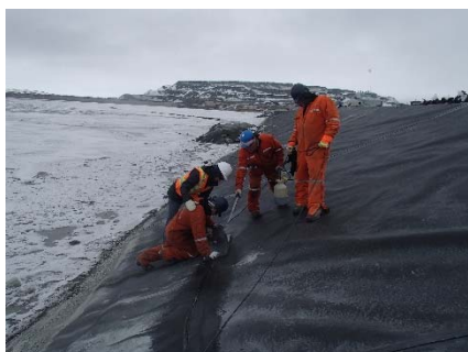
CD-1875 (2018-05-30), looking N from Sta. 0+835/-26 m. View of a vacuum box testing.
