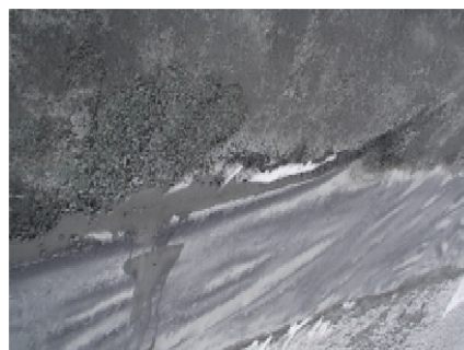
CD-1858 (2018-05-21), looking S from Sta. 0+970/-45 m. View of the bottom of the fine filter upstream slope. Some material is missing to achieve a smooth slope.
