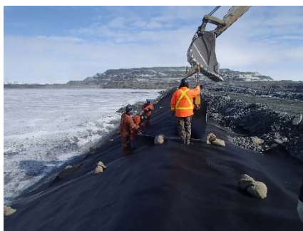
CD-1878 (2018-06-01), looking N from Sta. 0+720/-22 m. Installation of the LLDPE liner on the upstream slope 2H:1V between El. 143 m and 145 m from Sta. 0+740 m to 0+610 m (panel numbers 849 to 867).
