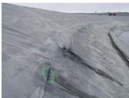
CD-1893 (2018-06-06), looking SW from Sta. 0+950/-27 m. View of repair patches on the extrusion weld at the bottom of the panels 803, 807, 808, 810, 814, 815, 816 and 818.
