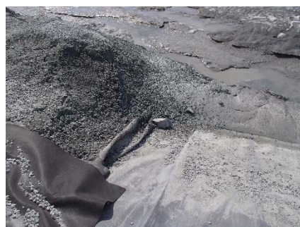
CD-1894 (2018-06-10), looking W from Sta. 0+800/-28 m. View of a block in direct contact with the LLDPE liner following the construction of the deposition fingers on Central Dike.
