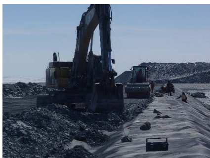
CD-1884 (2018-06-02), looking S from Sta. 0+530/-25 m. Backfilling of the geosynthetic tie-in from Sta. 0+610 m to 0+480 m and compaction of the tie-in material with a 10-tonne smooth-drum compactor with vibration (4 passes) from Sta. 0+610 to 0+480 m.
