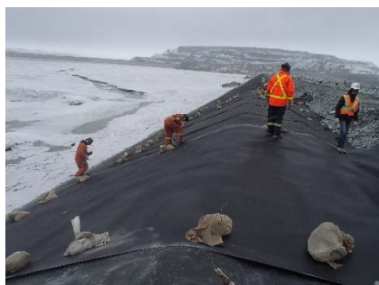
CD-1874 (2018-05-29), looking N from Sta. 0+760/-26 m. Installation of the LLDPE liner on the upstream slope 2H:1V between El. 143 m and 145 m from Sta. 0+760 m to 0+740 m (panel numbers 845 to 848).
