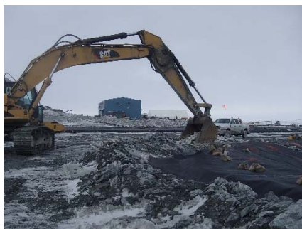
CD-1863 (2018-05-24), looking SW from Sta. 40+750/-18 m. Backfilling of the geosynthetic tie-in from Sta. 40+680 m to 0+950 m.
