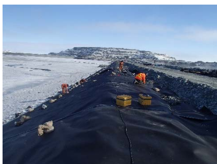
CD-1872 (2018-05-28), looking N from Sta. 0+900/-24 m. Installation of the LLDPE liner on the upstream slope 2H:1V between El. 143 m and 145 m from Sta. 0+900 m to 0+760 m (panel numbers 824 to 844).
