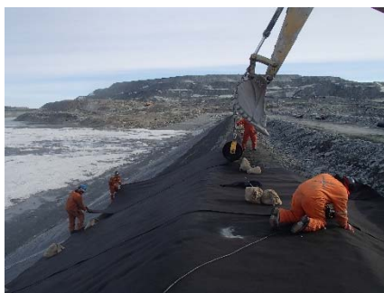
CD-1887 (2018-06-04), looking N from Sta. 0+310/-26 m. Installation of the geotextile on the upstream slope 2H:1V between El. 143 m and 145 m from Sta. 0+320m to 0+160 m.
