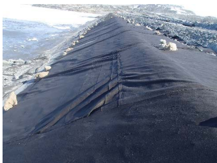
CD-1881 (2018-06-02), looking N from Sta. 0+530/-27 m. View of a geotextile panel with a horizontal weld in the slope at Sta. 0+520 m before its removal.
