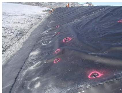
CD-1879 (2018-06-01), looking N from Sta. 0+735/-28 m. View of the repaired holes on panel 850.
