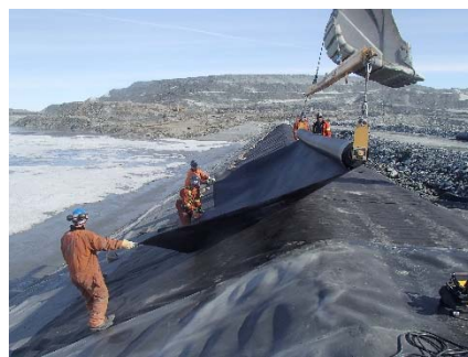
CD-1888 (2018-06-04), looking N from Sta. 0+325/-26 m. Installation of the LLDPE liner on the upstream slope 2H:1V between El. 143 m and 145 m from Sta. 0+320 m to 0+160 m (panel numbers 911 to 910).
