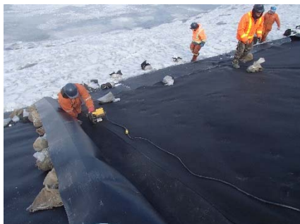
CD-1869 (2018-05-27), looking W from Sta. 0+915/-30 m. Installation of the geotextile on the upstream slope 2H:1V between El. 143 m and 145 m from Sta. 0+935 m to 0+900 m.
