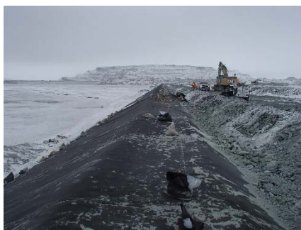
CD-1860 (2018-05-23), looking N from Sta. 0+790/-26 m. Installation of the geotextile on the upstream slope 2H:1V between El. 143 m and 145 m from Sta. 0+830 m to 0+750 m.
