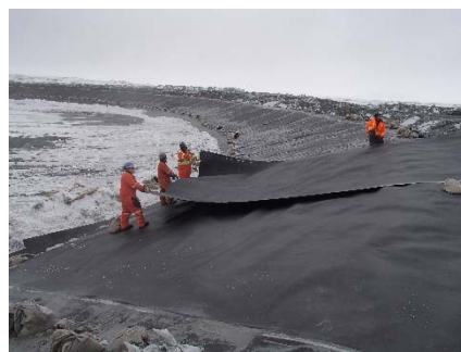
CD-1861 (2018-05-24), looking NE from Sta. 40+680/-8 m. Installation of the LLDPE liner on the upstream slope 3H:1V (SD5 side) to 2H:1V (Central Dike side) between El. 143 m and 145 m from Sta. 40+680 m to 0+950 m (panel numbers 802 to 817).
