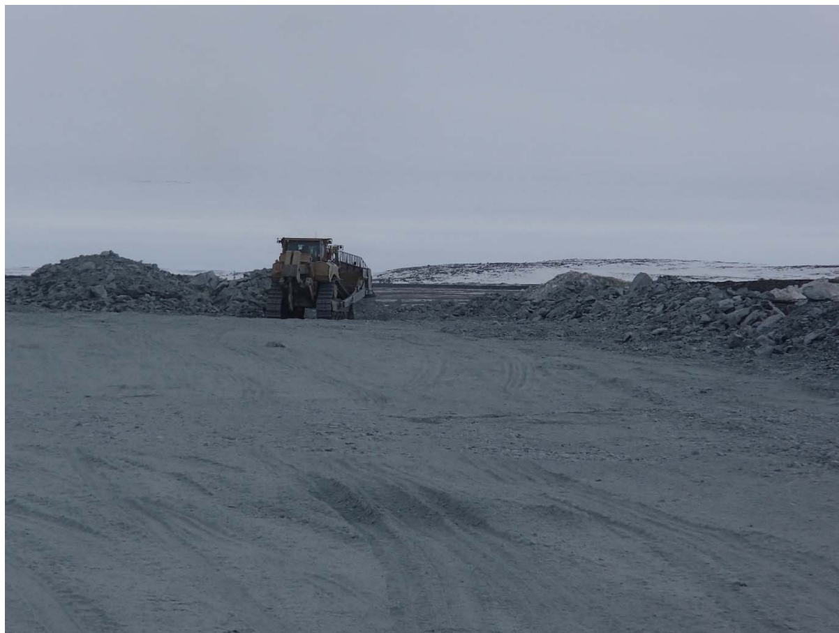
Photograph NCIS-021: From Sta. 1+550 m (approx.), looking S. Placement a 2 m thick (approx.) lift of UM rockfill from El. 150 m to El. 152 m (approx.) with a dozer from Sta. 1+535 m to 1+500 m (offset unavailable).
