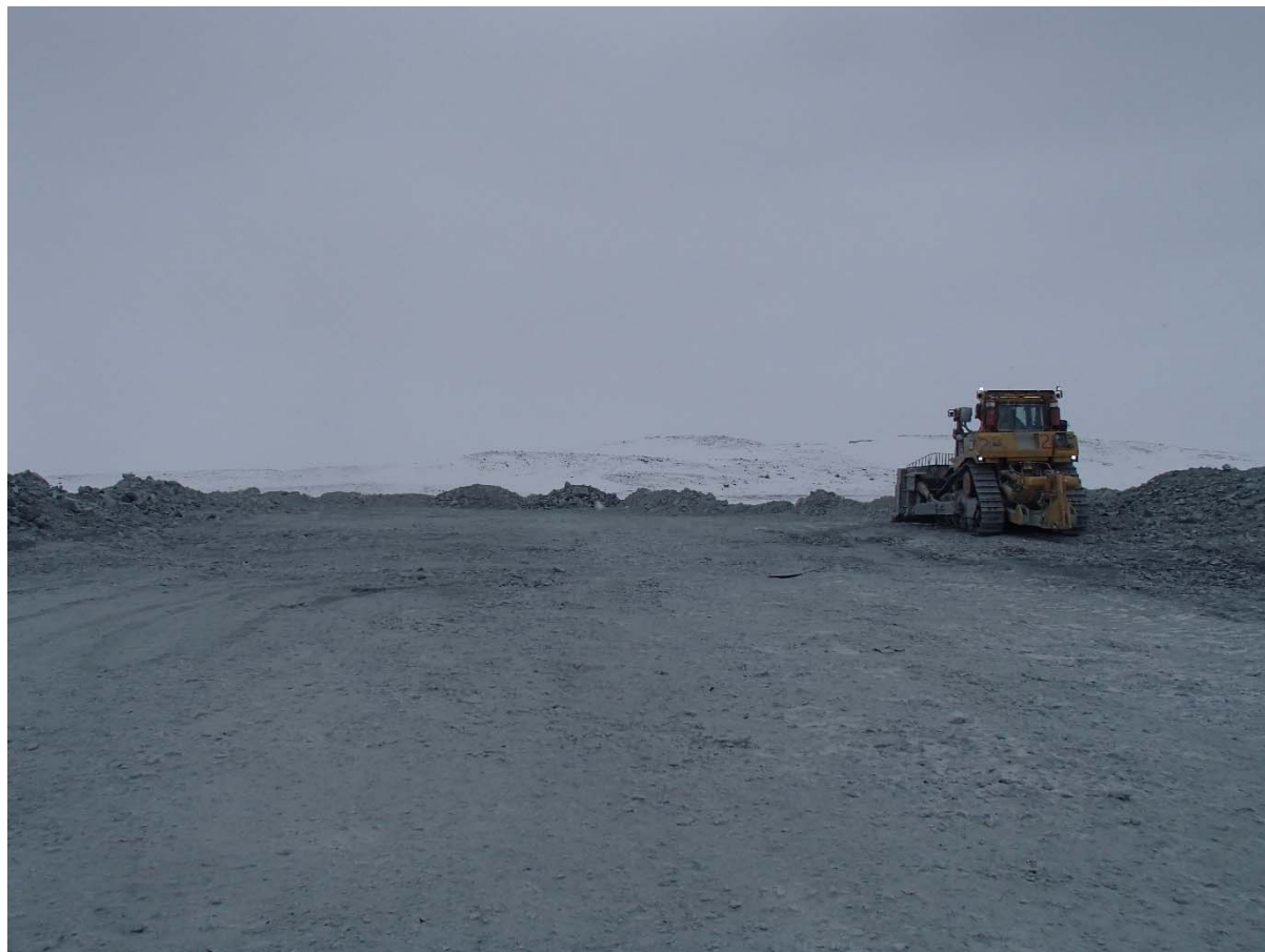
Photograph NCIS-009: Placement of a 2 m thick (approx.) lift of UM rockfill from El. 150 m to El. 152 m (approx.) with a dozer from Sta. 1+880 m to 1+825 m (offset unavailable).
