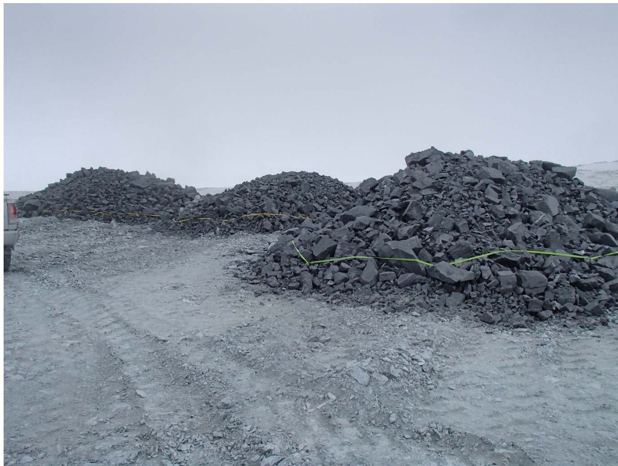
Photograph NCIS-016: From Sta. 1+750 m (approx.), looking SE. View of the Iron Formation rockfill (PAG material) piles on the North Cell Internal Structure to be cleaned from the structure embankment.
