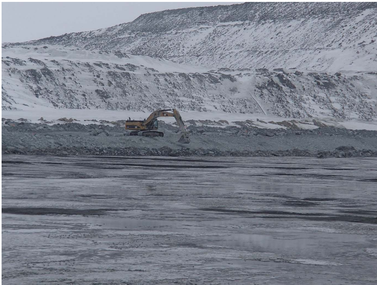
Photograph NCIS-010: Profiling of the upstream slope (3H:1V) from El. 150 to 152 m with an excavator from Sta. 2+777 m to 2+400 m (approx.).
