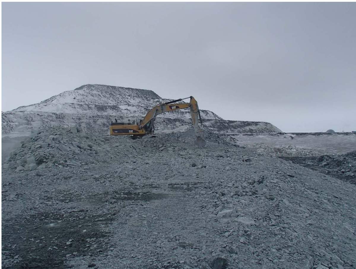
Photograph NCIS-013: From Sta. 2+600 m (approx.), looking NE. Correction of the crest elevation with an excavator to achieve a closer elevation to 152 m around Sta. 2+650 m.
