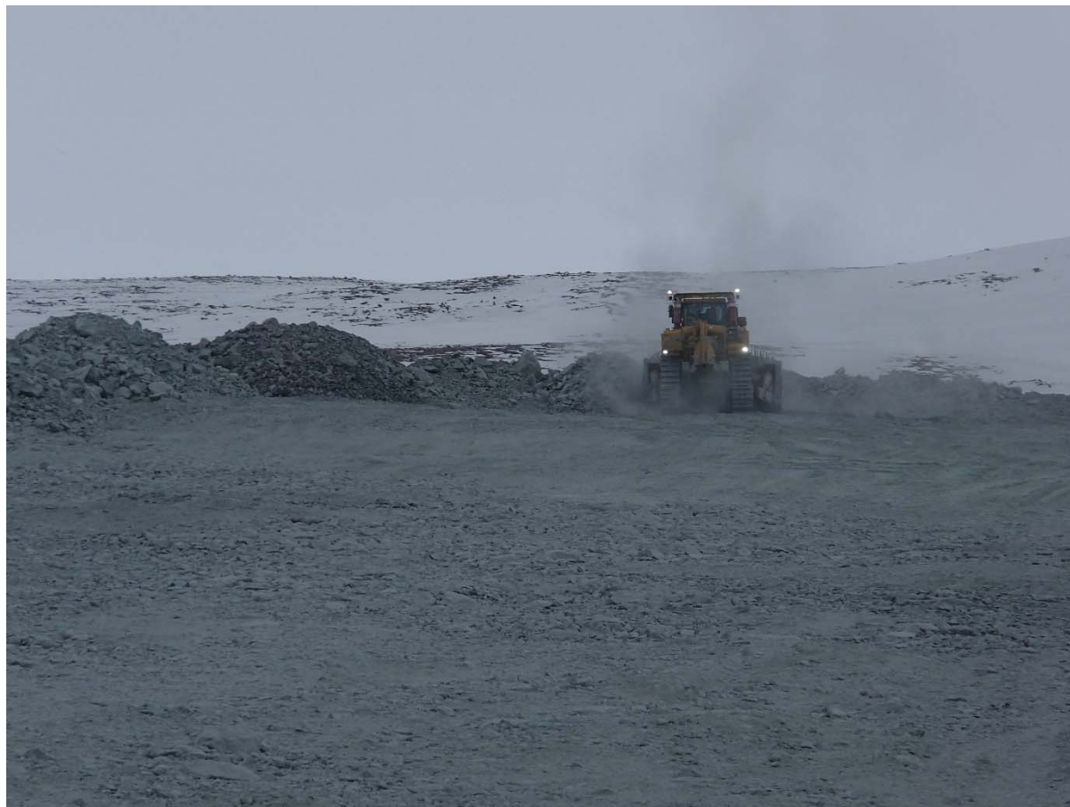
Photograph NCIS-011: From Sta. 2+000 m (approx.), looking SW. Placement a 2 m thick (approx.) lift of UM rockfill from El. 150 m to El. 152 m (approx.) with a dozer from Sta. 1+880 m to 1+767 m (offset unavailable).
