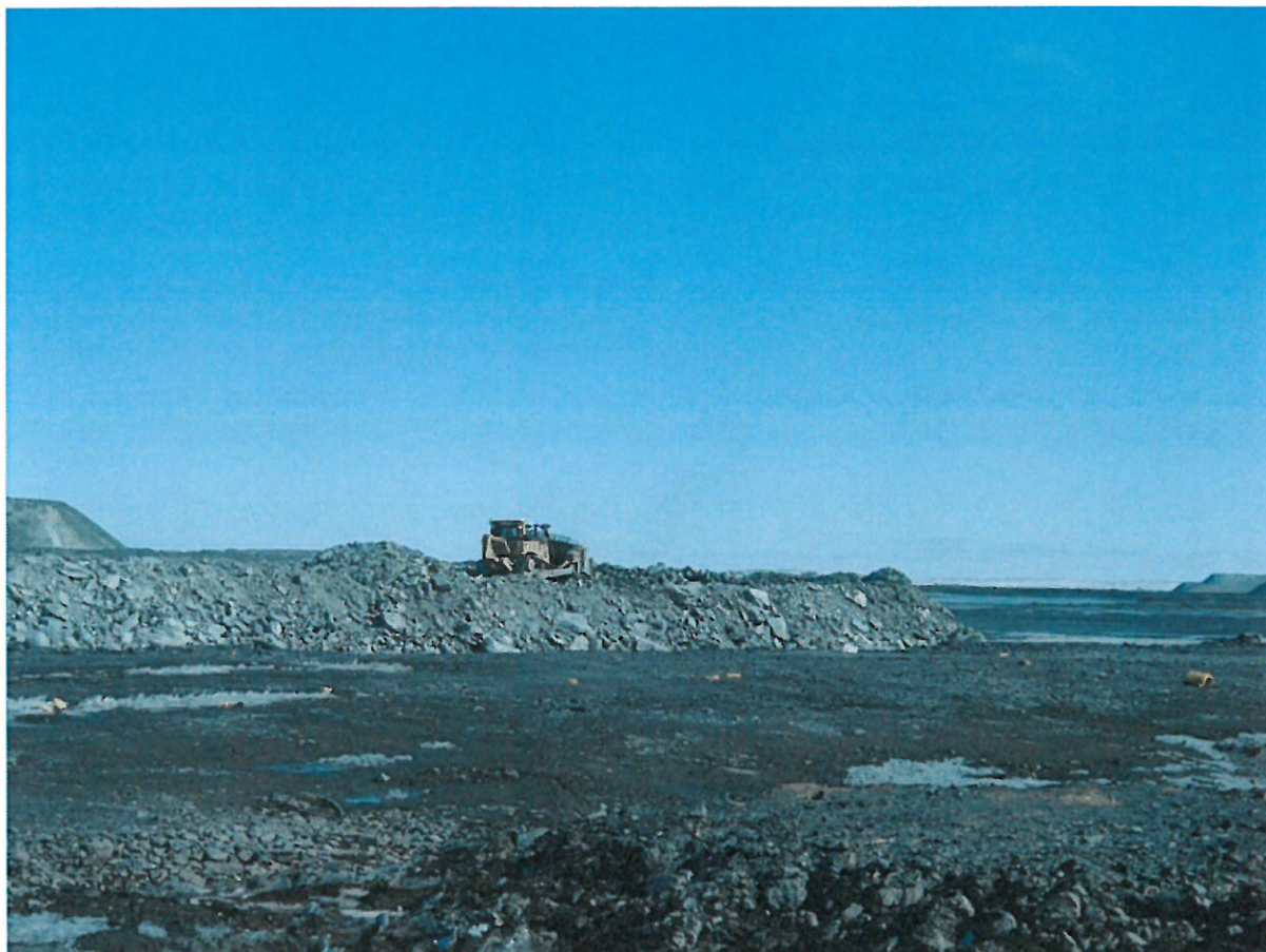
Photograph NCIS-025: From Sta. 1+475 m (approx.), looking SE. Placement of a 2 m thick (approx.) lift of UM rockfill from El. 150 m to El. 152 m (approx.) with a dozer from Sta. 1+450 m to 1+390 m (offset unavailable). The material is of good quality and is well graded.
