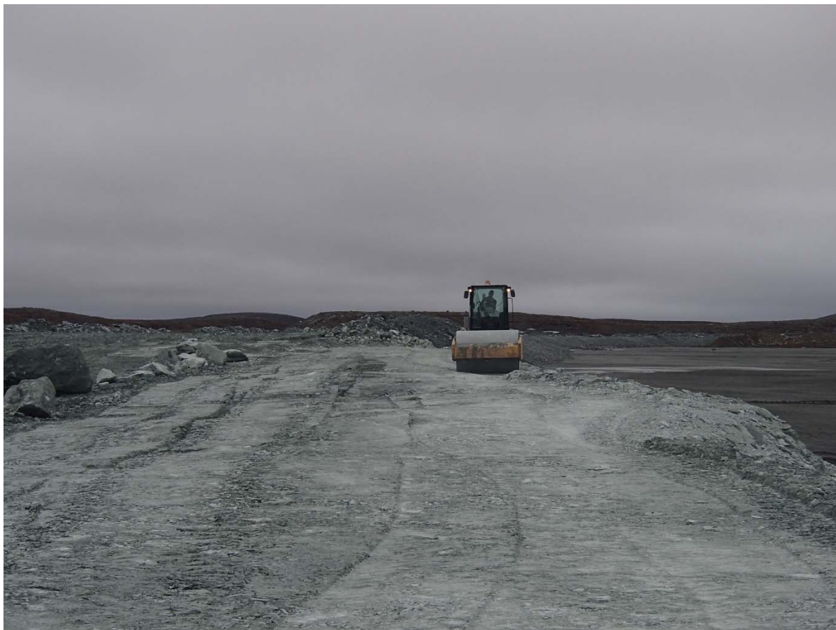
Photograph NCIS-043: From Sta. 1+250/-38 m (approx.), looking N. Compaction of the 1.5 to 2 m lift (approx.) of ultramafic (UM) rockfill at El. 150 m with a 10-tonne smooth-drum compactor with vibration (6 passes) between the haul truck traffic lane and the upstream slope from Sta. 1+330 to 1+200 m (offset -53 to -24 m).
