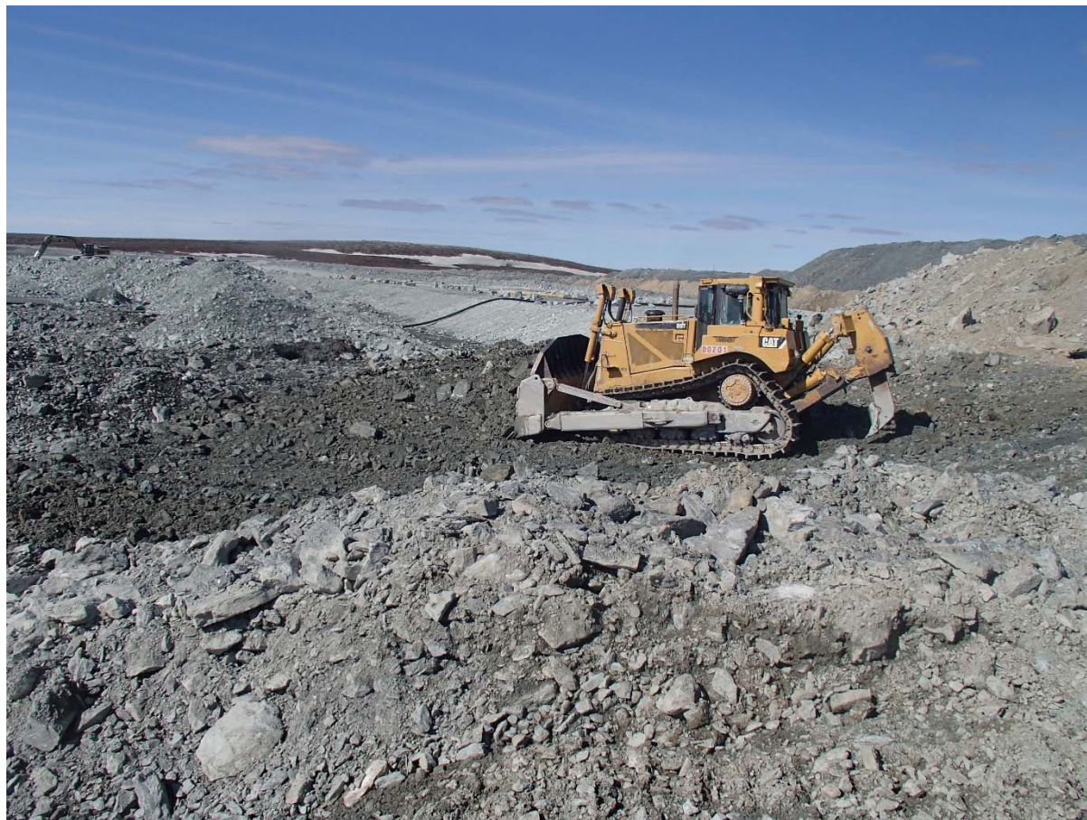
Photograph NCIS-049: From Sta. 2+870/-28 m (approx.), looking N. Removing of UM rockfill material from the capping with a dozer to level the surface to El. 150 m from Sta. 2+760 m to 2+850 m (offset -29 to -17 m).
