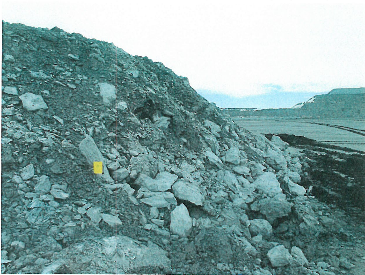
Photograph NCIS-028: From Sta. 1+340/+3 m, looking E. View of the LM rockfill lift approximately 3.2 m thick.
