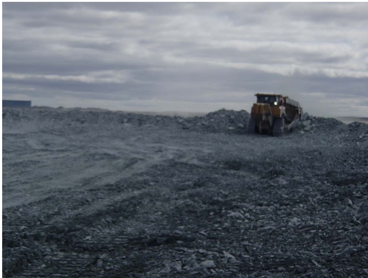
Photograph NCIS-044: From Sta. 1+200/-19 m (approx.), looking S. Placement of a 1.5 to 2 m thick (approx.) lift of UM rockfill from El. 148 m to El. 150 m (approx.) with a dozer from Sta. 1+150 m to 1+120 m (-92 m to +10 m). The material is of good quality and is well graded.
