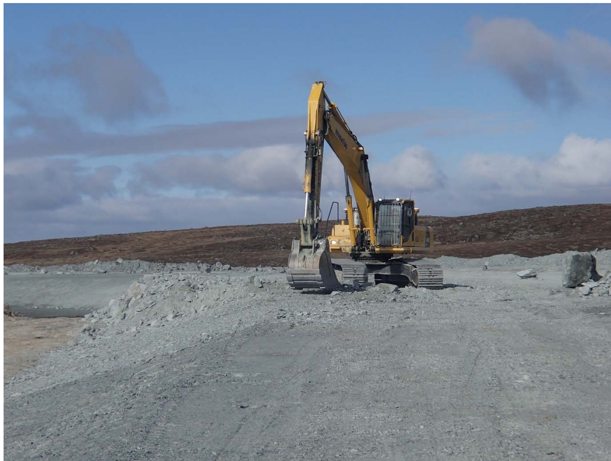
Photograph NCIS-034: From Sta. 1+900/-21 m (approx.), looking W. Profiling of the upstream slope (3H:1V) from El. 150 to 152 m with an excavator from Sta. 1+860 m to 1+750 m.
