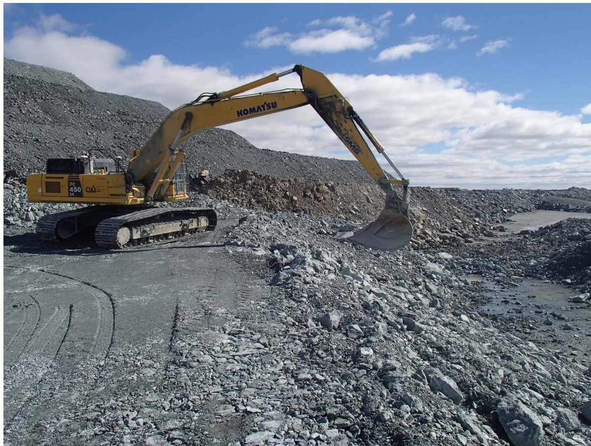
Photograph NCIS-045: From Sta. 2+760/-40 m (approx.), looking S. Profiling of the upstream slope (3H:1V) from El. 150 to 152 m with an excavator from Sta. 2+715 m to 2+825 m.
