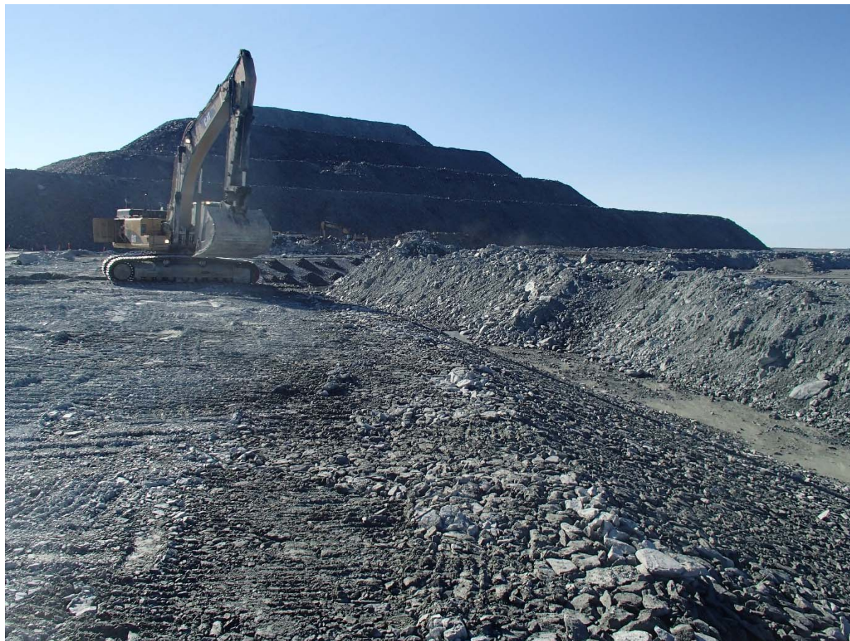
Photograph NCIS-051: From Sta. 2+630/-34 m (approx.), looking SE. Placement of a 0.5 m thick lift of coarse filter in the upstream slope from El. 150 m to 152 m with an excavator from Sta. 2+640 m to 2+815 m.
