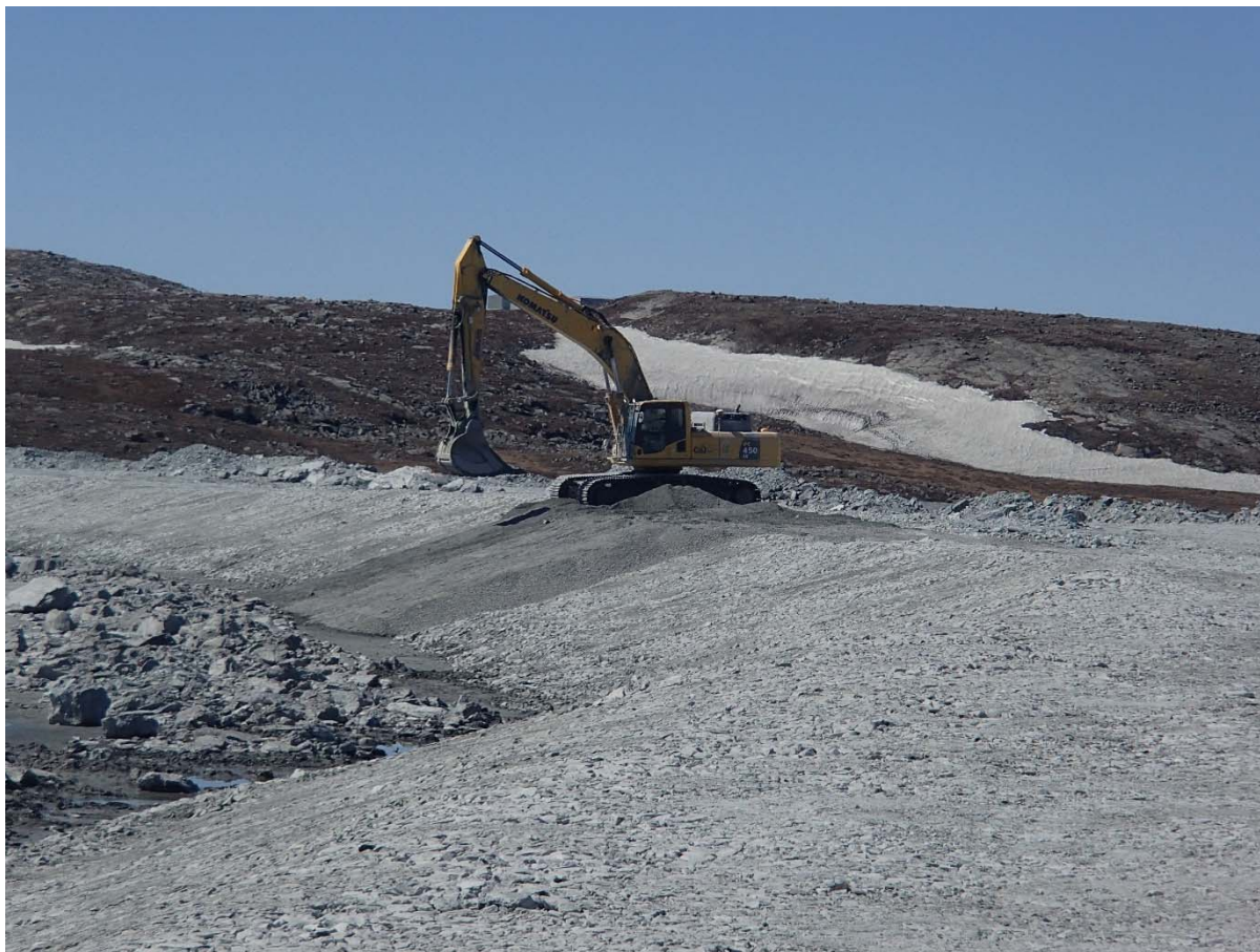
Photograph NCIS-039: From Sta. 2+200/-24 m (approx.), looking W. Placement of a 0.5 m thick lift of fine filter over the coarse filter in the upstream slope from El. 150 m to 152 m with an excavator from Sta. 2+460 m to 2+475 m and from Sta. 2+065 m to 1+980 m.
