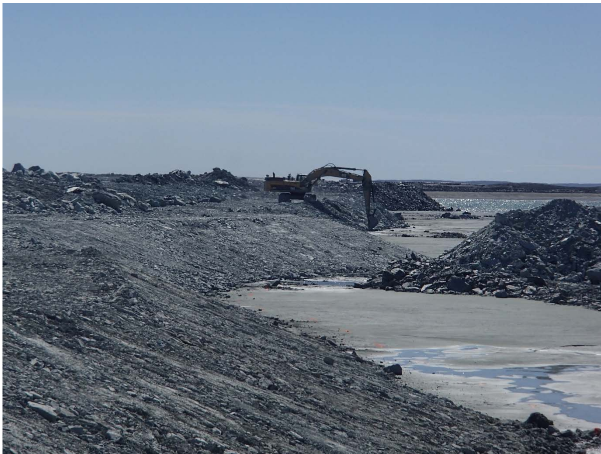
Photograph NCIS-072: From Sta. 2+790/-38 m (approx.), looking W. Profiling of the upstream slope (3H:1V) from El. 150 to 152 m with an excavator from Sta. 2+975 m to 3+070 m.
