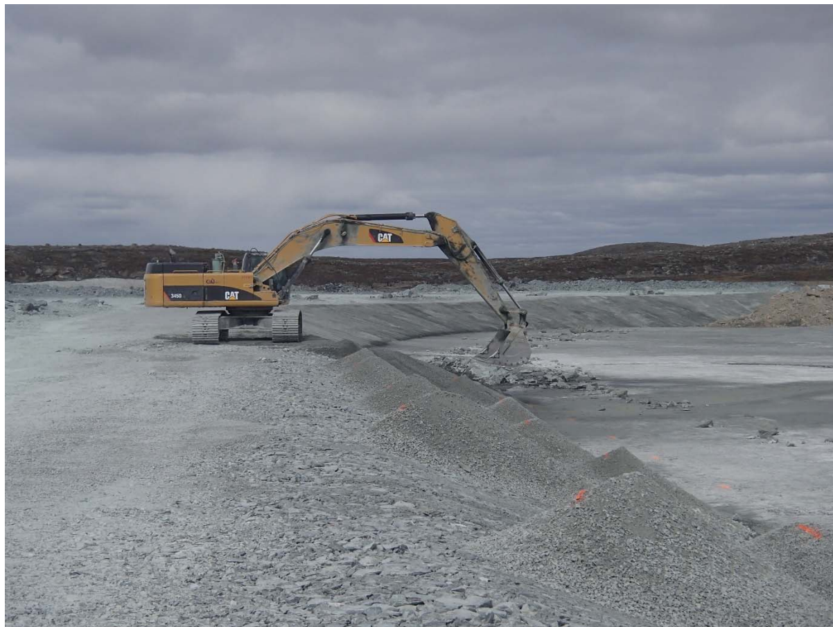
Photograph NCIS-062: From Sta. 1+525/-33 m (approx.), looking N. Placement of a 0.5 m thick lift of fine filter over the coarse filter in the upstream slope from El. 150 m to 152 m with an excavator from Sta. 1+330 m to 1+260 m and from Sta. 1+595 m to 1+550 m.
