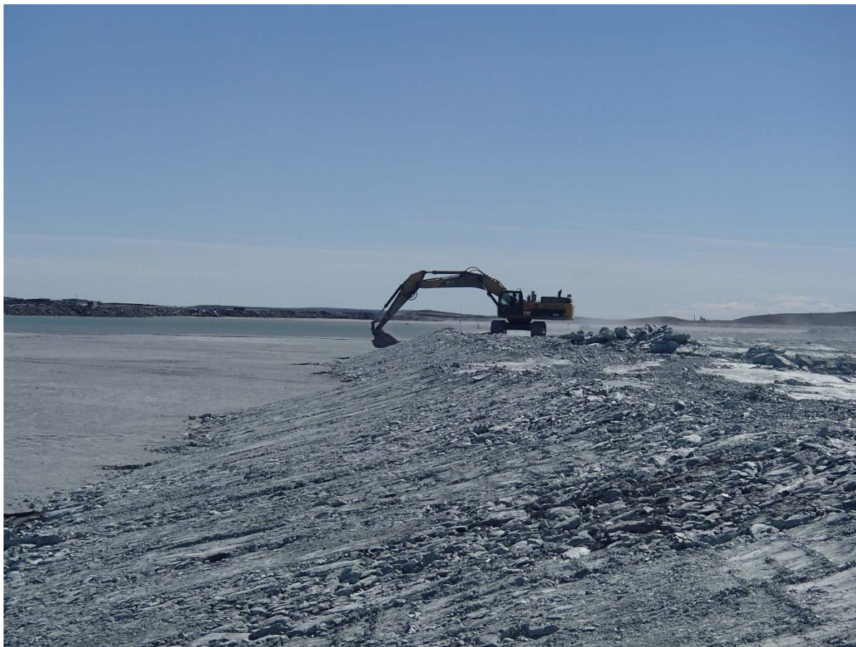
Photograph NCIS-056: From Sta. 1+290/-39 m (approx.), looking S. Profiling of the upstream slope (3H:1V) from El. 148 to 150 m with an excavator from Sta. 1+340 m to 1+130 m.
