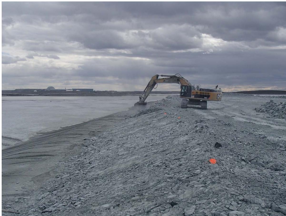
Photograph NCIS-077: From Sta. 1+310/-32 m (approx.), looking S. Profiling of the upstream slope (3H:1V) from El. 150 to 152 m with an excavator from Sta. 1+300 m to 1+175 m and from 3+070 m to 3+160 m.
