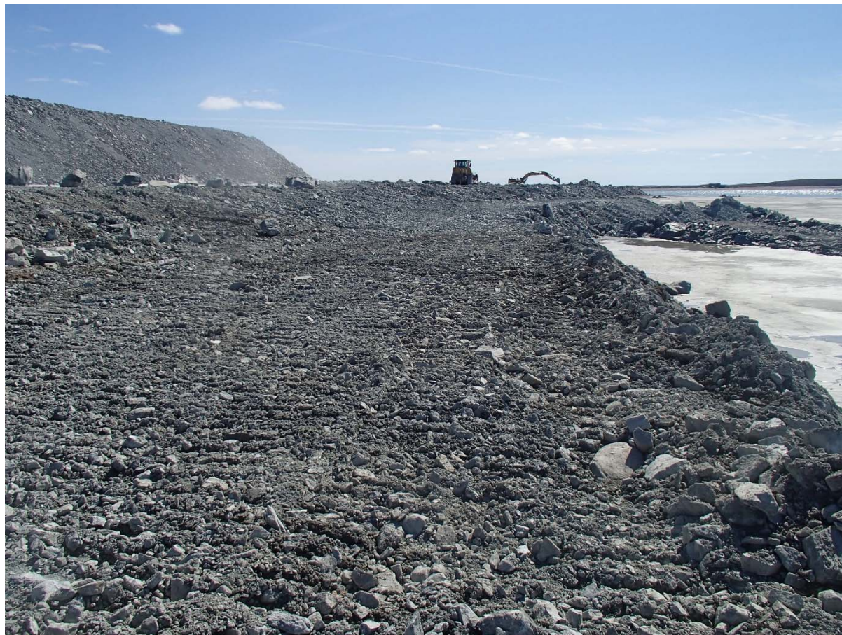
Photograph NCIS-053: From Sta. 2+840/-37 m (approx.), looking S. Removing of UM rockfill material from the capping with a dozer to level the surface to El. 152 m from Sta. 2+850 m to 2+980 m (offset -38 to -24 m).
