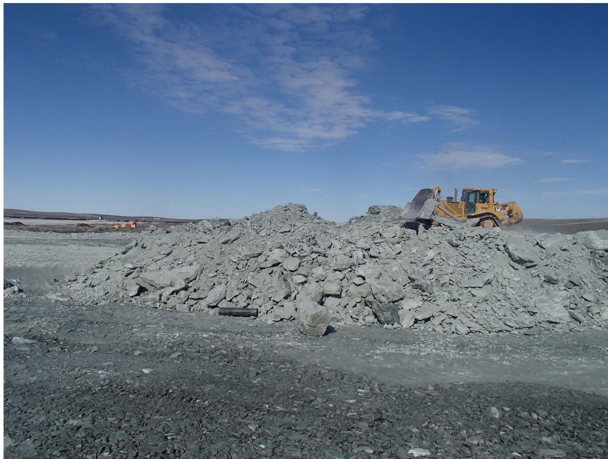
Photograph NCIS-064: From Sta. 1+200/-65 m (approx.), looking W. Placement of a 2 m thick (approx.) lift of UM rockfill from El. 150 m to El. 152 m (approx.) with a dozer from Sta. 1+320 m to 1+235 m (-65 m to -45 m). The material is of good quality and is well graded.
