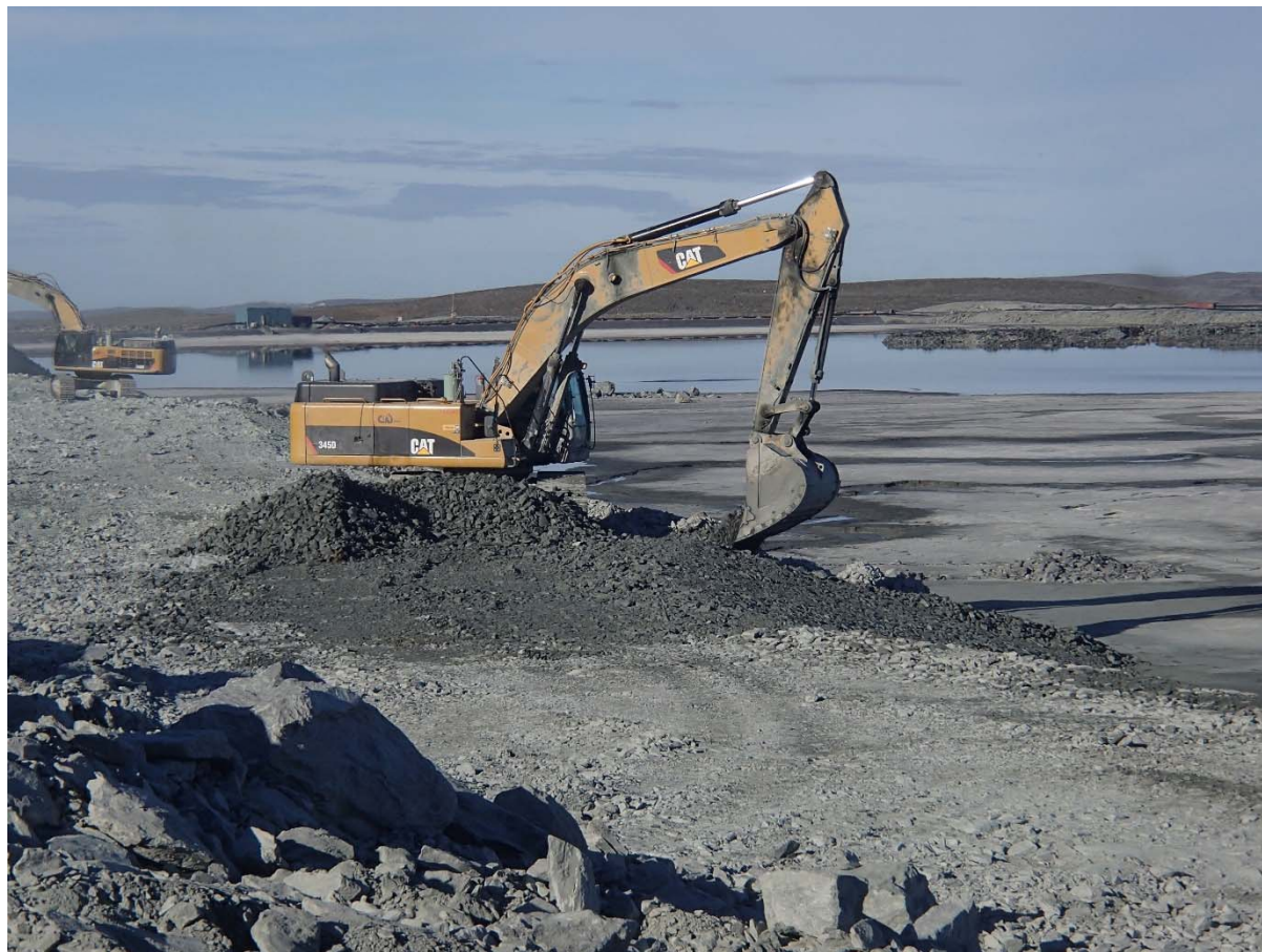
Photograph NCIS-076: From Sta. 2+940/-15 m (approx.), looking SW. Placement of a 0.5 m thick lift of coarse filter in the upstream slope from El. 150 m to 152 m with an excavator from Sta. 2+980 m to 3+160 m.
