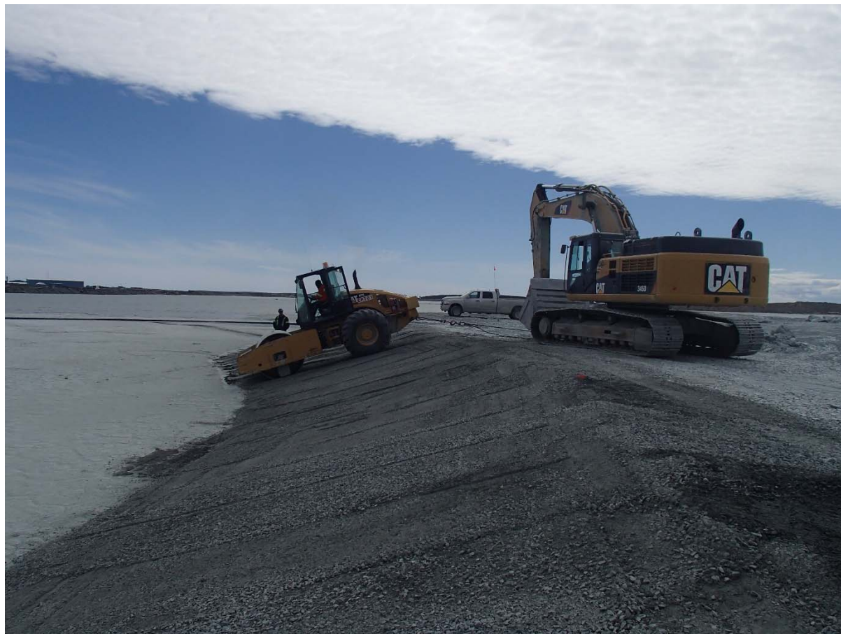
Photograph NCIS-070: From Sta. 1+160/-89 m (approx.), looking S. Compaction of the 0.5 m lift of fine filter between El. 150 and 152 m with a 10-tonne smooth-drum compactor with vibration (4 passes) in the upstream slope from Sta. 1+335 m to 1+100 m.
