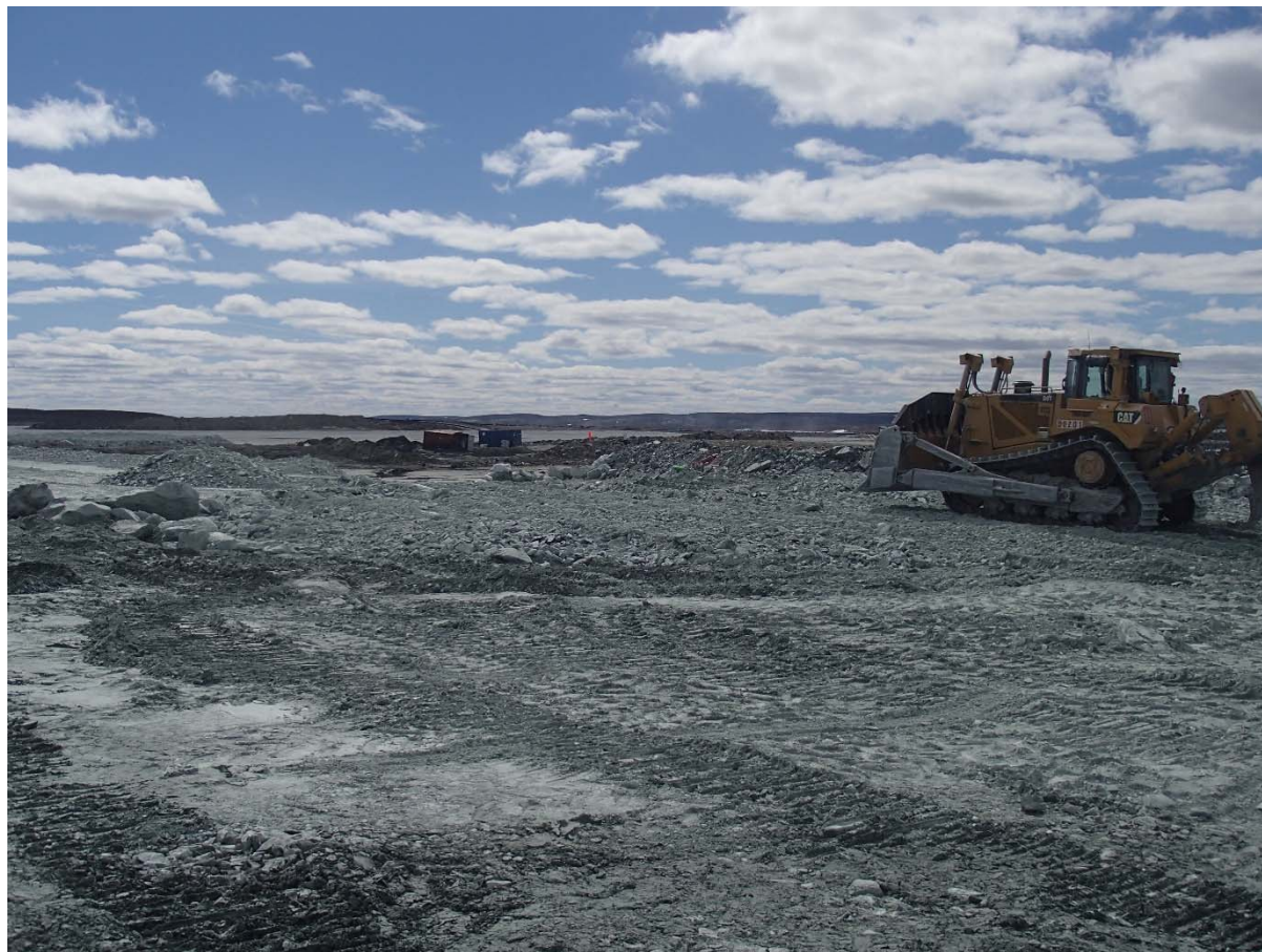
Photograph NCIS-060: From Sta. 1+365/-35 m (approx.), looking SW. Placement of a 2 m thick (approx.) lift of UM rockfill from El. 150 m to El. 152 m (approx.) with a dozer from Sta. 1+340 m to 1+320 m (-19 m to +16 m). The material is of good quality and is well graded.
