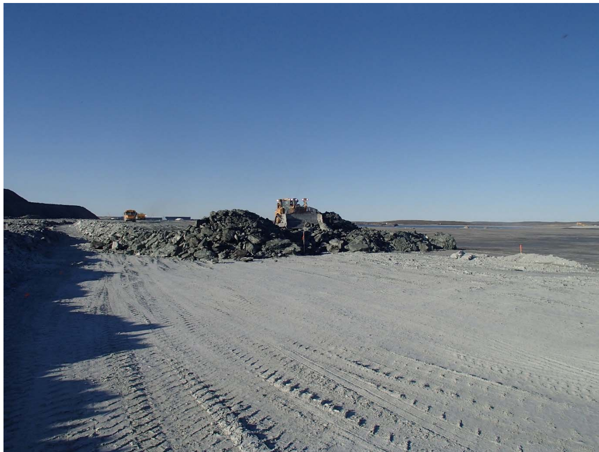
Photograph NCIS-093: From Sta 2+260/+12 m (approx.), looking S. Placement of a 2 m thick (approx.) lift of UM rockfill from El. 152 m to El. 154 m (approx.) with a dozer from Sta. 2+290 m to 2+280 m (+9 m to -22 m).
