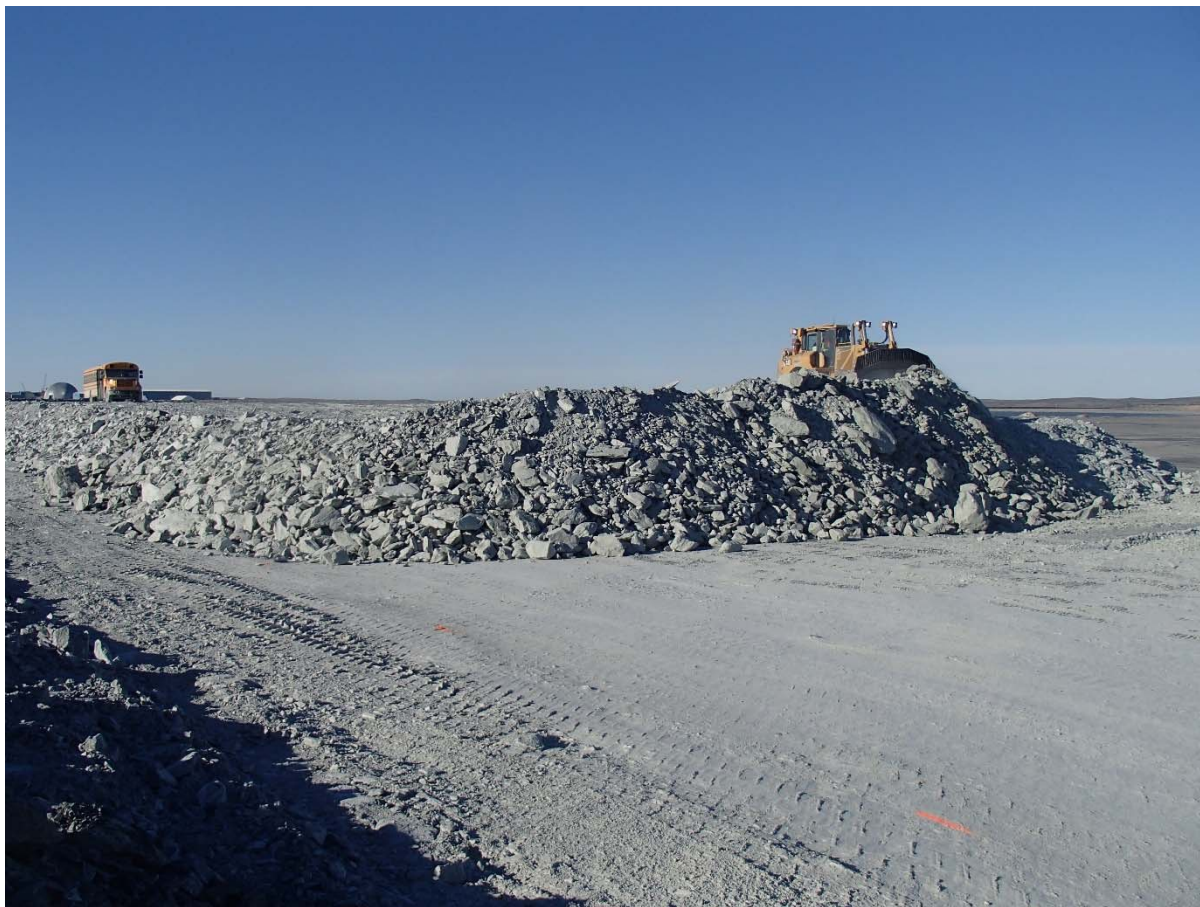
Photograph NCIS-091: From Sta 2+330/+13 m (approx.), looking S. Placement of a 2 m thick (approx.) lift of UM rockfill from El. 152 m to El. 154 m (approx.) with a dozer from Sta. 2+370 m to 2+290 m (+9 m to -22 m). The material is of good quality and is well graded.
