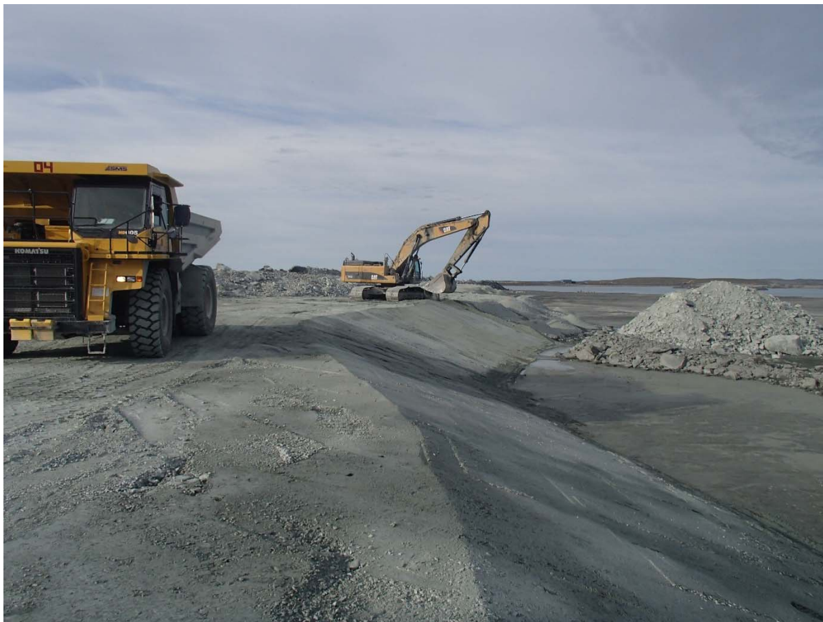
Photograph NCIS-081: From Sta2+975/-37 m (approx.), looking SE. Placement of a 0.5 m thick lift of fine filter over the coarse filter in the upstream slope from El. 150 m to 152 m with an excavator from Sta. 1+300 m to 1+210 m and from Sta. 2+940 m to 3+120 m.
