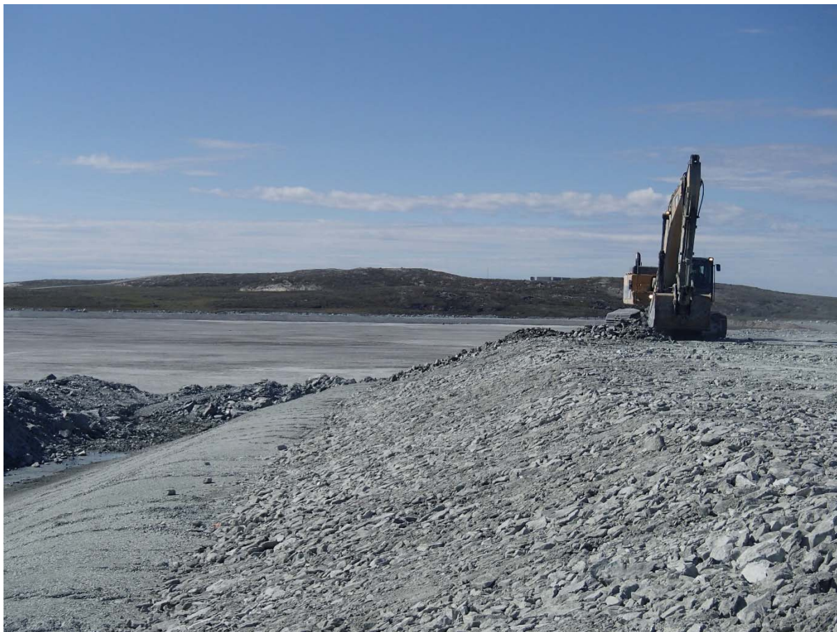
Photograph NCIS-102: From Sta. 2+680/-21 m (approx.), looking W. Placement of a 0.5 m thick lift of coarse filter in the upstream slope from El. 152 m to 154 m with an excavator from Sta. 2+575 m to 2+710 m and from Sta. 2+411 m to 2+460 m.
