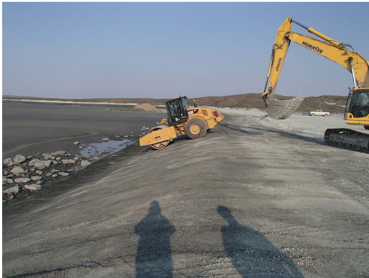
Photograph NCIS-088: From Sta 2+000/-35 m (approx.), looking W. Compaction of the 0.5 m lift (approx.) of fine filter between El. 150 m and 152 m with a 10-tonne smooth-drum compactor (4 passes) in the upstream slope from Sta. 2+028 m to 1+650 m.
