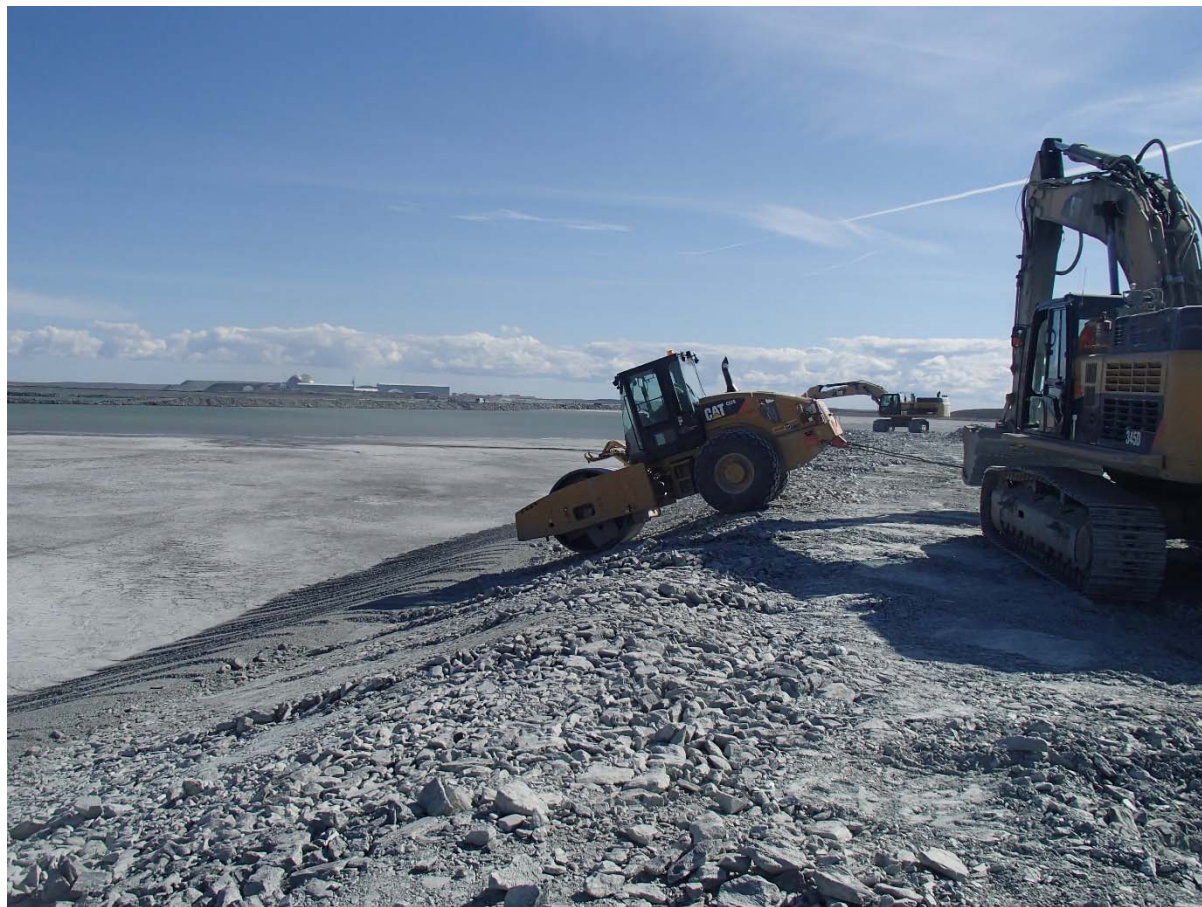
Photograph NCIS-099: From Sta. 1+180/-76 m (approx.), looking SE. Compaction of the 0.5 m lift (approx.) of coarse filter between El. 150 m and 152 m with a 10-tonne smooth-drum compactor with vibration (4 passes) in the upstream slope from Sta. 1+200 m to 1+170 m.
