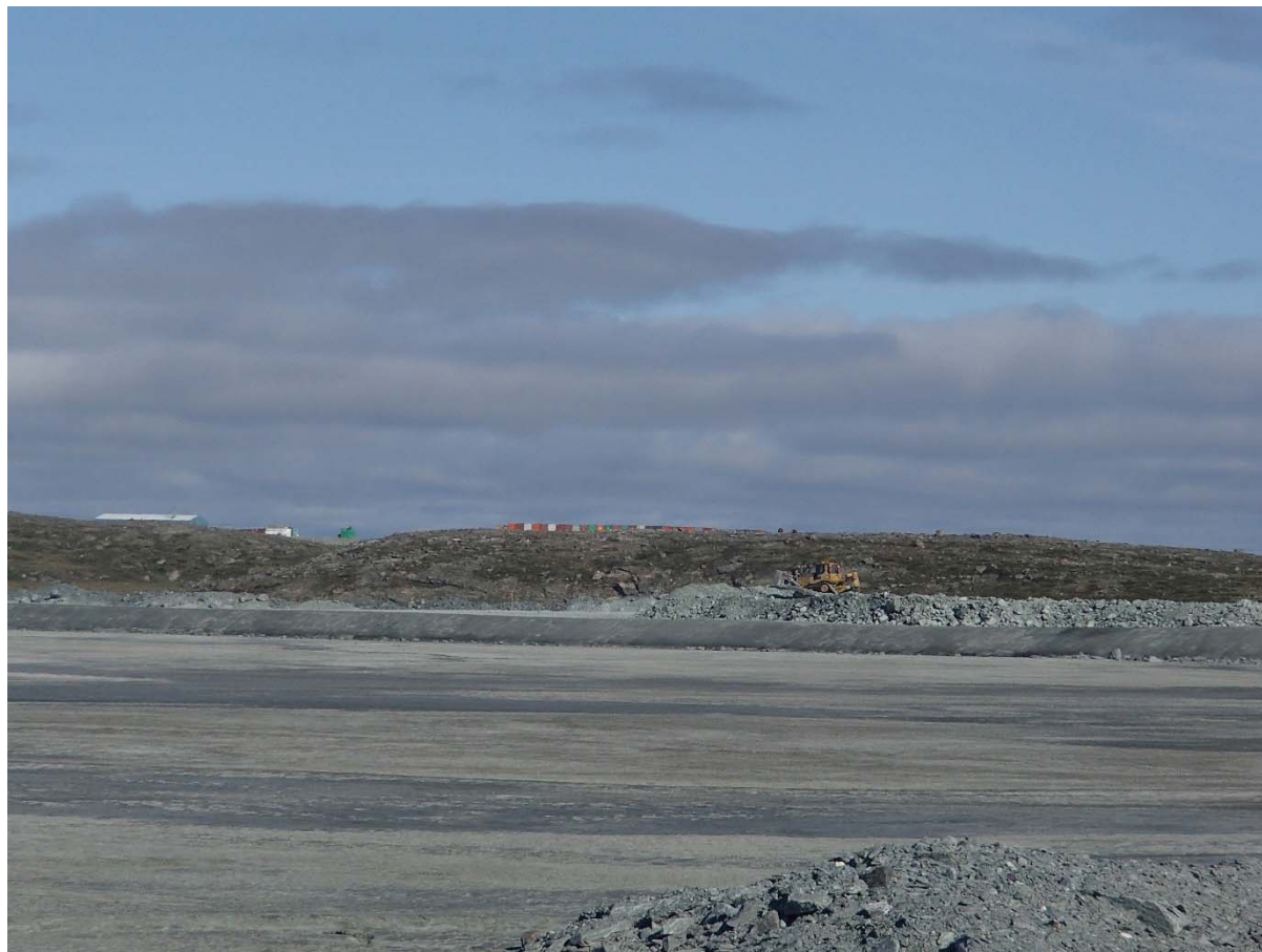
Photograph NCIS-106: From Sta. 2+620/-35 m (approx.), looking NW. Placement of a 2 m thick (approx.) lift of UM rockfill from El. 152 m to El. 154 m (approx.) with a dozer from Sta. 1+947 m to 1+863 m (+14 m to -26 m). The material is of good quality and is well graded.
