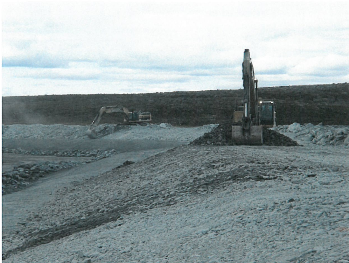
Photograph NCIS-109: From Sta. 2+450/-21 m (approx.), looking N. Placement of a 0.5 m thick lift of coarse filter in the upstream slope from El. 152 m to 154 m with an excavator from Sta. 2+293 m to 2+411 m.
