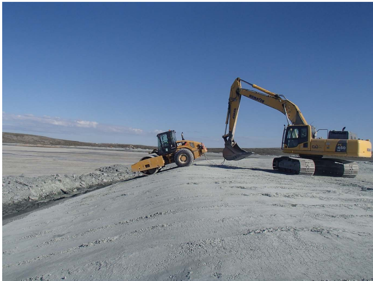
Photograph NCIS-112: From Sta. 2+610/-29 m (approx.), looking N. Compaction of the 0.5 m lift (approx.) of coarse filter between El. 152 m and 154 m with a 10-tonne smooth-drum compactor with vibration (4 passes) in the upstream slope from Sta. 2+080 m to 2+000 m.
