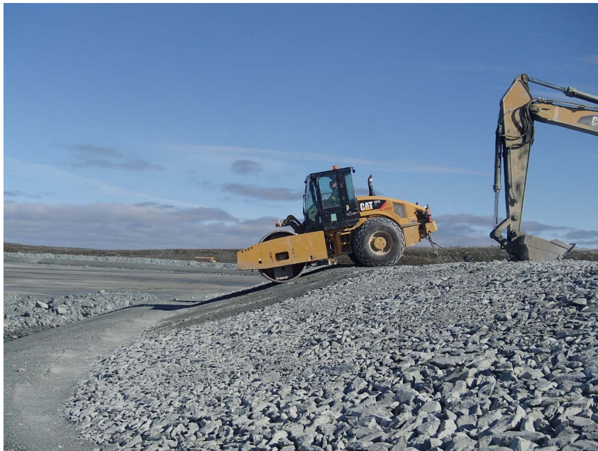
Photograph NCIS-105: From Sta. 2+630/-34 m (approx.), looking NW. Compaction of the 0.5 m lift (approx.) of coarse filter between El. 152 m and 154 m with a 10-tonne smooth-drum compactor with vibration (4 passes) in the upstream slope from Sta. 2+710 m to 2+411 m.
