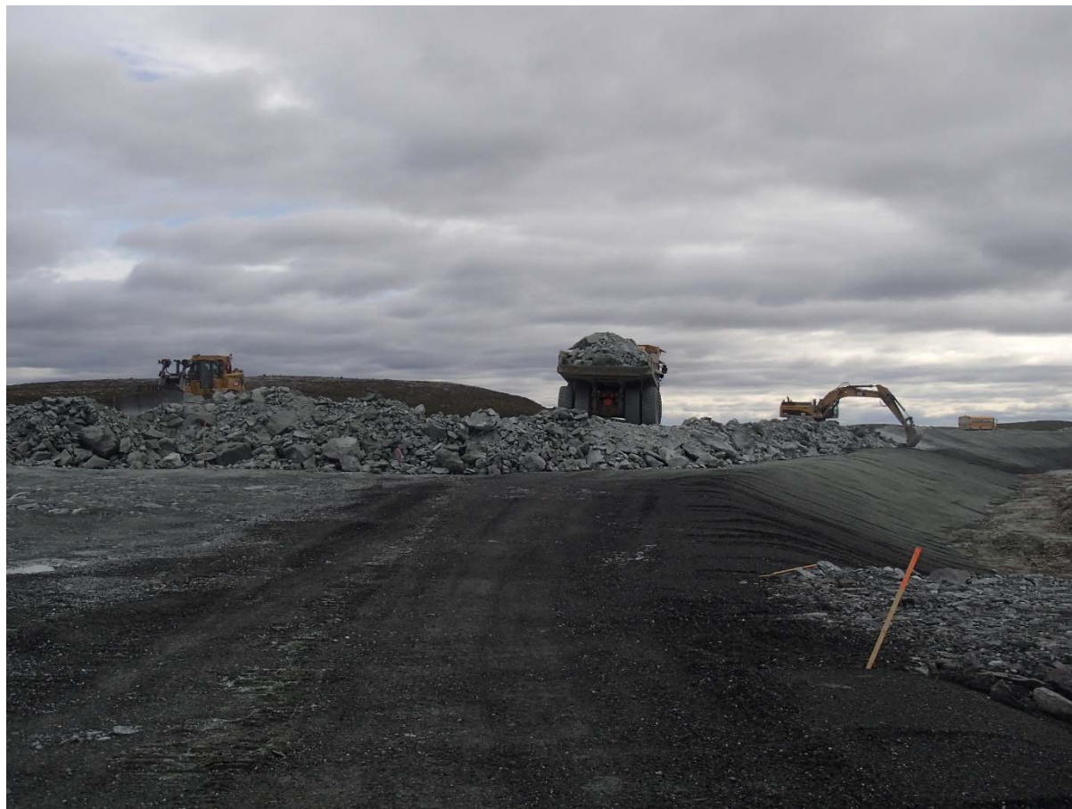
Photograph NCIS-128: From Sta. 1+680/-42 m (approx.), looking NE. Placement of a 2 m thick (approx.) lift of UM rockfill from El. 152 m to El. 154 m (approx.) with a dozer from Sta. 1+830 m to 1+660 m (+8 m to -31 m) and profiling of the upstream slope (3H:1V) from El. 152 to 154 m with an excavator from Sta. 1+880 m to 1+780 m.
