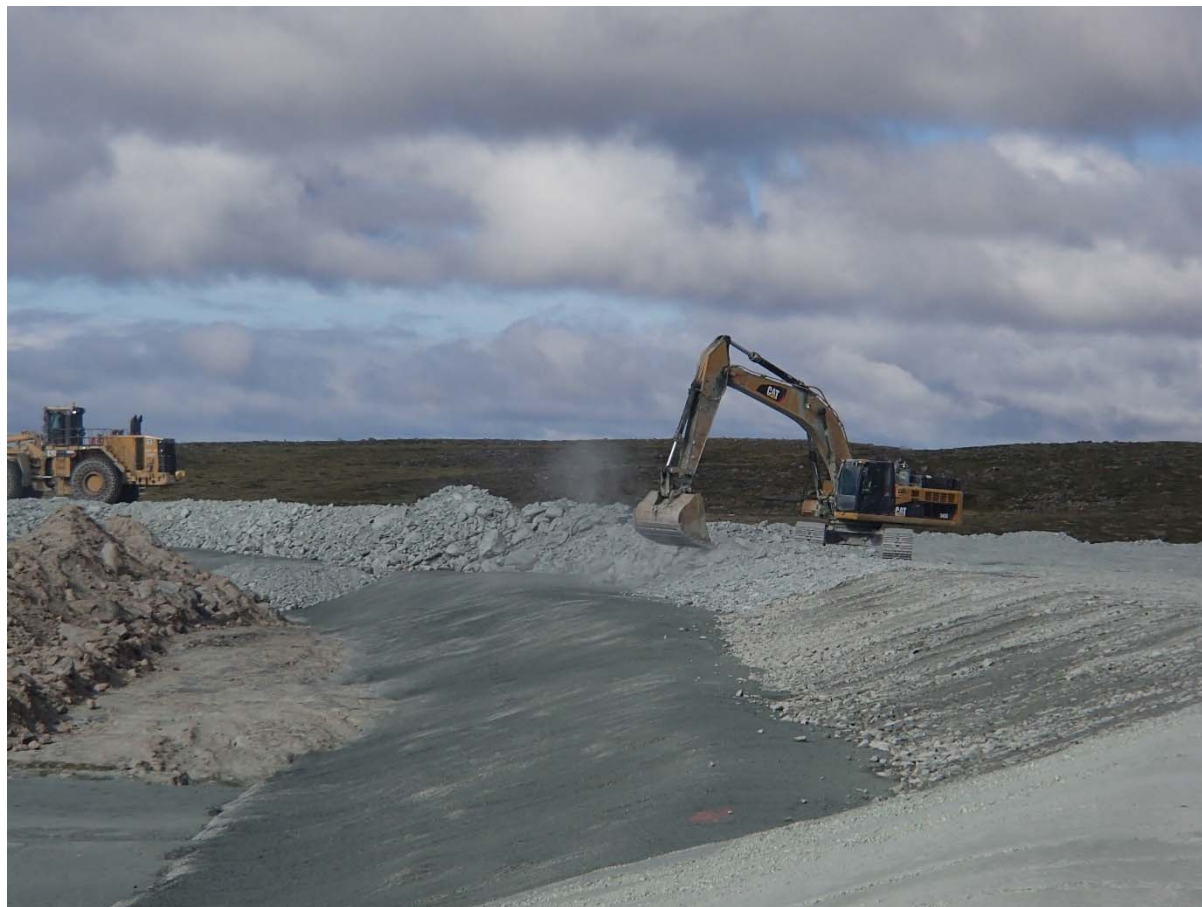
Photograph NCIS-132: From Sta. 1+940/-20 m (approx.), looking W. Profiling of the upstream slope (3H:1V) from El. 152 to 154 m with an excavator from Sta. 1+780 m to 1+660 m.
