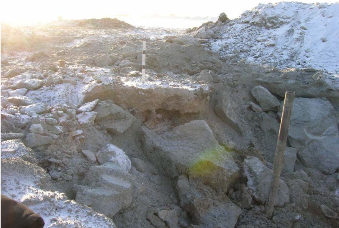
Photo 7 - "tube-a-manchette" (TAM) grouting tube (white) in test zone still to be excavated
