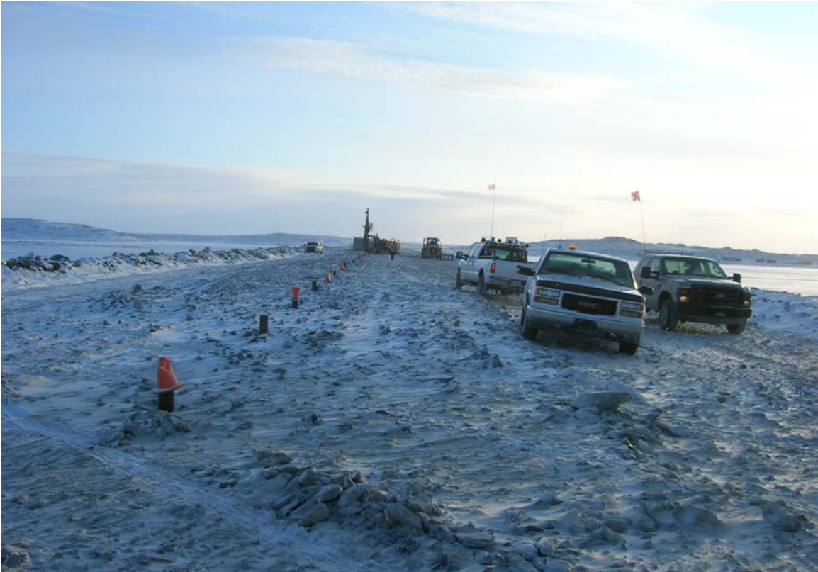
Photo 1 – East Dike crest with Primary holes grouted in casings protruding
