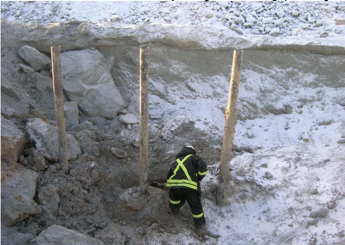
Photo 2 – Excavated grouted in casings and grout bulb at slurry wall rock contact
