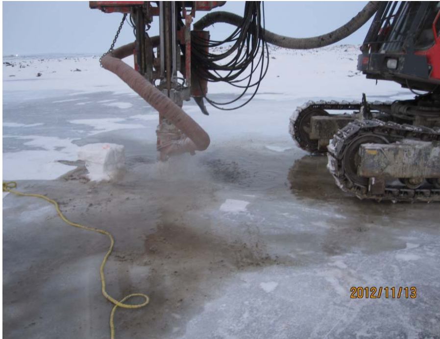
Picture B-1 Drilling Through Ice and Water Underneath
