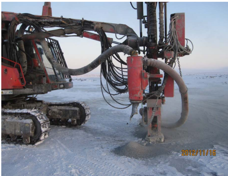
Picture B-2 Drilling at the Abutment
