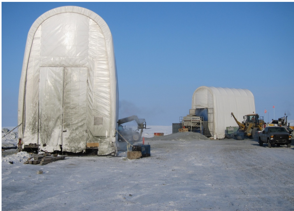
Photograph 104: Jet grouting coverall tents for drill rig and mixing station - April 18, 2011
