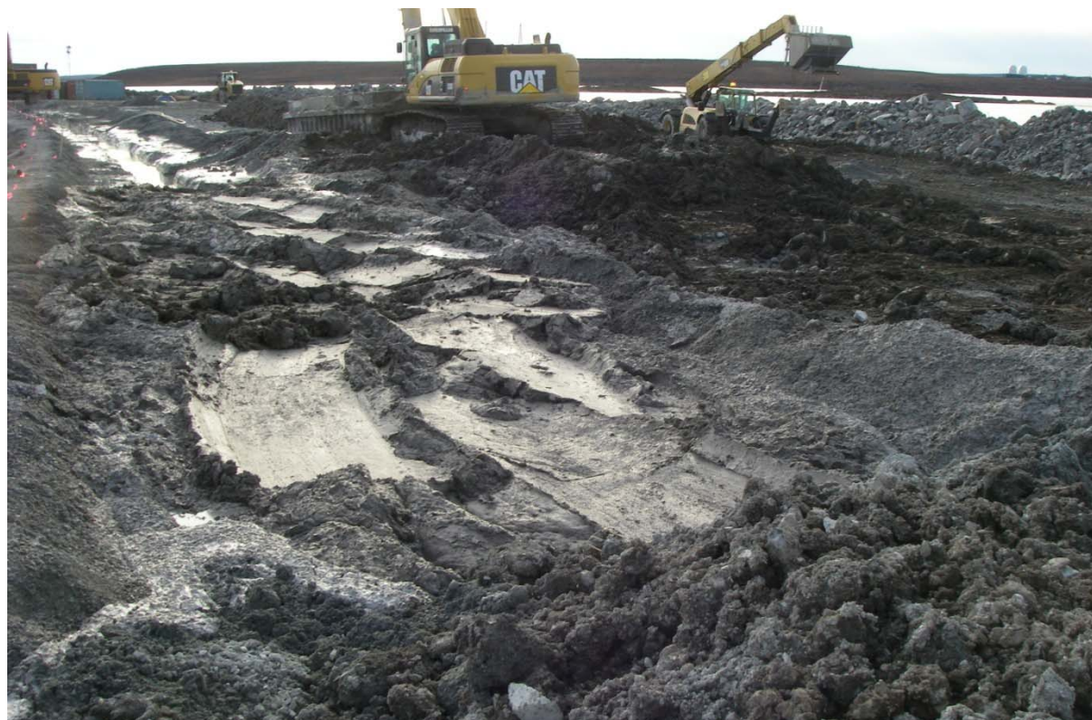
Photograph 32: Cement soil bentonite backfill within the cutoff trench - September 19, 2009
