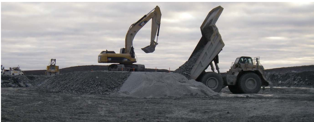
Photograph 23: Placement of the Densification Platform using Core Backfill in the center and Coarse Filter adjacent to the Core Backfill, Sta. 30+380 - September 4, 2009
