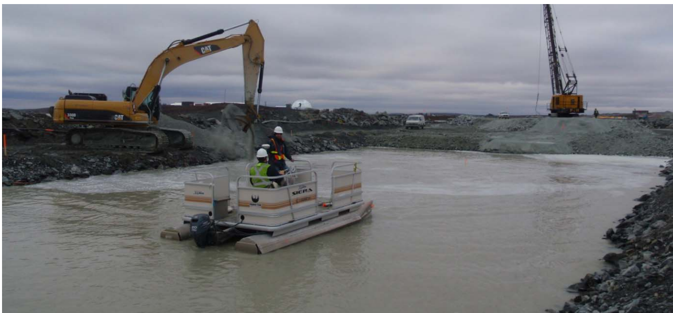
Photograph 14: Bathymetry survey by FGL between Sta. 30+800 and 30+860. Core Backfill placement on the downstream side and dynamic compaction of the core backfill - September 12, 2009
