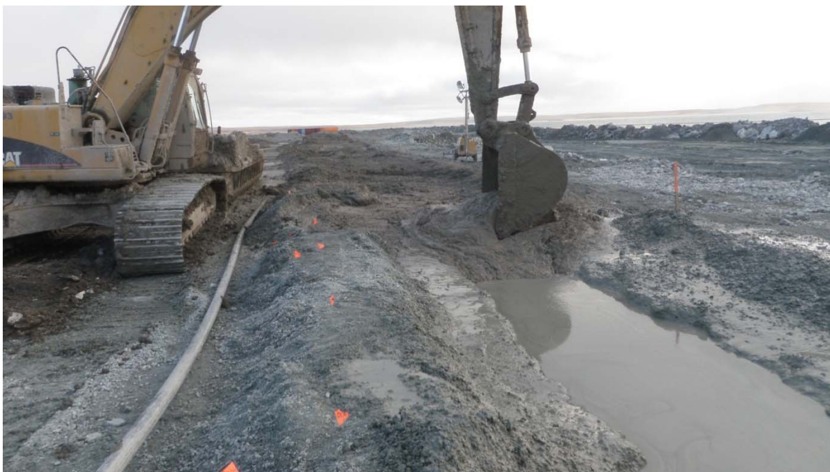
Photograph 84: Placement of cement soil bentonite mix within the cutoff trench, Sta. 31+900 - September 20, 2010
