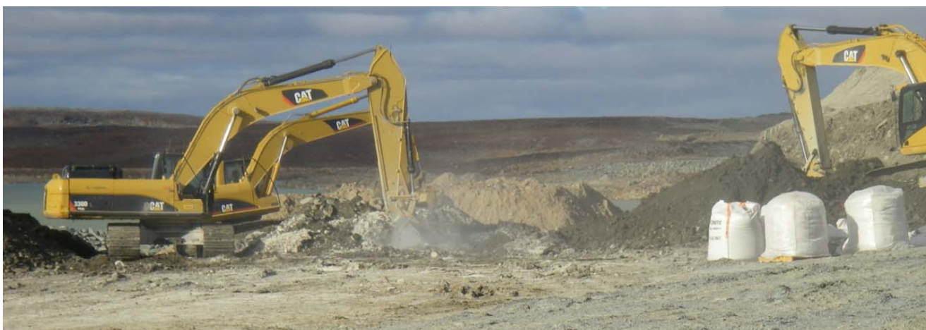
Photograph 26: Till screening to remove oversized particles and mixing of the till with dry bentonite powder - September 10, 2009
