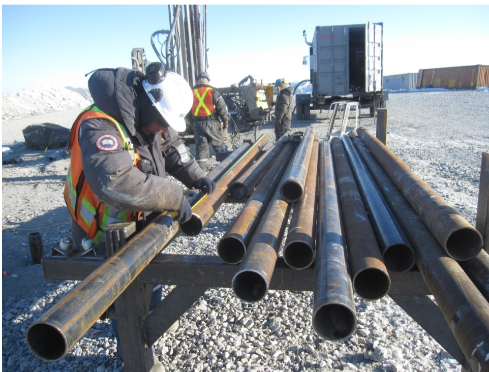
Photograph 100: QA measurement of installed casing lengths - May 2010
