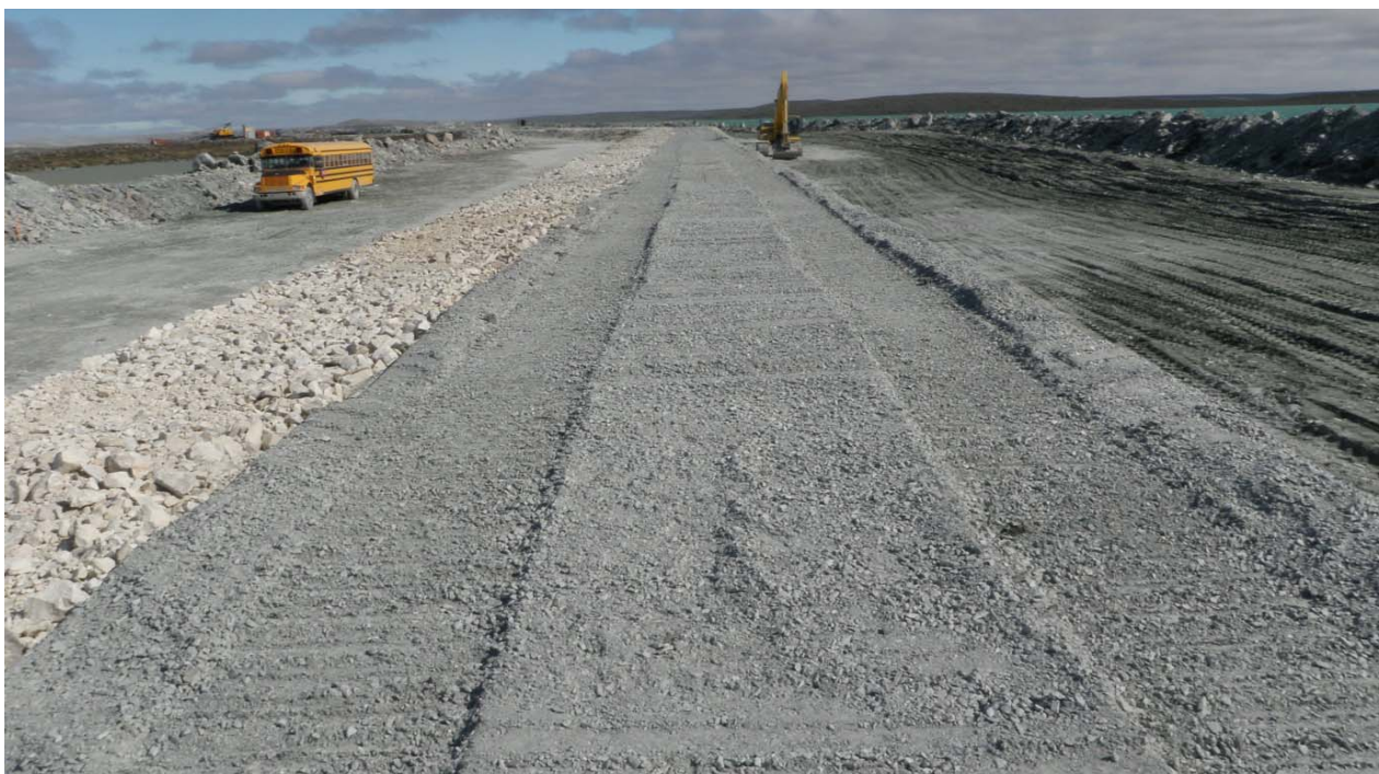
Photograph 72: Densification platform surface at Sta. 31+310. Coarse filter material placed on downstream side of platform - August 4, 2010
