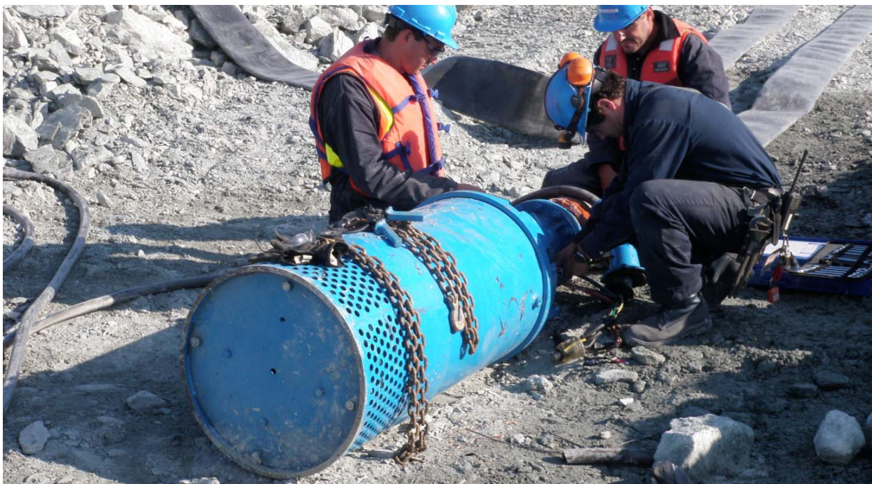
Photograph 51: Pump to be installed in excavation trench to pump water from trench to water management pond. Purpose was to try and reduce outward pressure on turbidity barriers through equalizing volumes of water being removed with those being displaced during material placement within trench - July 27, 2010
