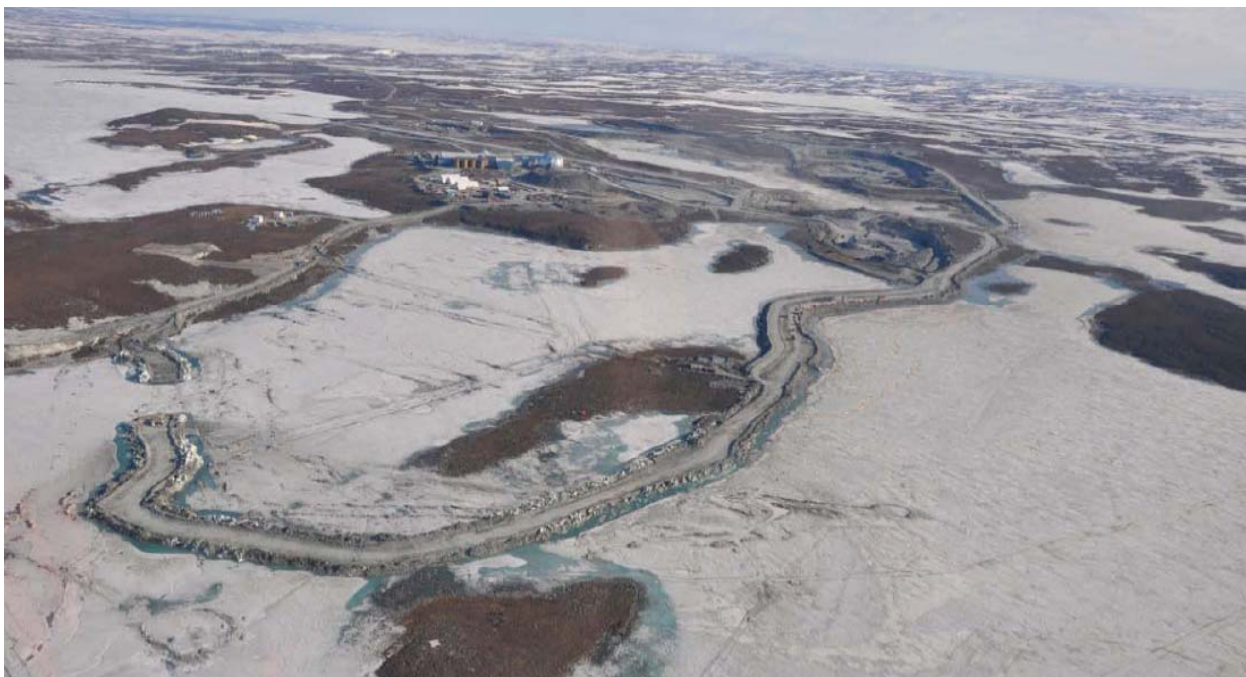
Photograph 41: Rockfill causeway construction from Goose Island to South Camp Island during winter 2010, to provide structure for anchoring turbidity barriers to for the remainder of the summer construction program - June, 2010
