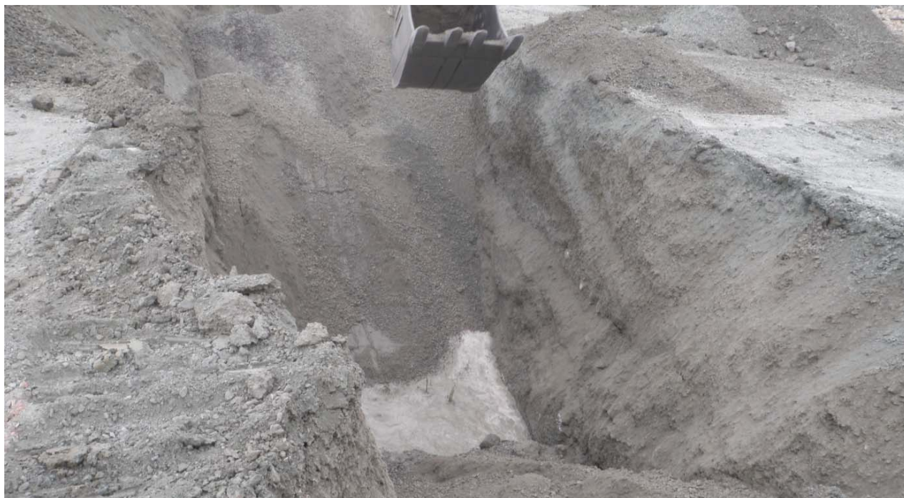
Photograph 77: Excavation of core backfill previously compacted with dynamic compaction at channel 3 in preparation for vibro-compaction – September 21, 2010
