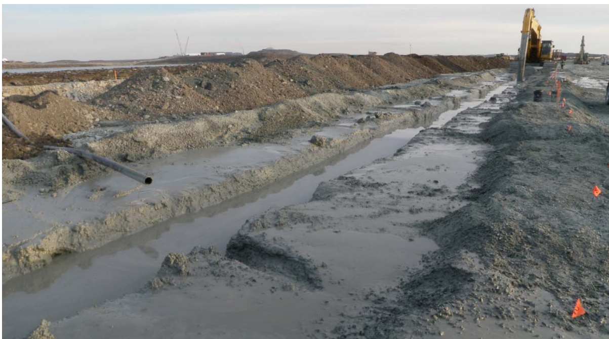
Photograph 82: Excavation of the cutoff trench at Sta. 31+091 and erosion of cutoff wall crest due to slurry placement – September 1, 2010
