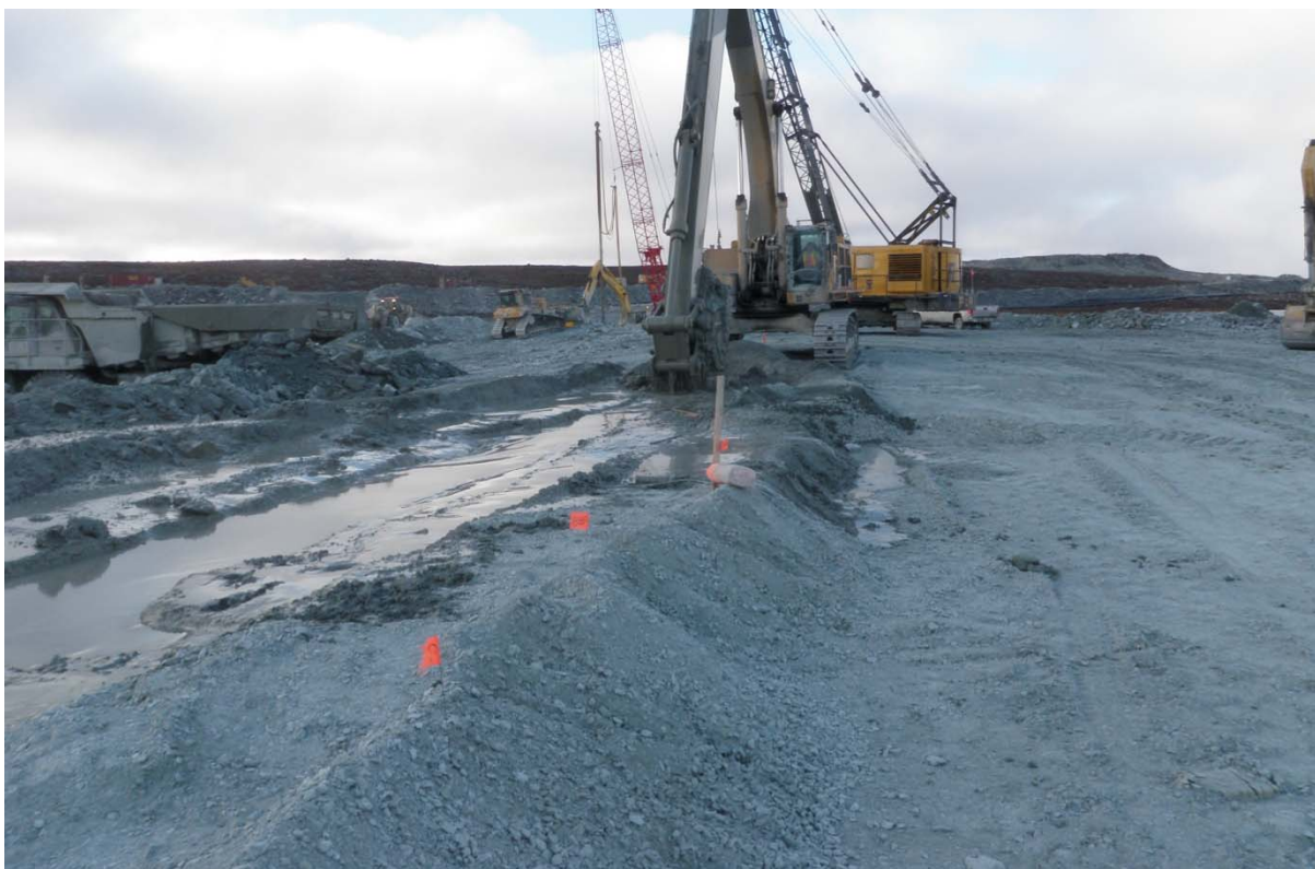
Photograph 85: Excavation of the cutoff trench at Sta. 31+984 – September 20, 2010
