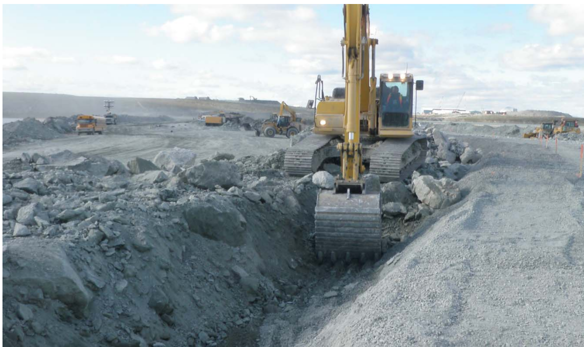
Photograph 75: Excavation of oversized fine rockfill on upstream side of densification platform in preparation for dynamic compaction - August 15, 2010
