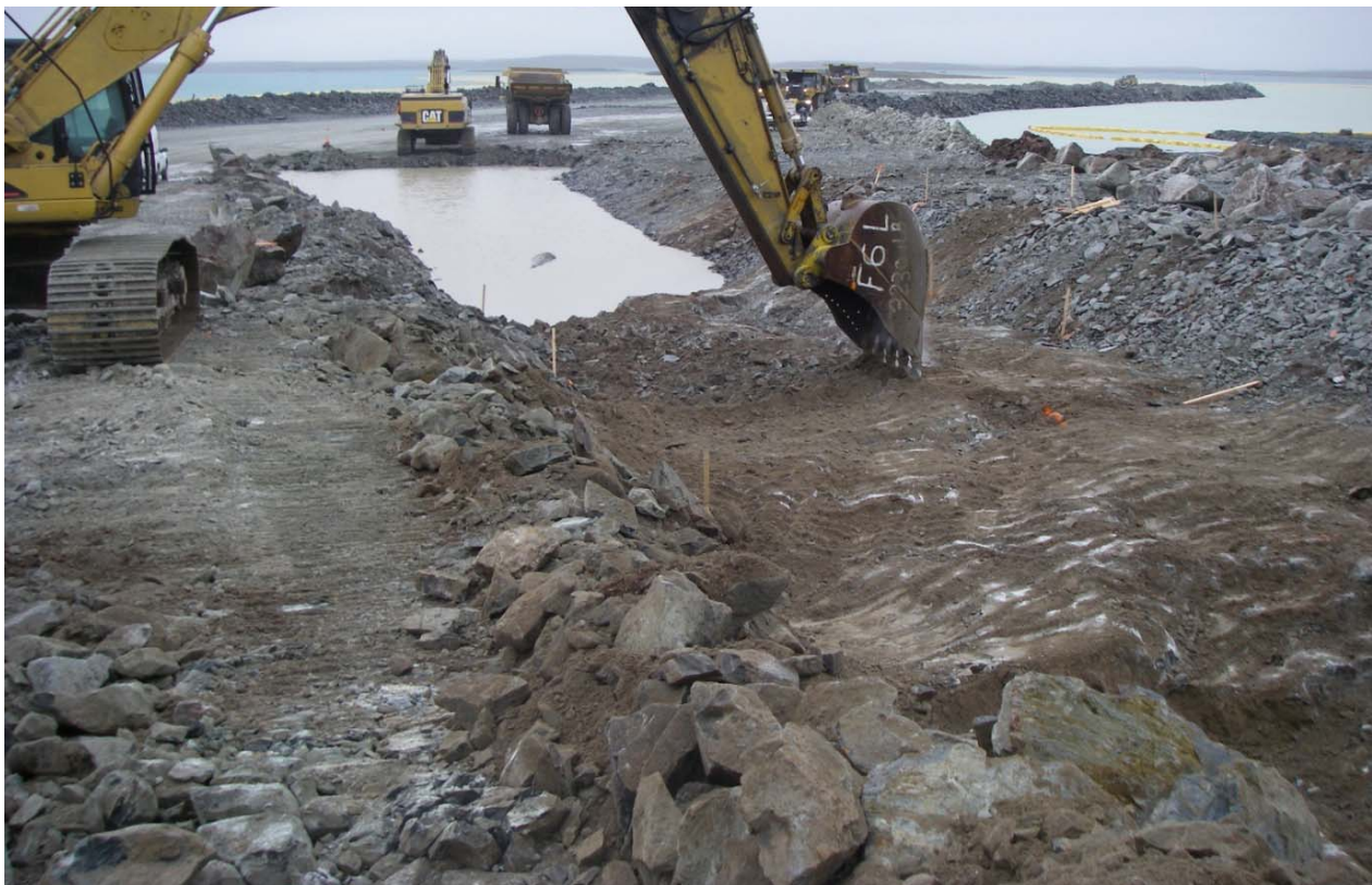
Photograph 37: Cleaning of the bedrock surface on the north abutment between Sta. 30+000 and 30+050 - August 12, 2009
