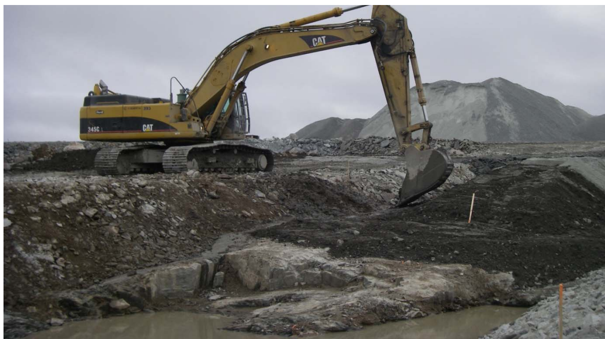
Photograph 39: Placement of till to form the north abutment cutoff between Sta. 30+000 and 30+050 - August 14, 2009
