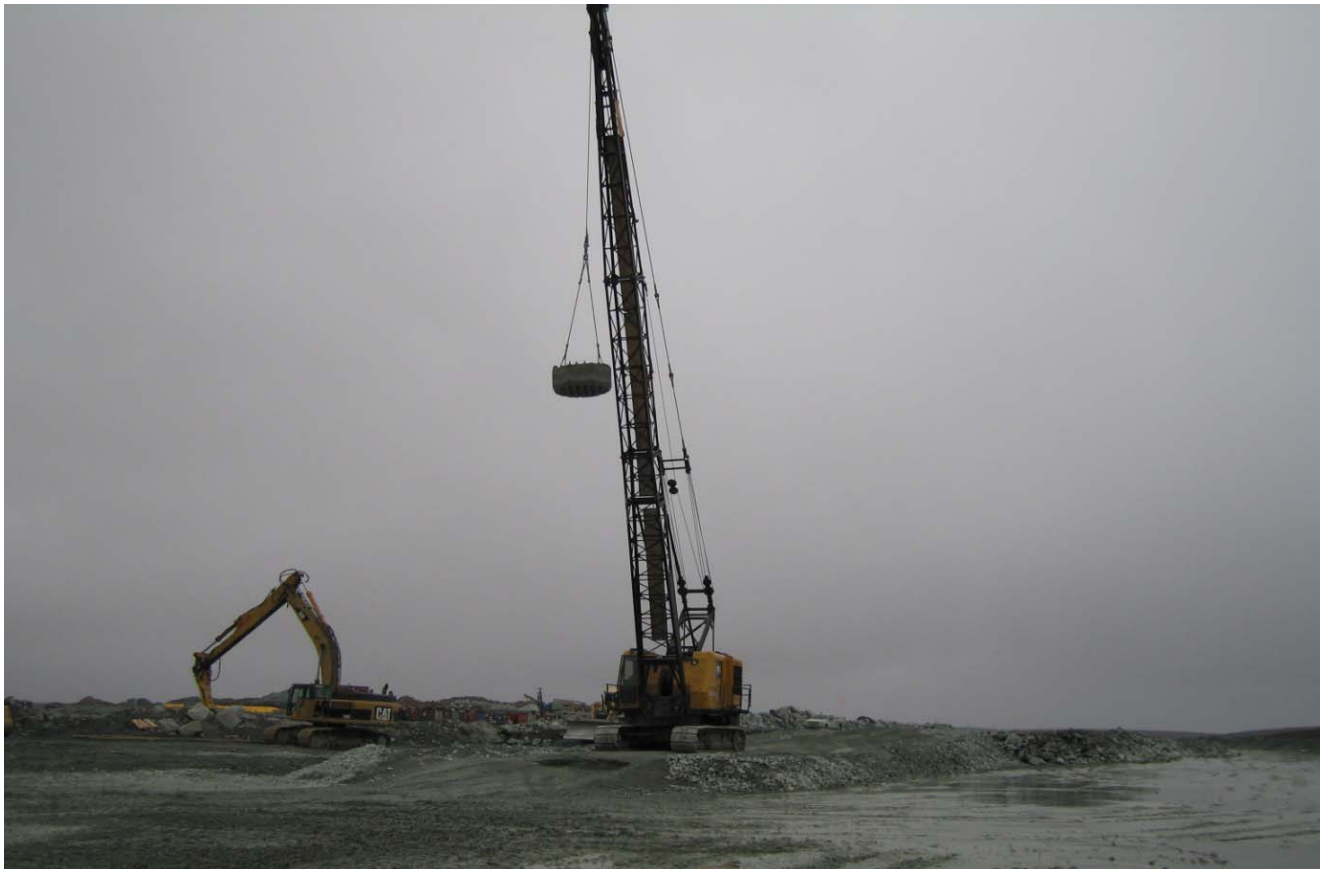
Photograph 21: Dynamic Compaction at Sta. 30+375 - September 2, 2009
