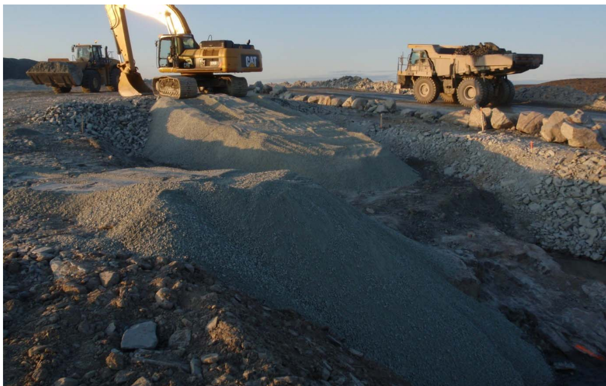
Photograph 40: Placement of 19 mm minus Core Backfill over the till placed on the north Abutment, Sta. 30+045 looking North - August 15, 2009
