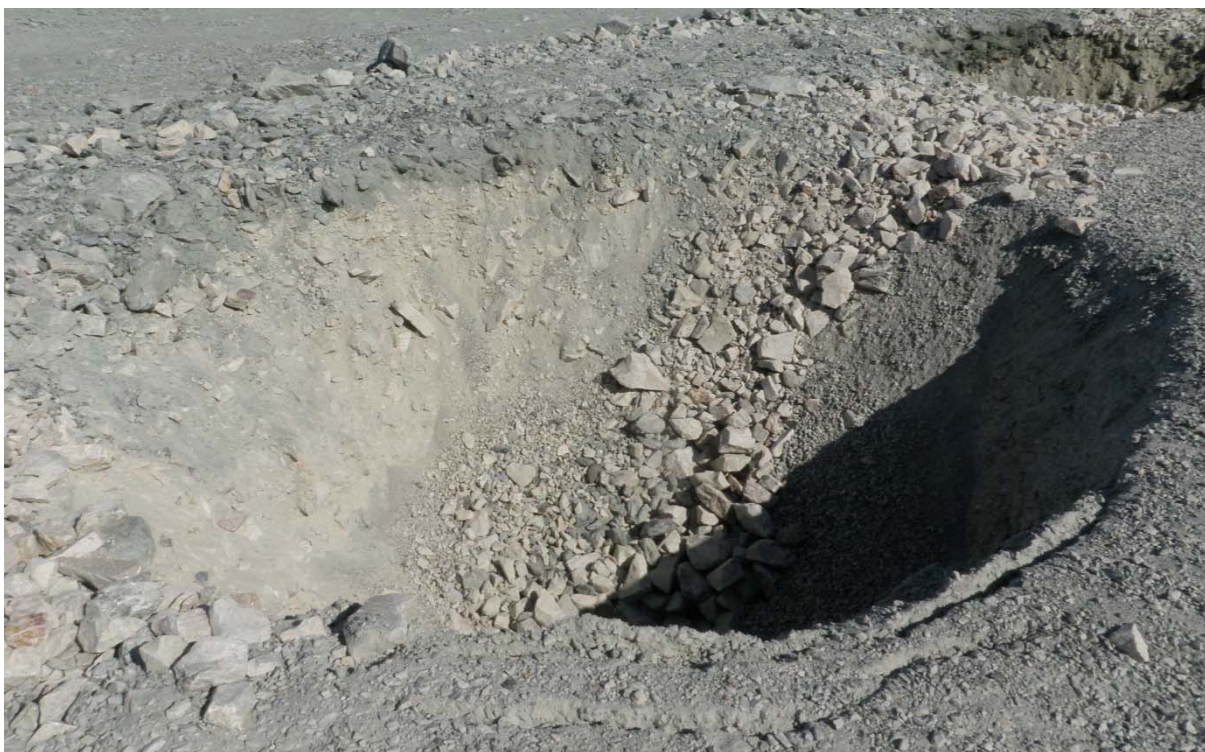
Photograph 74: Crater formed following dynamic compaction, Sta. 31+670 – August 15, 2010
