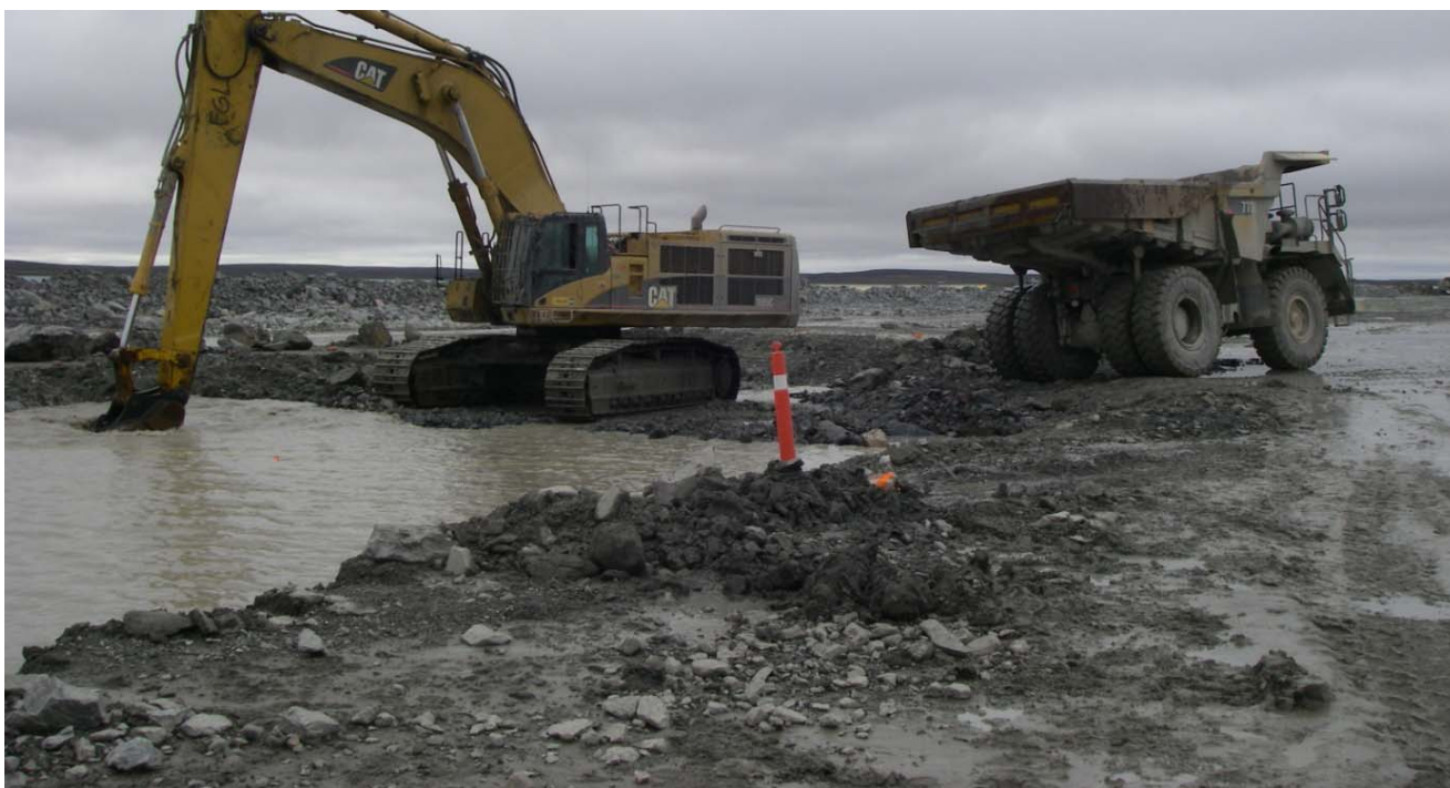
Photograph 6: Excavation of rockfill as part of the initial trench excavation, Sta. 30+200 - August 13, 2009
