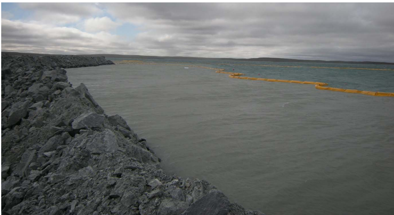
Photograph 45: Upstream turbidity barriers functioning during rockfill placement, Sta. 31+780 - August 4, 2010
