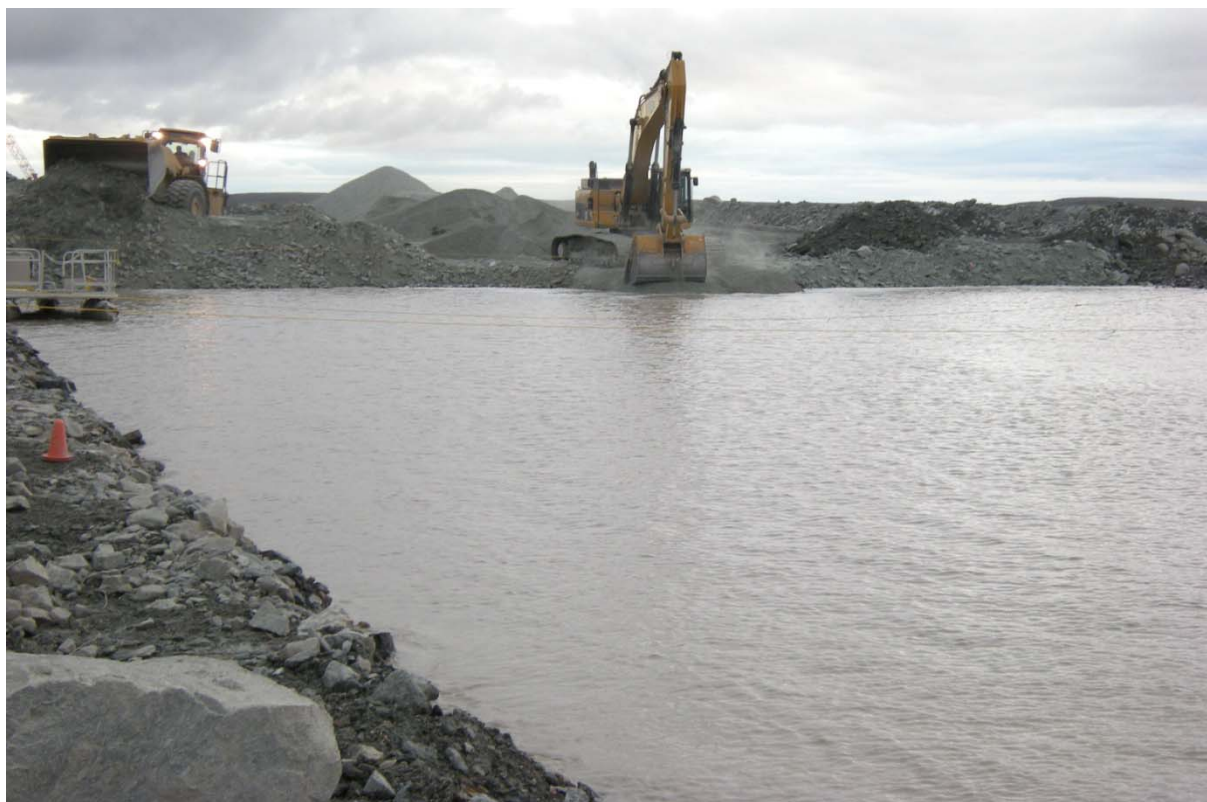
Photograph 67: Placement of core backfill material by pushing the core backfill forward and down. Coarse filter wing advanced with dozer on downstream side, Sta. 31+975 - August 25, 2010
