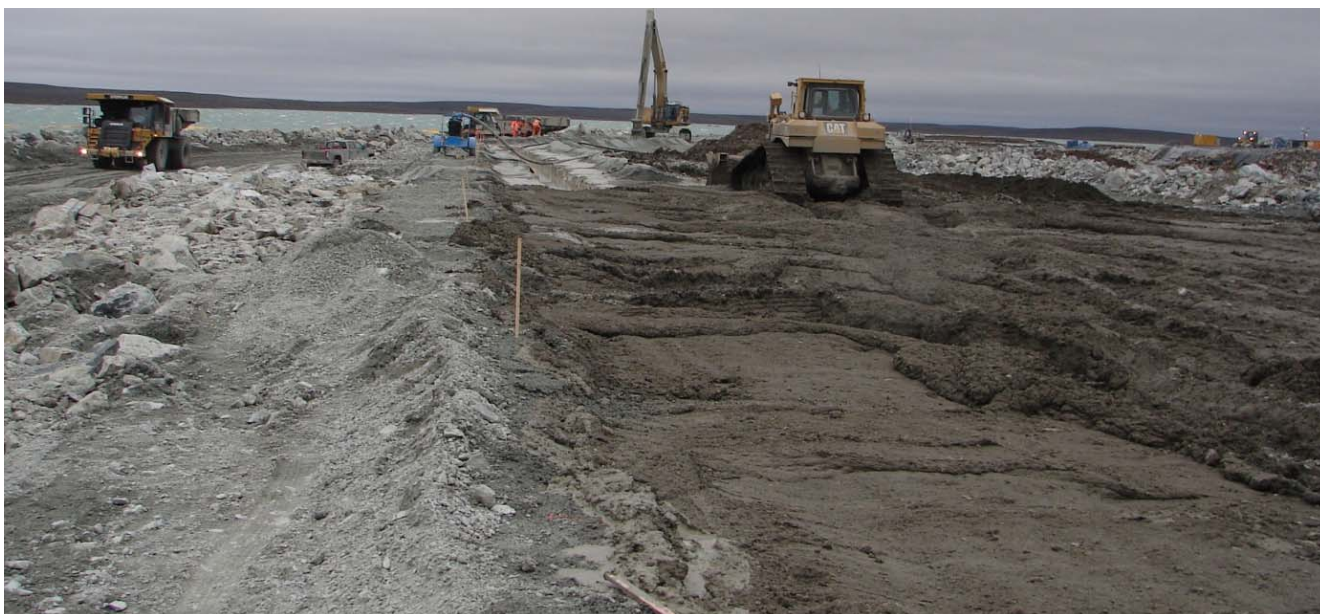
Photograph 34: Soil bentonite placed within the cutoff trench by a dozer, Sta. 30+628 to 670 - September 24, 2009
