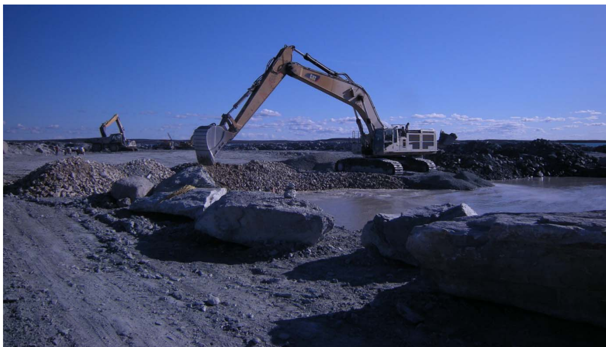
Photograph 65: Core backfill, coarse filter and fine rockfill placement at Sta. 31+835 - August 10, 2010
