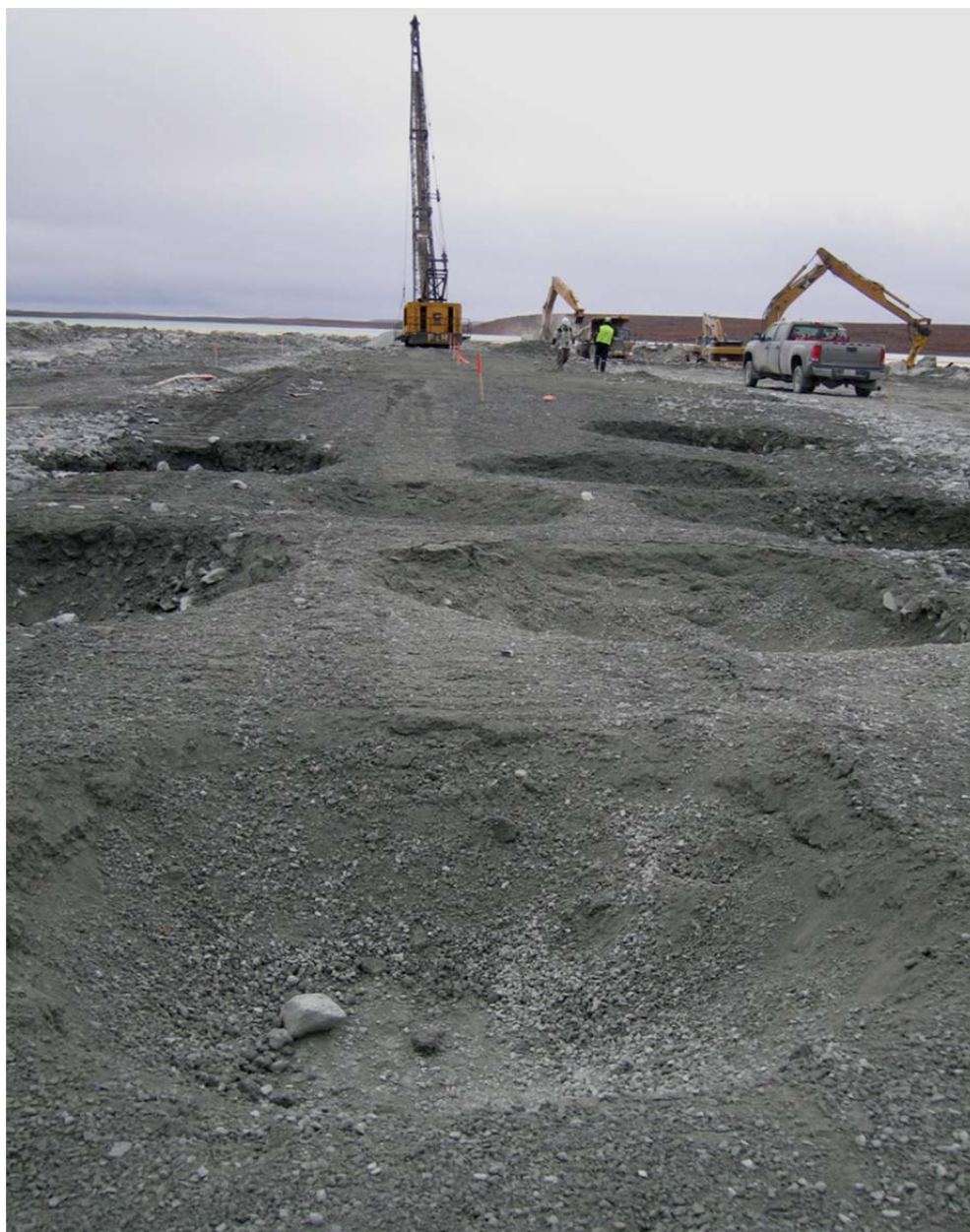
Photograph 22: Craters formed within the Core Backfill Zone following dynamic compaction, Sta. 30+230 looking north - September 2, 2009
