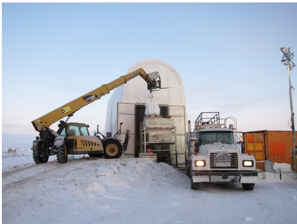
Photograph 105: Jet grouting cement supply by zoom boom and water truck - November 20, 2010
