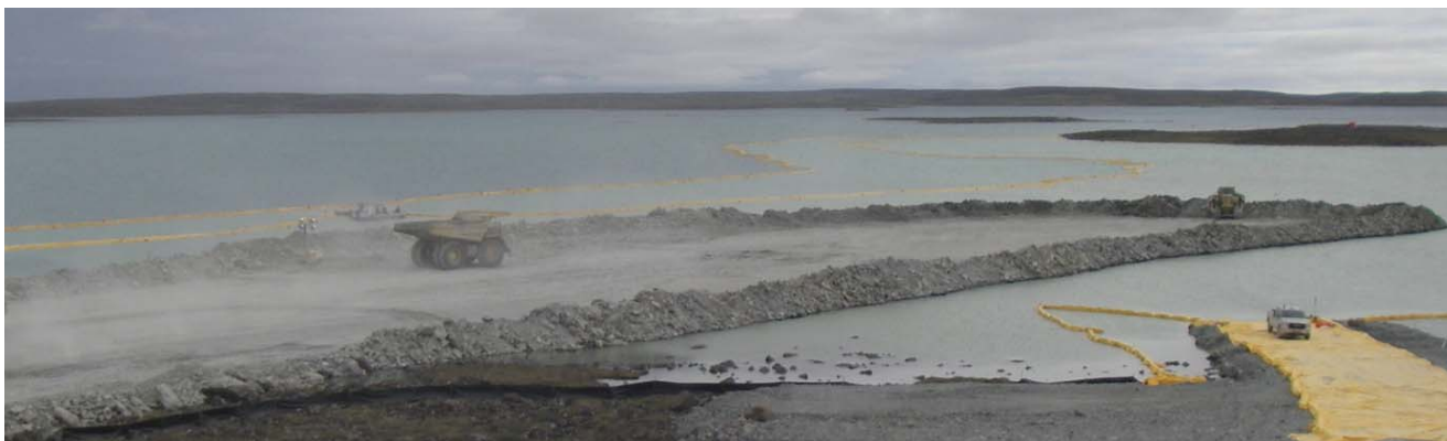
Photograph 1: Turbidity barriers functioning during rockfill placement - August 1, 2009
