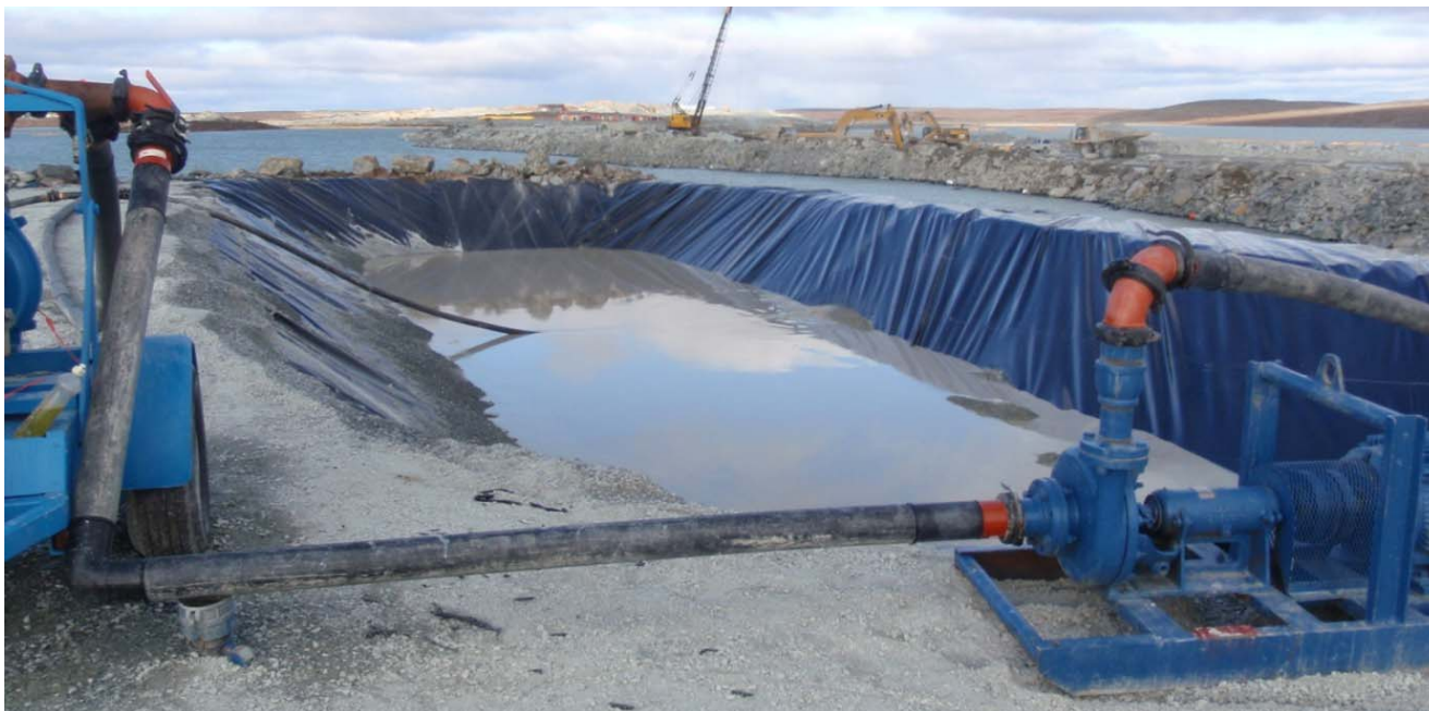
Photograph 25: Bentonite slurry pond constructed on Goose Island - September 10, 2009
