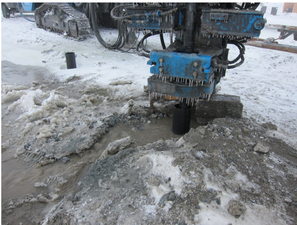
Photograph 101: 152 mm (6") LDPE pipe while triconing - April 1, 2011
