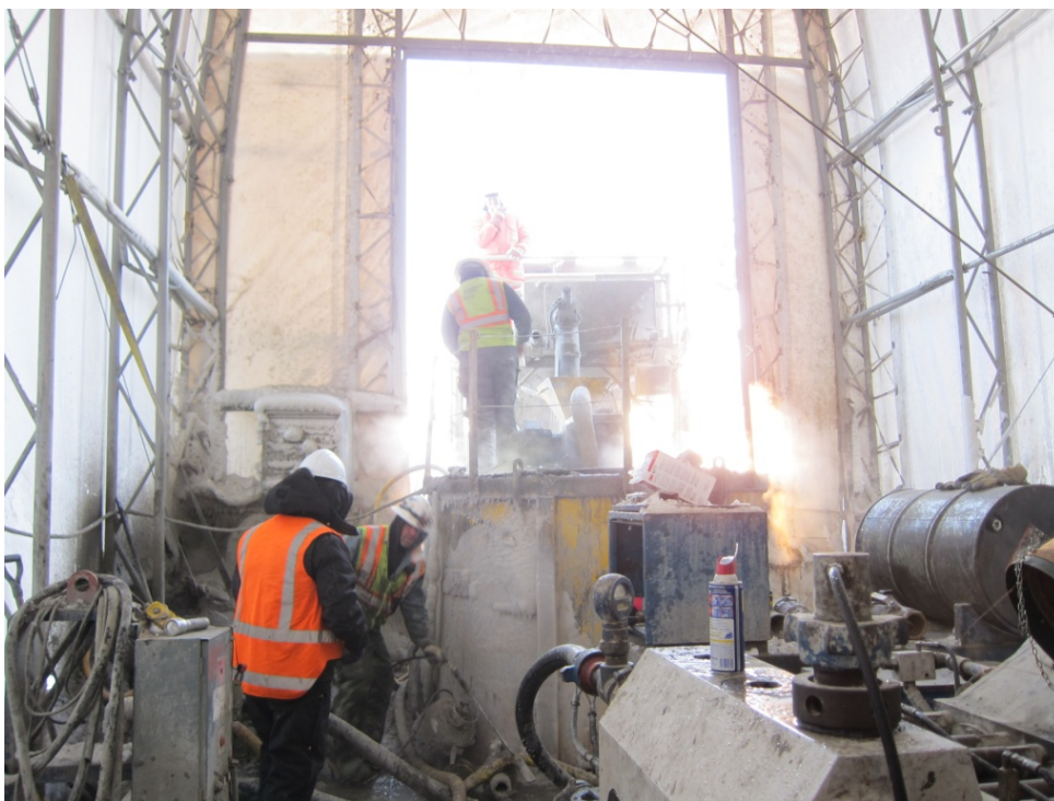
Photograph 106: Jet grouting mixing station - November 20, 2010
