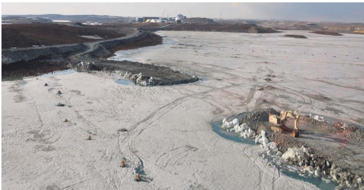
Photograph 42: Rockfill placement as part of the causeway construction at Sta. 31+950 - June 2010
