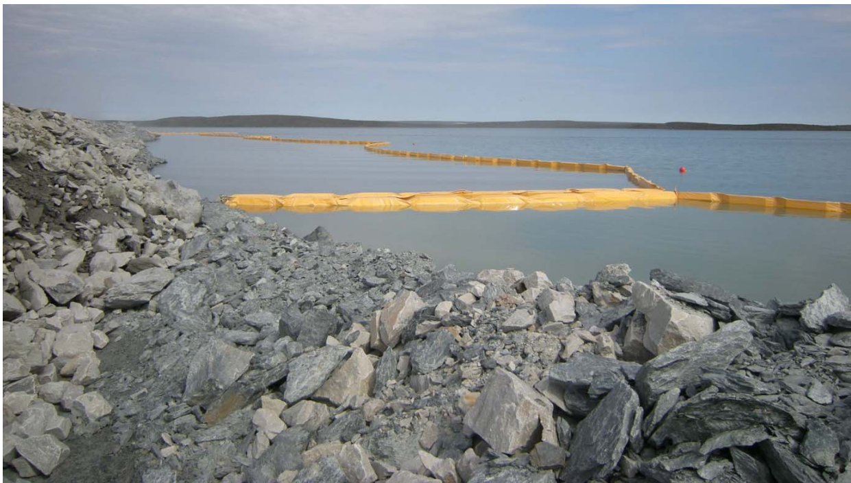
Photograph 44: Turbidity barriers on upstream side of causeway at Sta. 31+350, barriers placed as small cells and anchored to the causeway - July 23, 2010
