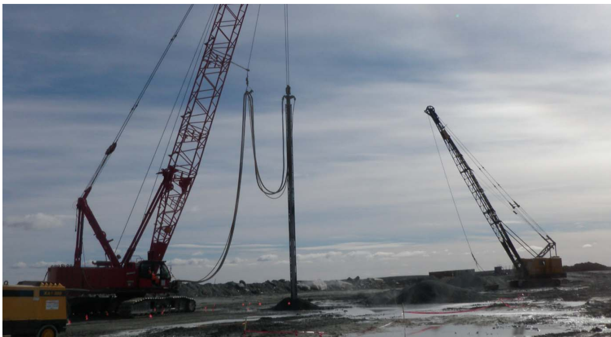
Photograph 70: Vibro-densification of core backfill - September 1, 2010
