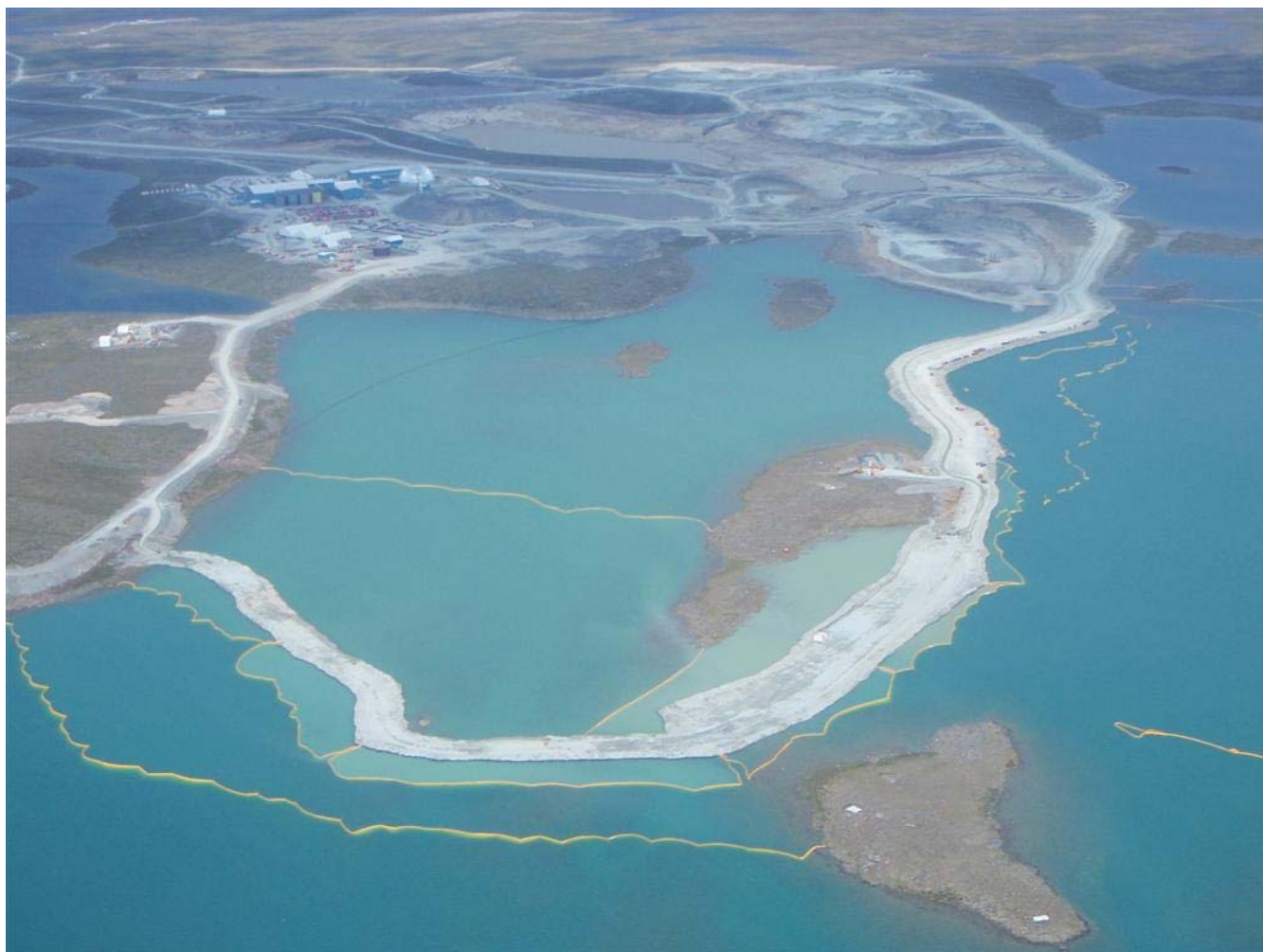
Photograph 47: Turbidity barriers and rockfill placement to widen causeway - August 2010
