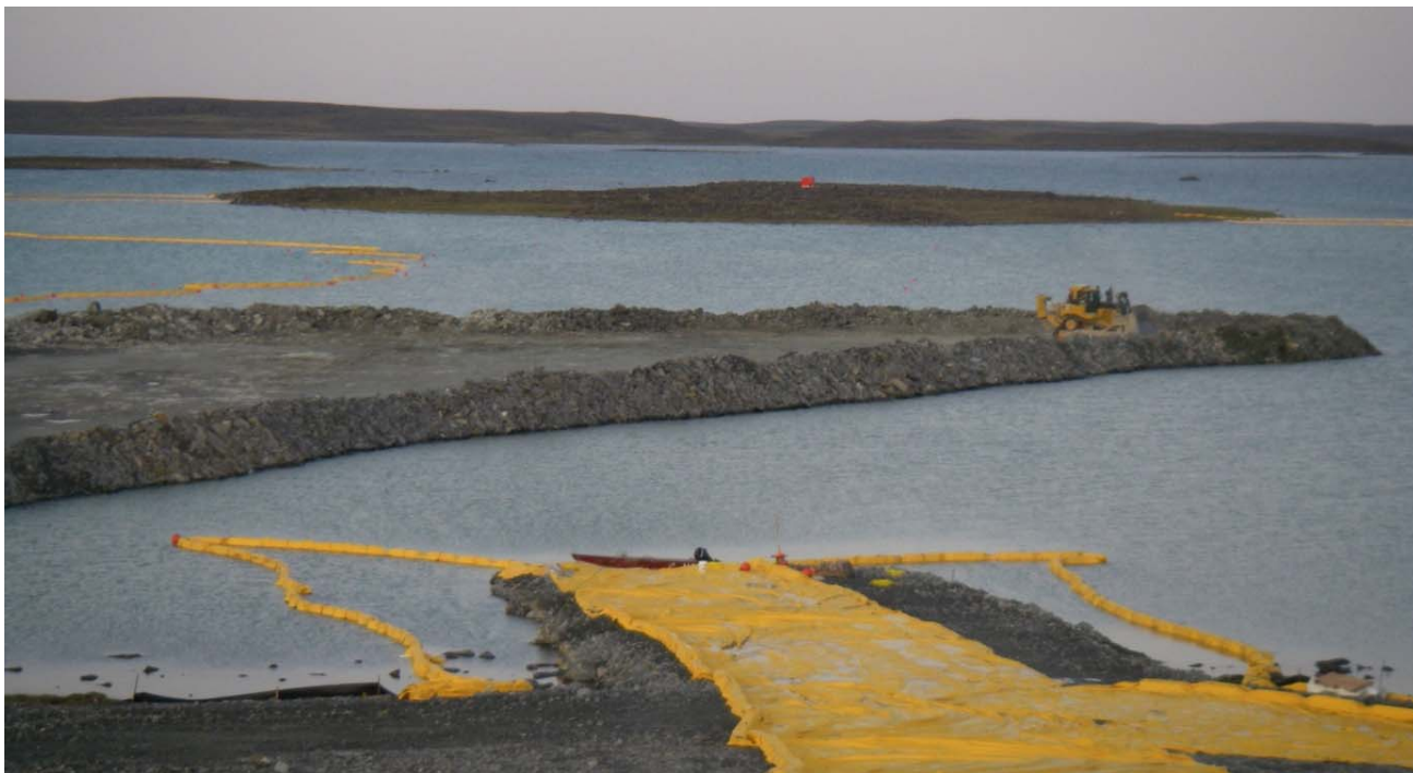
Photograph 3: Rockfill placement at approximately Sta. 30+366. Rockfill placement from the downstream (pit side) to the upstream to push lakebed sediments away from the dike centerline. Turbidity barrier installation in foreground - August 3, 2009
