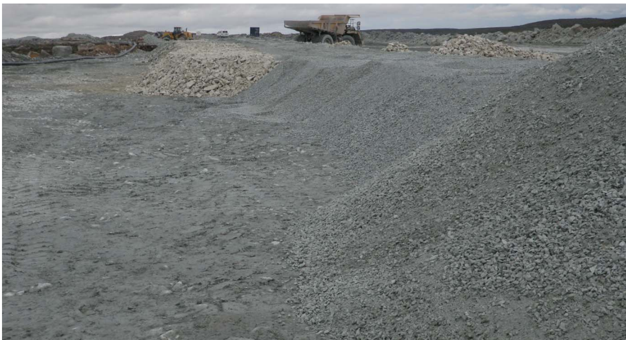
Photograph 71: Downstream side of densification platform at Sta. 31+100. Core backfill and coarse filter downstream wing - August 2, 2010
