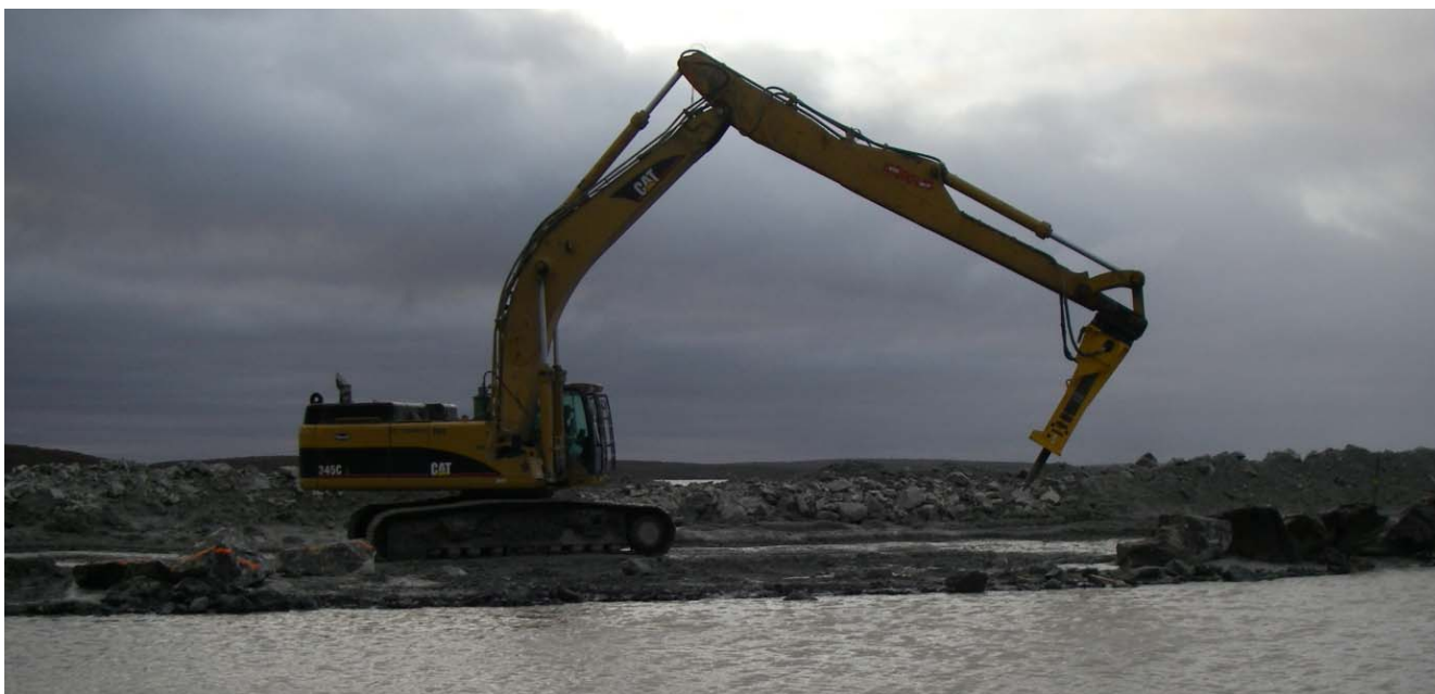
Photograph 13: CAT 345 excavator with long boom and breaker attachment used to smooth bedrock surface where irregularities were noted - September 6, 2009
