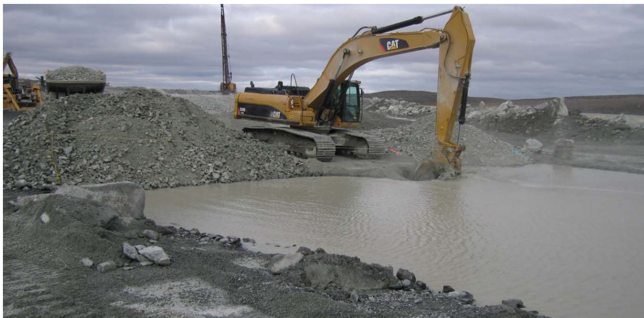
Photograph 18: Placement of the Core Backfill material by pushing the Core Backfill forward and down to minimize segregation, Sta. 30+500 - September 5, 2010
