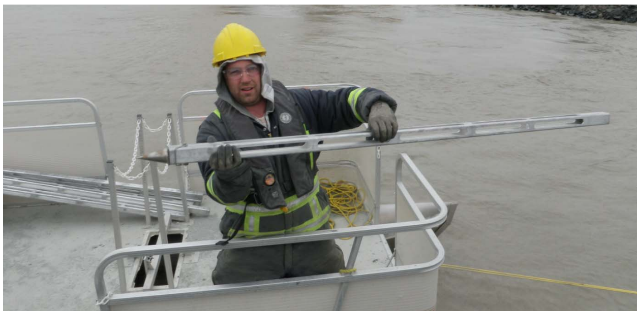
Photograph 59: Sample showing one of the rods used to survey base of initial trench excavation – August 16, 2010
