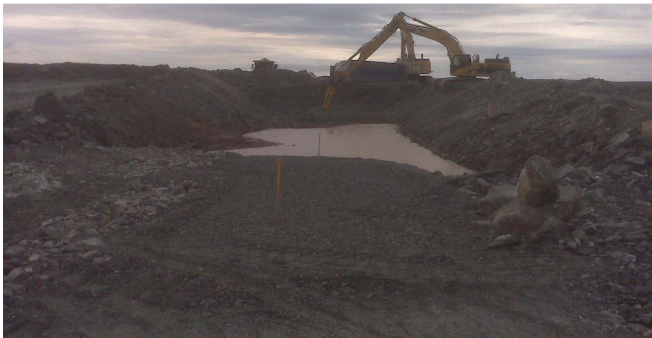
Photograph 57: Excavation of rockfill and frozen core backfill at tie-in of the north portion of the cutoff wall to the south portion, Sta. 30+850 - August 12, 2010
