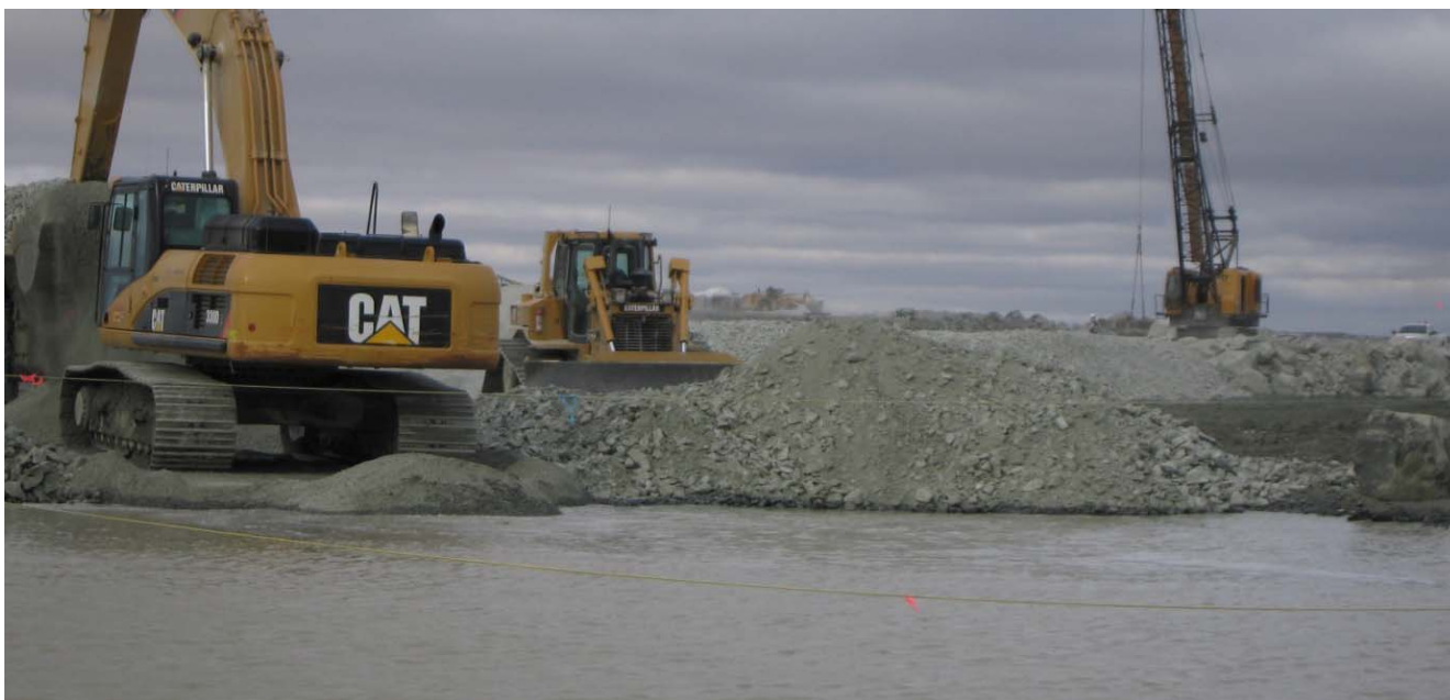
Photograph 19: Placement of the Coarse Filter upstream of Core Backfill by pushing forward with a dozer onto already placed material to minimize segregation, Sta. 30+500 - September 5, 2009
