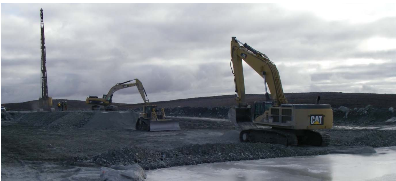
Photograph 24: Dynamic compaction and construction of the densification platform in the background and placement of Core Backfill and Coarse Filter within the initial trench excavation in the foreground, looking north from Sta. 30+450 - September 4, 2009
