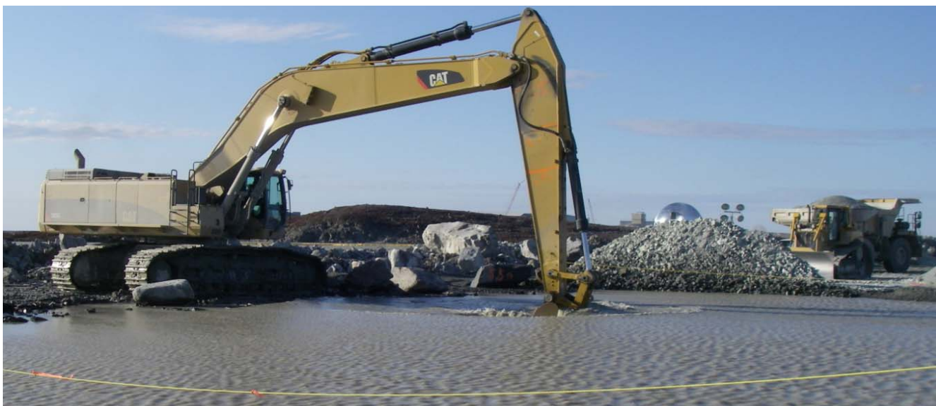
Photograph 20: Placement of Core Backfill on the downstream side of the initial trench excavation up to the level of the lakebed sediments, Sta. 30+550 - September 6, 2009
