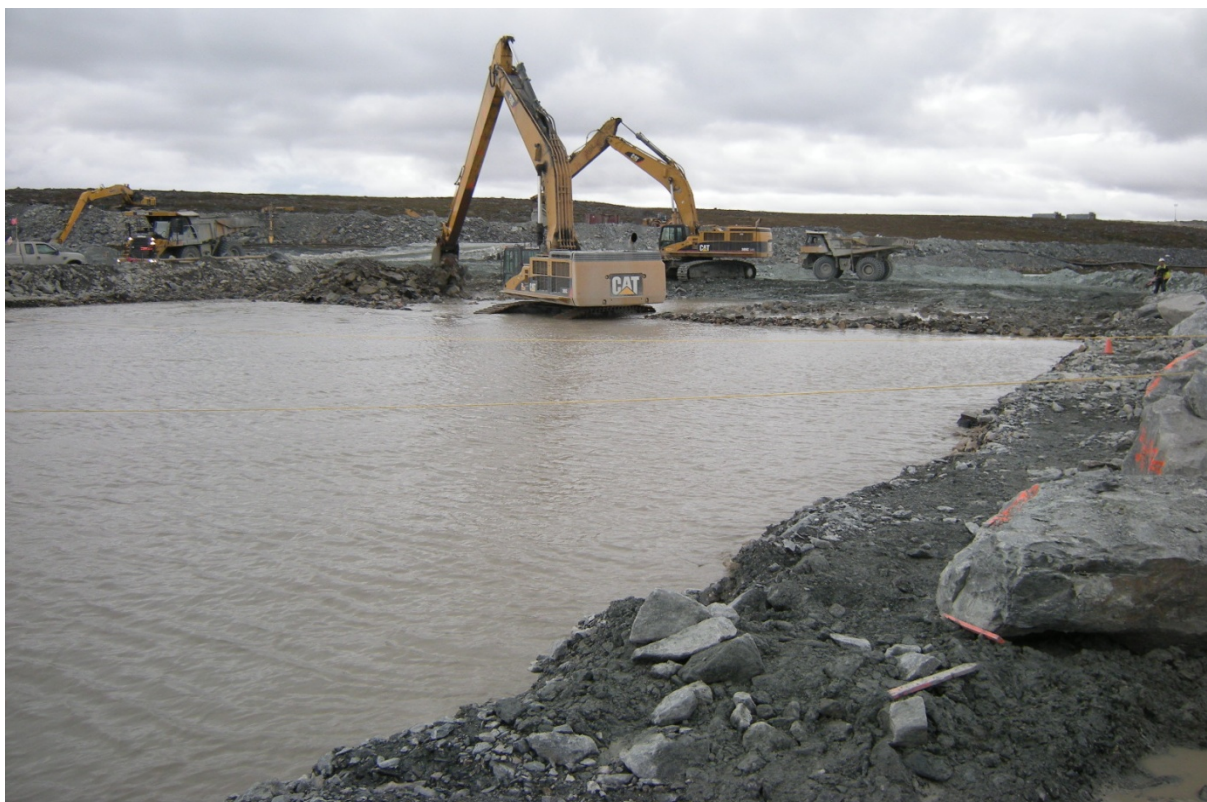
Photograph 60: Initial trench excavation, Sta. 32+007 - August 25, 2010
