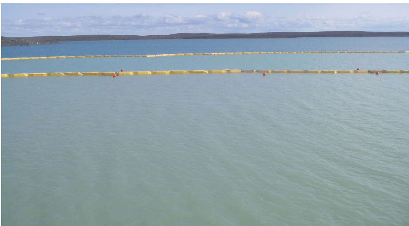
Photograph 2: Double line of turbidity barriers evident within Third Portage Lake, beyond the northern portion of the dike - August 6, 2010
