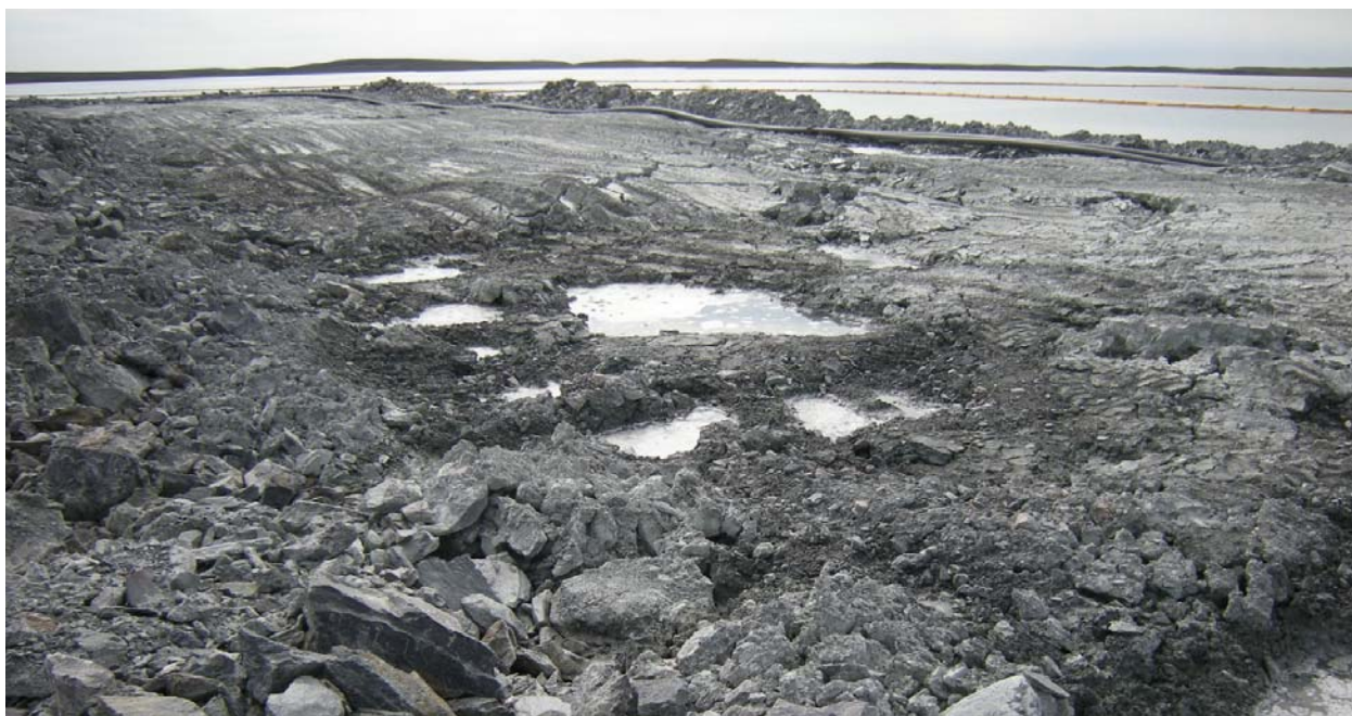
Photograph 43: Depression observed on causeway surface at Sta. 31+680, due to thawing of ice trapped in rockfill during winter causeway construction – July 23, 2010
