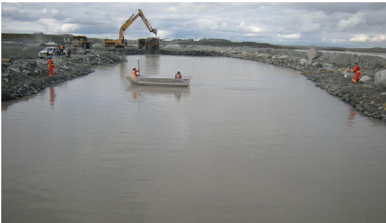
Photograph 55: Manual sounding and centreline marking in preparation for core backfill placement, Sta. 31+680 - August 3, 2010
