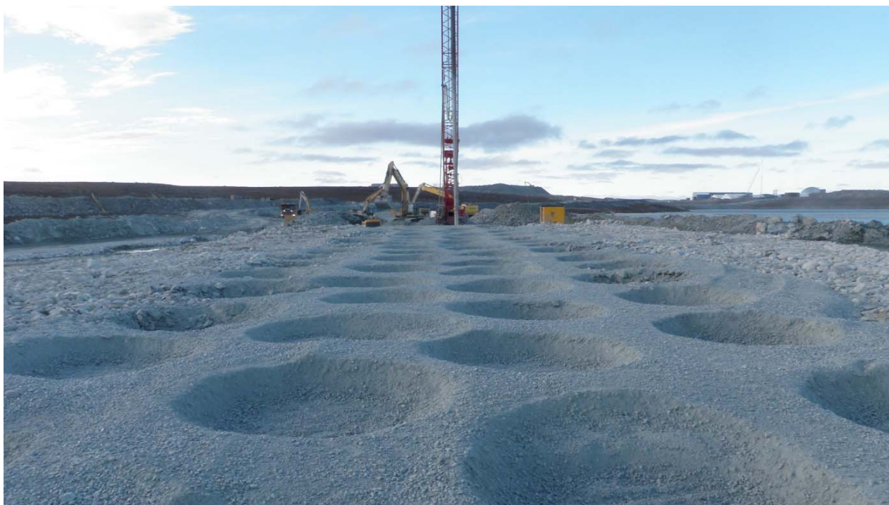
Photograph 76: Craters formed within the central core backfill zone following dynamic compaction, Sta. 31+841 to 31+930 - September 7, 2010
