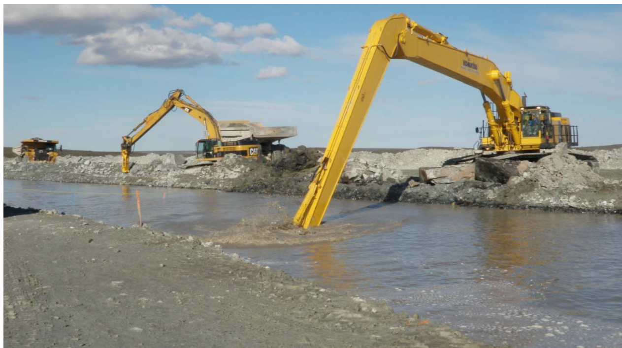
Photograph 53: Komatsu 1250 excavator removing loose material after CAT 385 excavator with breaker attachment shaped bedrock surface at Sta. 31+348 - August 1, 2010
