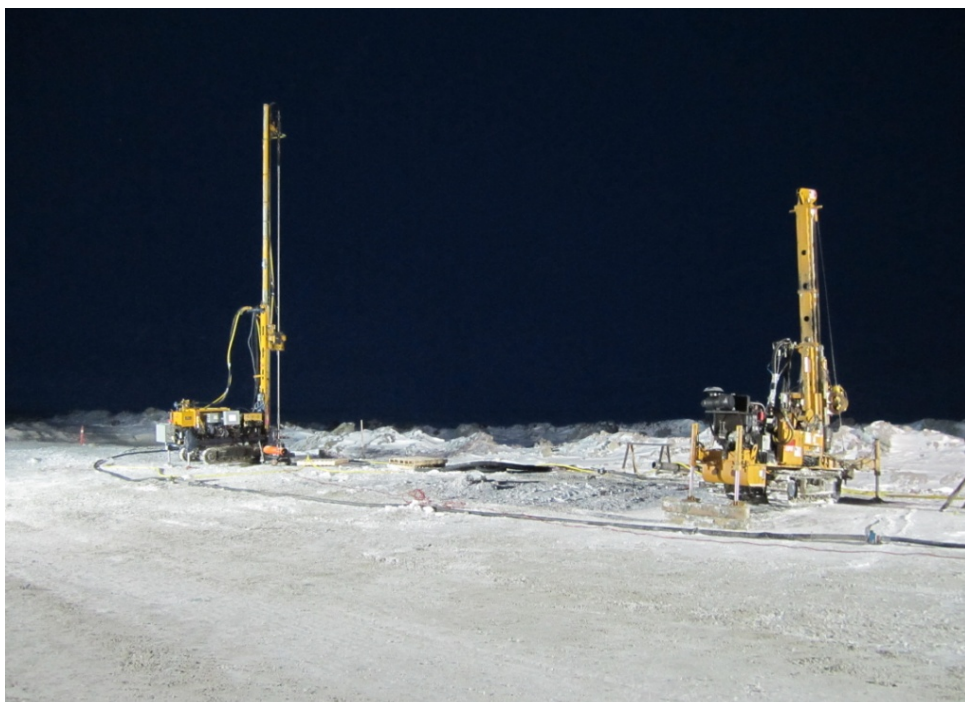
Photograph 110: Jet grouting early stages with two rig operation / pre-drilling - November 5, 2010
