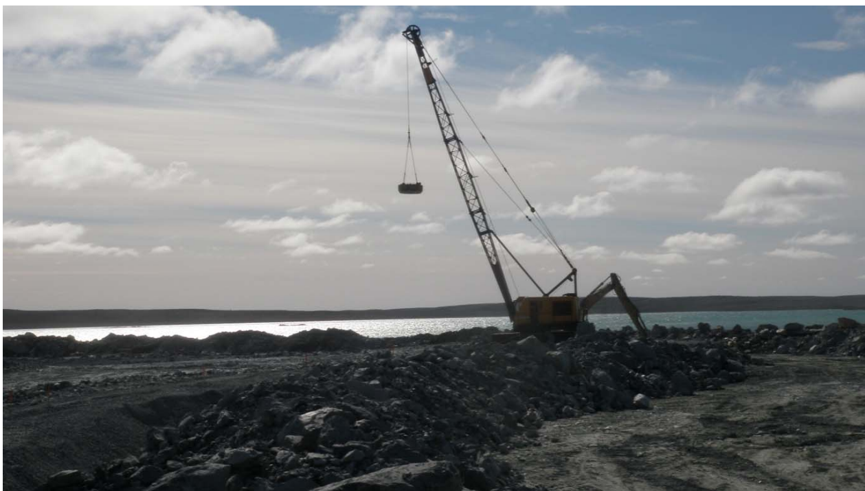
Photograph 73: Dynamic compaction of core backfill at Sta. 31+650 - August 15, 2009
