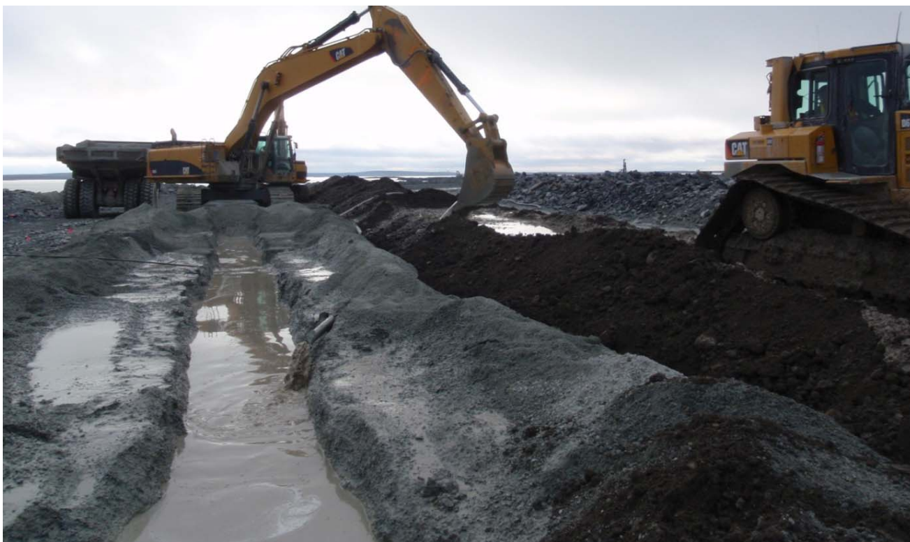
Photograph 27: Bentonite slurry is pumped into the cutoff trench excavation to provide trench support through the pipe visible in the foreground, Sta. 30+075. The excavator takes slurry from the trench to mix with the till and bentonite stockpile adjacent to the trench. The dozer is then used to mix the till to create the soil bentonite (SB) for placement in the trench - September 12, 2009
