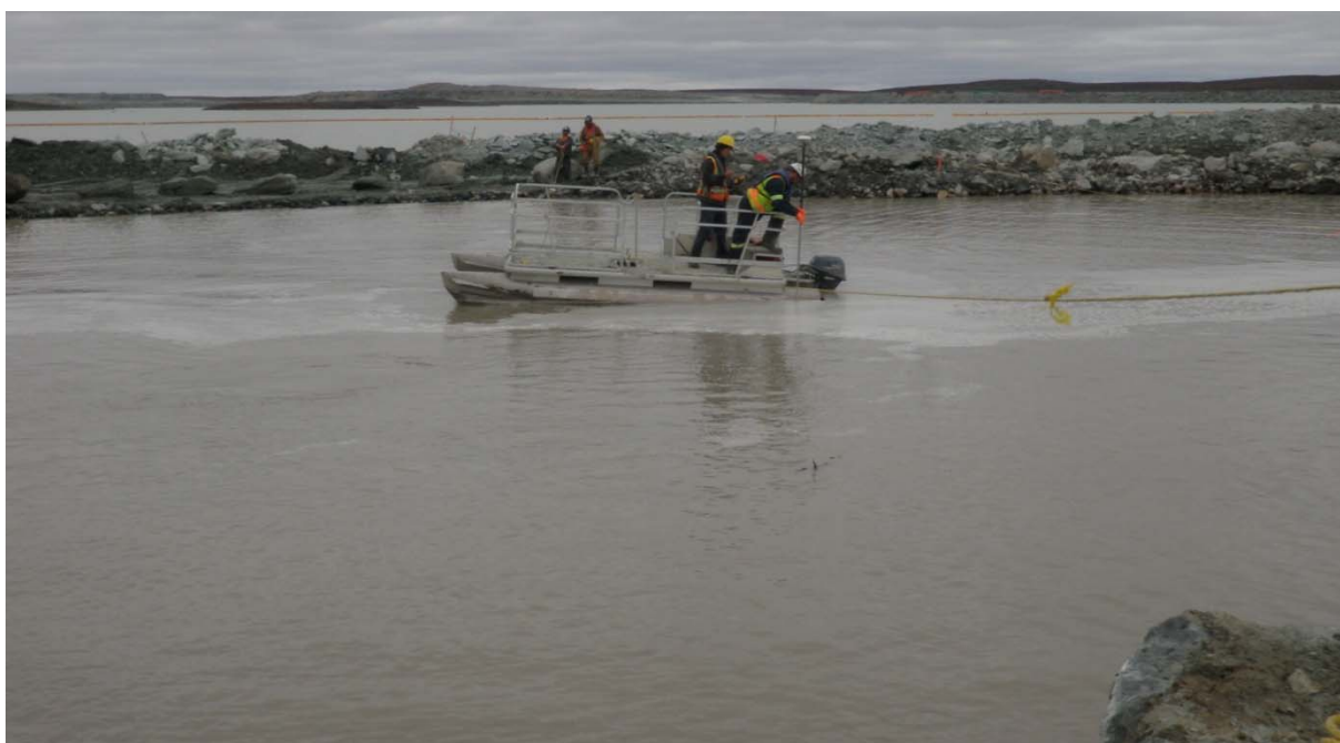
Photograph 61: Manual sounding of trench excavation, Sta. 32+050 - September 11, 2010
