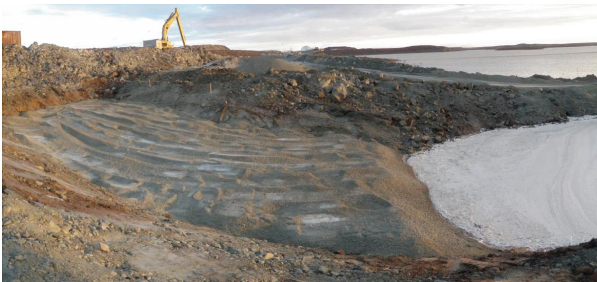
Photograph 87: Core backfill placement on top of ice-rich material at the south abutment, Sta. 32+140 to 32+166 - September 15, 2010
