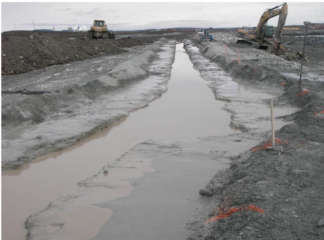
Photograph 35: Cutoff trench excavation widened at the bends, Sta. 30+725 - September 24, 2009
