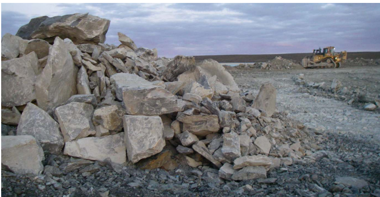
Photograph 4: Oversize rockfill is being placed on the sides of the dike platform – August 4, 2009
