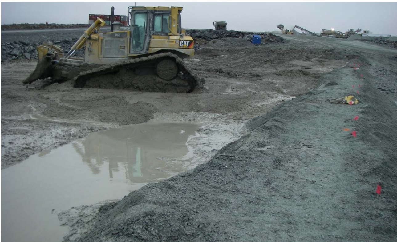
Photograph 30: Placement of the soil bentonite mix within the cutoff trench by a dozer, Sta. 30+106 - September 14, 2009
