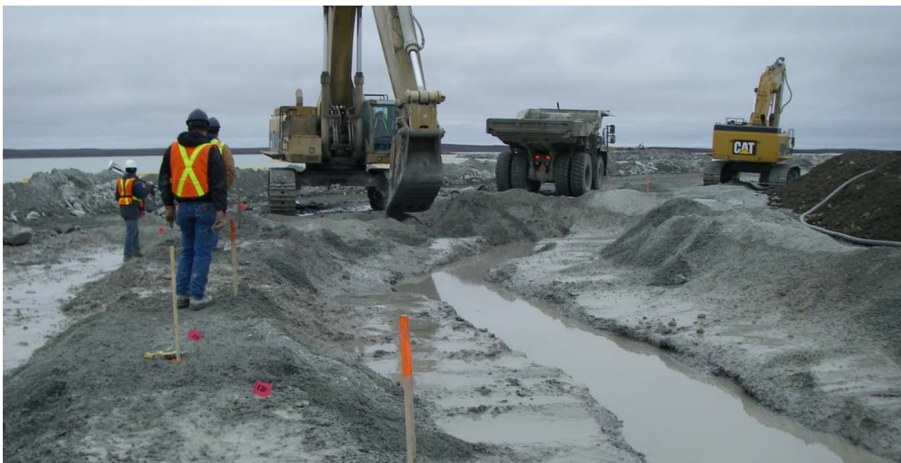
Photograph 29: Excavation of the cutoff trench and widening at the bends, Sta. 30+140 - September 13, 2009
