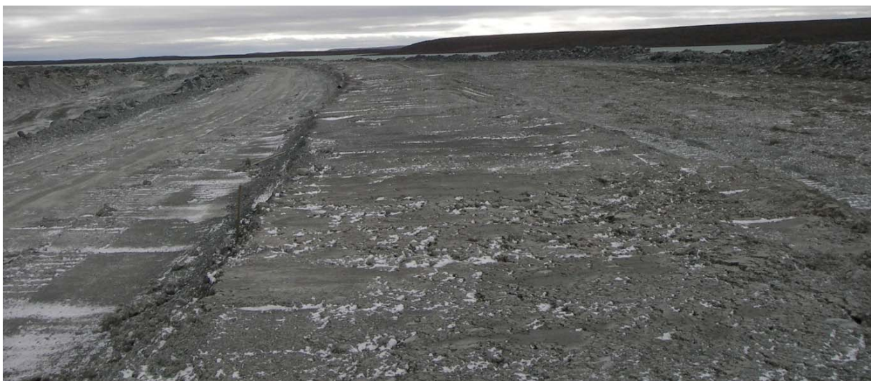
Photograph 36: Completed surface of cutoff trench - September 27, 2009
