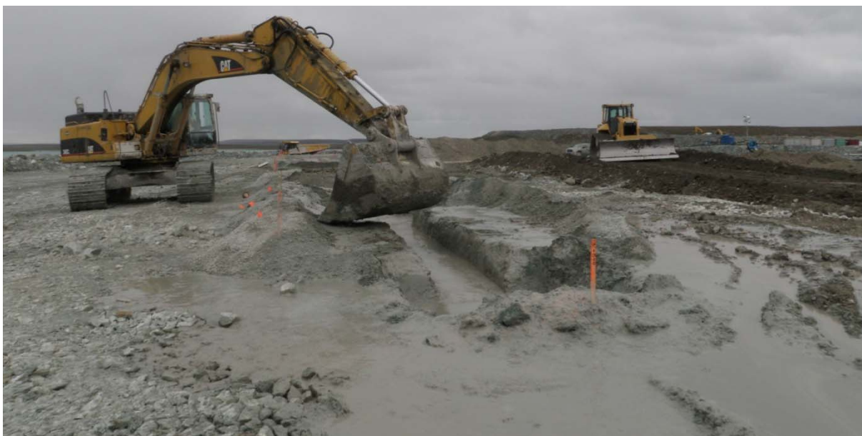
Photograph 79: CSB plug between Sta. 31+552 and 31+570. Dozer spreading till mixed with dry bentonite for SB preparation - August 25, 2010
