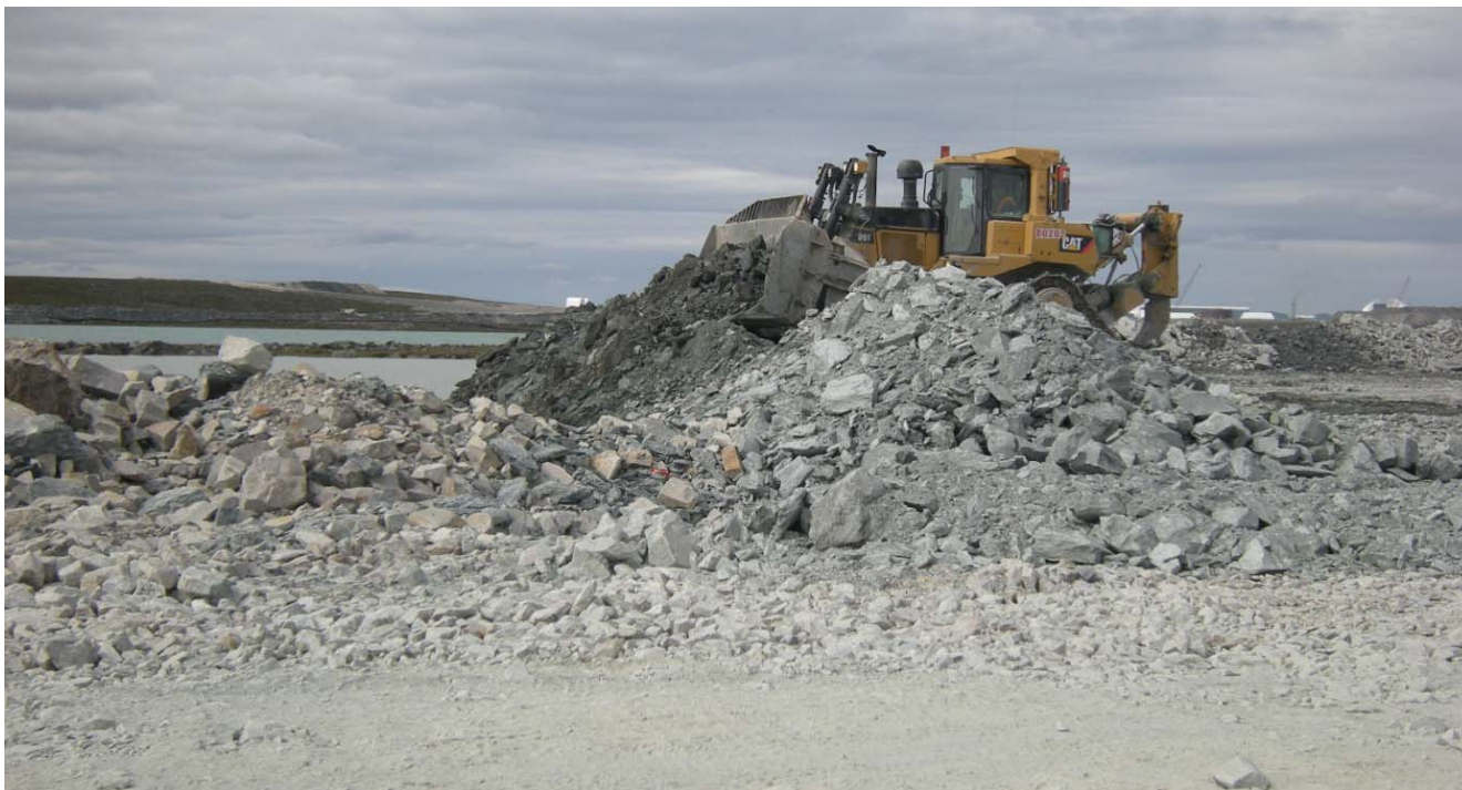
Photograph 48: Rockfill placement to widen causeway at Sta. 31+200 - July 22, 2010
