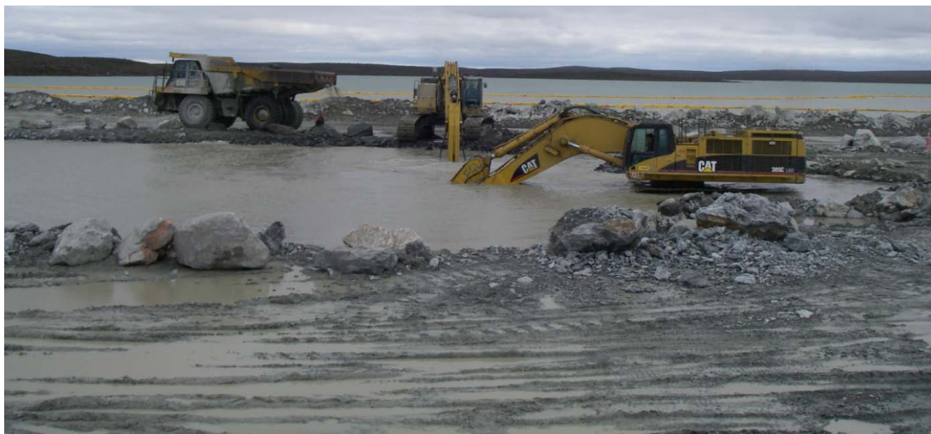
Photograph 7: Initial trench excavation at Sta. 30+400, excavation was at a depth of 10 m, excavator was sitting on a lower bench - August 20, 2009
