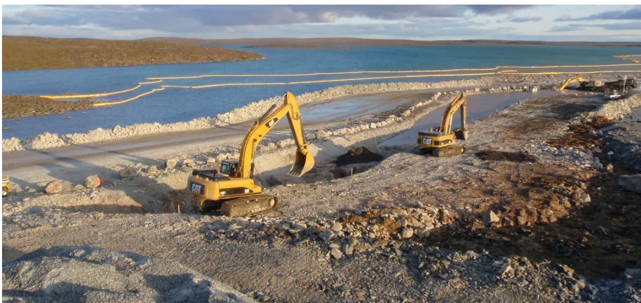
Photograph 38: Abutment excavation and initial trench excavation up to Sta. 30+190 - August 13, 2009
