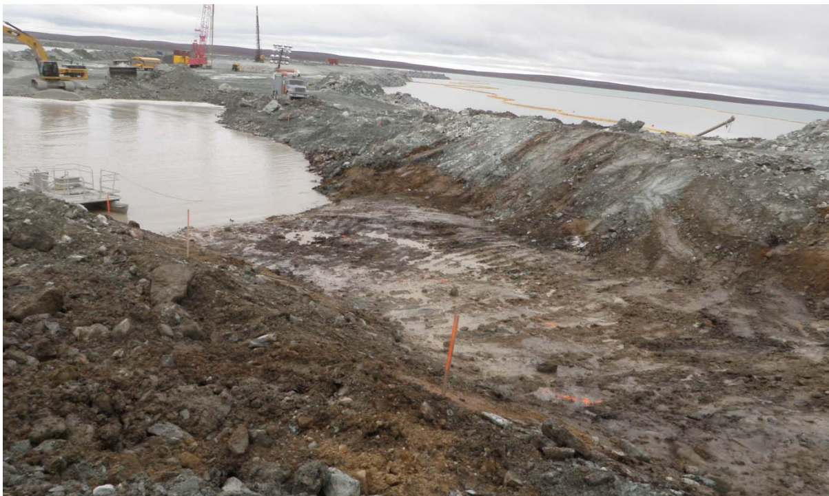
Photograph 86: South abutment foundation preparation. Ice rich material was left in place between Sta. 32+125 and 32+166 due to schedule constraints - September 14, 2010
