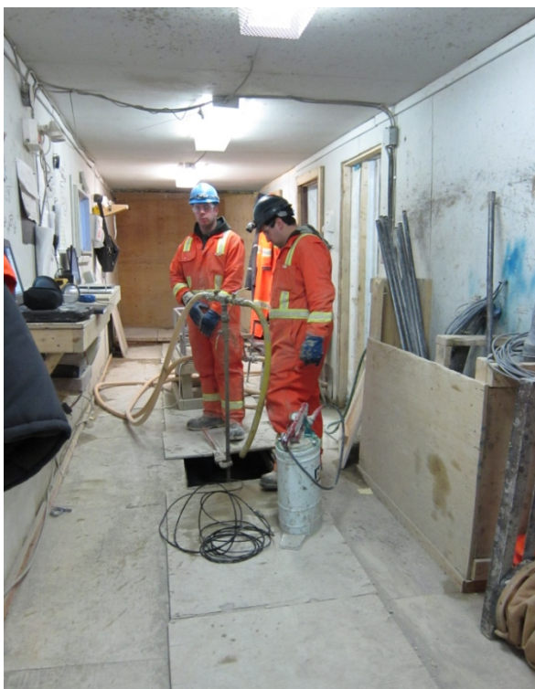
Photograph 103: Mobile grouting plant, injection side with removable floor - November 27, 2010
