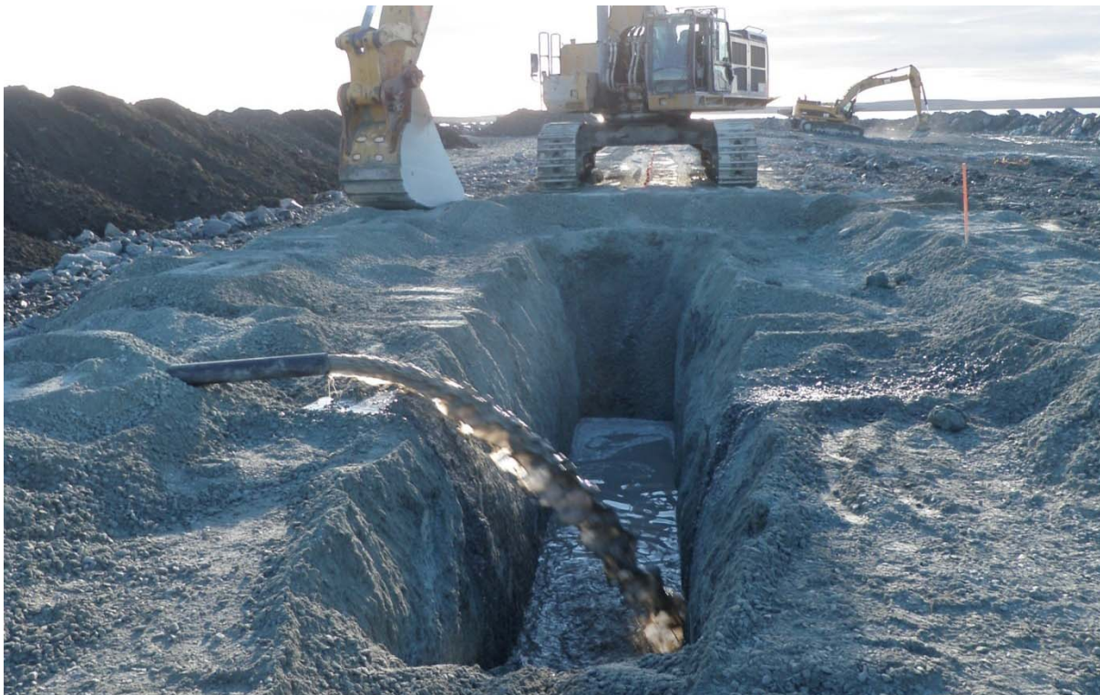
Photograph 78: Cutoff trench excavation and bentonite slurry placement – August 23, 2010
