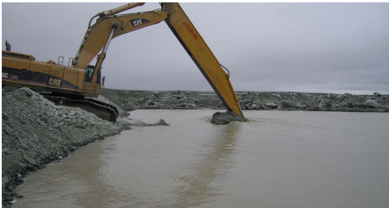
Photograph 17: Sediment at the bottom of the trench excavated prior to Core Backfill and Coarse Filter placement at Sta. 30+450 - September 3, 2009
