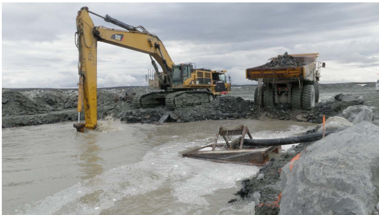
Photograph 52: Initial trench excavation with CAT 385 excavator at Sta.31+330. Pump installed on downstream side of trench – July 31, 2010
