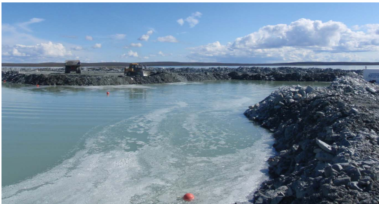
Photograph 50: Rockfill placement at Sta. 31+580 to connect to rockfill placement front 2 - August 1, 2010
