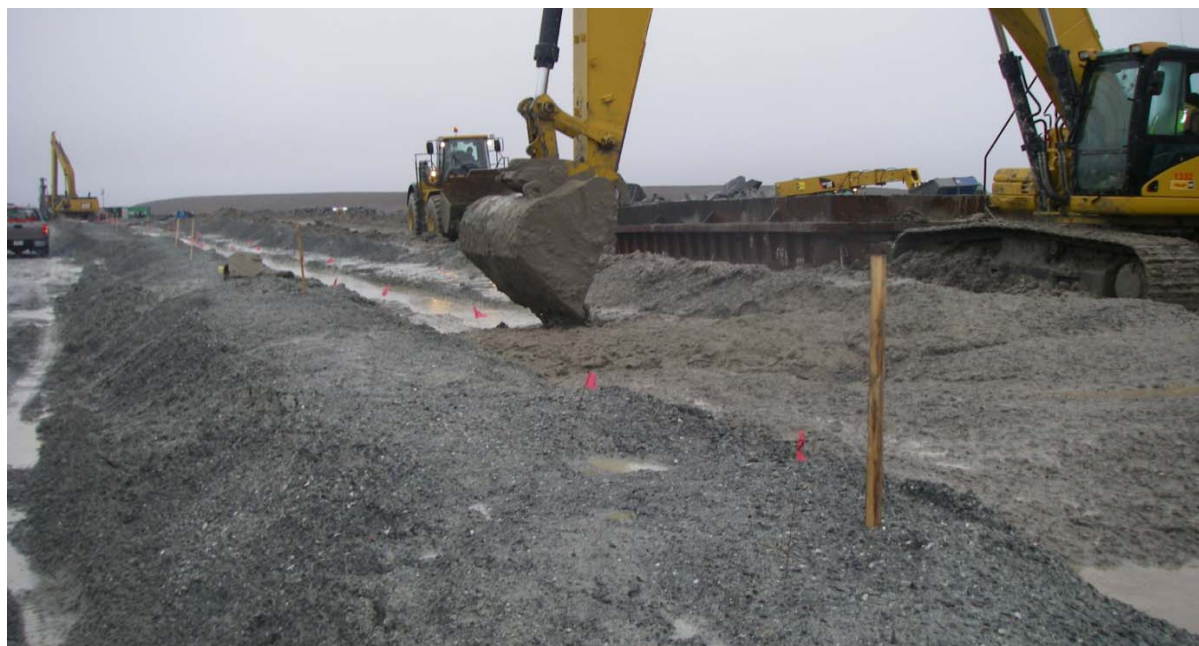
Photograph 31: Placement of cement soil bentonite mix within the cutoff trench. The cement soil bentonite (CSB) mixed on site within the box visible in front of the excavator - September 18, 2009
