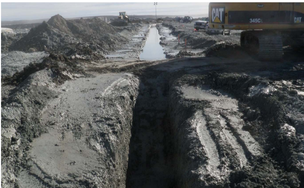
Photograph 83: From top to bottom: Cutoff trench with bentonite slurry, CSB plug at Sta. 31+806 and cutoff wall excavation – September 7, 2010
