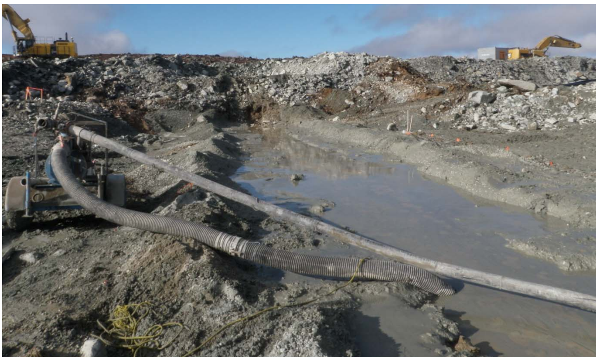
Photograph 88: Cutoff trench at south abutment, Sta. 30+140 - September 23, 2009
