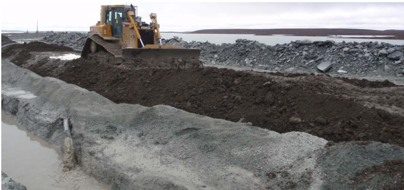
Photograph 28: The dry till and bentonite mixed with the bentonite slurry by a dozer to form the soil bentonite mix, Sta. 30+075 - September 12, 2009
