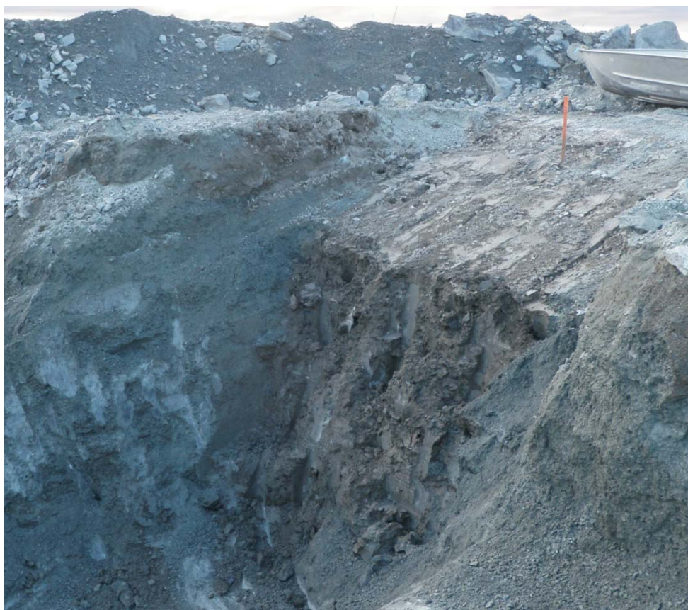
Photograph 58: Core backfill and CSB excavation at north portion tie-in, approximately Sta. 30+860 - August 12, 2010
