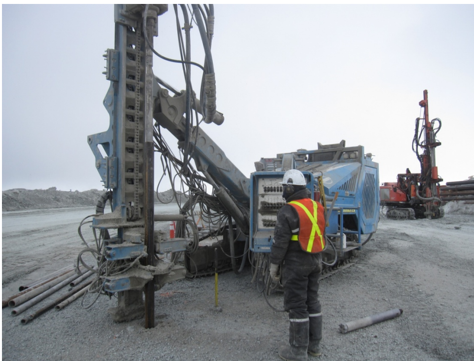
Photograph 99: Casing installation - April 2010
