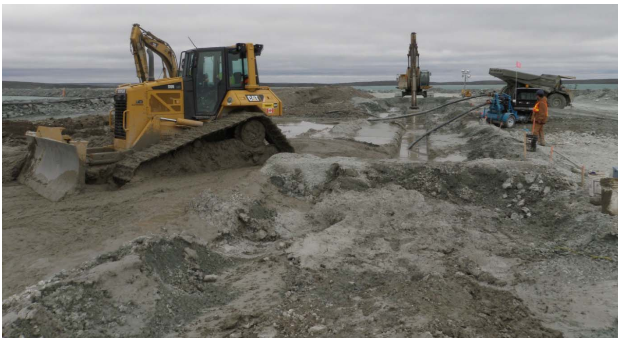
Photograph 80: SB placement into cutoff wall with dozer - August 26, 2010
