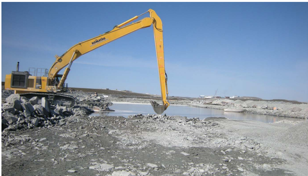
Photograph 56: Komatsu 1250 excavator removing sediments prior to core backfilling of initial trench - August 7, 2010
