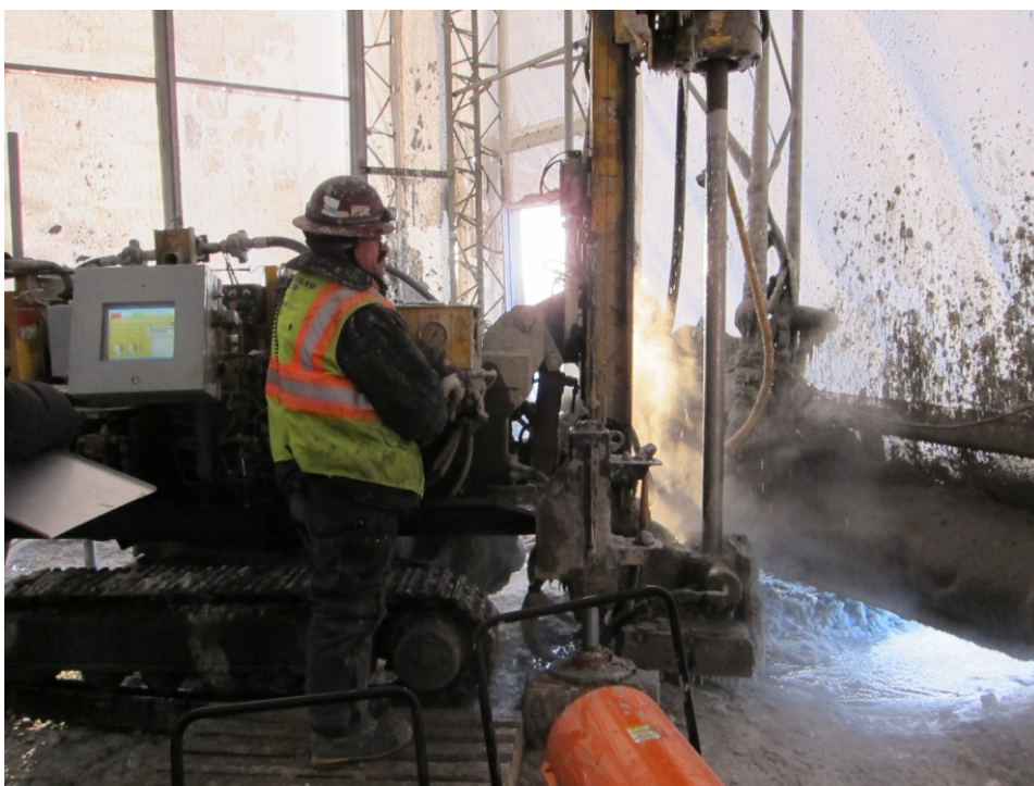
Photograph 111: Jet grouting single rig operation within coverall tent - November 20, 2010
