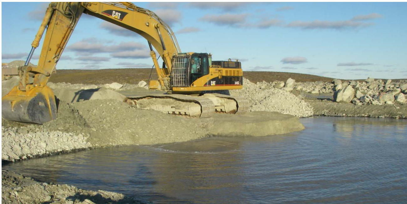
Photograph 15: Core Backfill and Coarse Filter placement at Sta. 30+310 - August 22, 2009
