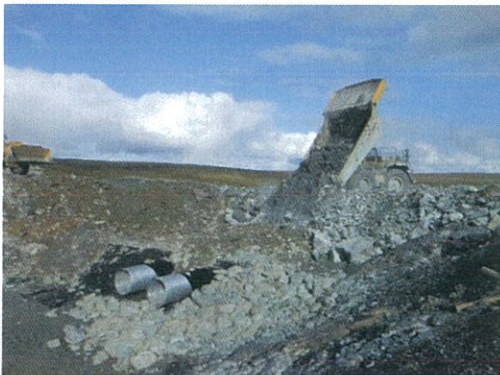
(08-15-2012) Rockfill over VR Culvert
