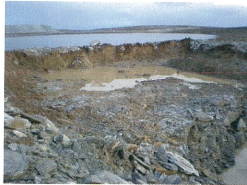
(08-26-2012) NP1 - 1st Breach 2
