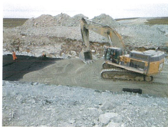
(08-10-2012) Culvert Vault Road 0-3/4
