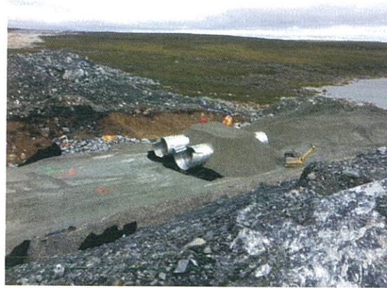
(08-11-2012) Culvert Vault Road 1st sheets
