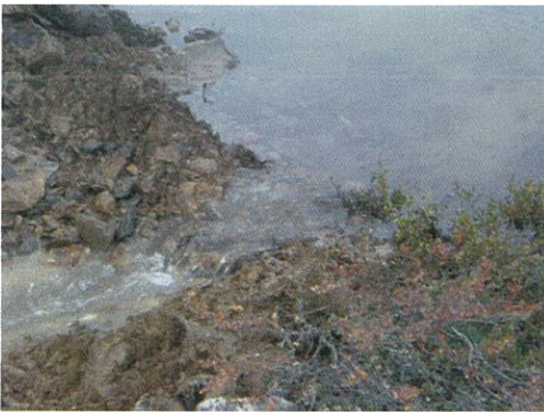
(08-26-2012) NP1 - 1st Breach 6
