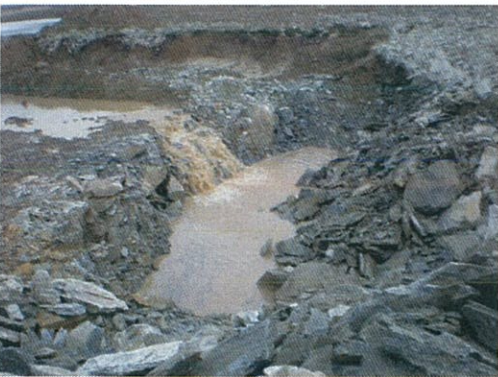
(08-26-2012) NP1 - 1st Breach 7
