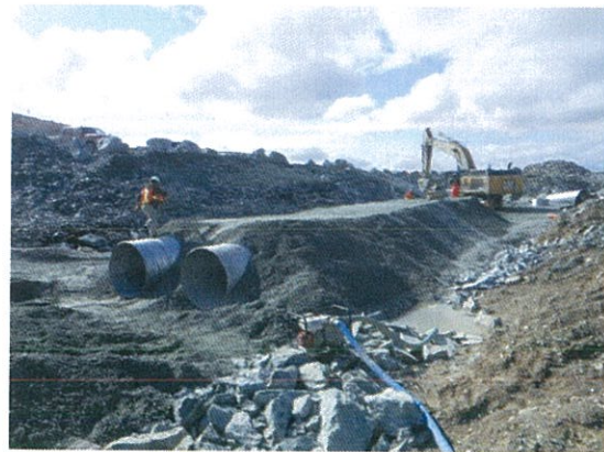
(08-12-2012) Culvert Vault Road Compaction
