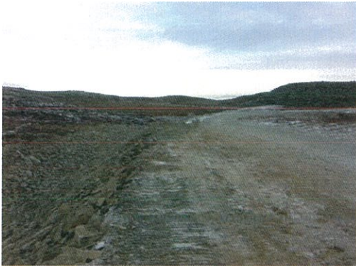
(10-09-2012)WD Dam – Access Road
