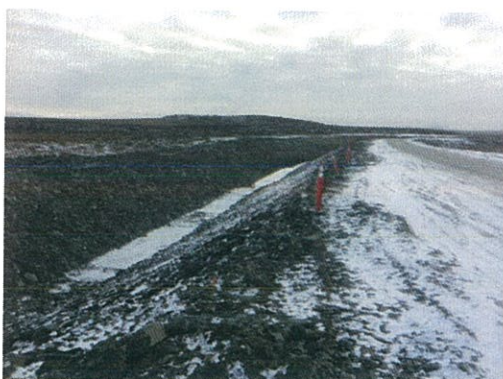
(10-09-2012)ED - Completed Ditches 2
