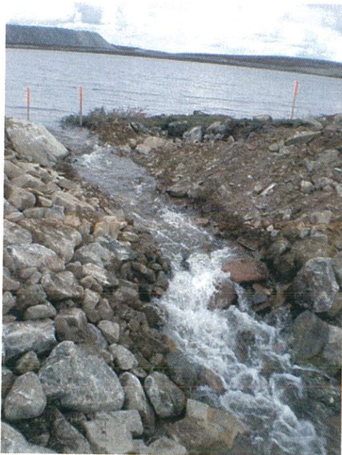
(08-26-2012) NP1 - 1st Breach 12
