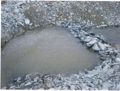
(09-17-2012)NP1 – 3rd Breach 5
