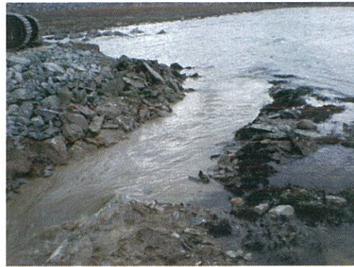
(09-17-2012)NP1 – 3rd Breach 2
