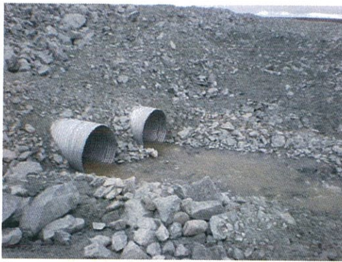
(09-17-2012)NP1 – 3rd Breach 6
