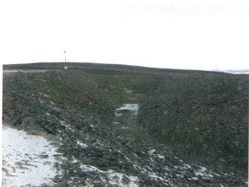
(10-09-2012)ED - Completed Ditches 1
