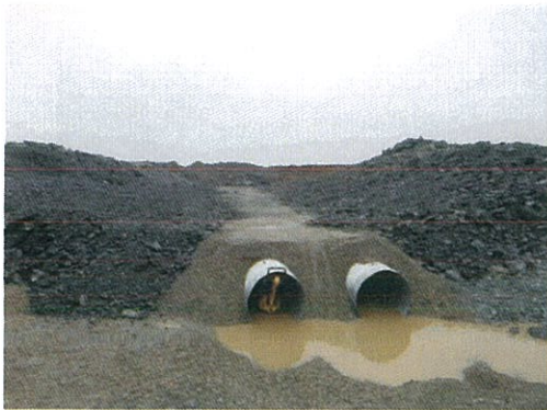
(08-14-2012) Rockfill over VR Culvert
