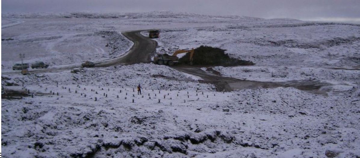
Preparing to blast ice-rich material and excavating blasted material
