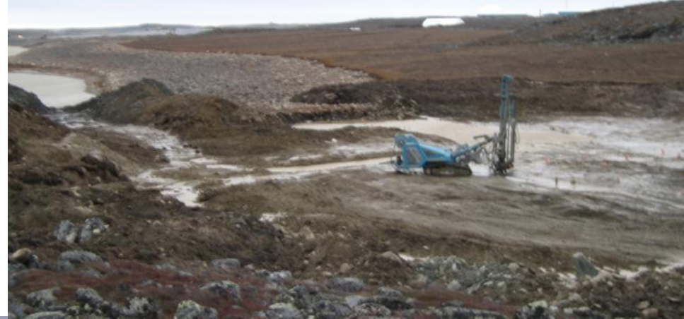
Preparing to blast ice-rich material and excavating blasted material
