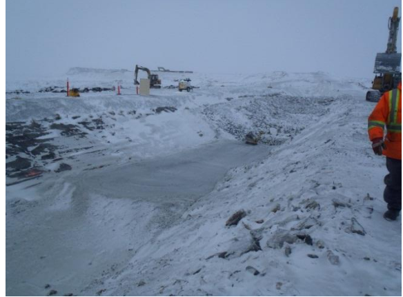
(Mar 6 2013) Fine filter with bentonite placed above geomembrane and compacted
