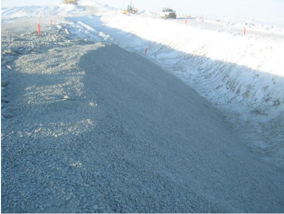
(Feb 13 2013) Compacted fine filter layer
