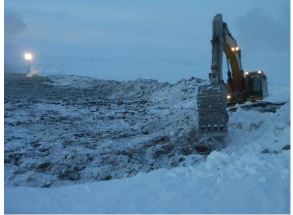
(Feb 5 2013) Snow, ice, overburden, and boulder removal
