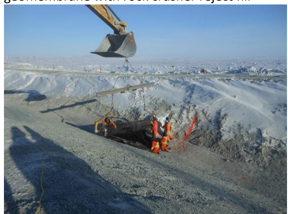
(Feb 28 2013) First attempt to roll out the Teranap geomembrane
