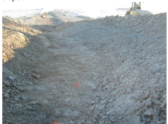
(Feb 9 2013) Placement of coarse filter over rockfill key trench slope
