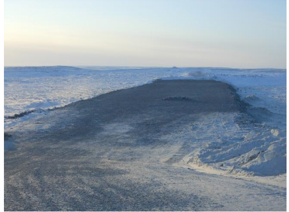
(Mar 21 2013) Vault Dike before addition of berms and thermistor installation
