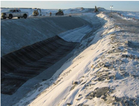
(Mar 3 2013) Coletanche geomembrane placement successful
