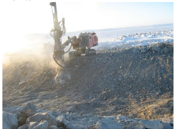
(Feb 9 2013) Drilling boulder to smooth out slope
