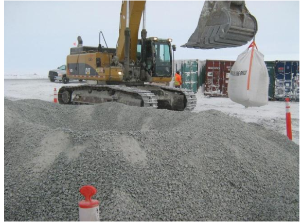
(Feb 10 2013) Mixing bentonite with fine filter for compaction tests
