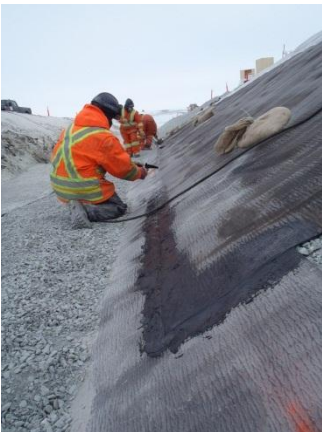
(Mar 4 2013) Horizontal geomembrane welding
