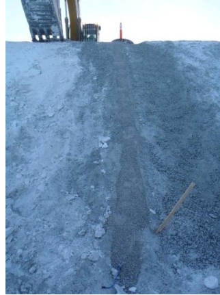
(Feb 26 2013) Thermistor TH5 installed before geomembrane with rock crusher reject fill
