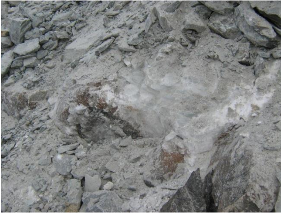
(Feb 10 2013) Ice found in till slope after blasting
