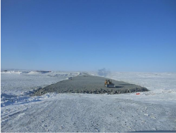
(Mar 20 2013) Adding rockfill to the top of Vault Dike
