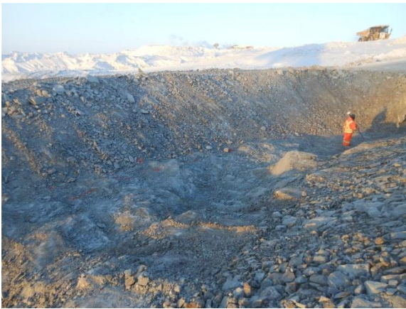
(Feb 9 2013) Key trench after blasting, excavation and grading
