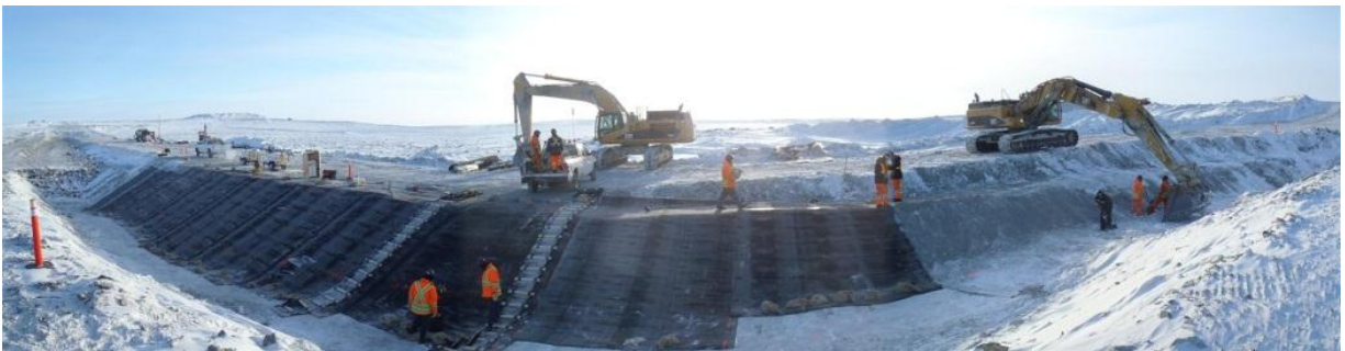
(Mar 10 2013) Vault Dike general overview during geomembrane placement
