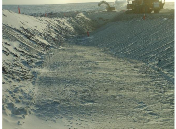
(Feb 13 2013) Complete fine filter with bentonite layer in key trench
