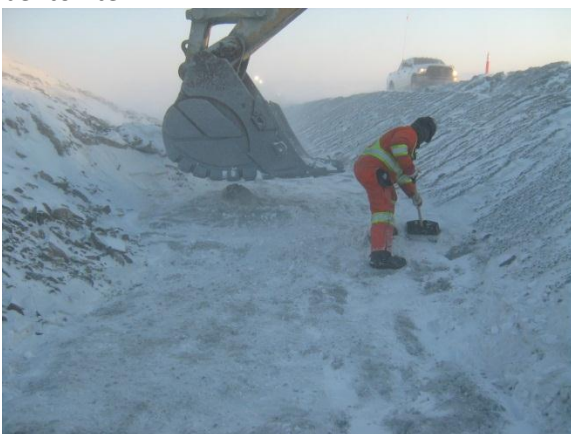
(Feb 12 2013) Snow cleaning above fine filter and bentonite mix
