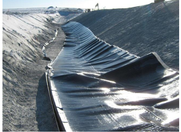
(Feb 28 2013) Ripples in Teranap geomembrane
