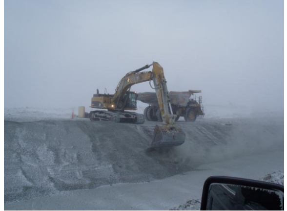
(Mar 11 2013) Fine filter placement above geomembrane
