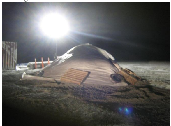
(Feb 21 2013) Bentonite and fine filter mix stockpile with cover
