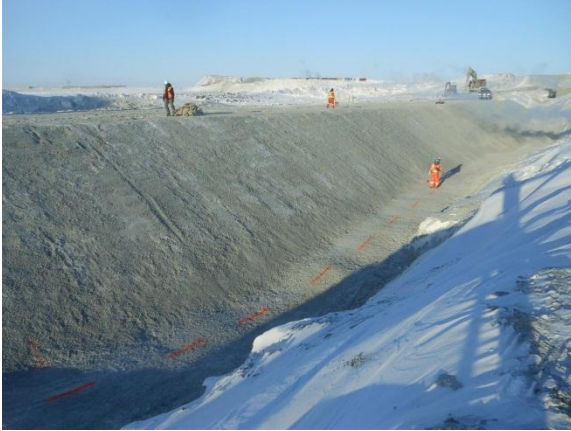
(Feb 28 2013) Line showing where the geomembrane edge should lie
