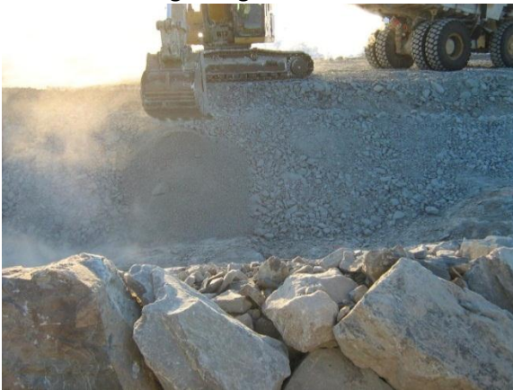
(Feb 9 2013) Placement of fine filter over coarse filter on key trench slope
