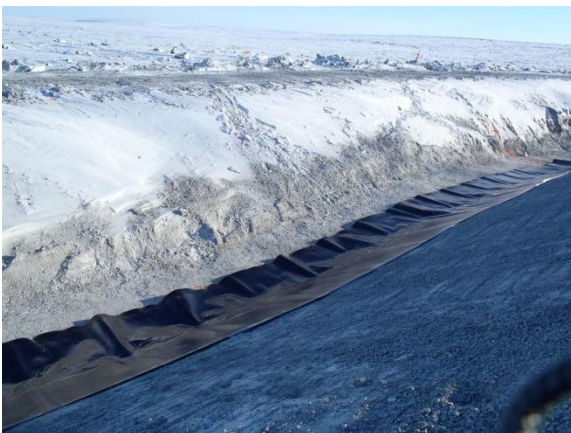
(Feb 28 2013) Geomembrane on bottom of south slope, does not lie flat and begins to crack where the slope meets the key trench floor
