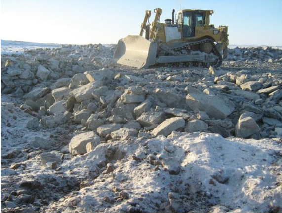
(Feb 5 2013) Rockfill placement for working platform
