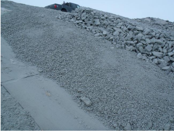
(Mar 5 2013) Fine and coarse filters above geomembrane
