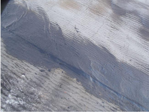
(Mar 10 2013) Vertical seams on Coletanche geomembrane
