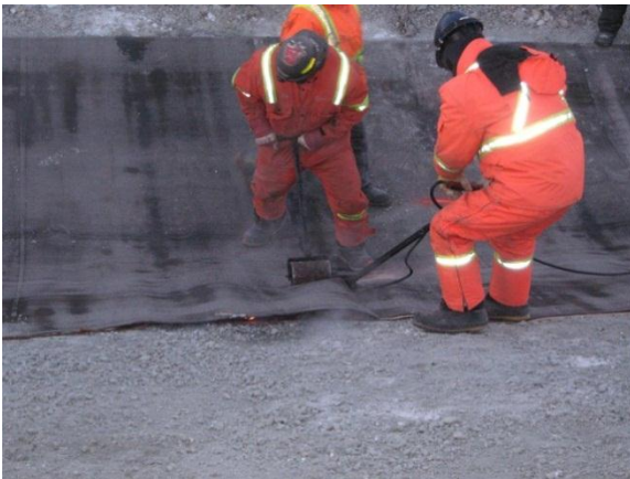
(Mar 3 2013) Welding the geomembrane
