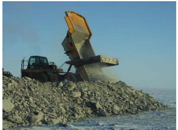
(Mar 19 2013) Placing rockfill on the top of Vault Dike
