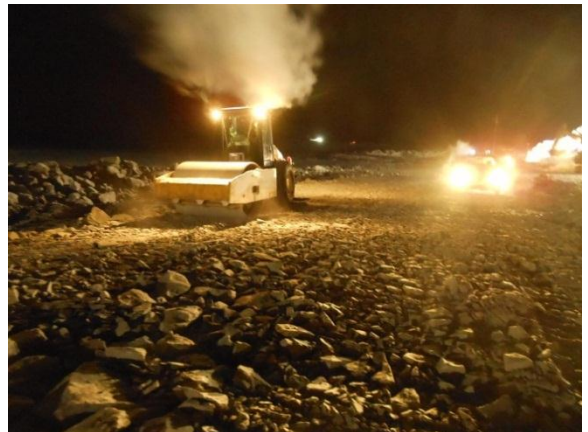
(Feb 5 2013) Compaction of working platform with vibratory roller
