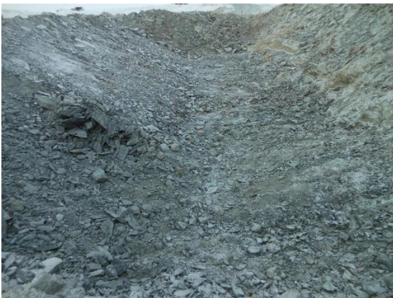
(Feb 7 2013) Key trench after blasting and excavation
