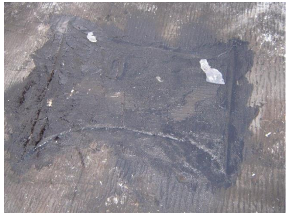
(Mar 3 2013) Patch on Coletanche geomembrane
