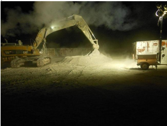
(Feb 16 2013) Bentonite and fine filter mixing
