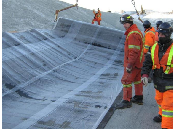
(Mar 3 2013) Rolling out the Coletanche geomembrane
