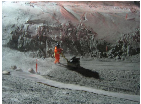
(Mar 3 2013) Compacting fine filter and bentonite layer over the geomembrane
