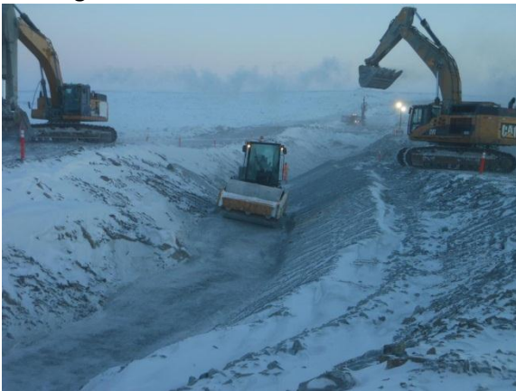
(Feb 12 2013) Compacting fine filter and bentonite mix
