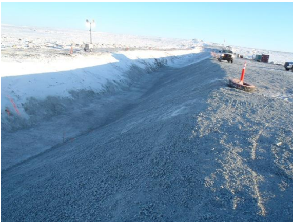
(Feb 27 2013) Key trench and slope ready for geomembrane installation
