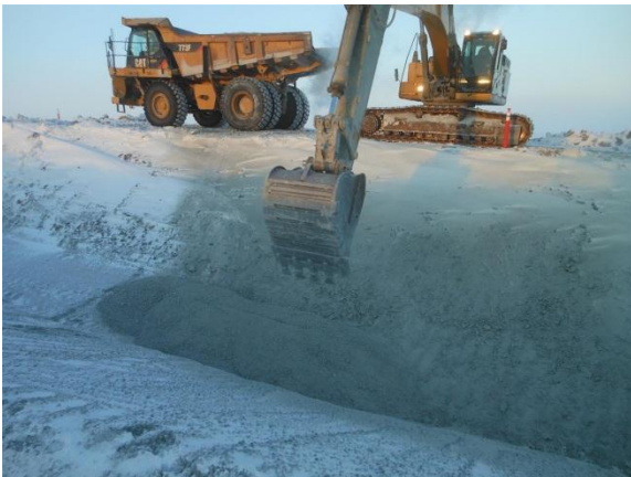
(Feb 13 2013) Fine filter with bentonite placement
