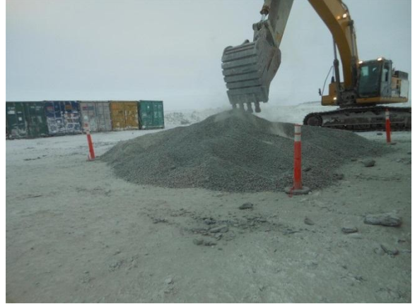
(Feb 10 2013) Gently mixing bentonite and fine filter
