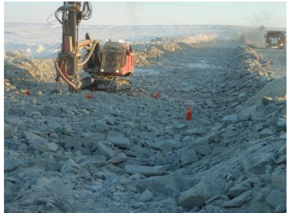
(Feb 6 2013) Drilling blast pattern
