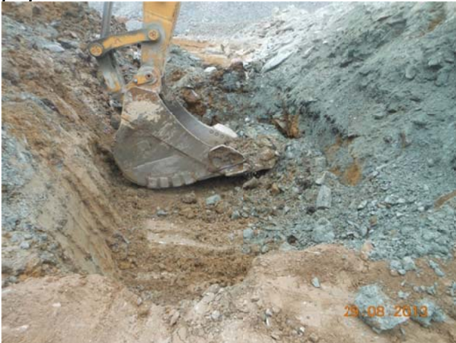
Figure 2: excavation of the foundation to permafrost / bedrock). The width of the trench at the bottom was at least one bucket wide. Note the excavated material is discarded on the upstream side.
