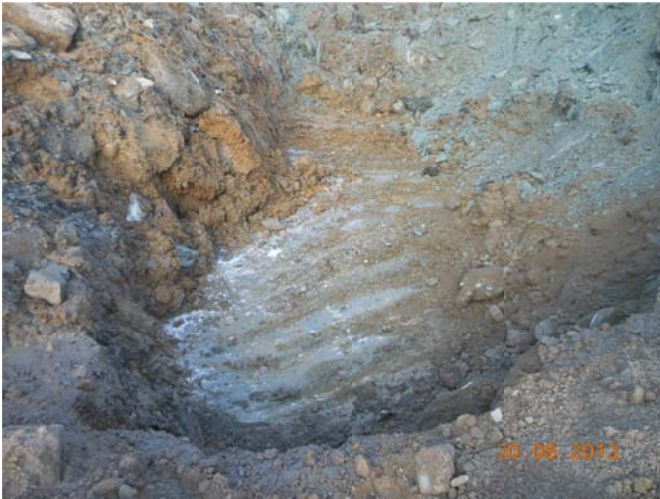
Figure 1: Excavation of the active layer until reaching the permafrost. Between 0.5 and 3.8 m were required to reach proper foundation.
