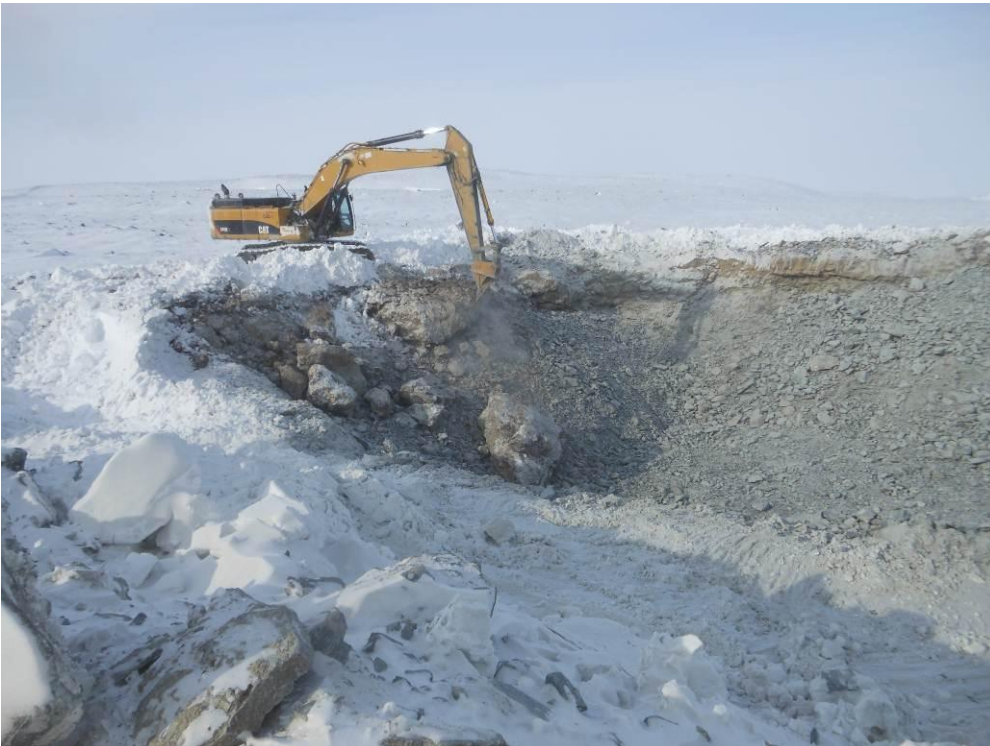
Figure 2.6: CAT 345D with ripper attachment removing till overhangs from crest
