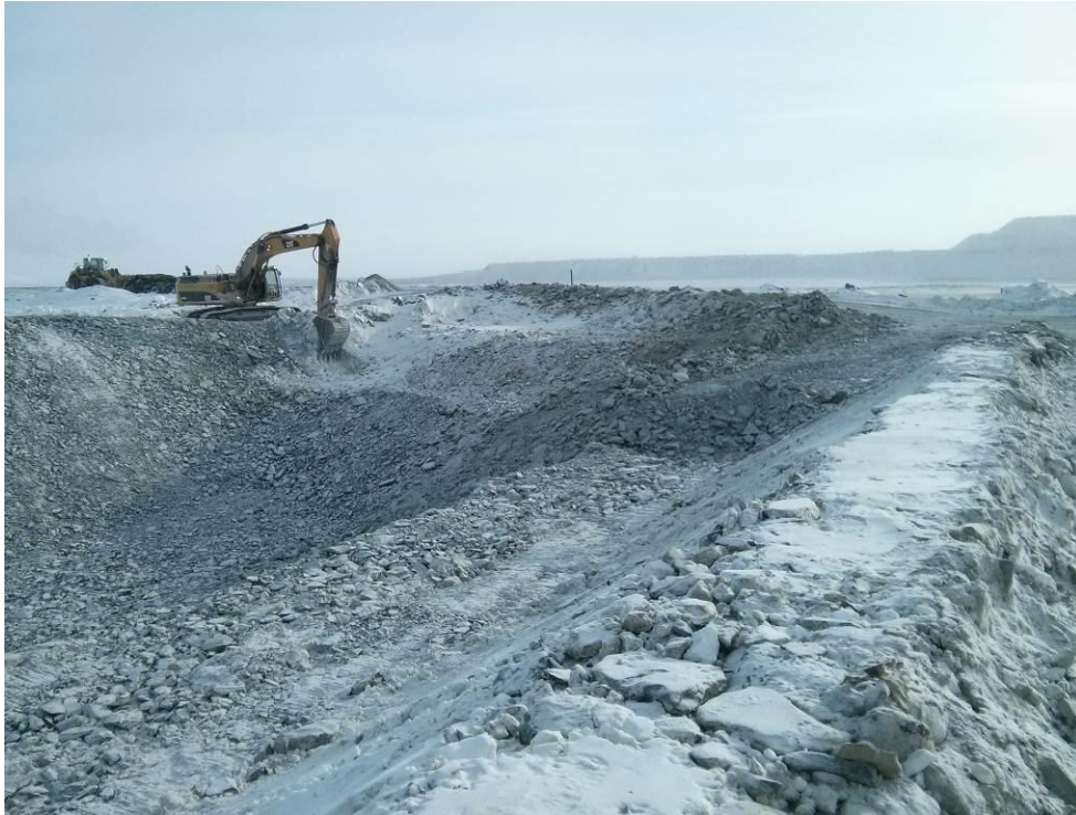
Figure 2.10: Finalized interception sump construction
