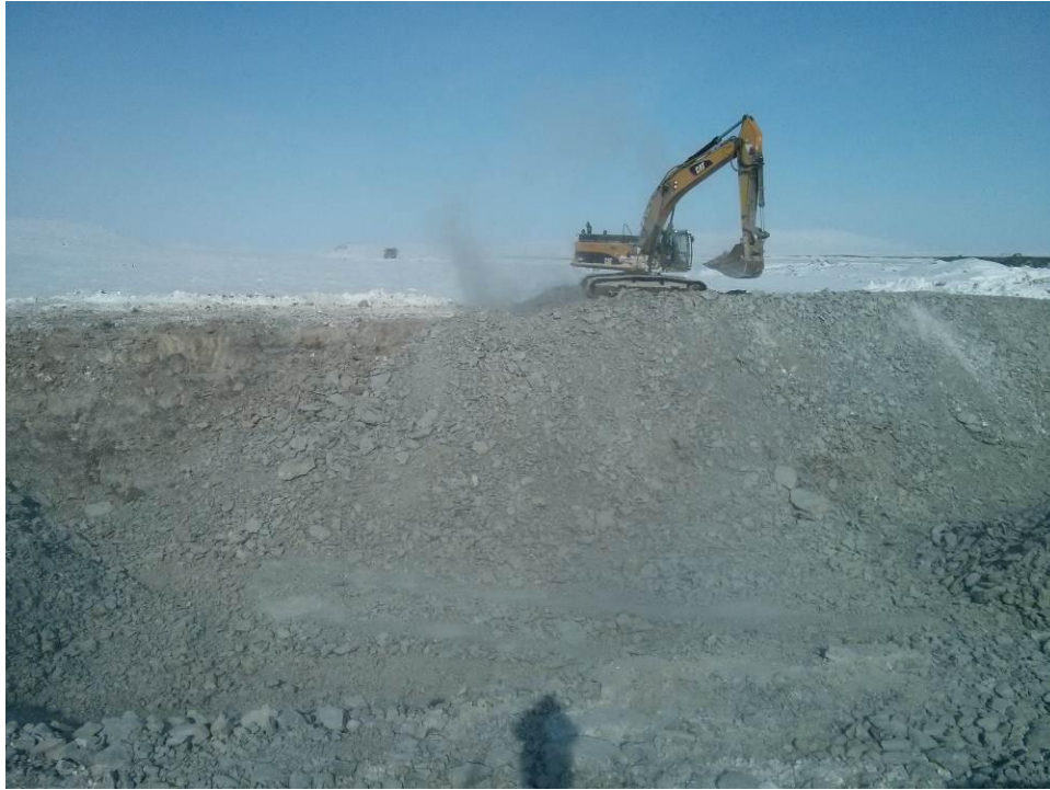
Figure 2.7: CAT 345D placing material on the slope of the sump
