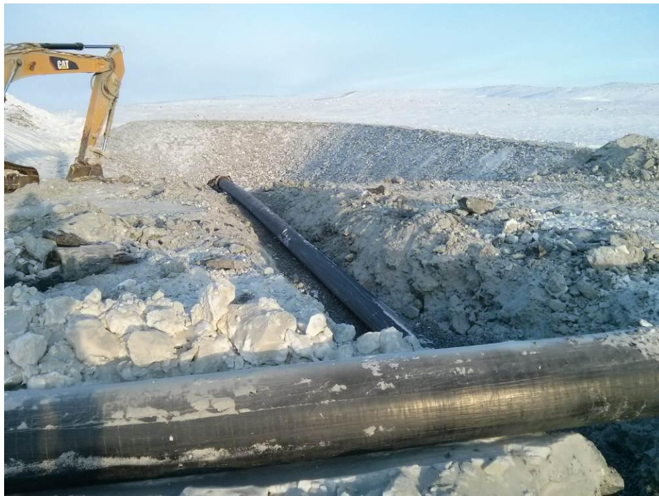
Figure 2.11: Buried 14" DR17 HDPE pipe for interception sump pumping
