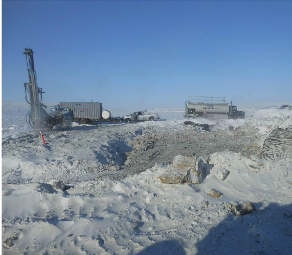
Figure 2.3: Rockmaster drilling the sump drill pattern
