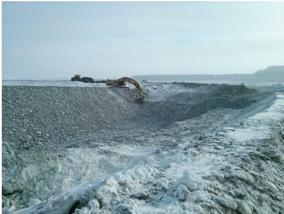
Figure 2.8: CAT 345D placing material on the slope of the sump
