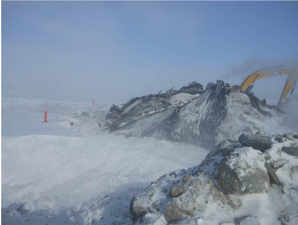
Figure 2.4: March 24 th blast muck pile with blasting mats and CAT 345D
