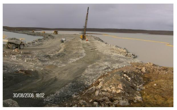
Photograph 28: Phase I and Phase II dynamic compaction of core backfill, looking north at Sta. 60+180, August 30, 2008.
