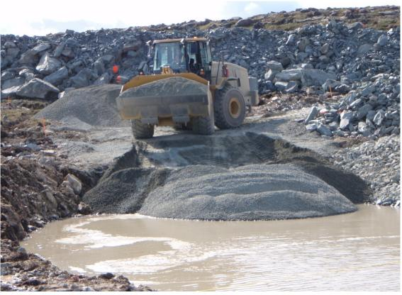
Photograph 10: Core Backfill Placement, looking south at Sta. 60+100, August 17, 2008.
