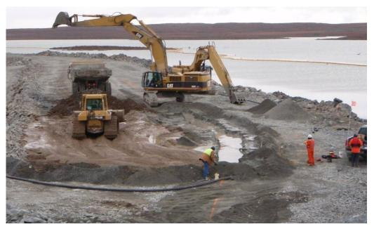
Photograph 41: Status of Slurry wall construction excavation at Sta. 60+163, QC sampling and testing by contractor of slurry at Sta. 60+112, September 8, 2008.
