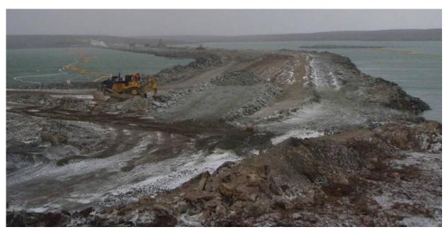
Photograph 46: Rockfill surfacing placement looking North 60+150, September 16, 2008.
