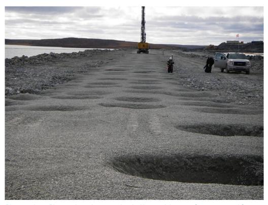
Photograph 40: Phase 4 dynamic compaction, looking south between Sta. 60+600 and Sta. 60+800, September 7, 2008.
