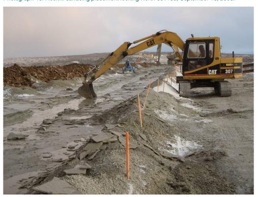
Photograph 47: Ice removal from slurry trench looking north at Sta. 60+450, September 17, 2008.
