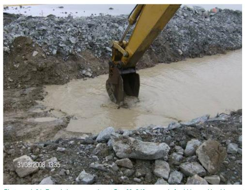
Photograph 31: Foundation preparation at Sta. 60+840, removal of cobbles and boulders up to 0.6 m diameter removed from trench base, August 31, 2008.
