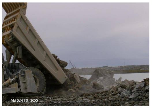
Photograph 6: Initial rockfill advancement continues towards north abutment, looking West at Sta. 60+650, August 14, 2008.
