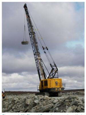
Photograph 39: Phase 4 Dynamic compaction with rig and hammer, at Sta. 60+600. September 7, 2008.
