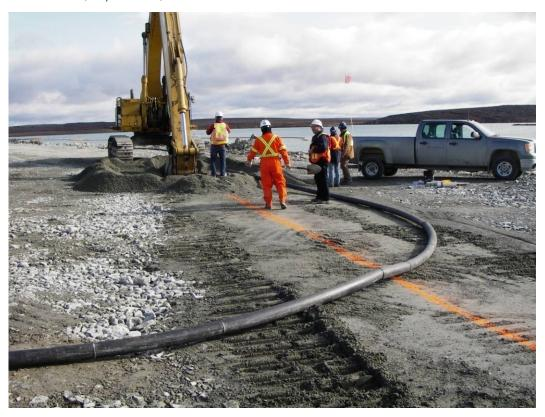
Photograph 37: Start of cut-off trench excavation by contractor at Sta. 60+096, 100 mm diameter HDPE pipe in place, centerline of trench layout shown in orange, looking north, September 7, 2008.
