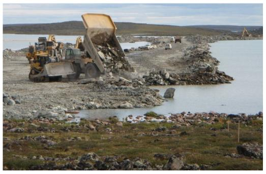
Photograph 9: Rockfill placement from Sta. 60+800 to the north abutment, looking south, August 16, 2008.
