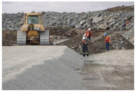
Photograph 21: Raising Core Backfill second lift to 135.1 masl and with 150 mm minus coarse rockfill wings, approx. Sta. 60+110, August 25, 2008.
