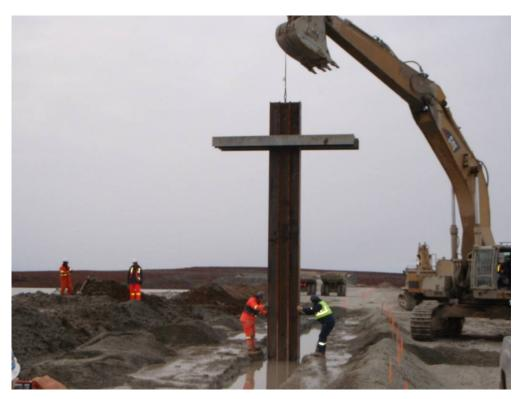
Photograph 42: A beam (gate) was installed in the trench to control and hold back the SB backfill from the excavation face at Sta. 60+393 due to sloping bedrock surface, September 13, 2008.
