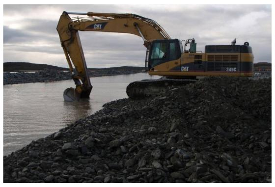
Photograph 22: Coarse Filter Placement at Sta. 60+500, looking south, August 25, 2008.
