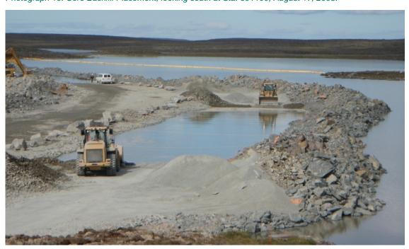
Photograph 11: Core Backfill placement at Sta. 60+200, looking north, August 18, 2008.
