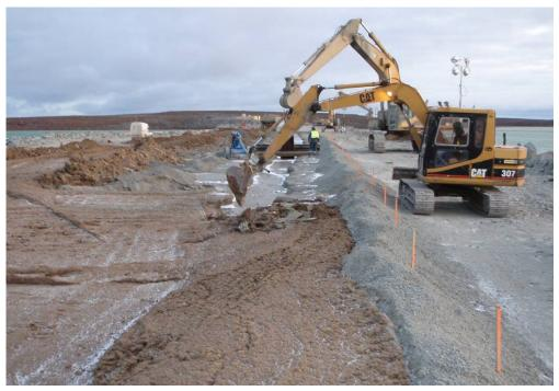
Photograph 43: Ice Removal from the slurry trench in the morning prior to SB mixing and backfilling, looking north at Sta. 60+450, September 16, 2008.
