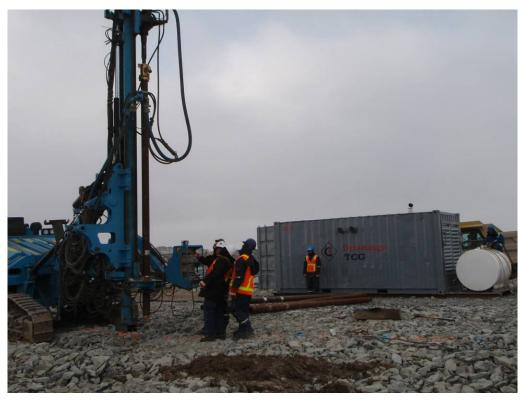
Photograph 55: Start of casing installation with Novamac Rockmaster 990 at approx. Sta 60+268. September 20, 2008.
