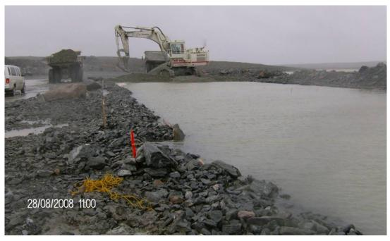
Photograph 23: AEM excavator placing Core Backfill and 150 mm minus rockfill wing from north end of Dike at Sta. 60+630, looking north, August 28, 2008.
