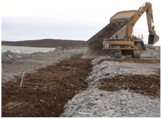
Photograph 58: Load of 150 mm minus rockfill placed over till and SB cut-off wall to Elev. 136.1 masl between Sta. 60+392 and Sta. 60+562 looking south, September 23, 2008.
