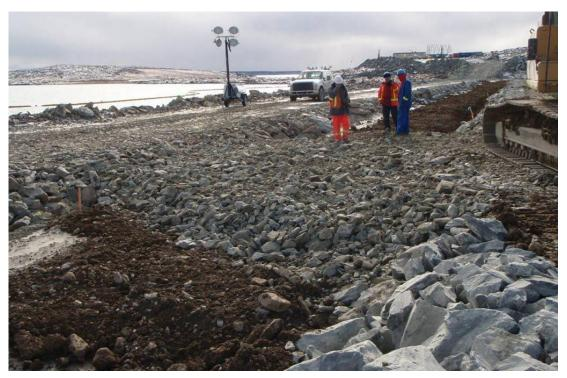
Photograph 50: Rockfill material of 150 mm minus placed over till and SB backfill as part of the thermal cap and future drilling and grouting pad, Sta. 60+314, September 18, 2008.
