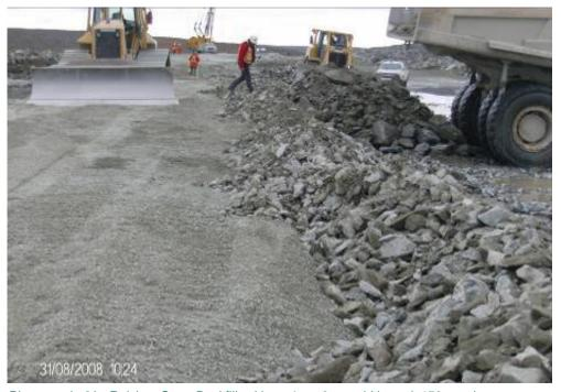
Photograph 30: Raising Core Backfill with a 4 to 6 m width and 150 mm/quarry run material on downstream side at Sta. 60+560.
