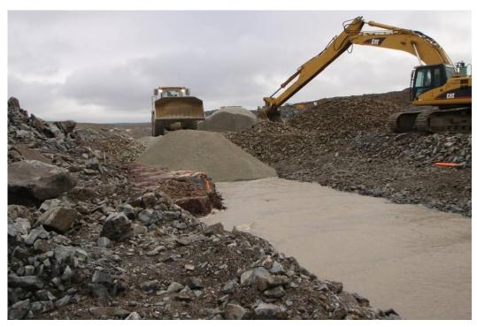
Photograph 12: Coarse filter and Core Backfill placement with excavator and loader, respectively, looking west at Sta. 60+310, August 19, 2008.
