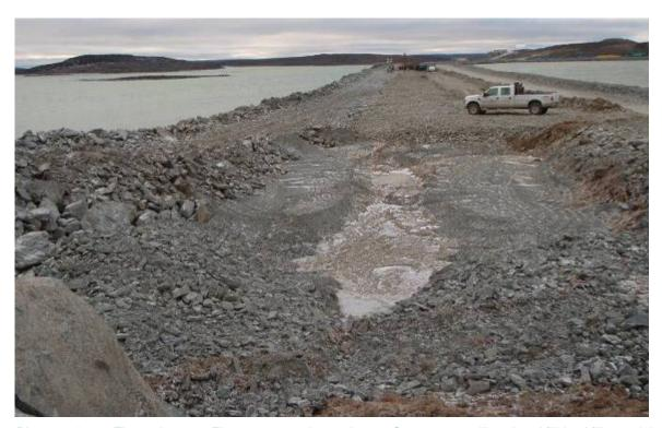
Photograph 62: Thermal cap to Elev. 136.1 masl complete to Sta. 60+830, till and rockfill backfill remaining to the north abutment, looking south, October 9, 2008.
