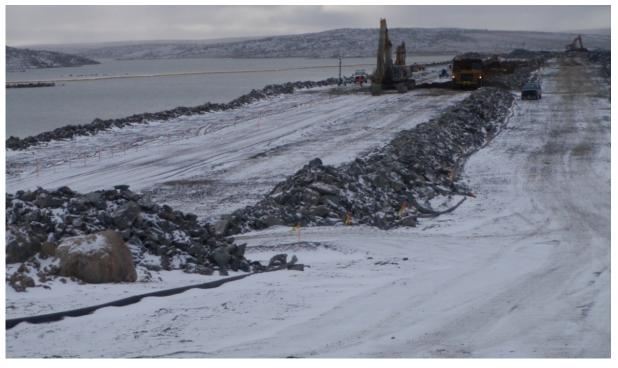
Photograph 51: SB cut-off wall excavation at Sta. 60+650, looking south, September 18, 2008.
