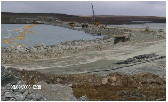
Photograph 32: Status of East Dike, dynamic compaction continues, note slurry pond construction in background, 100 mm diameter HDPE slurry pipe line layout in foreground, September 3, 2008.
