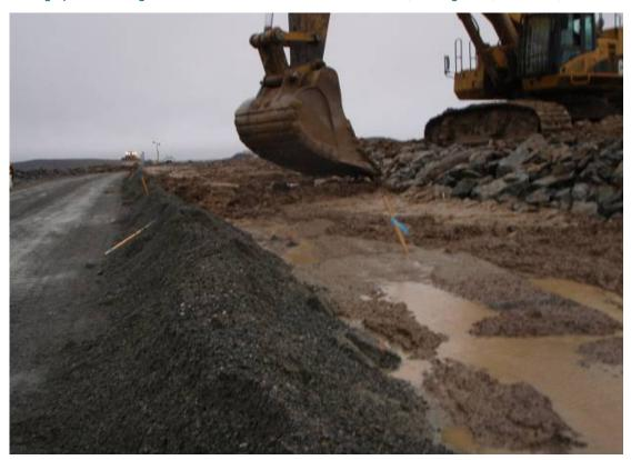
Photograph 61: Placement of till cap over SB cut-off wall at Sta. 60+600 looking south, October 7, 2008.
