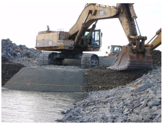
Photograph 16: Simultaneous Core Backfill and 150 mm minus rockfill wing material placement and nominal compaction with bucket at Sta. 60+325, August 21, 2008.
