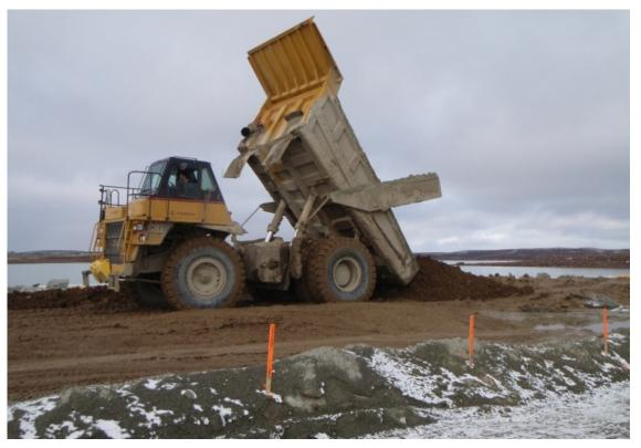
Photograph 52: Bentonite Enriched Till unloading at Sta. 60+500, looking west, September 18, 2008.
