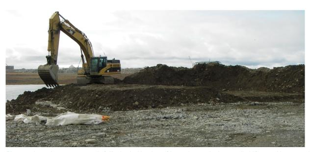
Photograph 36: A 9 m x 11 m pad of till mixed with a bag of bentonite powder in controlled lifts to achieve 1.5% bentonite added content, September 6, 2008.
