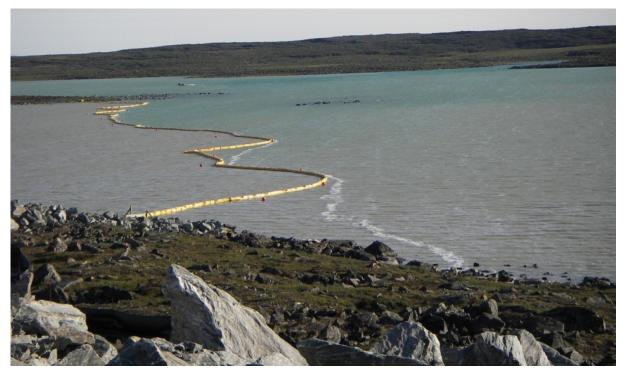
Photograph 5: Turbidity barrier function at East (lake side) of Dike, looking northeast, August 13, 2008.
