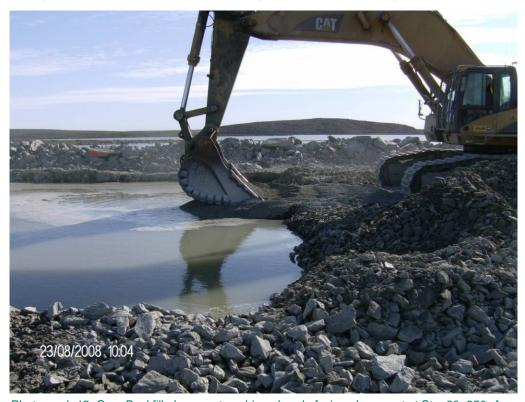
Photograph 19: Core Backfill placement pushing ahead of wing placement at Sta. 60+350, August 23, 2008.
