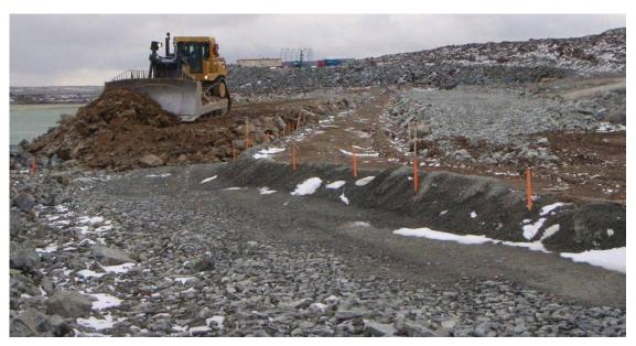
Photograph 48: Thermal Cap placement upstream of SB cut-off wall, looking south at Sta. 60+260, September 17, 2008.
