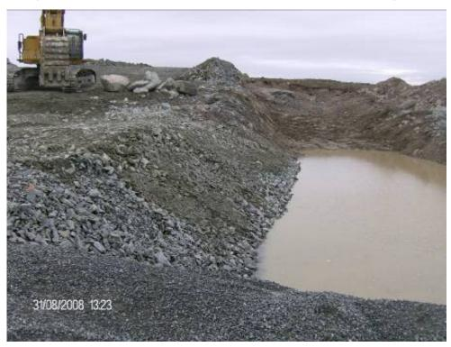
Photograph 29: Coarse filter placement tie-in to north abutment at Sta. 60+820 to Sta. 60+840, note-trench foundation preparation at north abutment exposed bedrock.
