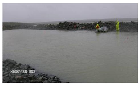
Photograph 24: Cross line bathymetry survey setting up at Sta. 60+502, looking east, August 28, 2008.
