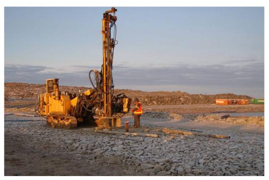
Photograph 56: Start of casing Installation with 2nd rig -Novamac Rockmaster 945 looking west at Sta. 60+200, September 22, 2008.
