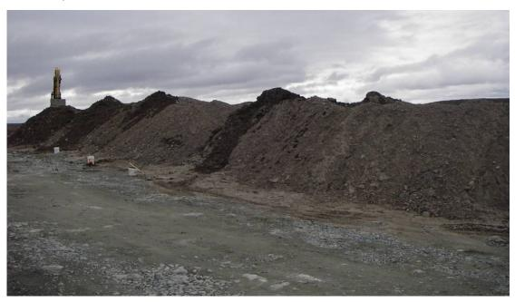
Photograph 35: Till stockpile for soil-bentonite slurry wall construction, excavator removing oversize boulders, September 4, 2008.
