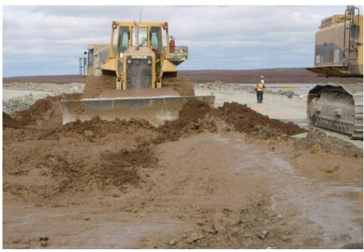
Photograph 38: Mixing of slurry with soil-bentonite, west of cut-off trench excavation prior to trench backfill, September 7, 2008.
