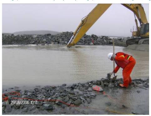
Photograph 25: A long reach 385 excavator cleaning the trench base from the south end of the trench at approx. Sta. 60+505, looking east, August 29, 2008.
