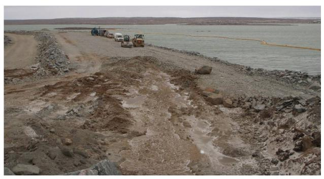
Photograph 54: Compaction of thermal cap over SB cut-off wall from Sta. 60+105 to Sta. 60+275, looking north, September 20, 2008.
