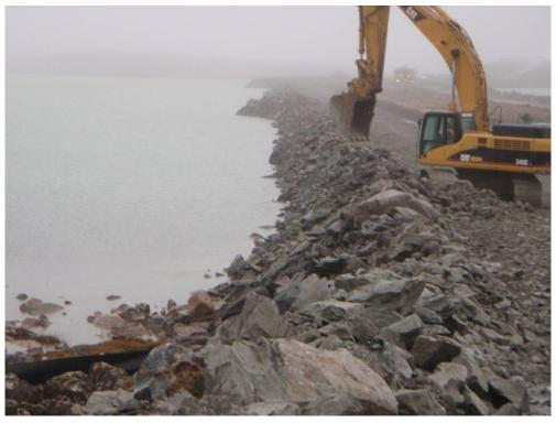
Photograph 59: Start of upstream rockfill re-sloping at approx. Sta. 60+830, September 25, 2008.
