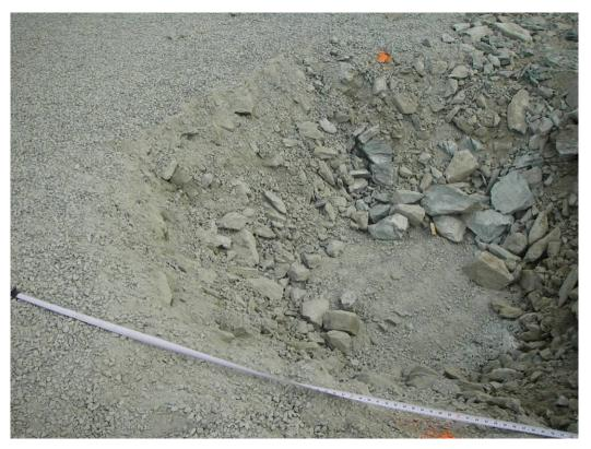
Photograph 34: A 2.5 m diameter and 1.0 m deep crater created during Phase 1/Phase 2 dynamic compaction at Sta. 60+860, September 4, 2008.
