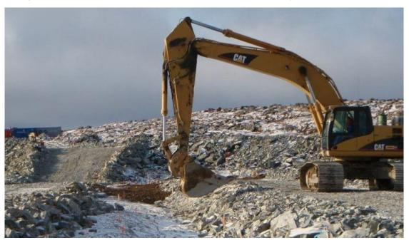
Photograph 49: Till placement over SB backfill prior to 150 mm minus rockfill placement to bring fill material to Elev. 136.1 as part of the SB cut-off wall thermal cap, September 18, 2008.
