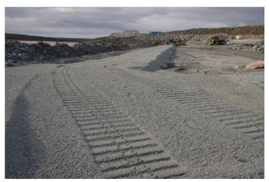
Photograph 20: Raising core backfill in lifts, showing El. 133.2 masl to El. 134.3 masl, south abutment to Sta. 60+220, looking south, August 24, 2008.
