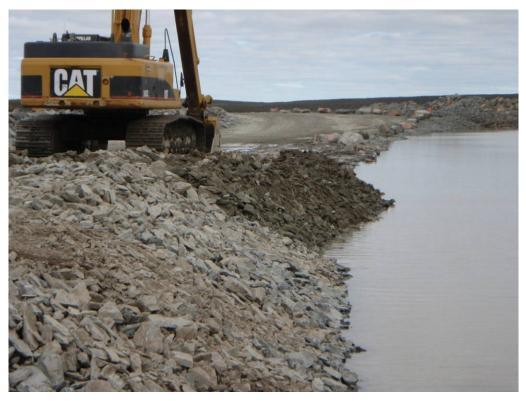
Photograph 7: Coarse Filter placement looking north-Sta. 60+125, August 16, 2008.
