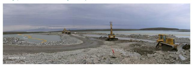
Photograph 2: East Dike rockfill placement to Sta. 60+500, trench excavation to approx. Sta. 60+320, August 9, 2008.
