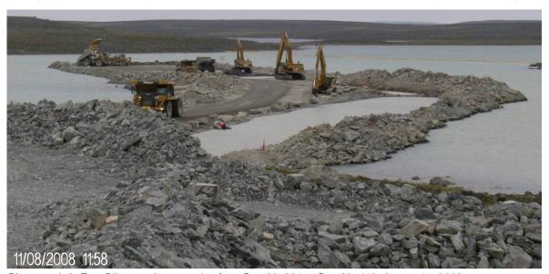
Photograph 3: East Dike trench excavation from Sta. 60+391 to Sta. 60+410, August 11, 2008.
