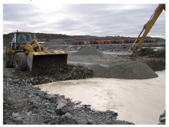
Photograph 13: Crushed rockfill and core backfill placement at Sta. 60+400, looking south, August 20, 2008.
