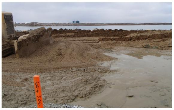
Photograph 53: Backfill with soil-bentonite mix in slurry trench, at Sta. 60+506 looking west, September 18, 2008.
