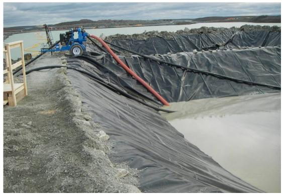
Photograph 33: Hydration of bentonite slurry mix in slurry pond set up (HDPE liner, pump and HDPE slurry lines), September 4, 2008.
