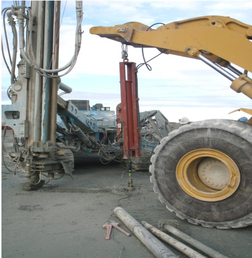
Figure 1: LPT Hammer Hoisted by a Caterpillar 966 Front End Loader
