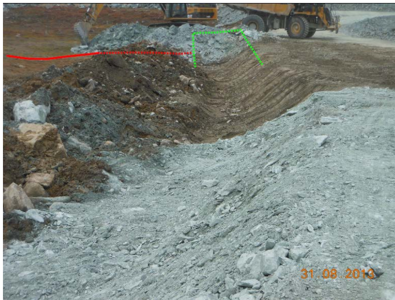
Photo 7 – Construction of Waste Rock Plug
