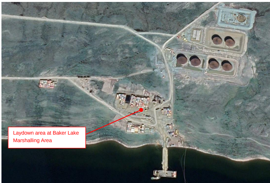
Fig. 2: Laydown area at Baker Lake Marshalling Area – Aerial view (ref : Google Earth-2019)
