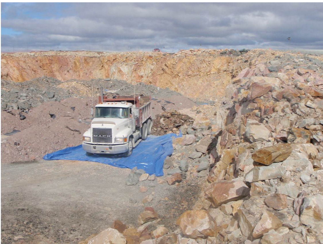
Picture #6 Storage of the contaminated soil on tarps
