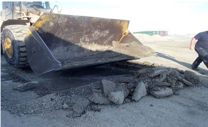
5. May 23rd – 0-20 mm granular material removal
