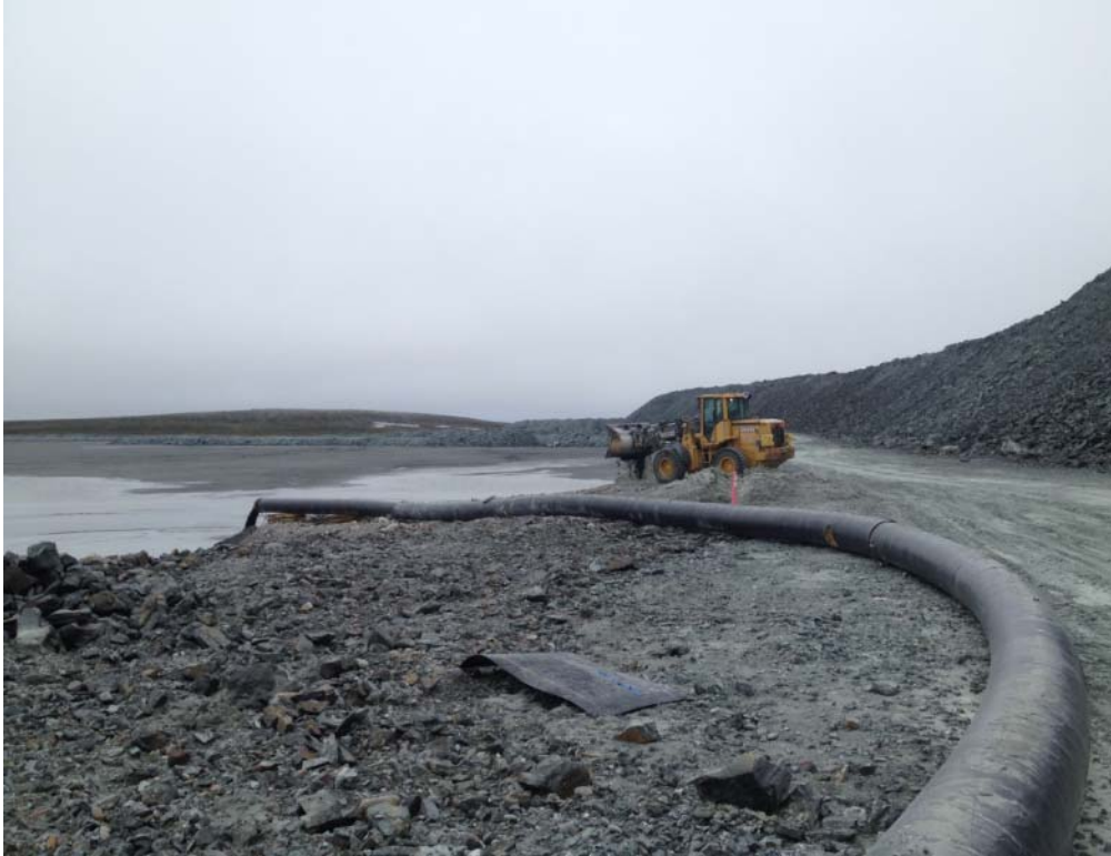
Photo 3 – Disposal of the contaminated soil in TSF
