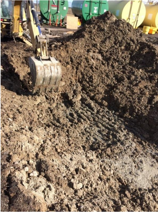
Figure 1: Backhoe excavating contaminated soil
