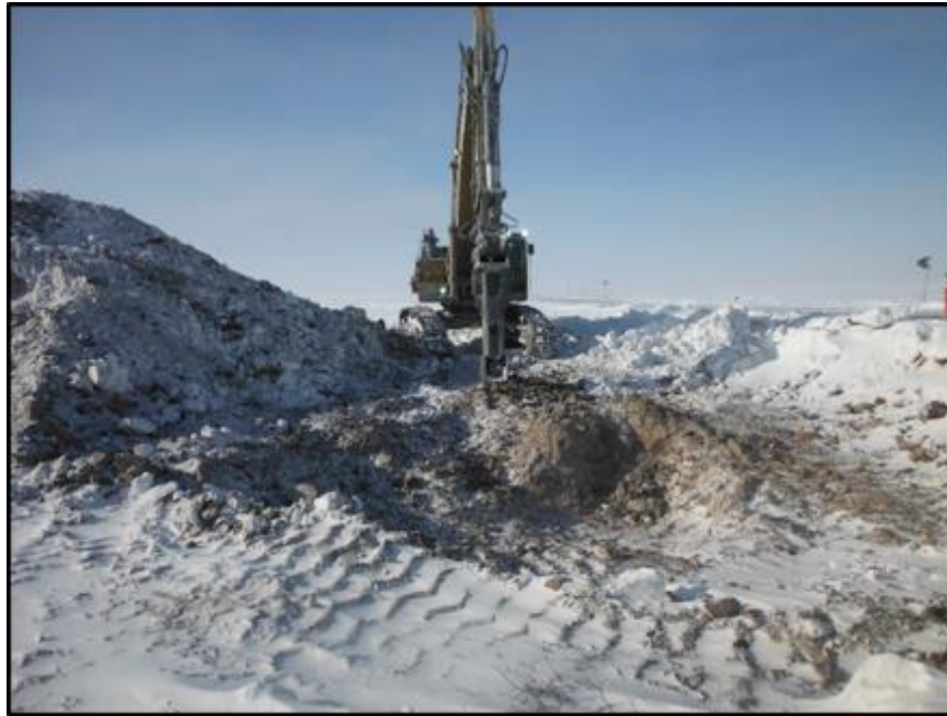
April 21: Using the hammer to remove material.
