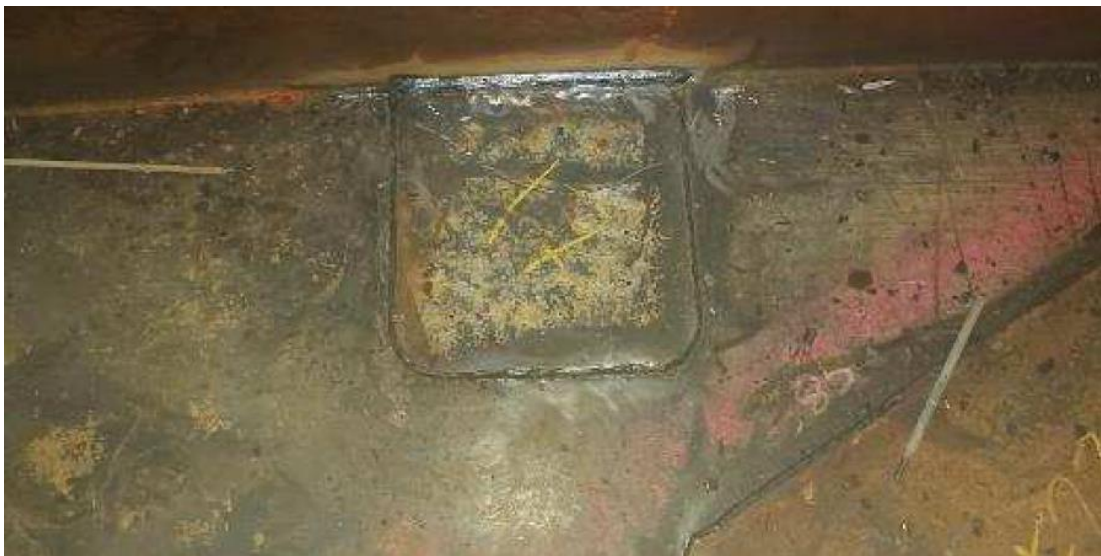
Patch plate over hole inside Fuel Tank #5
