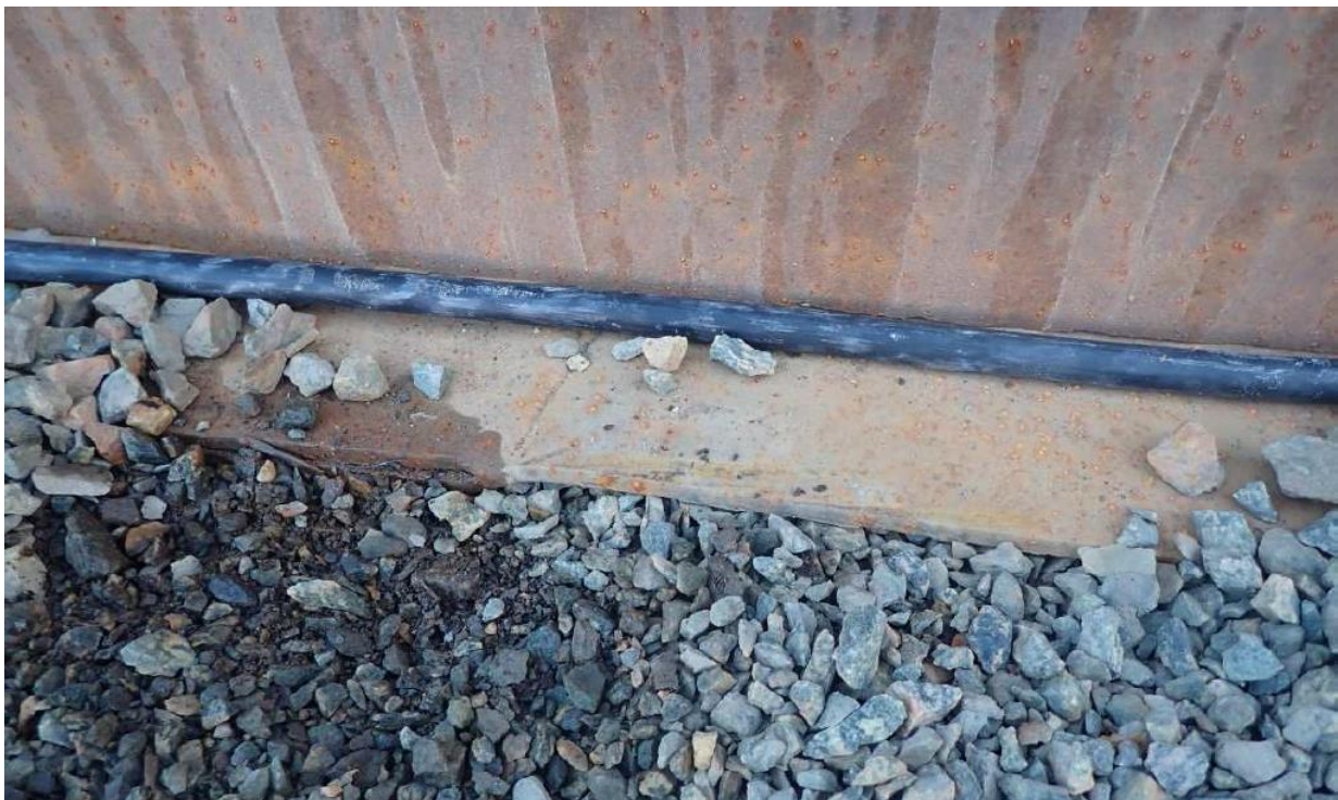
Visual observation of Fuel leaking out of the tank
