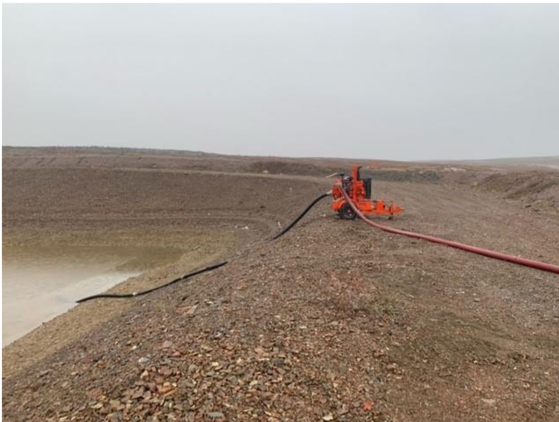
Figure 8. Pump Intake in Secondary Containment of Tanks #5-6 (2021/09/10)
