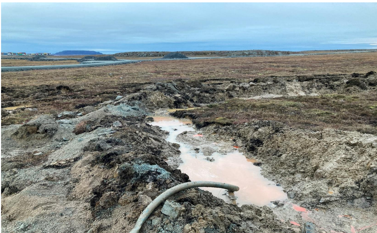
Figure 5. Sump, Trench & Berm Containing Contaminated Runoff (2021-09-09)
