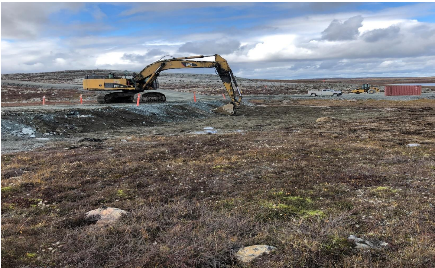
Figure 8. Incident Location Backfilled with Till Material (2021-09-12)
