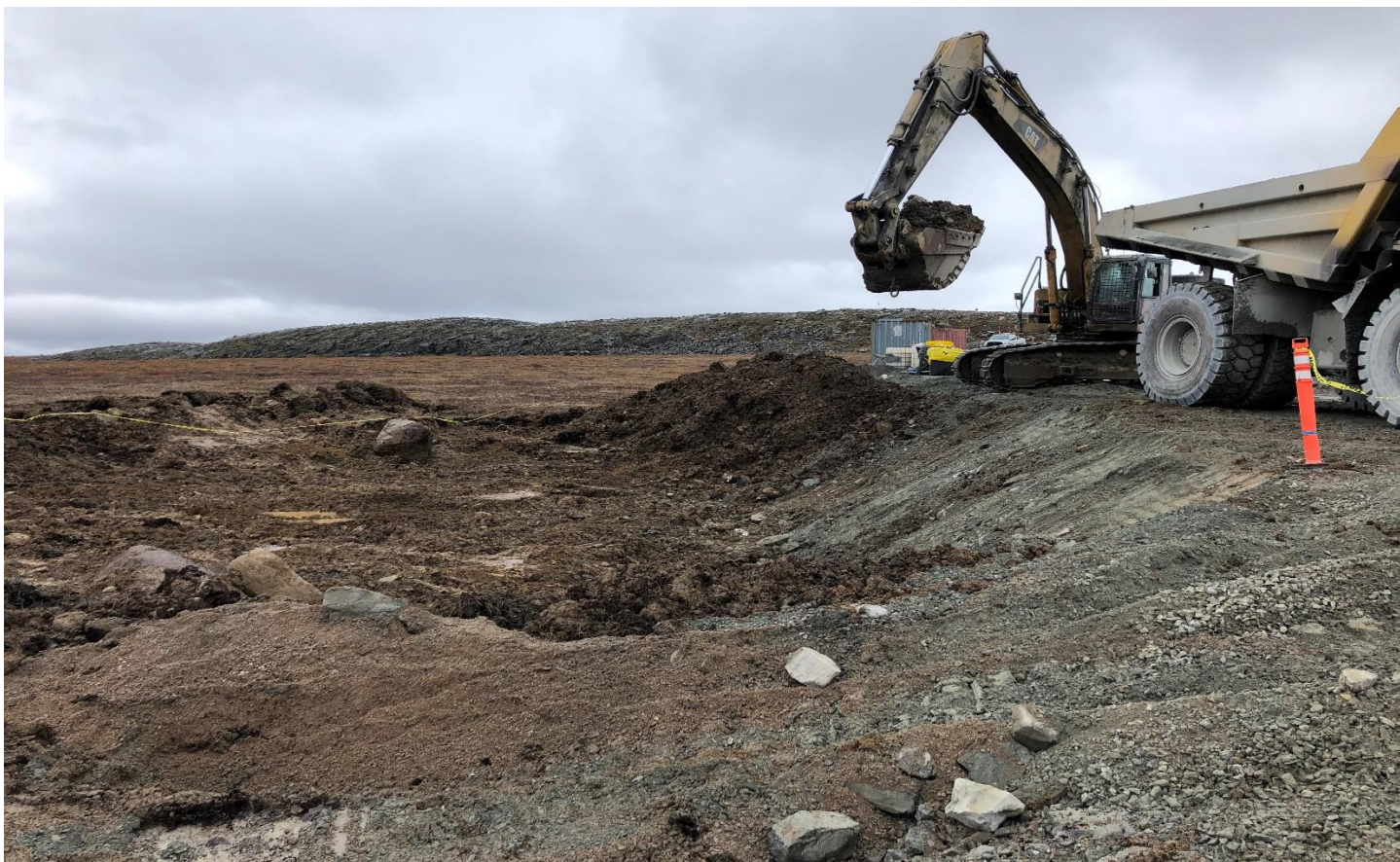
Figure 6. Excavation of Contaminated Soil (2021-09-10)
