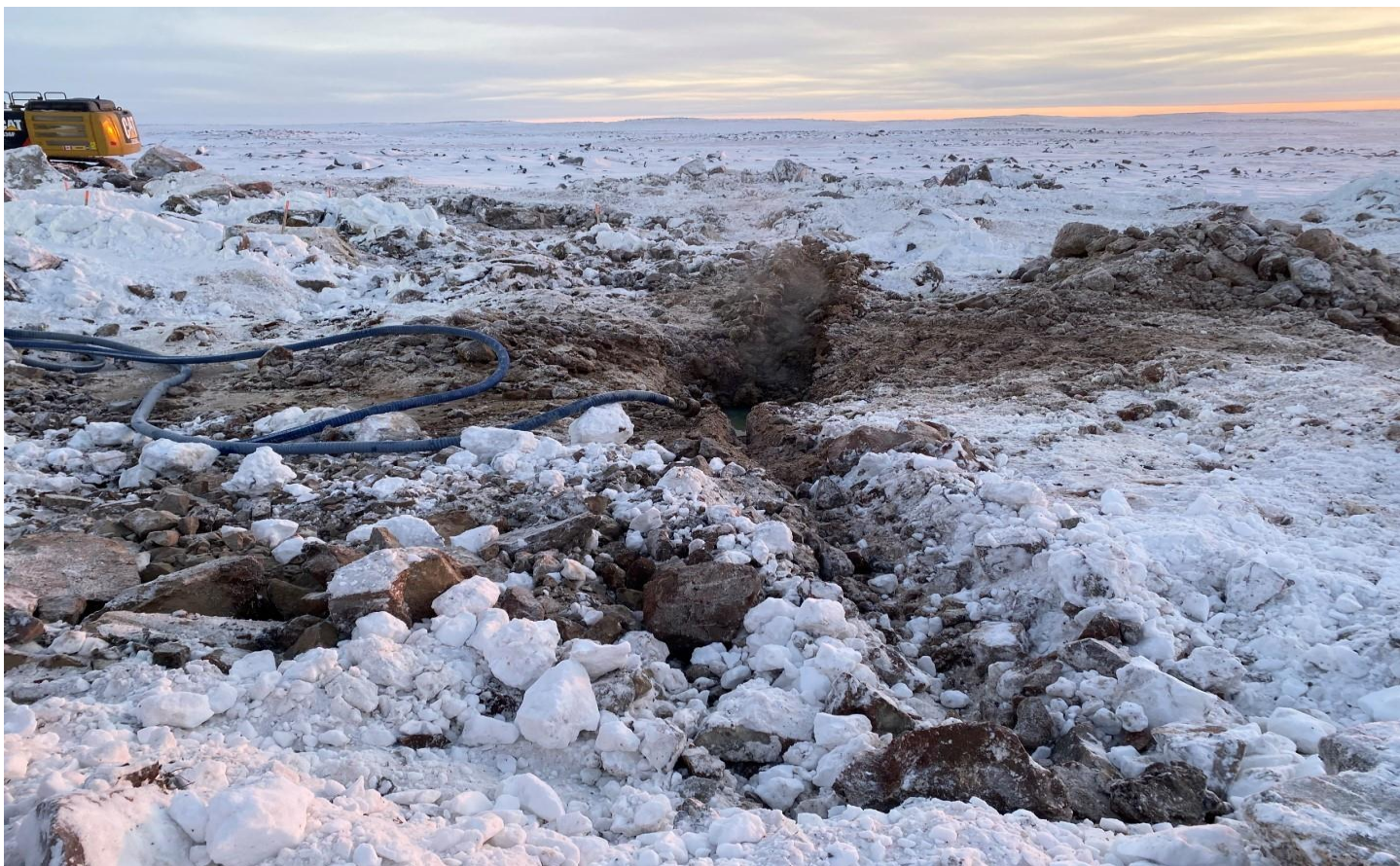
Figure 9. Surface drainage trenches -2022-12-02
