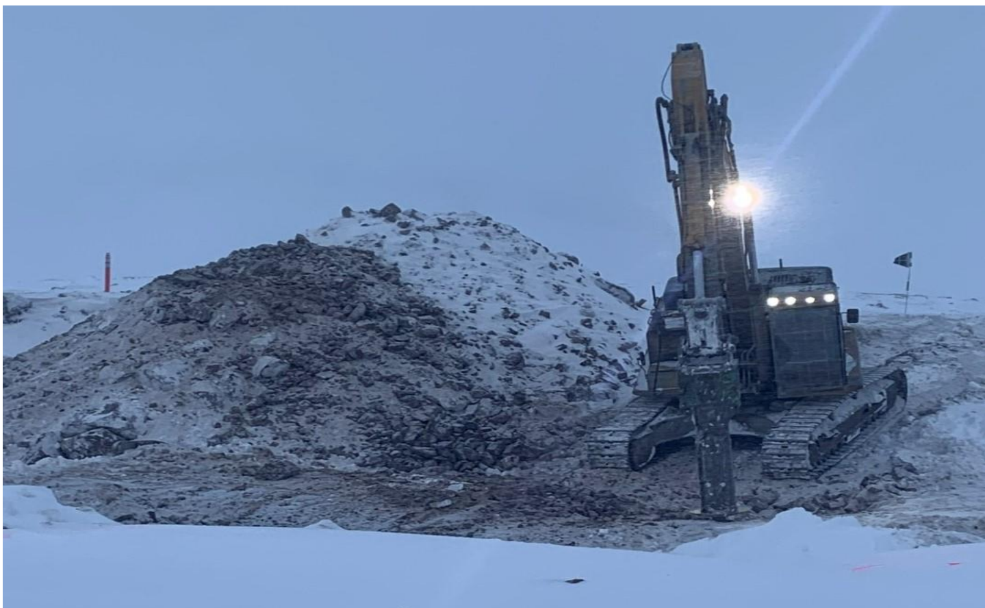
Figure 15. Excavation of spill area 2022-12-12
