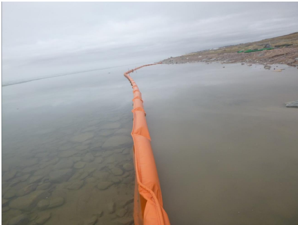
Figure 6. Contained turbidity & sediments at Baker Lake (2023/06/07)
