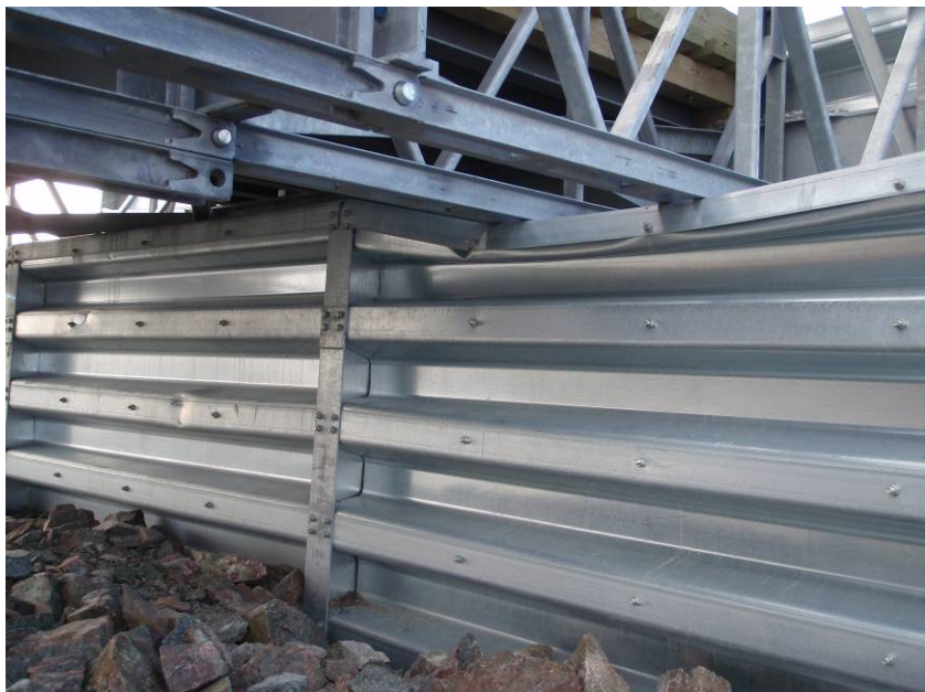
PHOTOGRAPH 6 – Bridge 1 - R02, km 8+750
