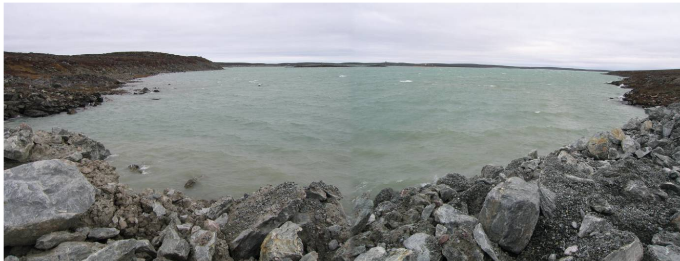
PHOTOGRAPH 3 – South Camp Dike
