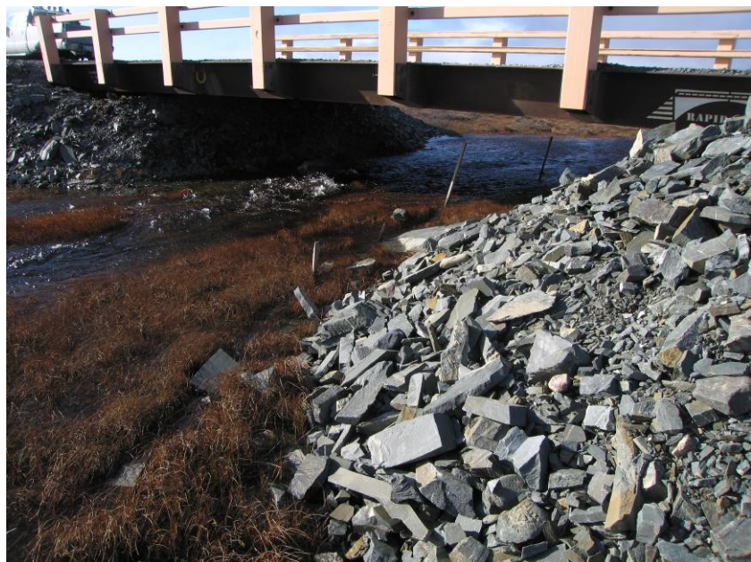
PHOTOGRAPH 30 – Bridge 5 - R13, km 62+060
