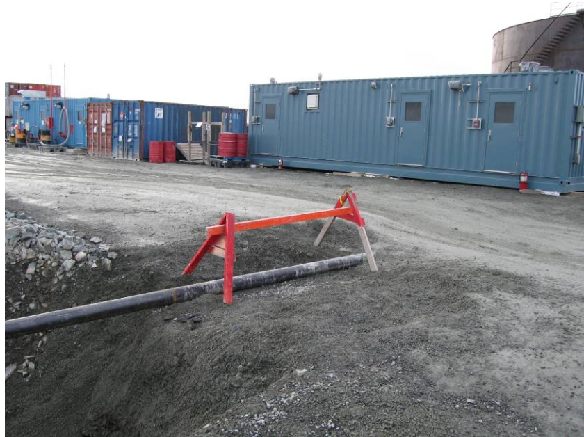
PHOTOGRAPH 6 – Meadowbank Tank Farm
