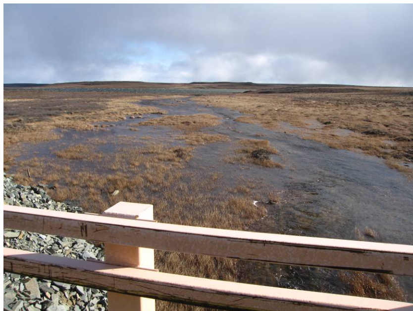
PHOTOGRAPH 29 – Bridge 5 - R13, km 62+060
