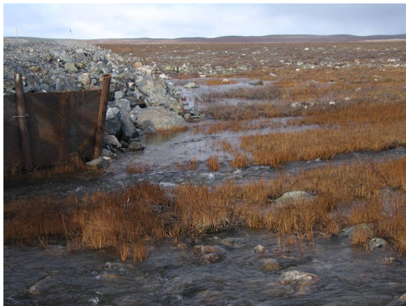
PHOTOGRAPH 59 – Bridge 9 - R19, km 83+100
