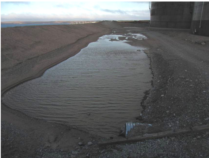
PHOTOGRAPH 16 – Baker Lake Tank Farm
