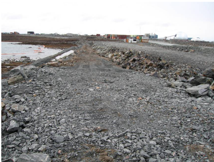
PHOTOGRAPH 1 – West Channel Dike
