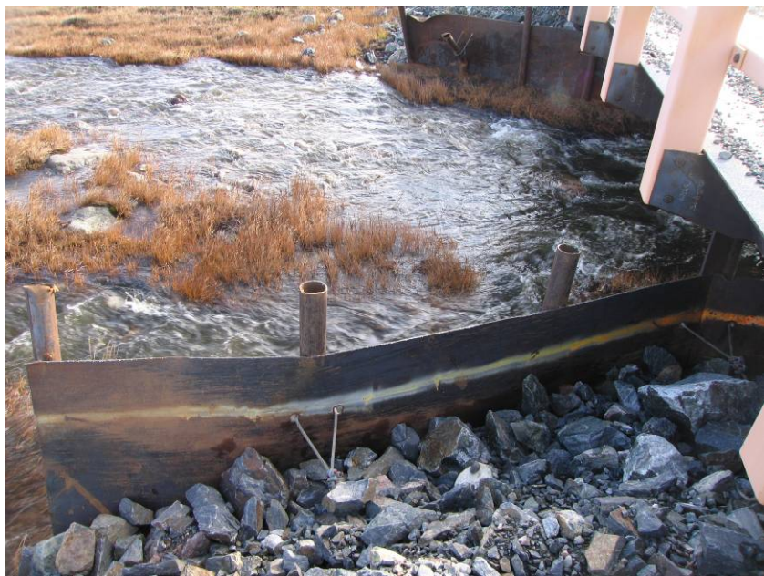
PHOTOGRAPH 52 – Bridge 9 - R19, km 83+100
