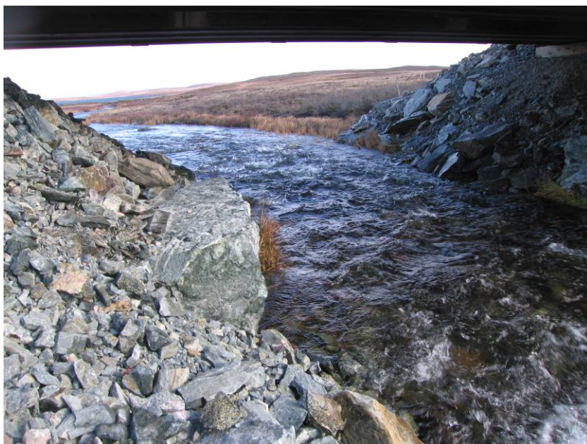
PHOTOGRAPH 24 – Bridge 4 - R09, km 48+500
