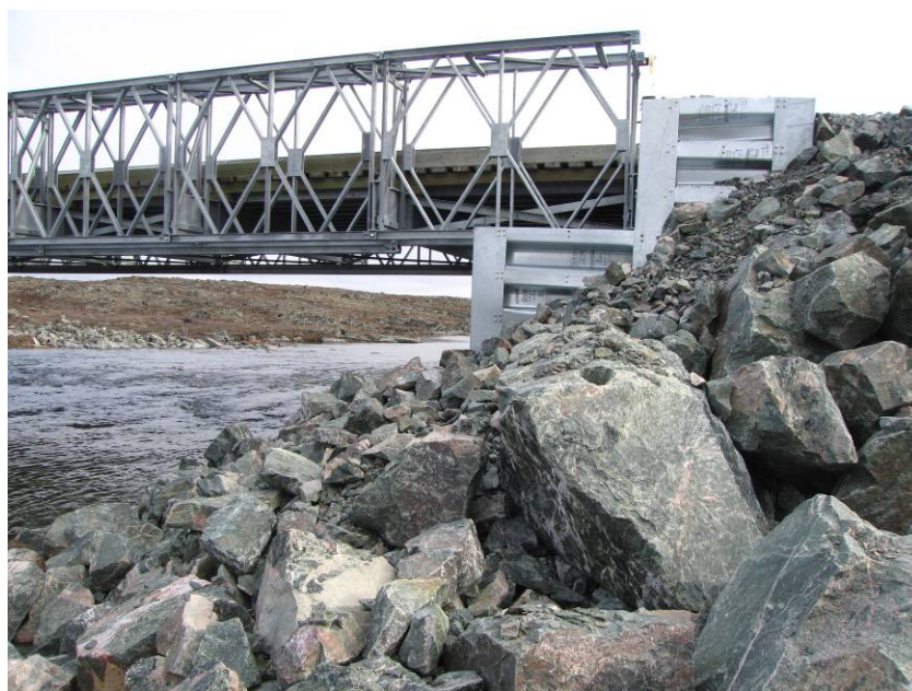
PHOTOGRAPH 20 – Bridge 3 - R06, km 23+100
