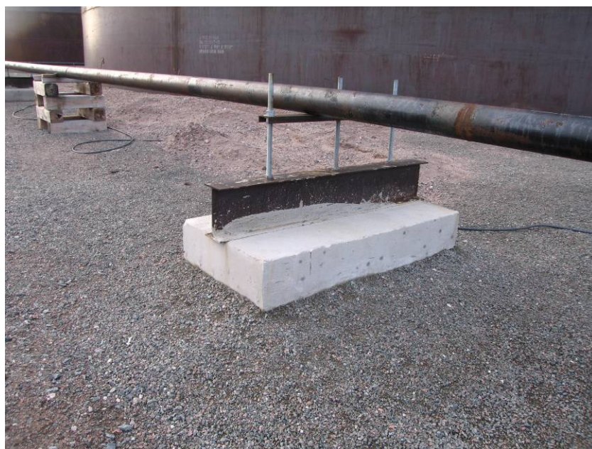
PHOTOGRAPH 22 – Baker Lake Tank Farm
