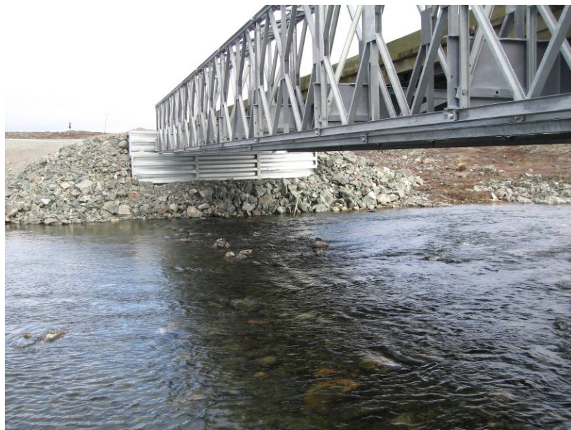
PHOTOGRAPH 19 – Bridge 3 - R06, km 23+100
