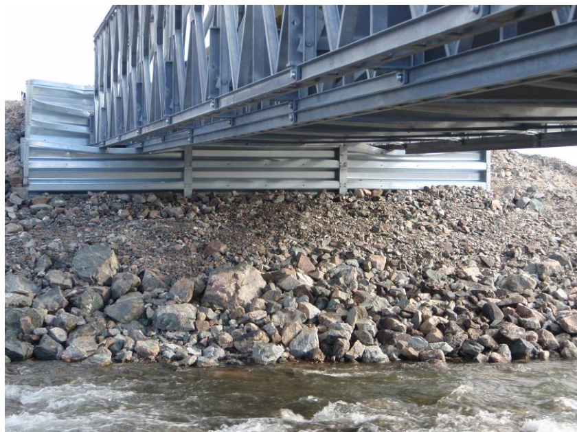
PHOTOGRAPH 7 – Bridge 1 - R02, km 8+750
