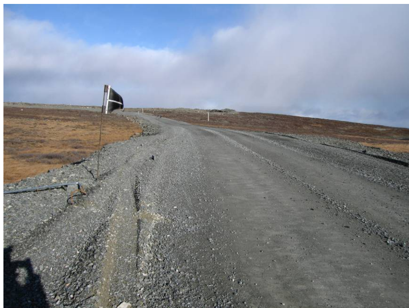
PHOTOGRAPH 29 – Bridge 5 - R13, km 62+060
