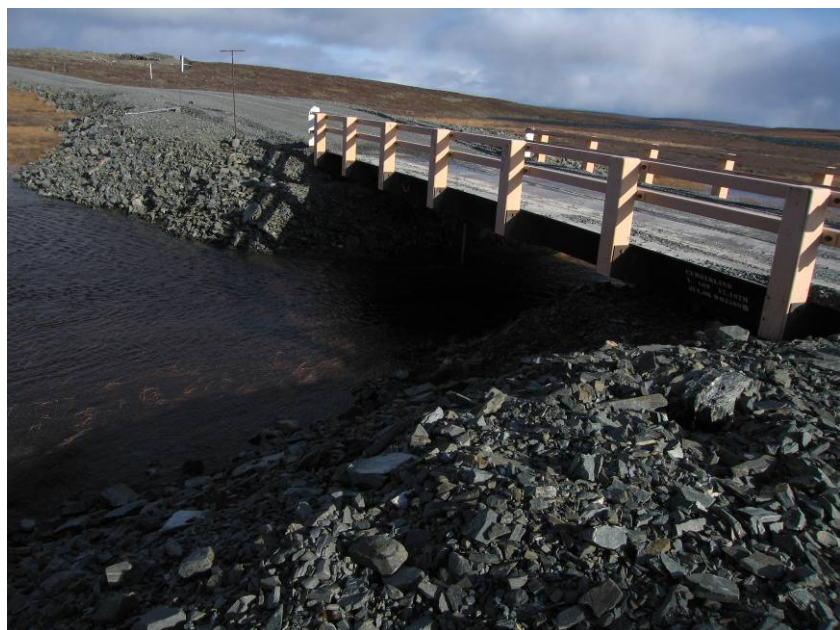
PHOTOGRAPH 31 – Bridge 5 - R13, km 62+060
