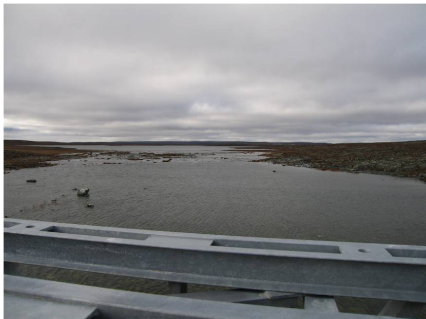
PHOTOGRAPH 17 – Bridge 3 - R06, km 23+100
