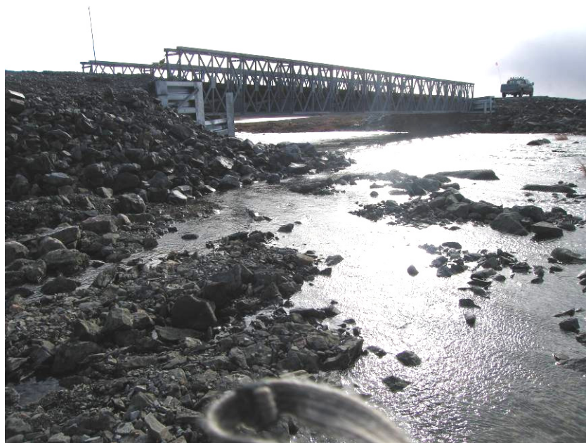
PHOTOGRAPH 37 – Bridge 6 - R15, km 69+200
