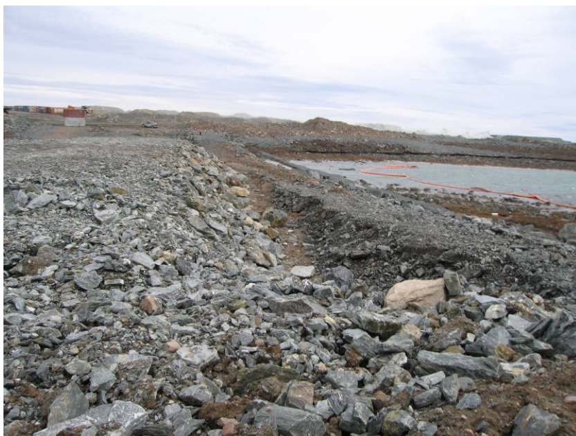
PHOTOGRAPH 2 – West Channel Dike
