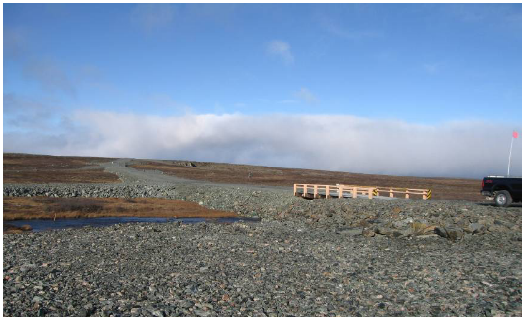
PHOTOGRAPH 26 – Bridge 4 - R09, km 48+500
