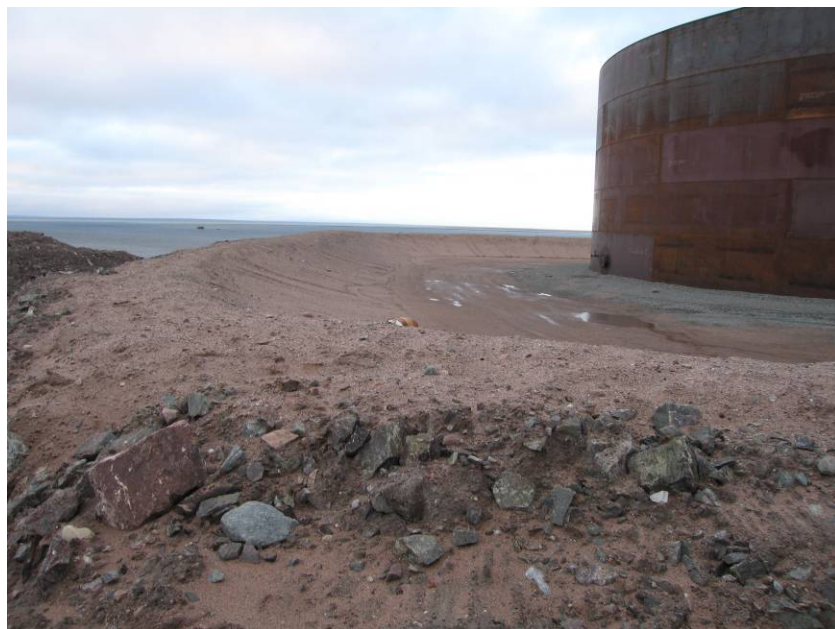
PHOTOGRAPH 7 – Baker Lake Tank Farm
