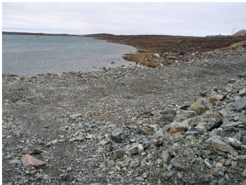
PHOTOGRAPH 2 – South Camp Dike
