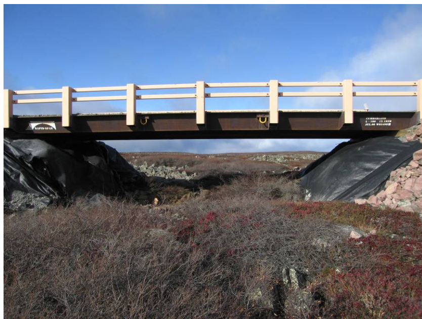
PHOTOGRAPH 50 – Bridge 8 - R18, km 79+500
