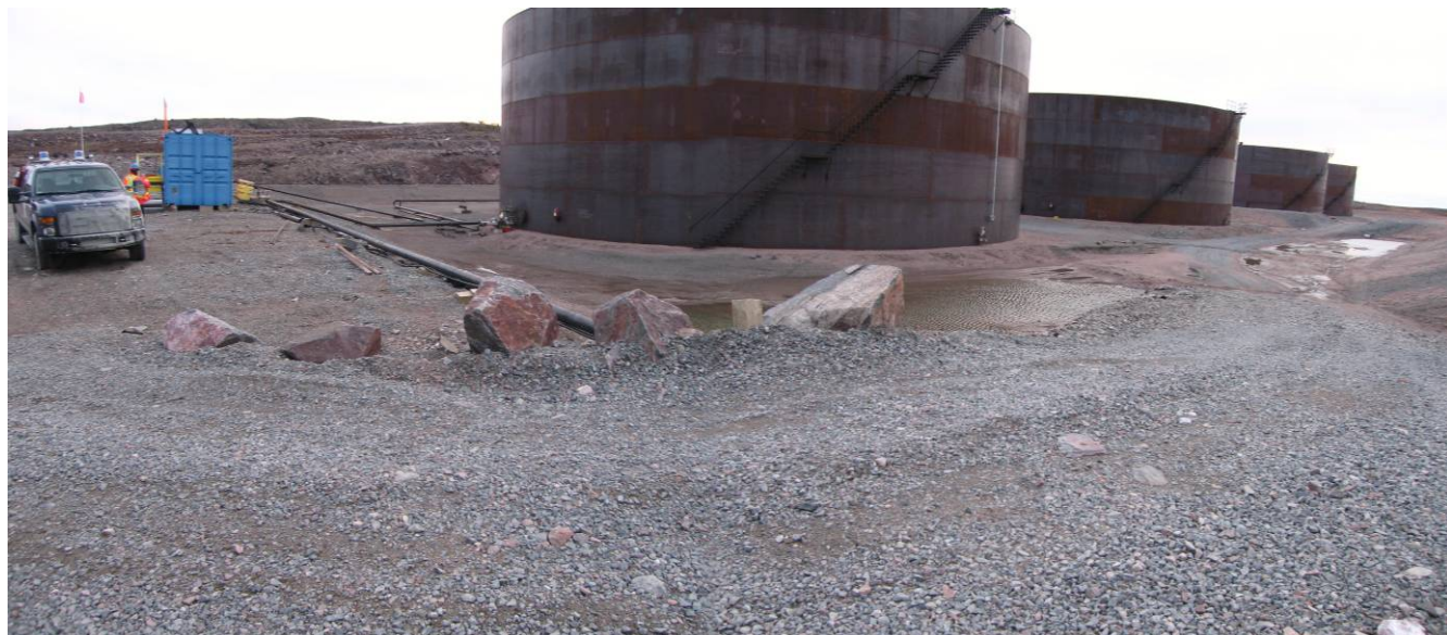
PHOTOGRAPH 2 – Baker Lake Tank Farm
