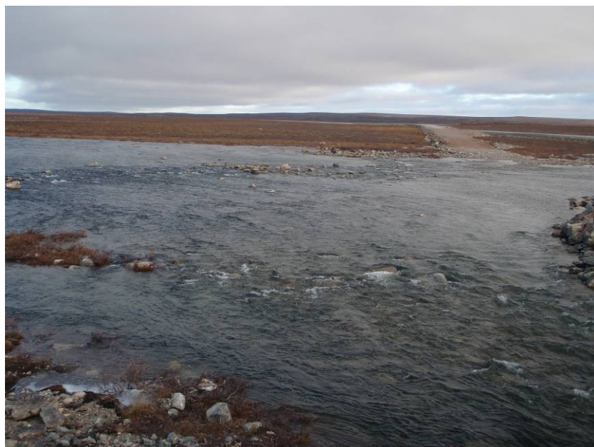
PHOTOGRAPH 4 – Bridge 1 - R02, km 8+750
