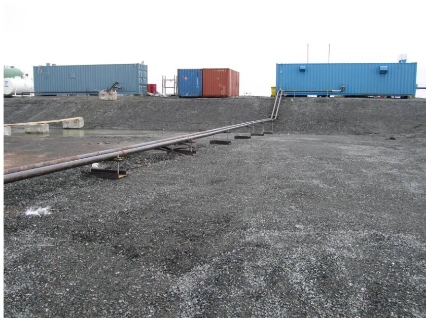
PHOTOGRAPH 7 – Meadowbank Tank Farm
