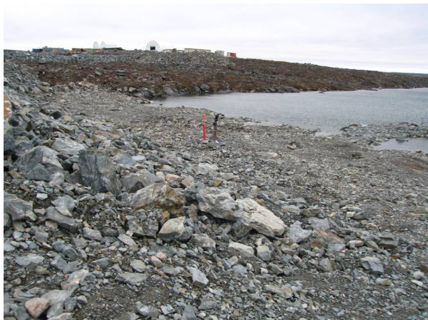
PHOTOGRAPH 1 – South Camp Dike
