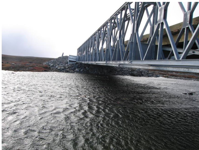
PHOTOGRAPH 38 – Bridge 6 - R15, km 69+200
