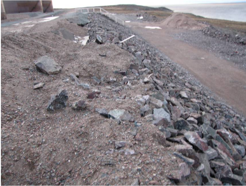
PHOTOGRAPH 3 – Baker Lake Tank Farm
