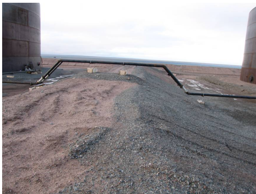
PHOTOGRAPH 8 – Baker Lake Tank Farm
