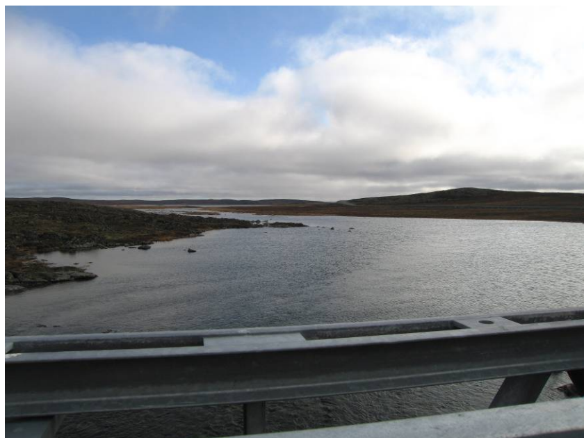
PHOTOGRAPH 18 – Bridge 3 - R06, km 23+100
