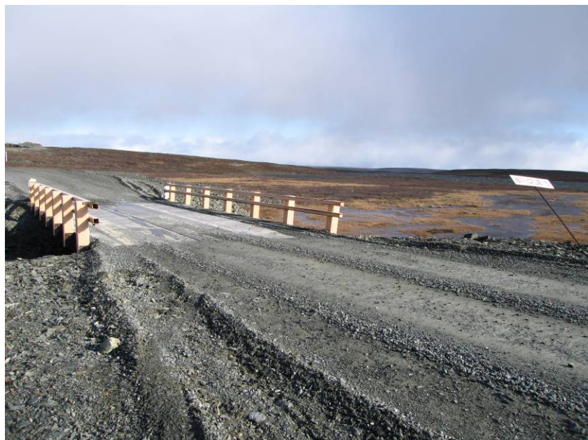
PHOTOGRAPH 27 – Bridge 5 - R13, km 62+060
