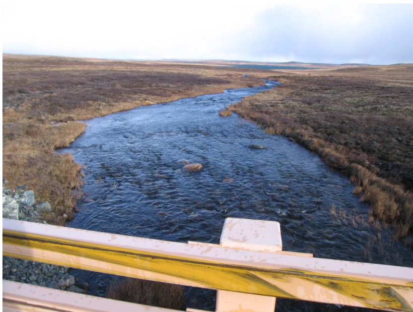
PHOTOGRAPH 23 – Bridge 4 - R09, km 48+500
