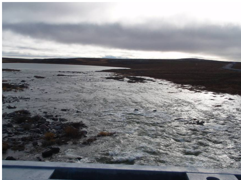
PHOTOGRAPH 3 – Bridge 1 - R02, km 8+750
