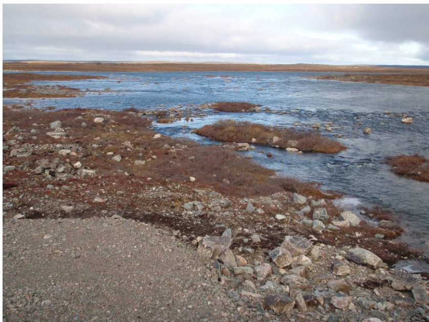
PHOTOGRAPH 5 – Bridge 1 - R02, km 8+750
