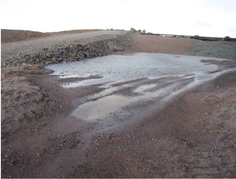
PHOTOGRAPH 15 – Baker Lake Tank Farm
