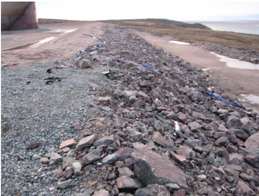
PHOTOGRAPH 4 – Baker Lake Tank Farm
