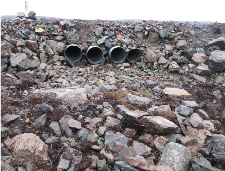
PHOTOGRAPH D2-17: 4 new culverts, approximately km 8+850
