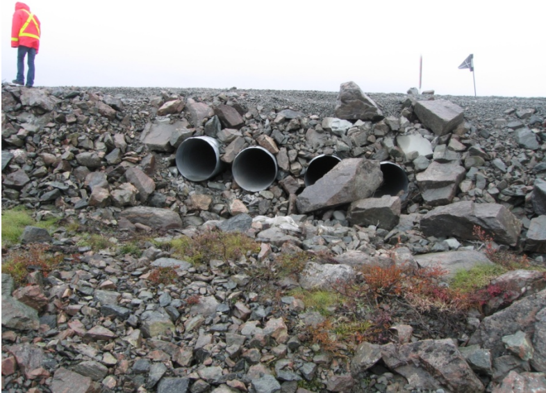
PHOTOGRAPH D2-19: 4 new culverts, approximately km 8+850
