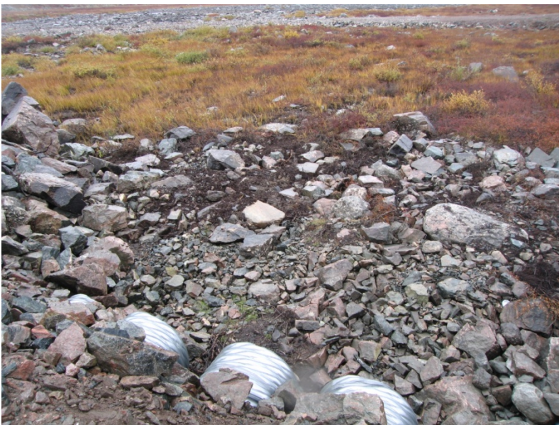
PHOTOGRAPH D2-18: 4 new culverts, approximately km 8+850
