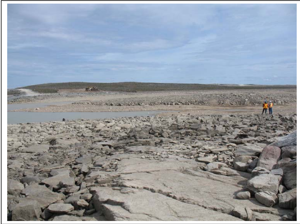
Photo # 11 Stormwater Dike, variation of foundation conditions
