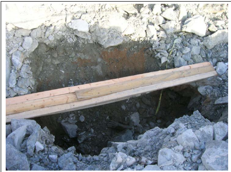
Photo # 8 East Dike, sinkhole at stn. 6+472
