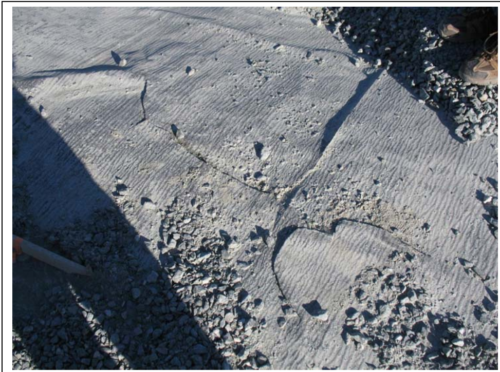
Photo # 12 Stormwater dike, liner damaged by construction subsequent to installation
