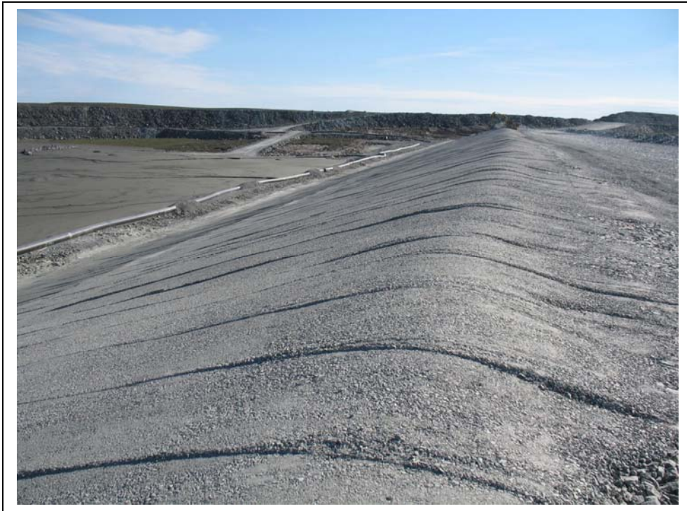
Photo # 10 Stormwater dike, placed and compacted bedding
