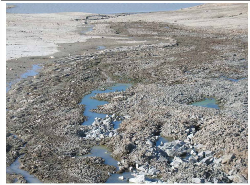
Photo # 20 Central dike axis, flow slide in lakebed sediments
