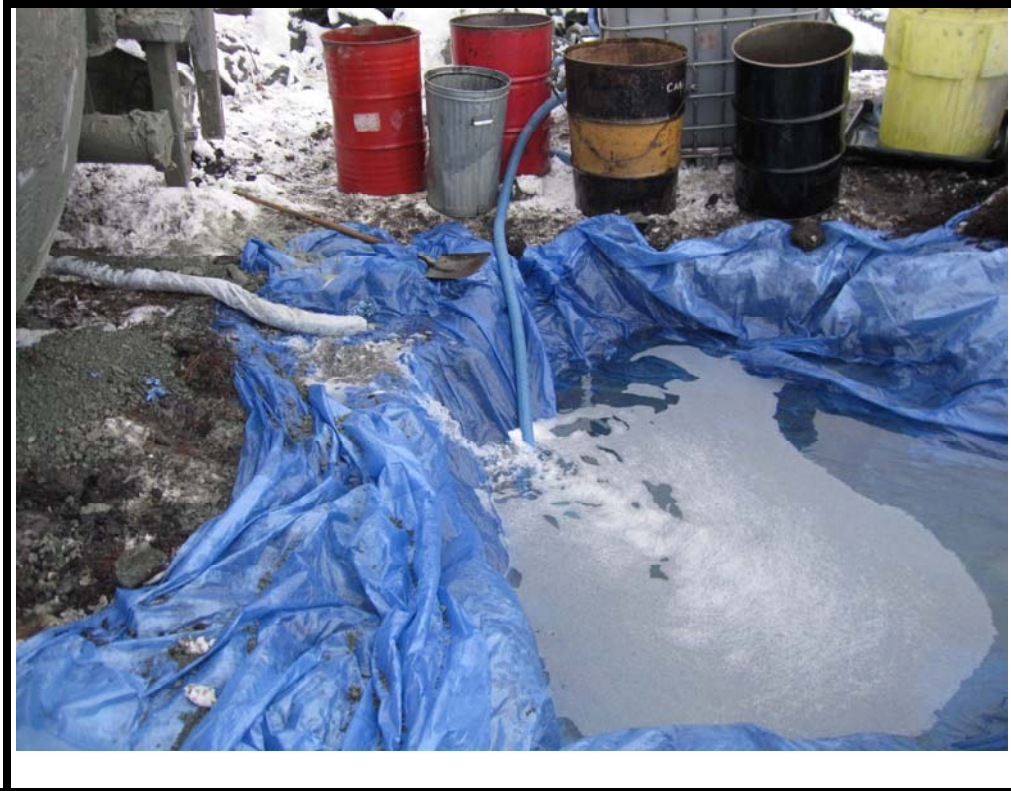
Photo No 3 : View of the first pond where the fuel leaching from the tanker was pumped directly in another 40,000 L tanker truck.
