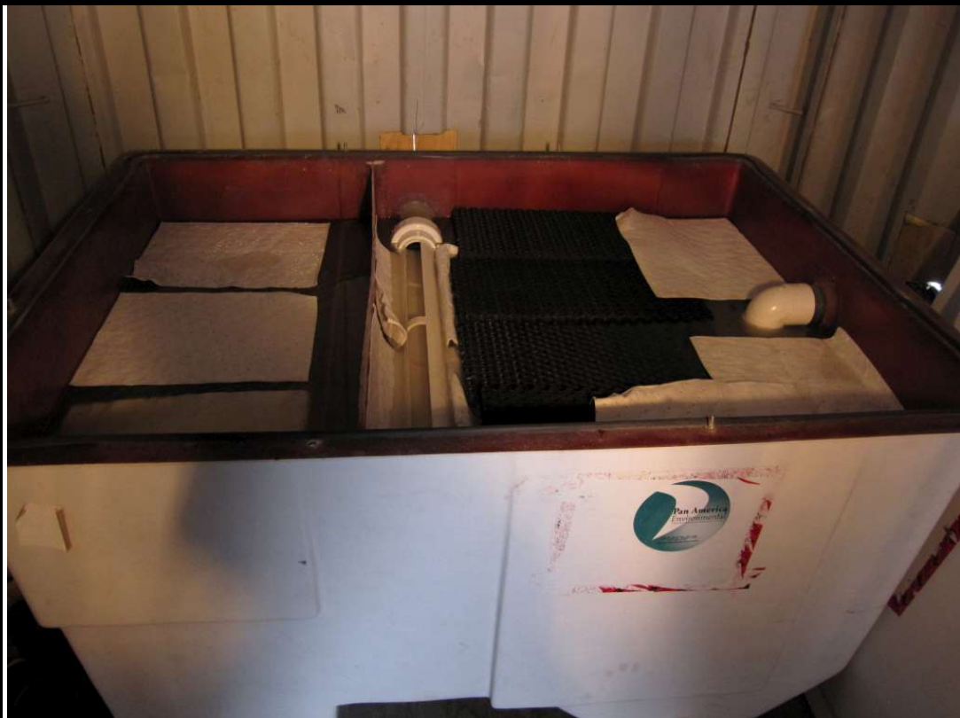
Photo No 12: Absorbents pads placed in the oil separator to help the contamination recovery.
