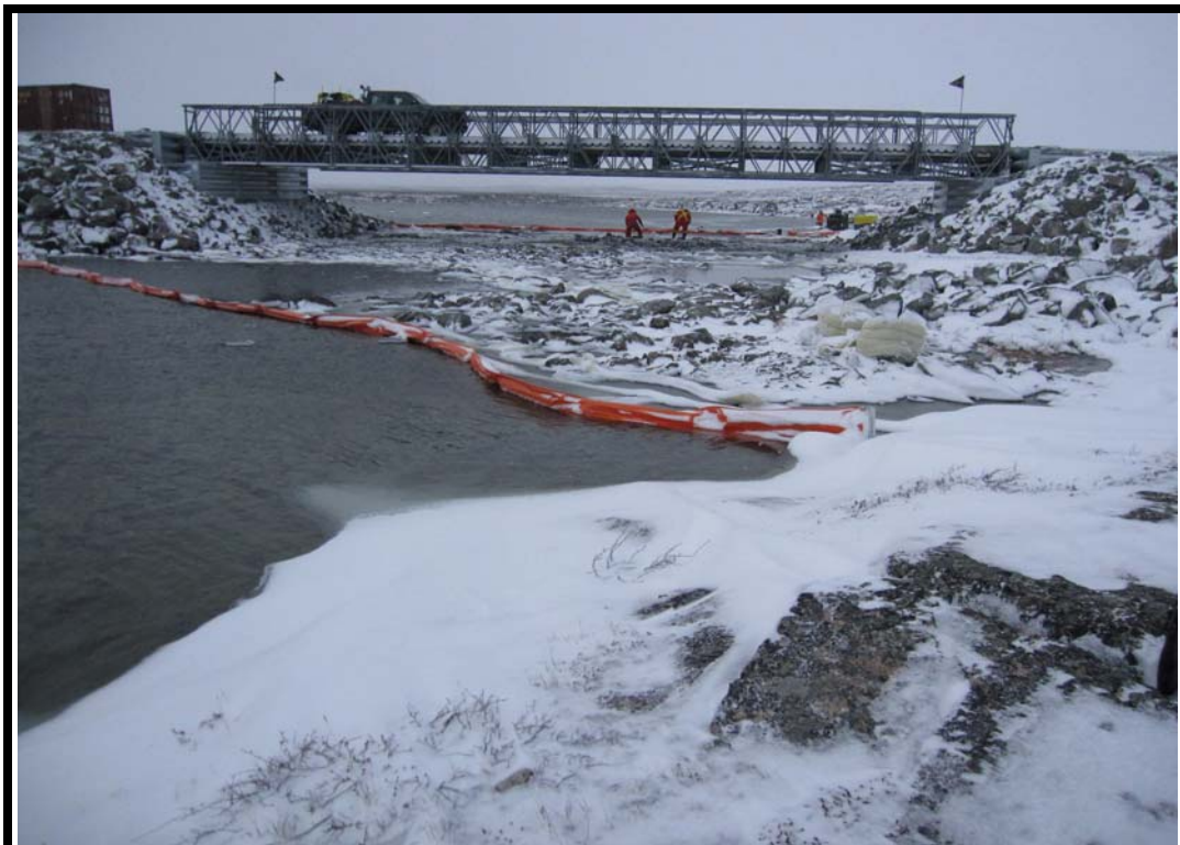
Photo No 7 : Maritime barriers were installed under the bridge.
