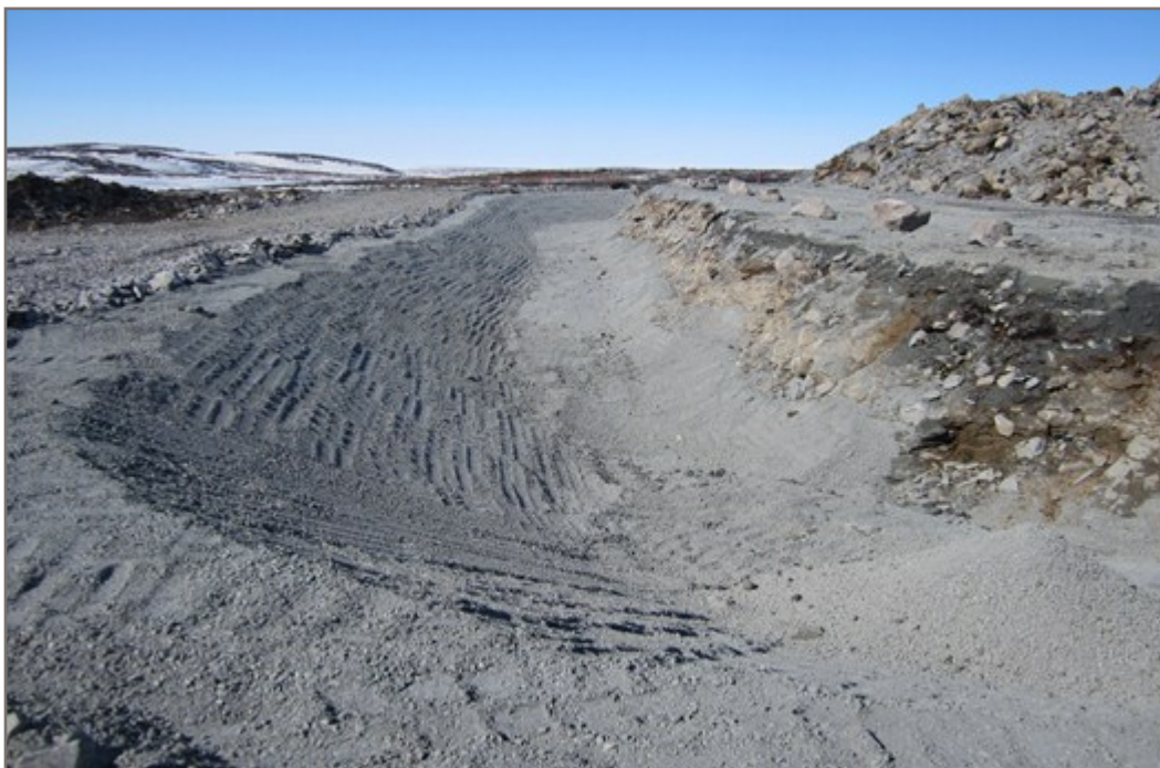
Photo 16: West End of Interception Trench Facing Northwest Completed Bentonite Placement
