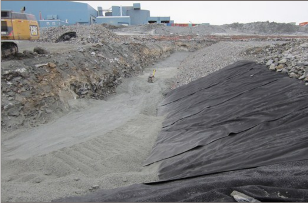
Photo 11: East End of Interception Trench Facing Northeast Geotextile Placement with Overlap and Tie-in at Top
