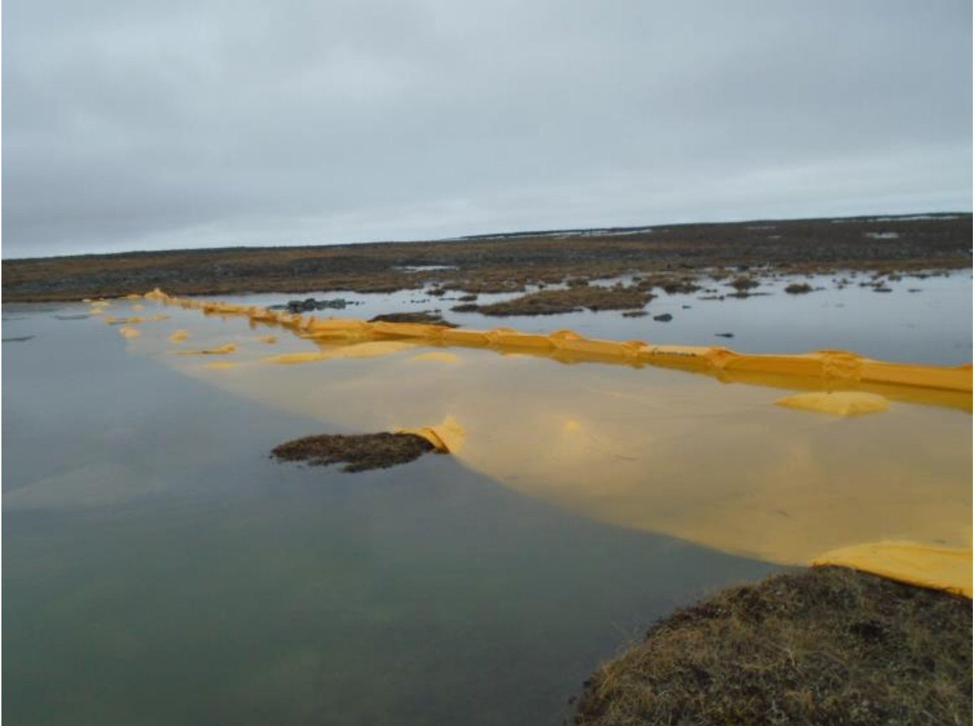
Photo 3: Turbidity barrier #3 at the outlet of NP-1 Lake
