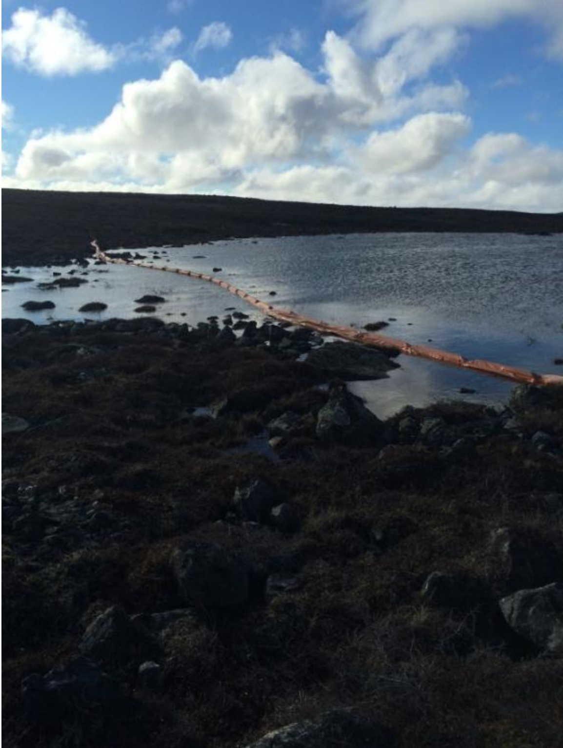
Photo 4: Turbidity barrier #4 at the inlet of Dogleg
